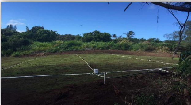
Above: Grass Stabilizing the Final Restored Site, June 2016
