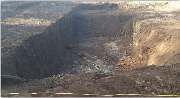
Above: Limits of Excavation in Deep Contaminated Area, April 2016
