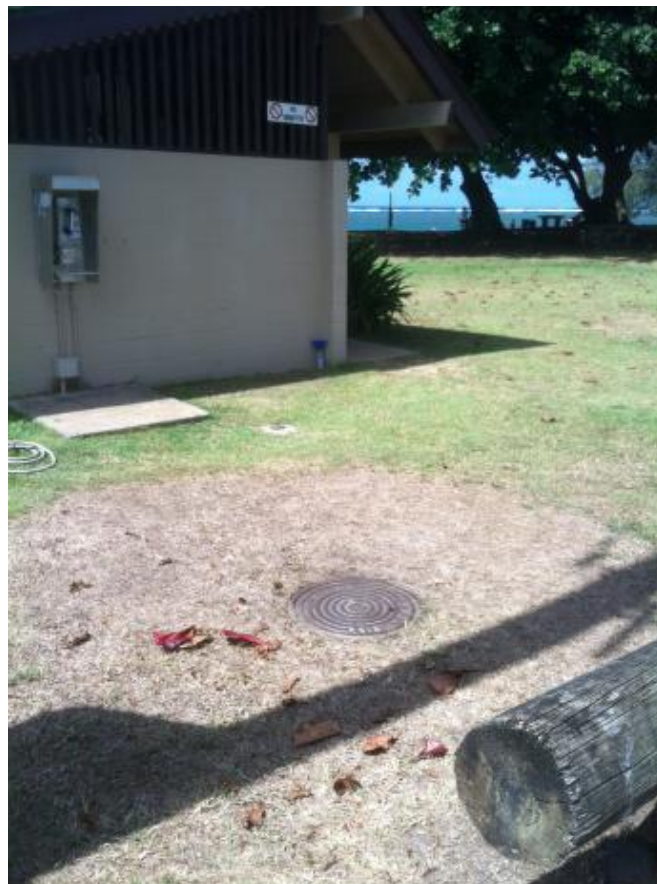
Fig. 21, The burnt outline of a cesspool cover. Possibly caused by overflow due to excessive water usage and a high water table.
