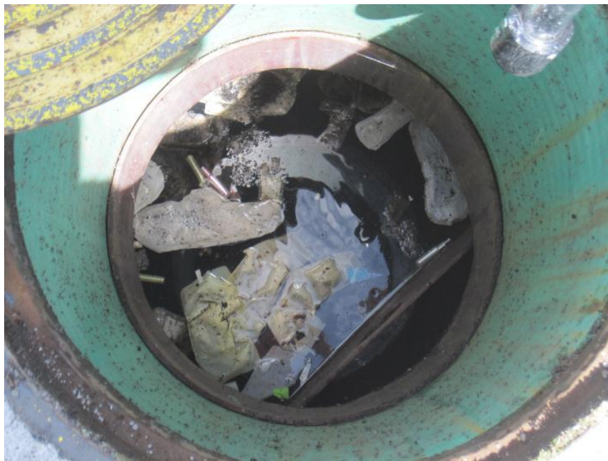
Fig. 27, A septic tank with feminine hygiene products that could potentially compromise the OSDS.
