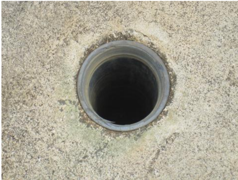
Fig. 20, An exposed cover of a failing cesspool creates a hazardous situation.
