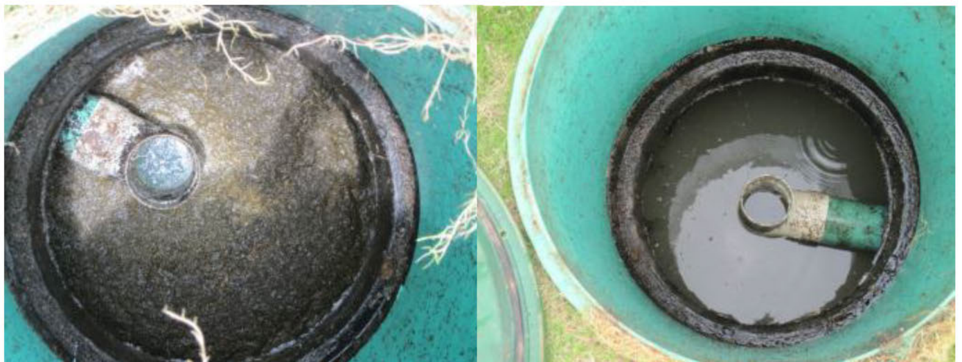
Fig. 12 and 13, Septic tank inlet and outlet compartments respectively. Both pictures are from the same system.
