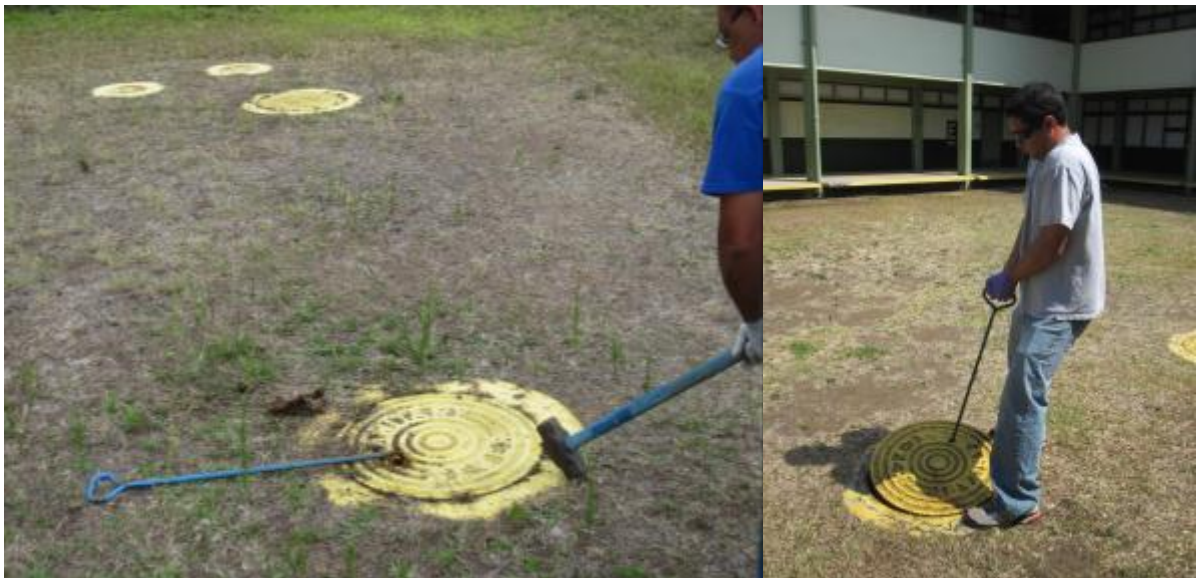
Fig. 6 and 7, Manhole covers being removed in order to conduct a system assessment.
