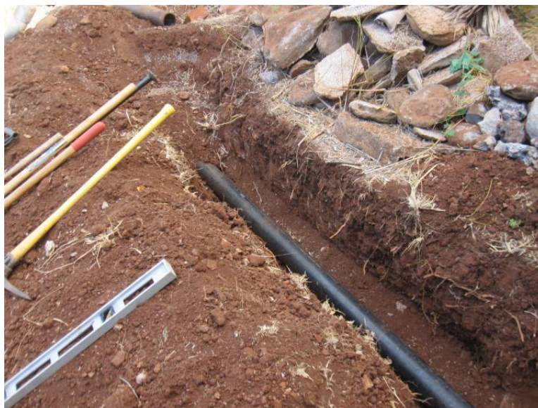
Fig. 31, A damaged sewer line leading to an OSDS that caused plumbing to back up. The septic tank was working properly once this problem was addressed.
