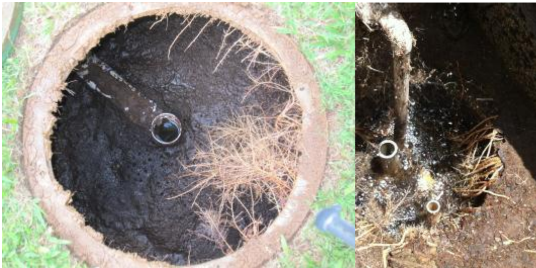
Fig. 19 and 20, Both pictures are failing ATU systems with root intrusion from outside plants.
