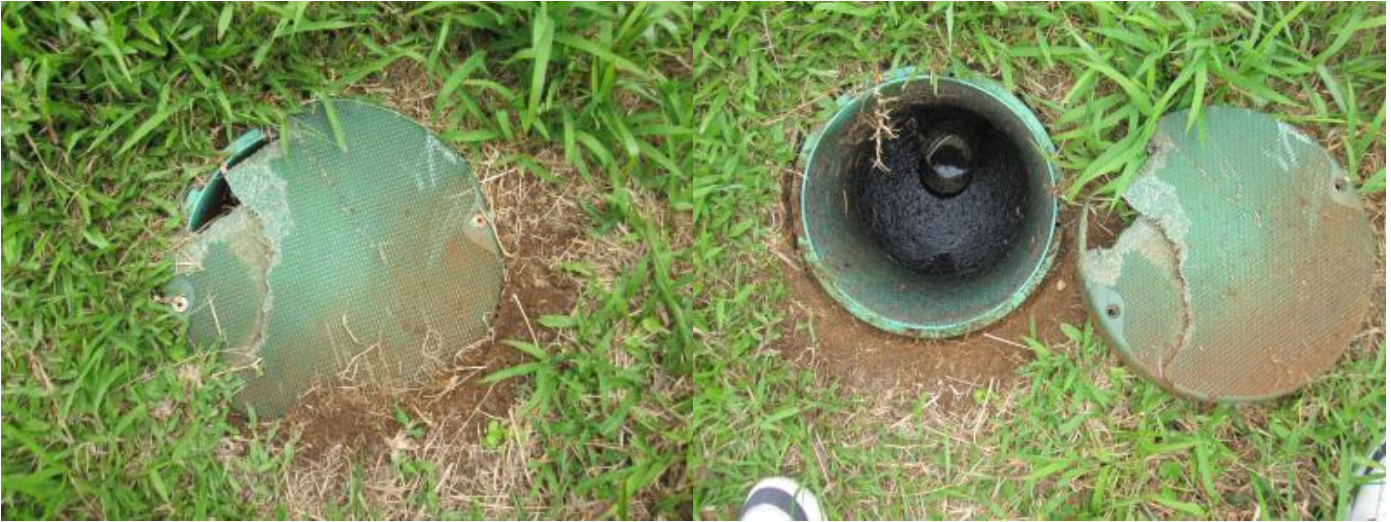
Fig. 25 and 26, A septic tank cover is damaged. This allows storm run-off and sediment to enter and overload the system.
