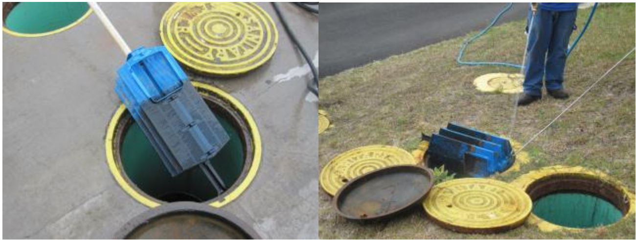
Fig. 8 and 9, Workers from a Big Island septic pumping company perform routine maintenance by cleaning effluent screens.
