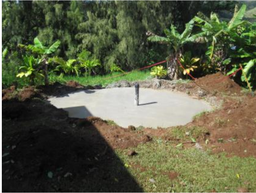
Fig. 22, A recently repaired cesspool cover that had previously collapsed.
