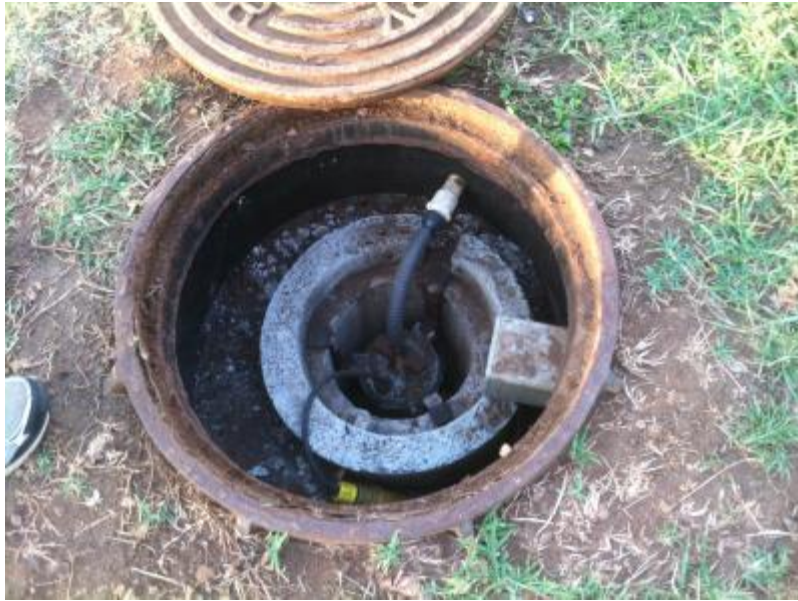
Fig. 18, A failing ATU unit that has no signs of operation. Air compressor was cold and wiring was corroded.
