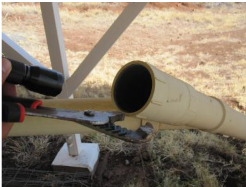
Fig. 10, Inspection ports provide an access point for OSDS assessments in which manhole covers cannot be located.
