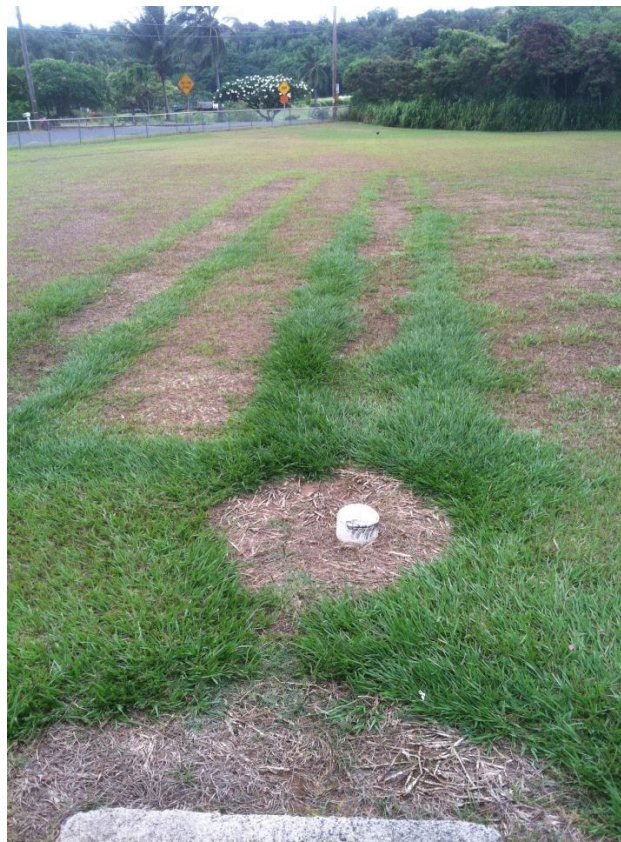
Fig. 30, A drainfield with abnormally lush vegetation . This OSDS is located adjacent to a river. A high water table may have contributed to this situation.
