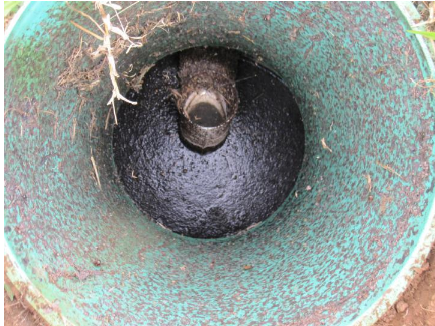
Fig. 29, High water markings from a septic tank. This indicates that an overflow has happened in the past.
