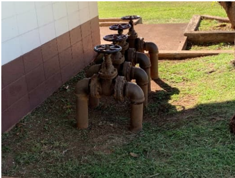
Photograph 39: Irrigation Valves
