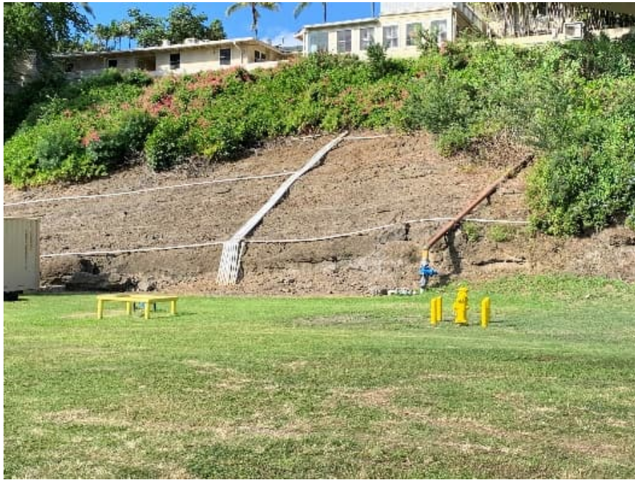
Photograph 48: Service Connection Area
