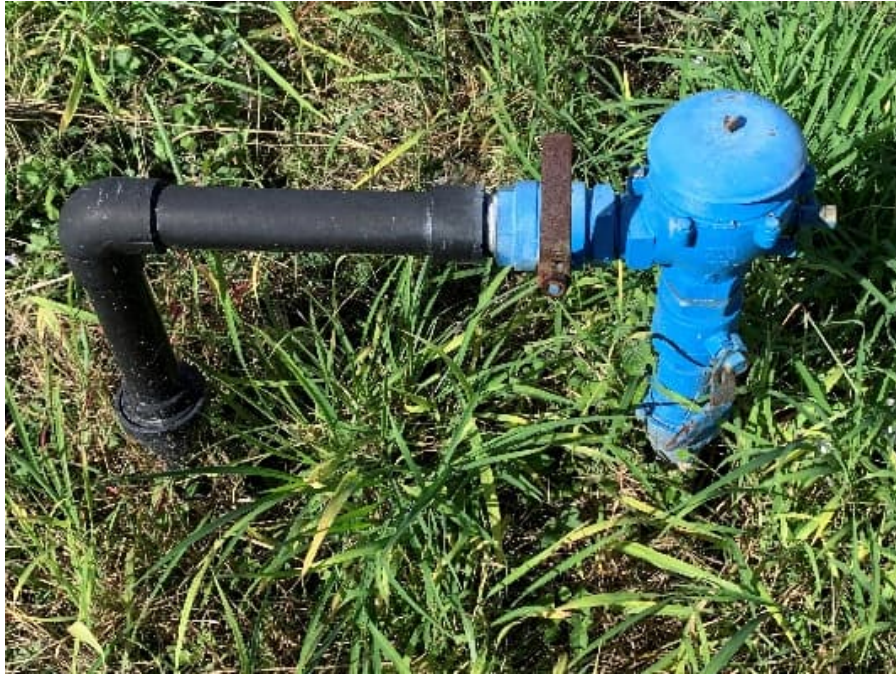
Photograph 53: Backflow Preventer
