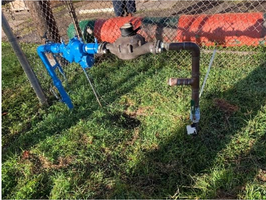
Photograph 3: Backflow Preventer
