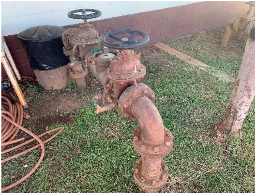
Photograph 38: Backflow Preventer
