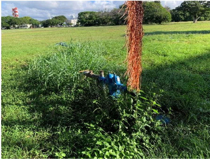
Photograph 9: Backflow Preventer
