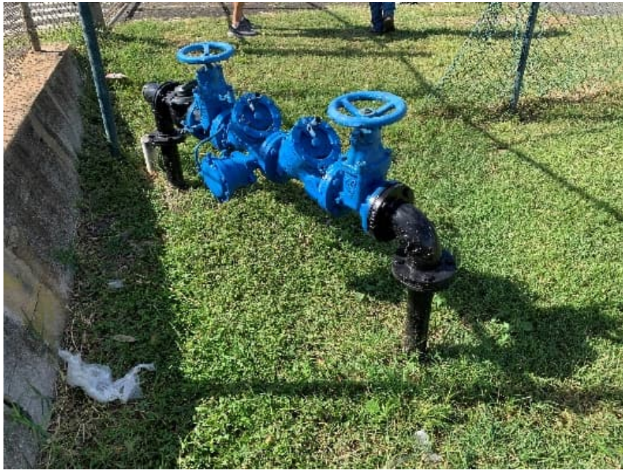
Photograph 65: Backflow Preventer
