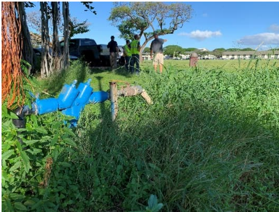
Photograph 10: Backflow Preventer
