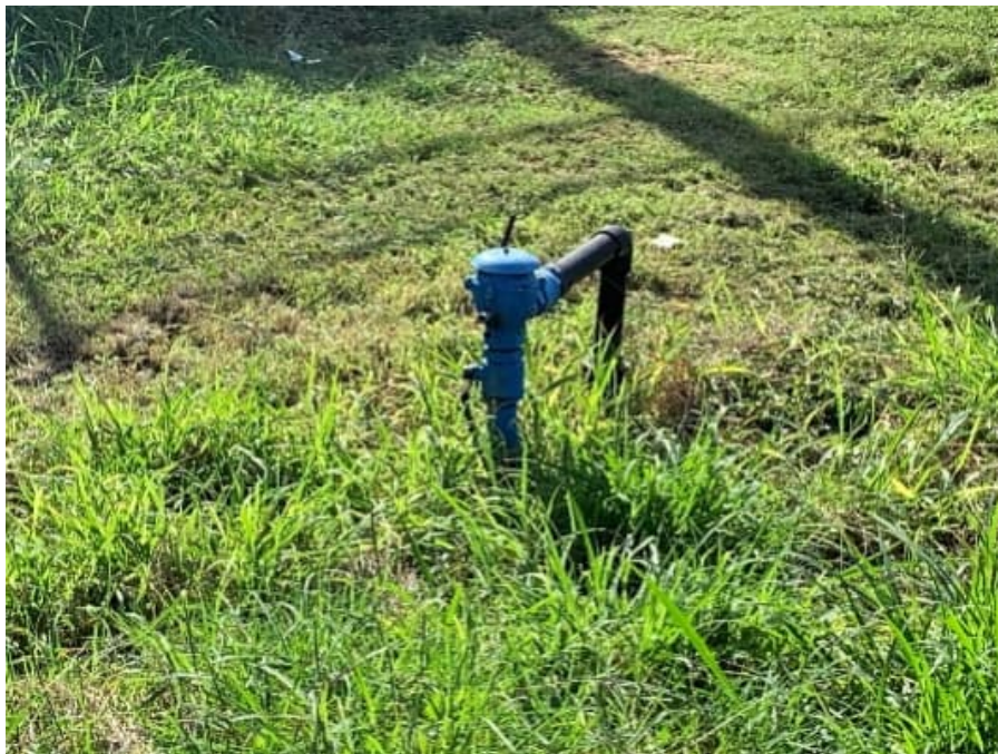
Photograph 52: Backflow Preventer
