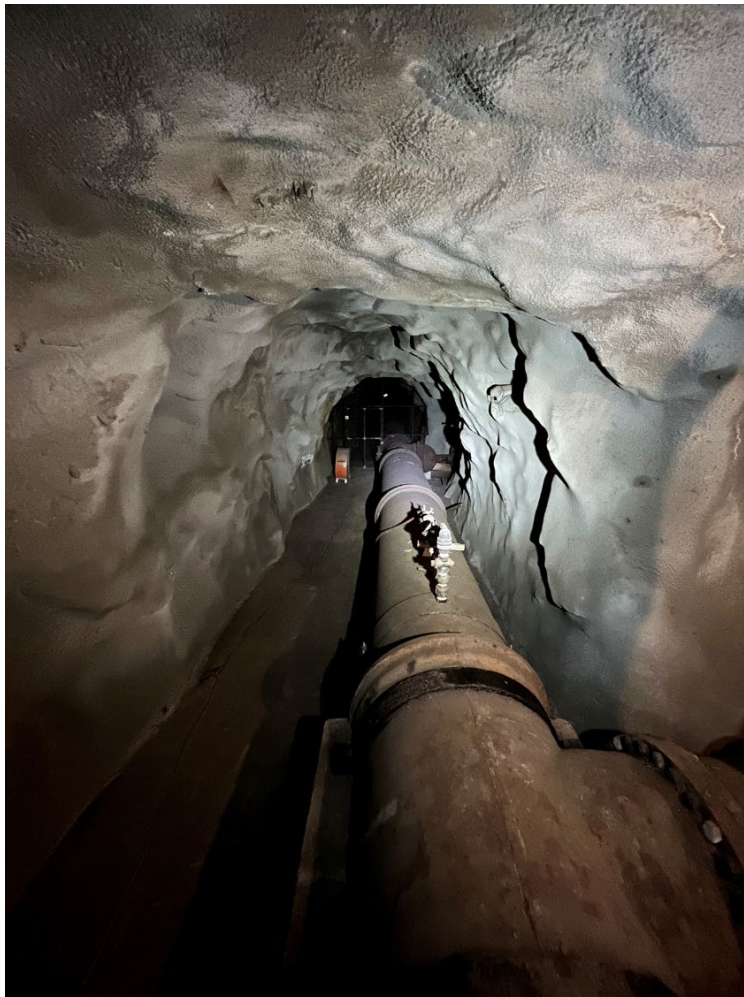
Figure 2-6. Photo of Moanalua Tunnel
