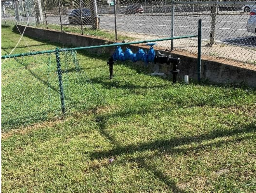
Photograph 61: Backflow Preventer
