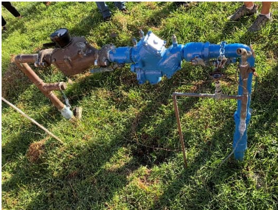
Photograph 6: Backflow Preventer
