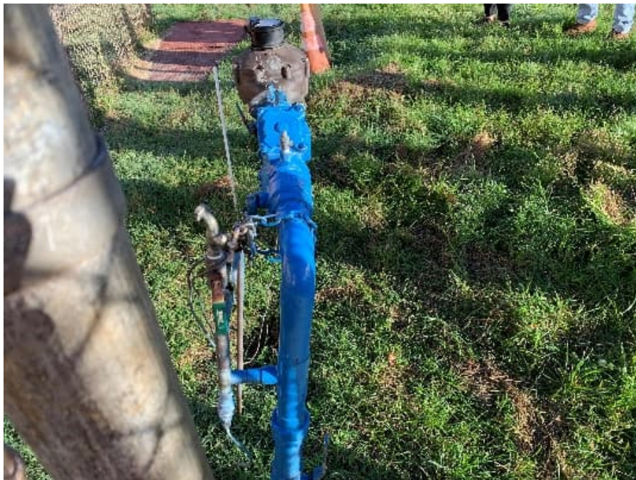
Photograph 4: Backflow Preventer
