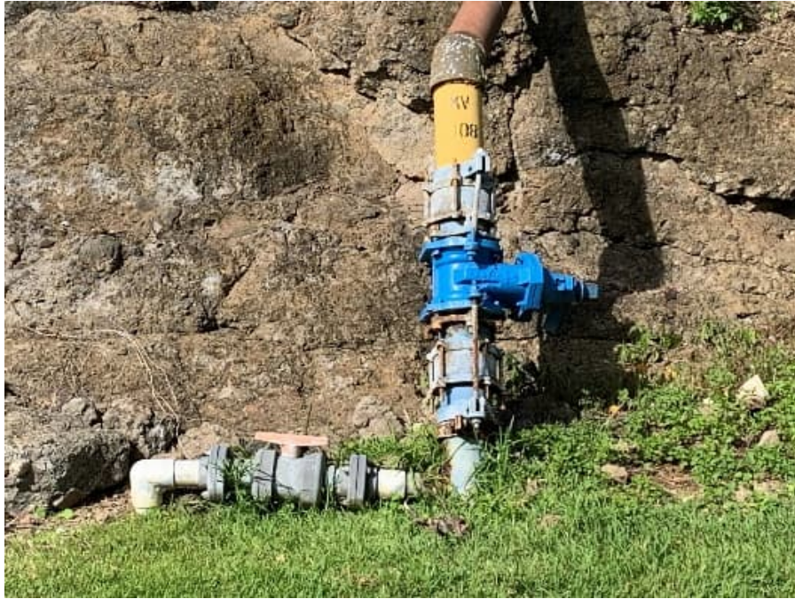
Photograph 42: Existing Service Connection
