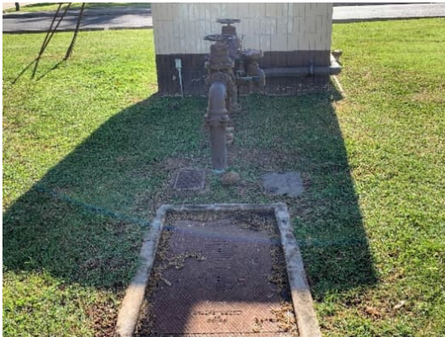
Photograph 29: Backflow Preventer
