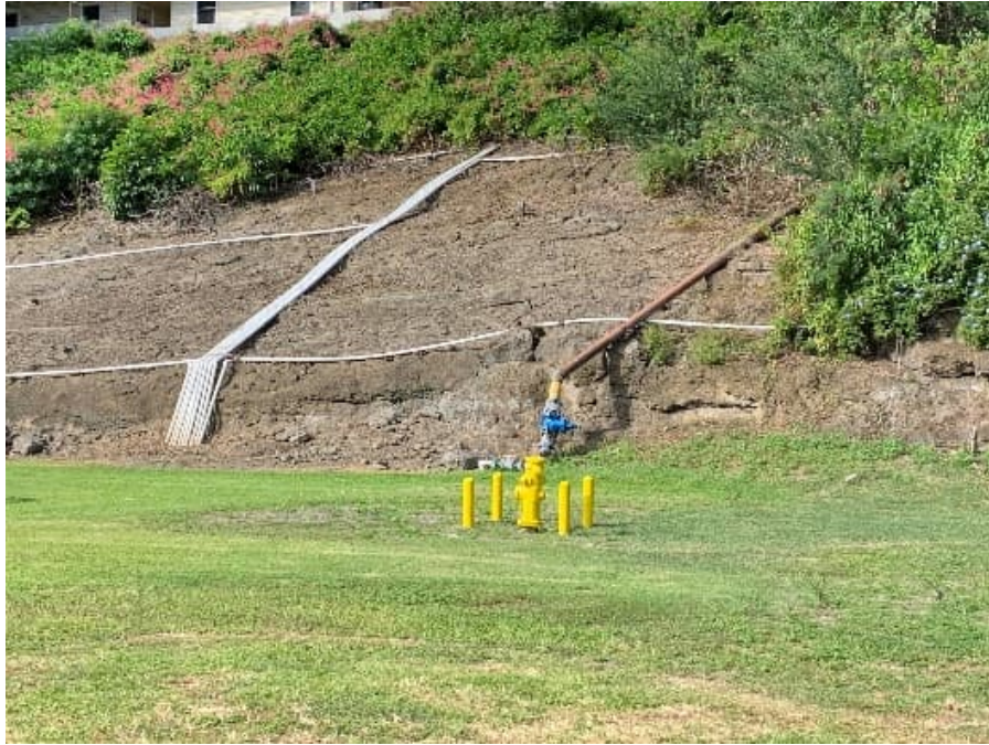
Photograph 40: Existing Service Connection
