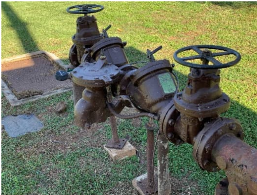
Photograph 33: Backflow Preventer
