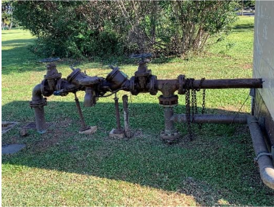
Photograph 28: Backflow Preventer
