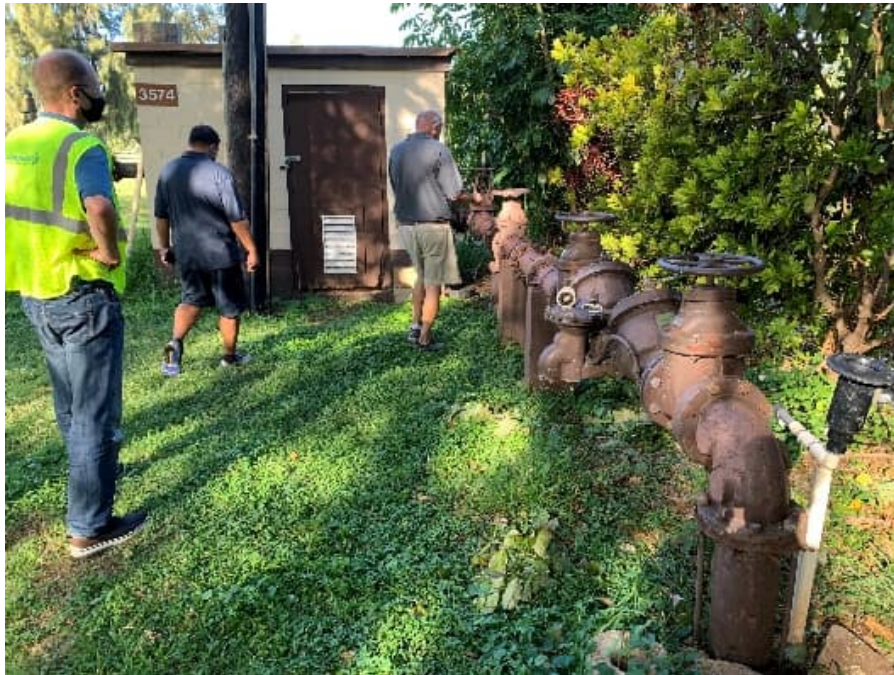
Photograph 20: Backflow Preventer
