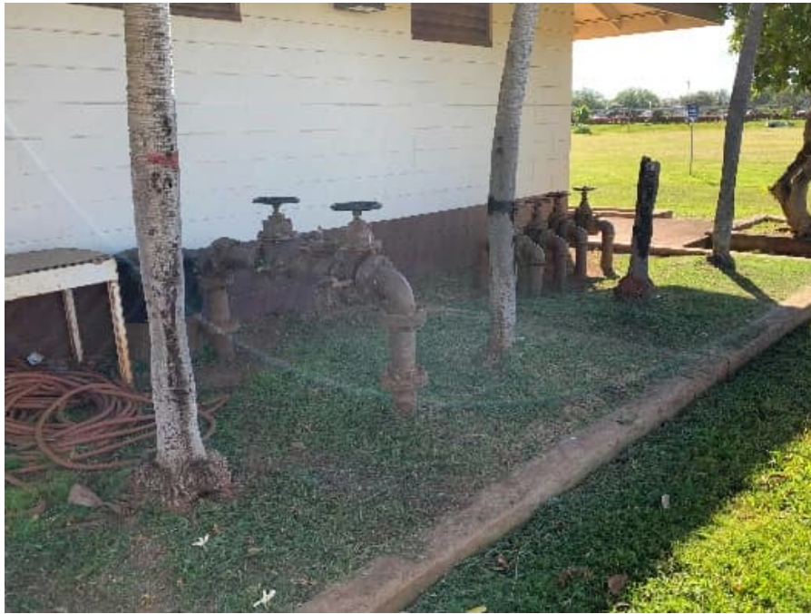
Photograph 36: Backflow Preventer
