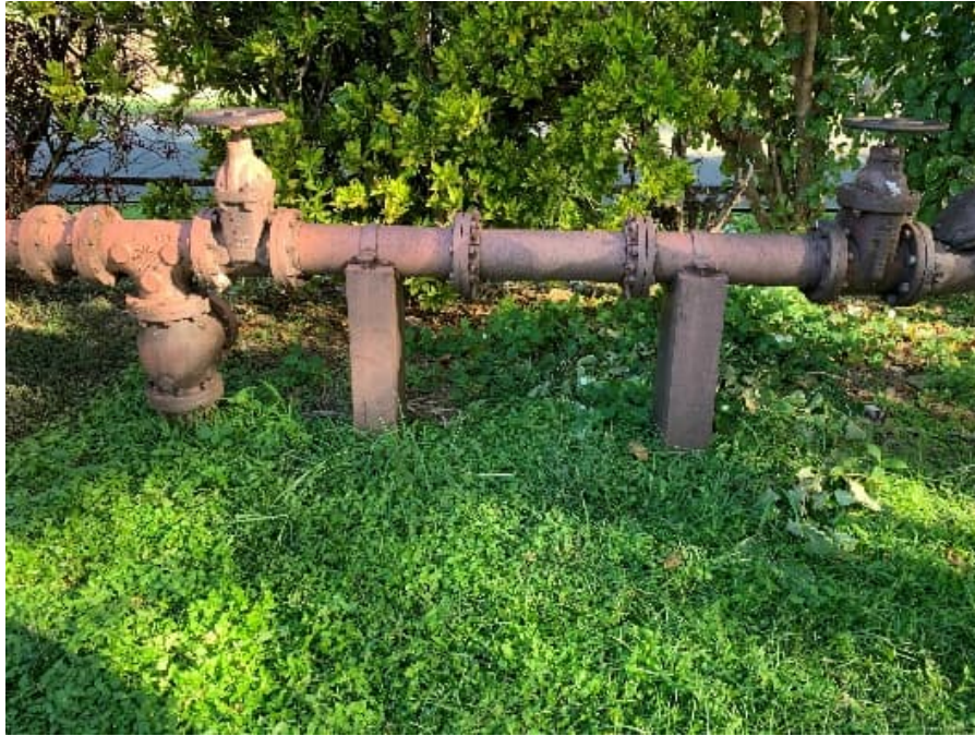
Photograph 22: Backflow Preventer
