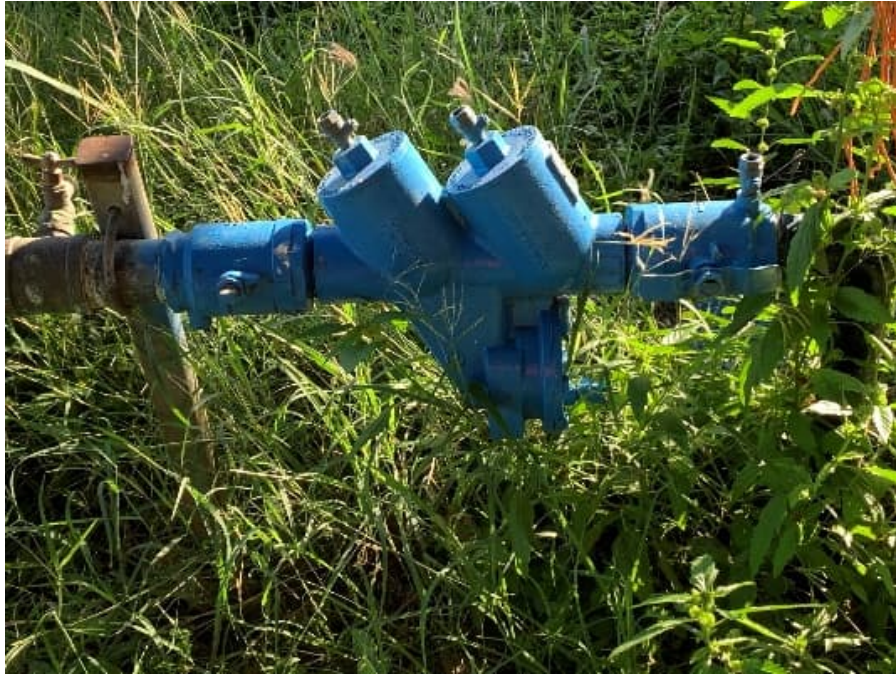
Photograph 13: Backflow Preventer
