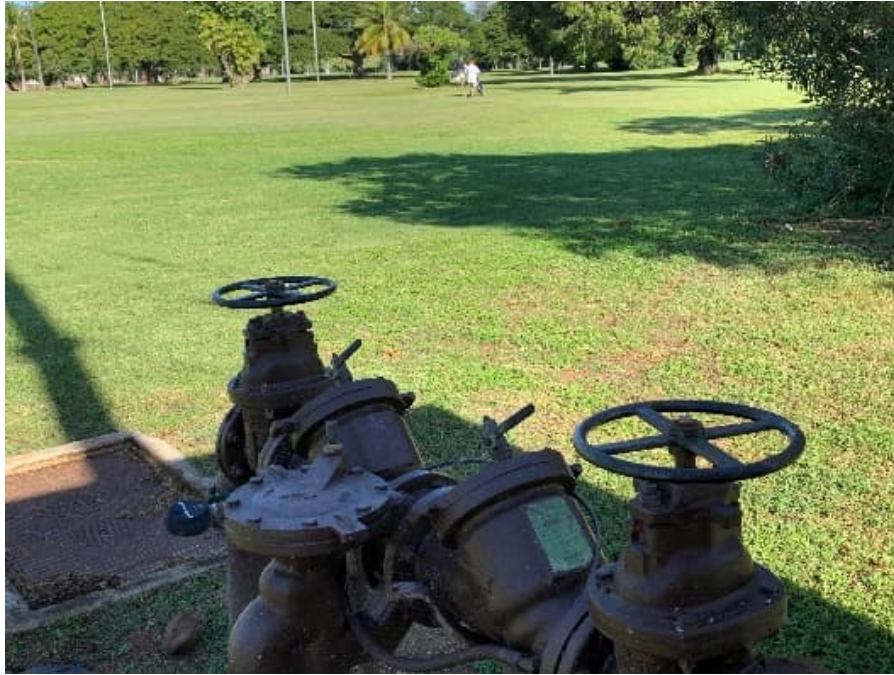
Photograph 34: Backflow Preventer
