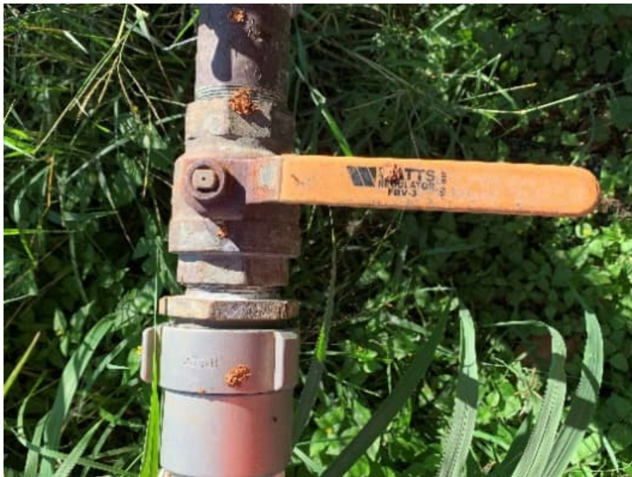
Photograph 12: Backflow Preventer
