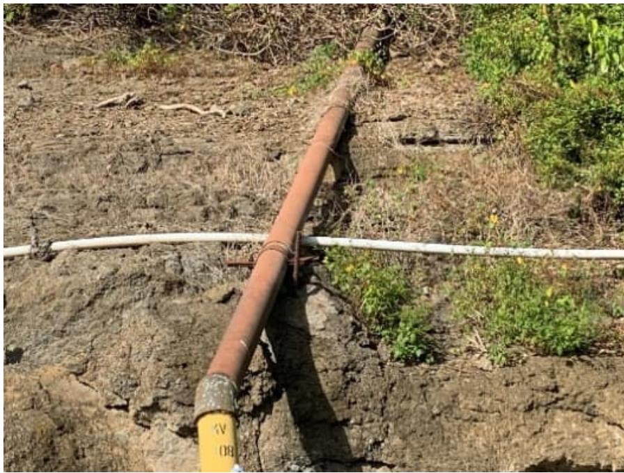
Photograph 43: Existing Main along Hillside
