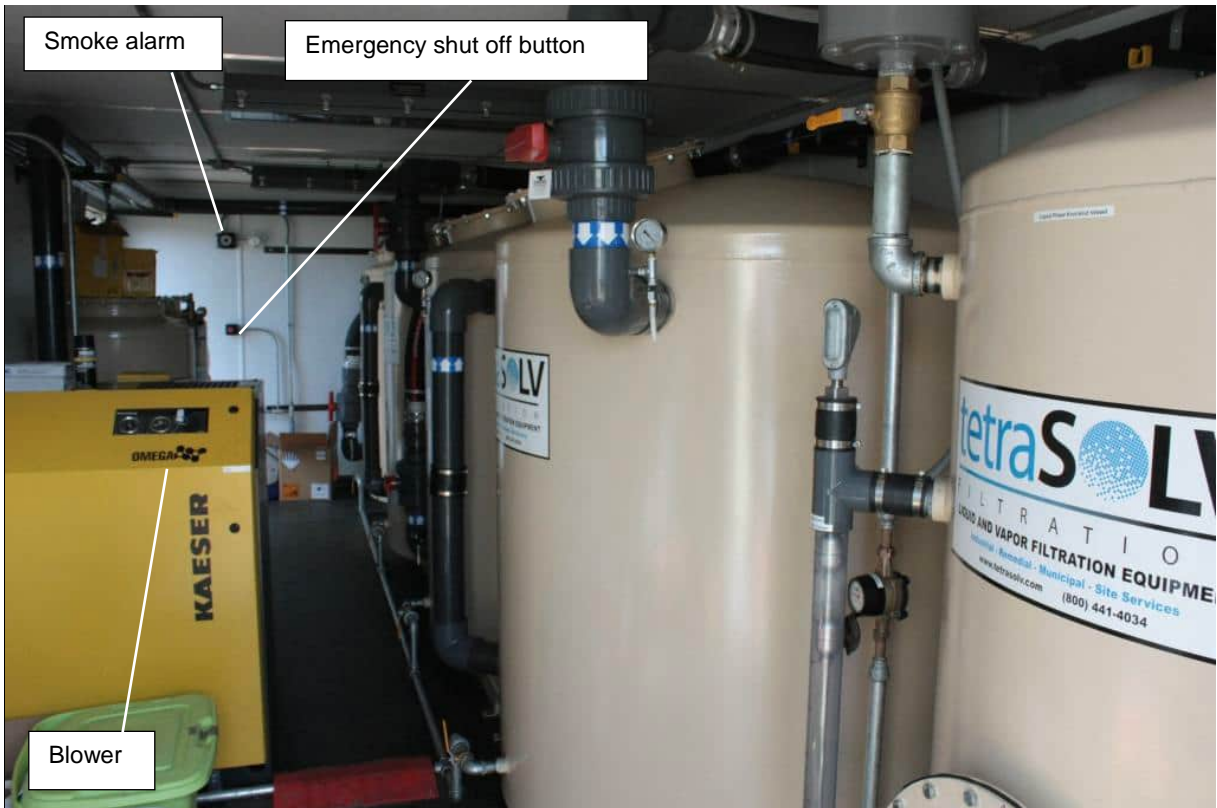
Photo 6. Inside of the treatment room
