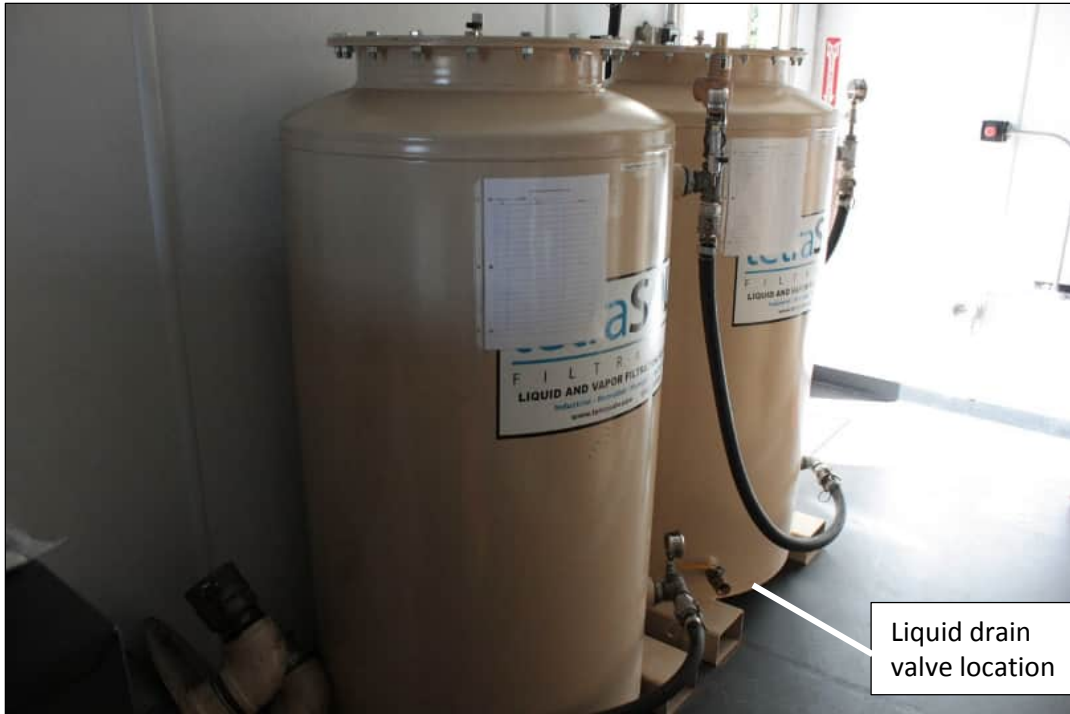
Photo 6. Valve location on an LGAC train vessel used to drain liquid before LGAC changeout.
