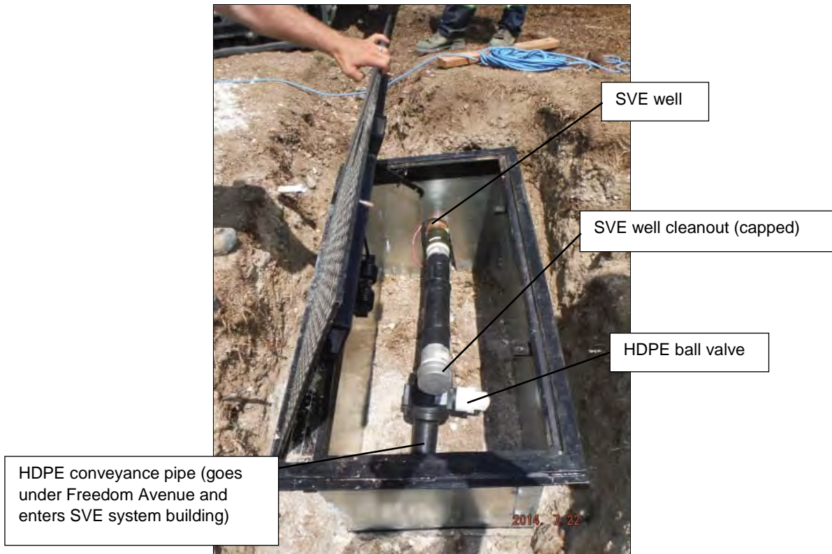
Photo 13. View inside a SVE well vault during installation
