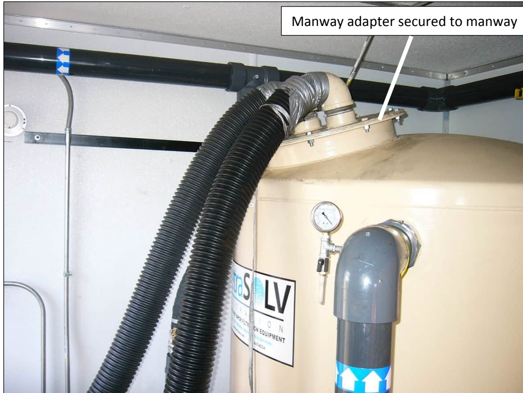
Photo 4. Manway adapter secured onto GAC vessel and flexible hose attached during refill of vessel with fresh GAC.
