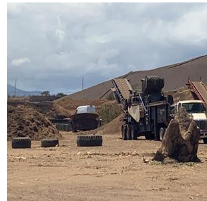
Figure 4-4. Central Maui Landfill Organics Processing Area
