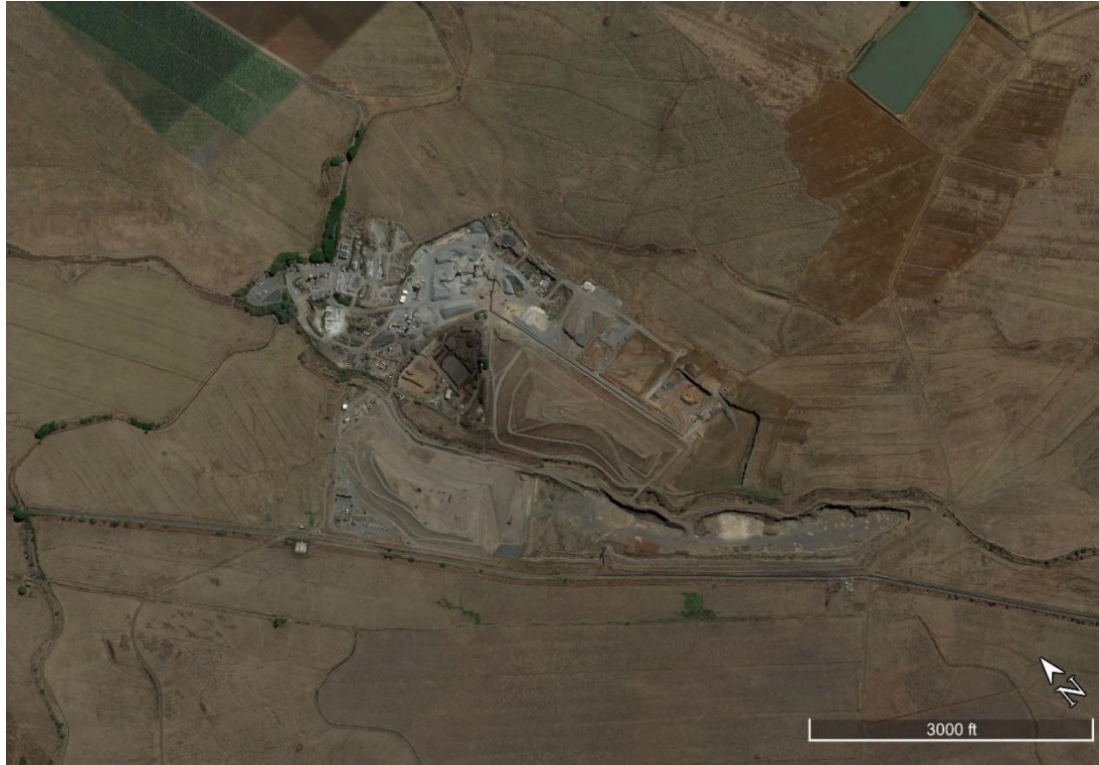
Figure 9-2. Central Maui Landfill
