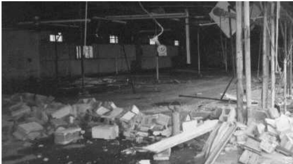
Figure 5: Building Demolition Waste
