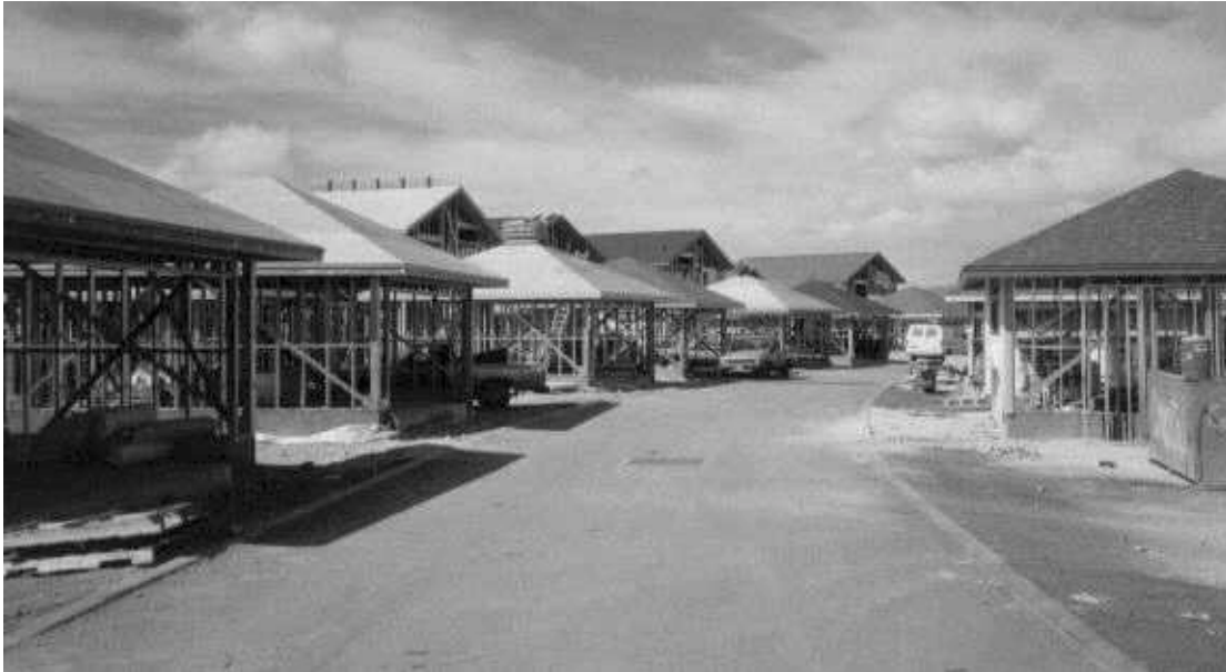
Figures 8a and 8b: Steel Construction
