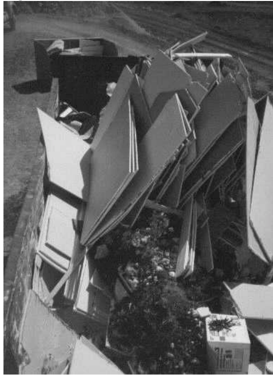
Figure 7: Construction Site Dumpster
