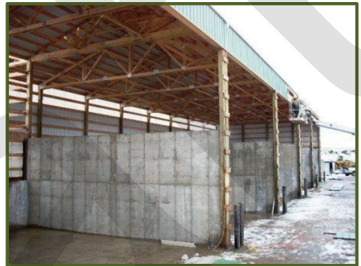
Bunker with roof (Latah Co., ID)
