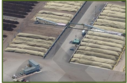
Membrane-covered system (Everett, WA)
