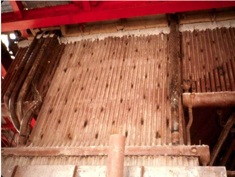
Figure 12-1 - Waterwall Furnace Section 1
