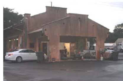
Photo 5-8. Collection base yard in Wailuku has one small office.
