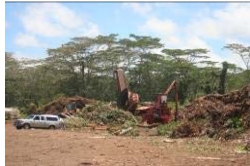
Photo 9-8. EKO grinding at the Hilo Landfill
