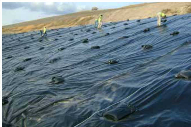
Temporary Rain Shed Cover
