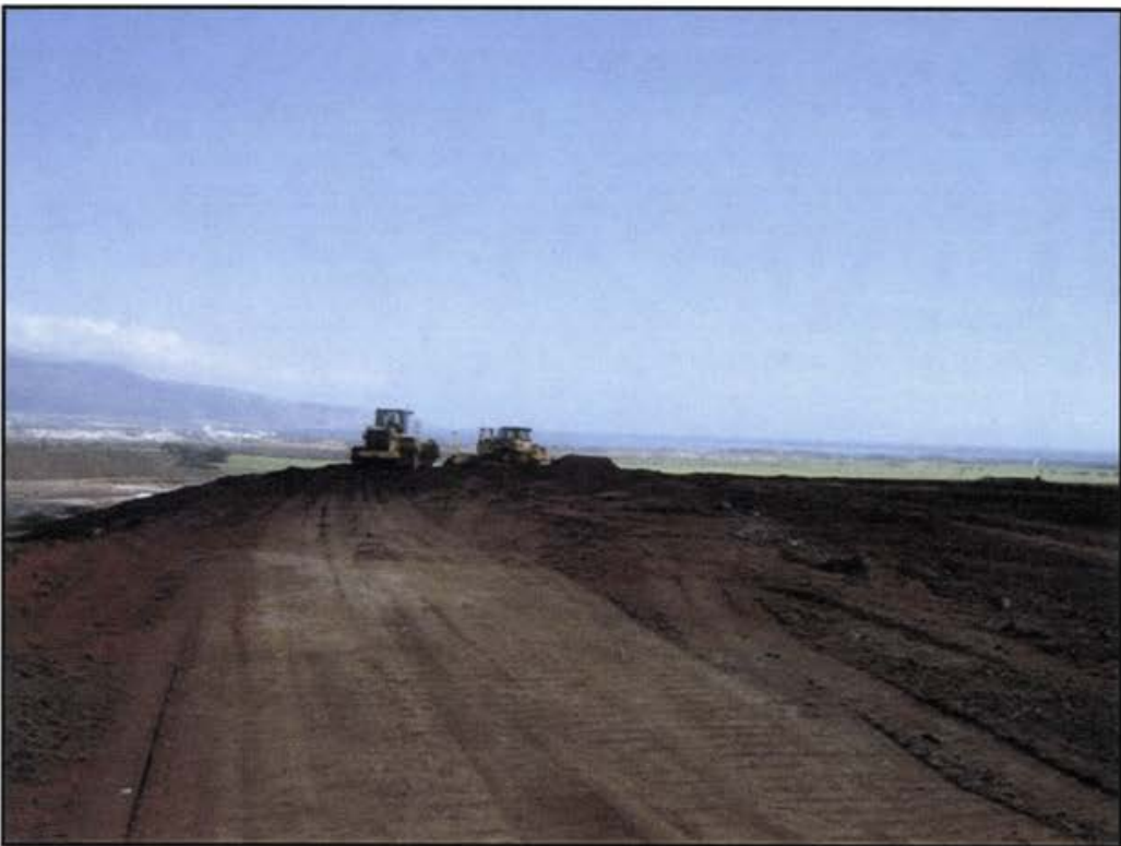
Photo 14 Grading and compaction of MFC soils on the top deck of the landfill
