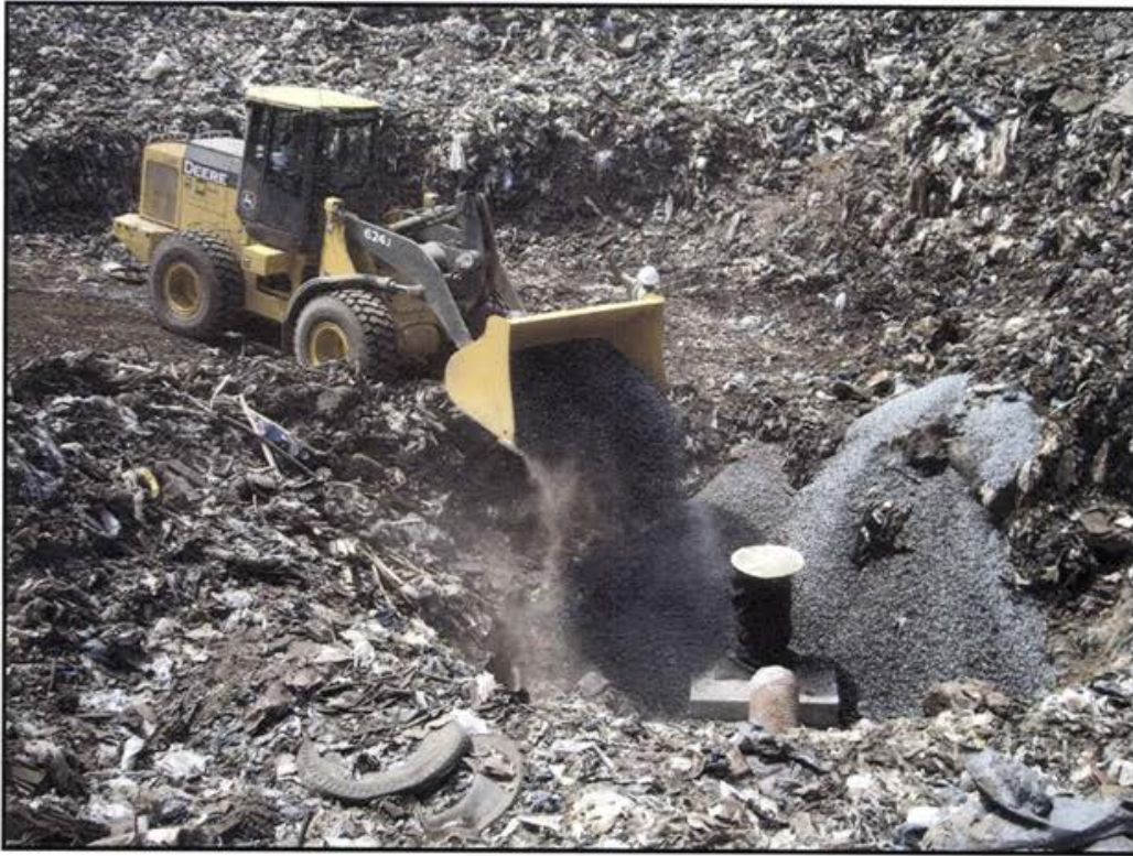
Photo 3 Placement of drainage rock backfill around 18-inch HDPE vertical inlet pipe.
