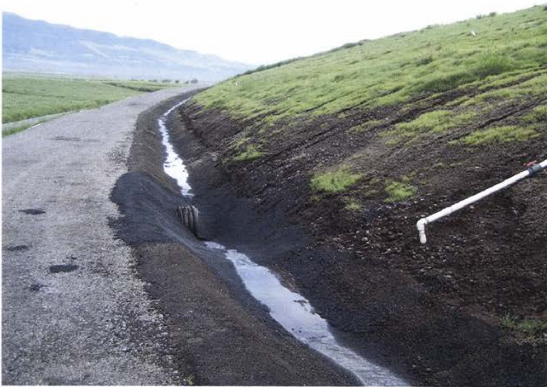
Photo 24 Inlet to overseide drain from mid-slope bench asphalt V-Ditch
