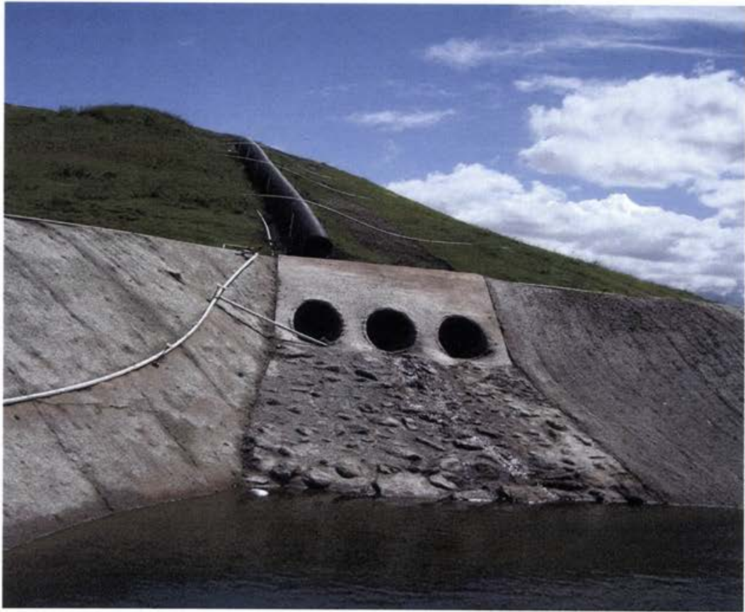
Photo 29 Main drainage discharge to stilling basin
