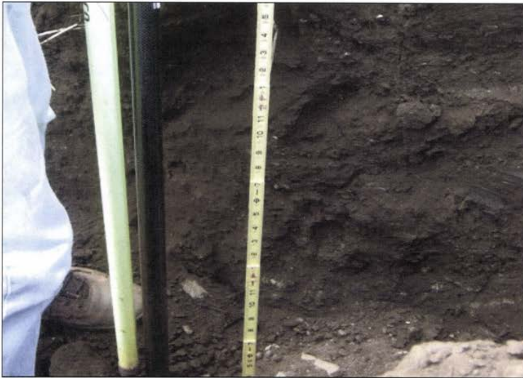
Photo 19 Measuring thickness of Monolithic Final Cover (MFC) at test pit location.
