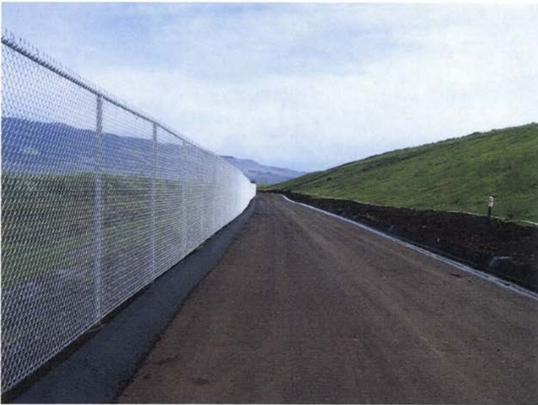
Photo 26 East perimeter drainage road with curbs and reconstructed fence
