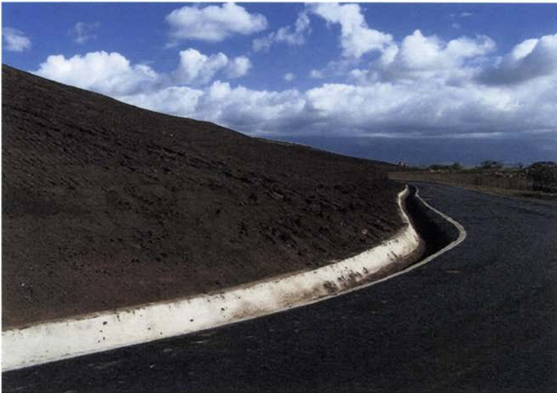
Photo 22 Completed concrete trapezoidal drainage channel along paved perimeter road.
