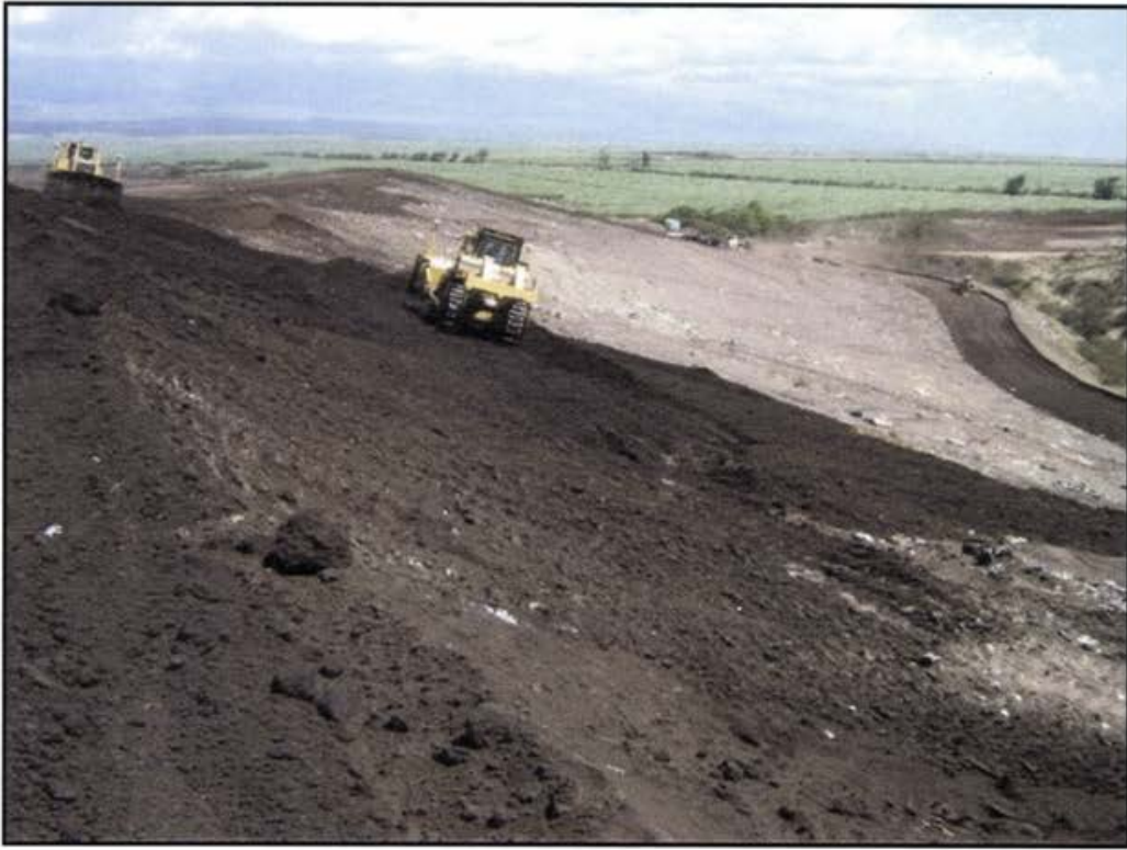
Photo 13 Placement and grading of MFC soils on upper portion of west slope.
