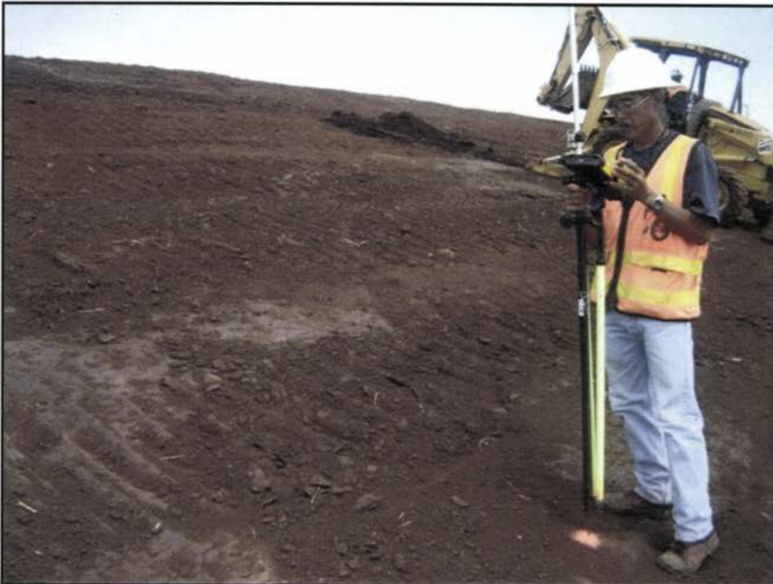
Photo 18 Surveying location of test pit for verification of Monolithic Final Cover (MFC) thickness.
