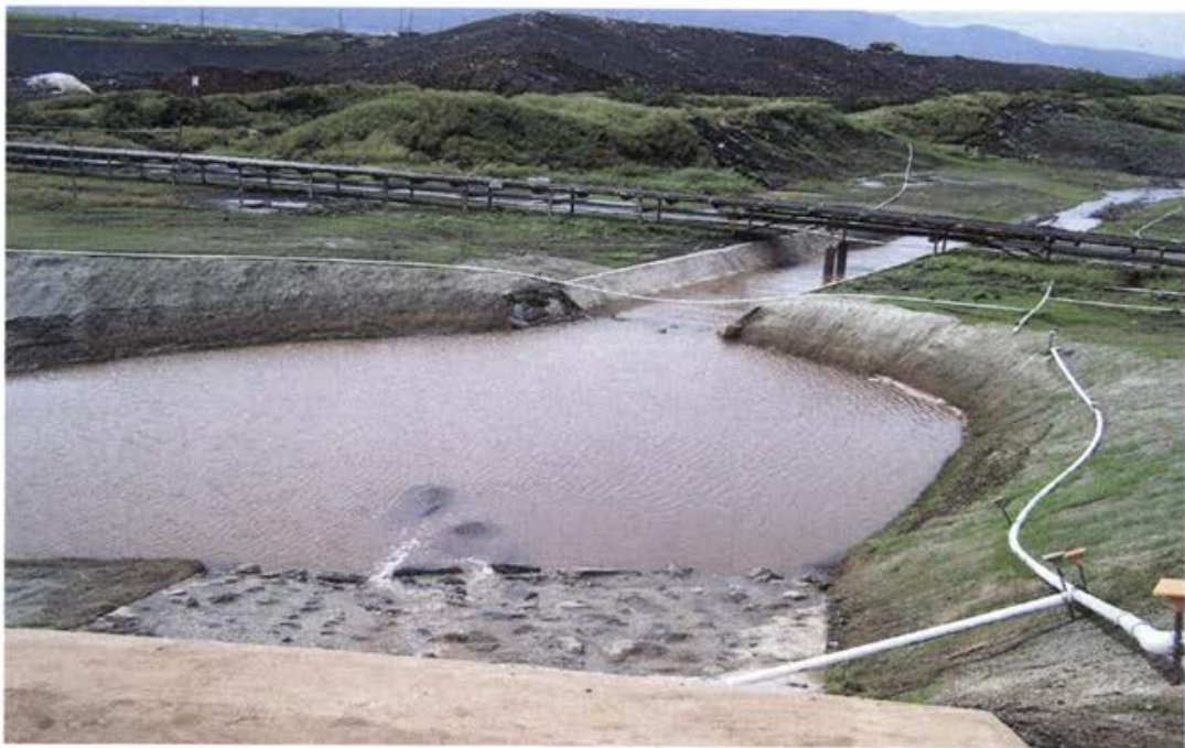
Photo 29 Main drainage discharge to stilling basin
