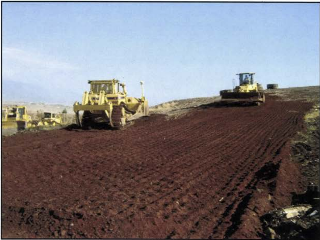
Photo 10 Grading and compacting of imported MFC soils.
