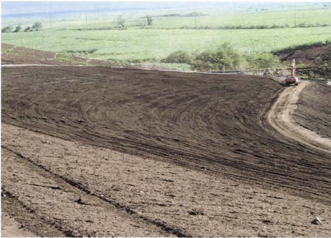
Photo 21 Completed MFC on upper portion of west slope.
