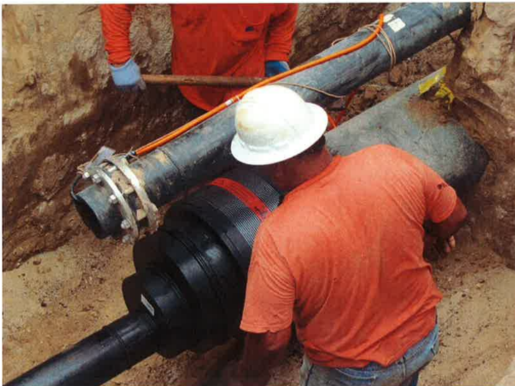
Photo 58. 18 inch HDPE reducing fitting to connect the existing system to the new Wet Well #1 assembly.
