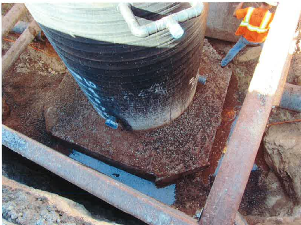
Photo 53. Wet Well #1 completed ballast system.
