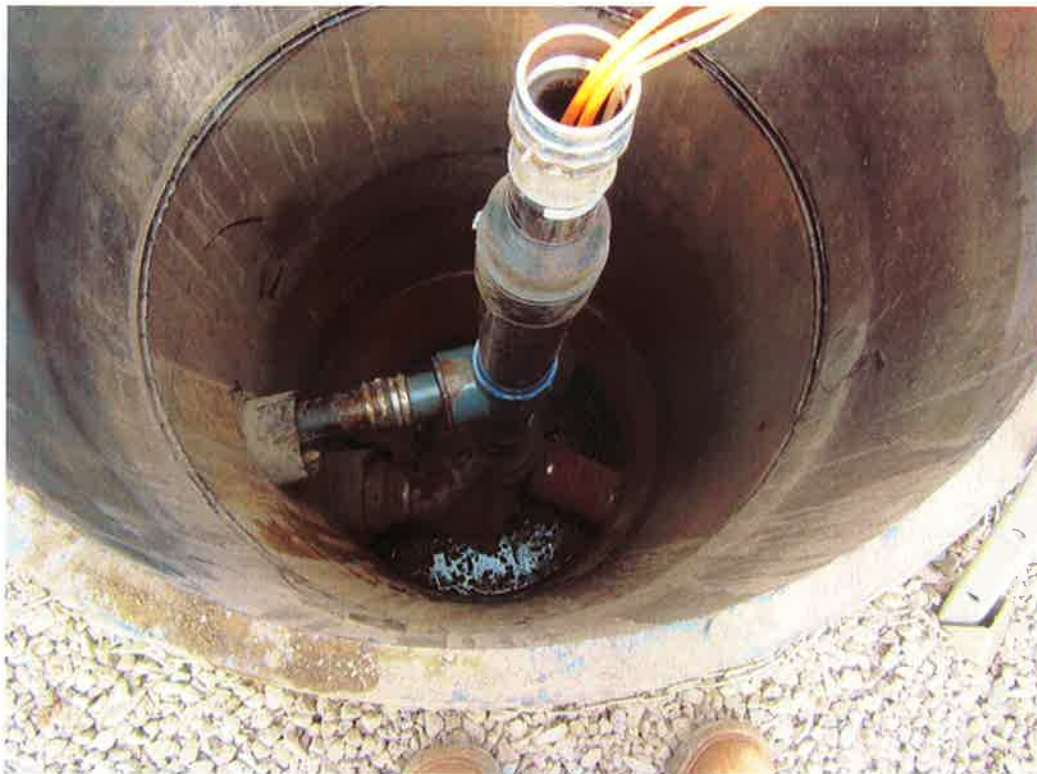
Photo 110. LCM 14 system installation in accordance with RFI 14r1.
