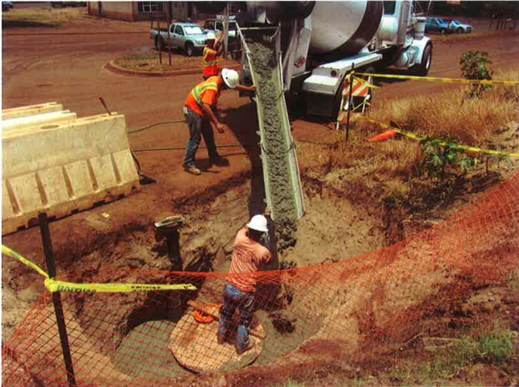
Photo 85. LCM 2-13 lean concrete foundation poured around LCM to support final cap (typical).
