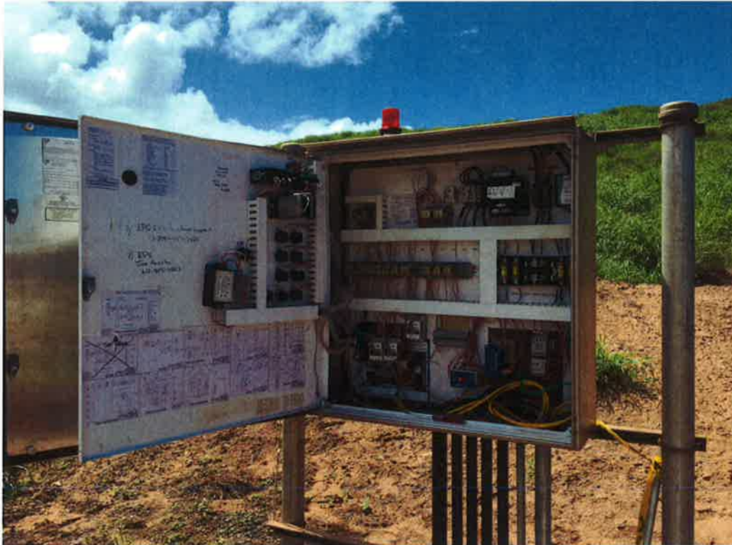
Photo 119. Interior of Wet Well #2 control panel for after full re-wiring in EPG's Minnesota shop (typical).
