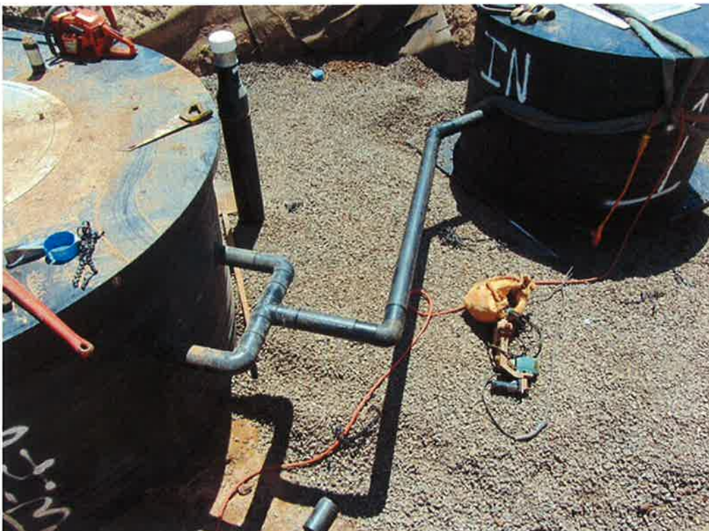
Photo 70. New 3-inch HDPE discharge piping, which connects the new Wet Well #1 assembly to the meter valve box.
