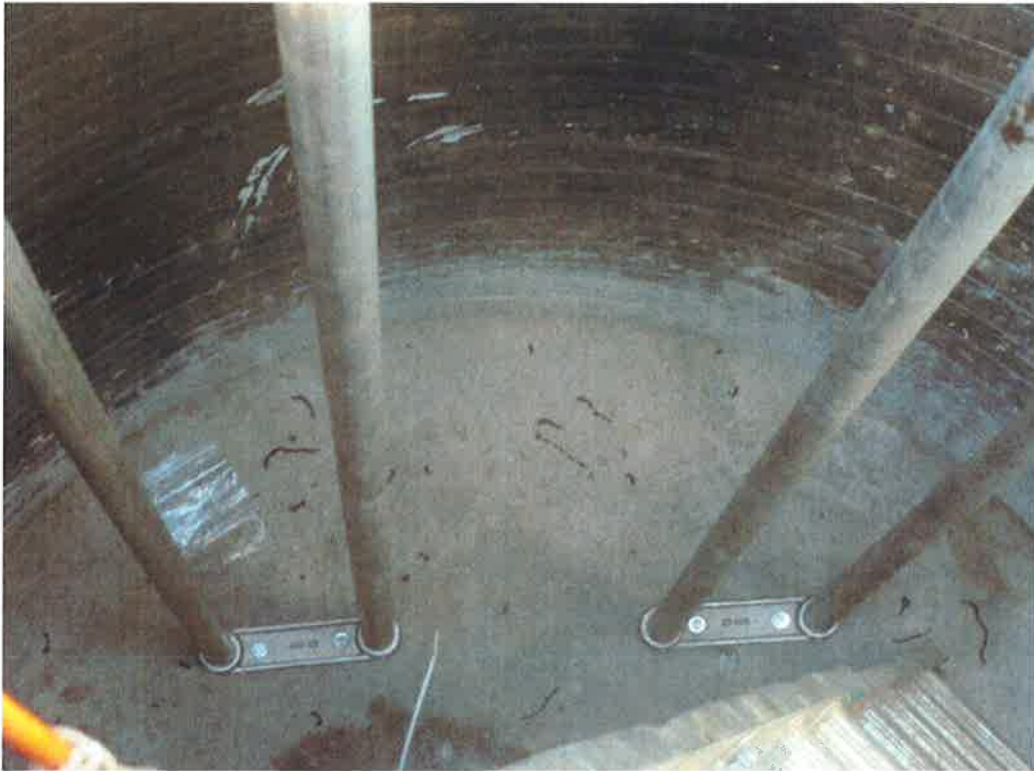
Photo 79. Wet Well #1 rail system support bolted to poured concrete floor (later removed)..
