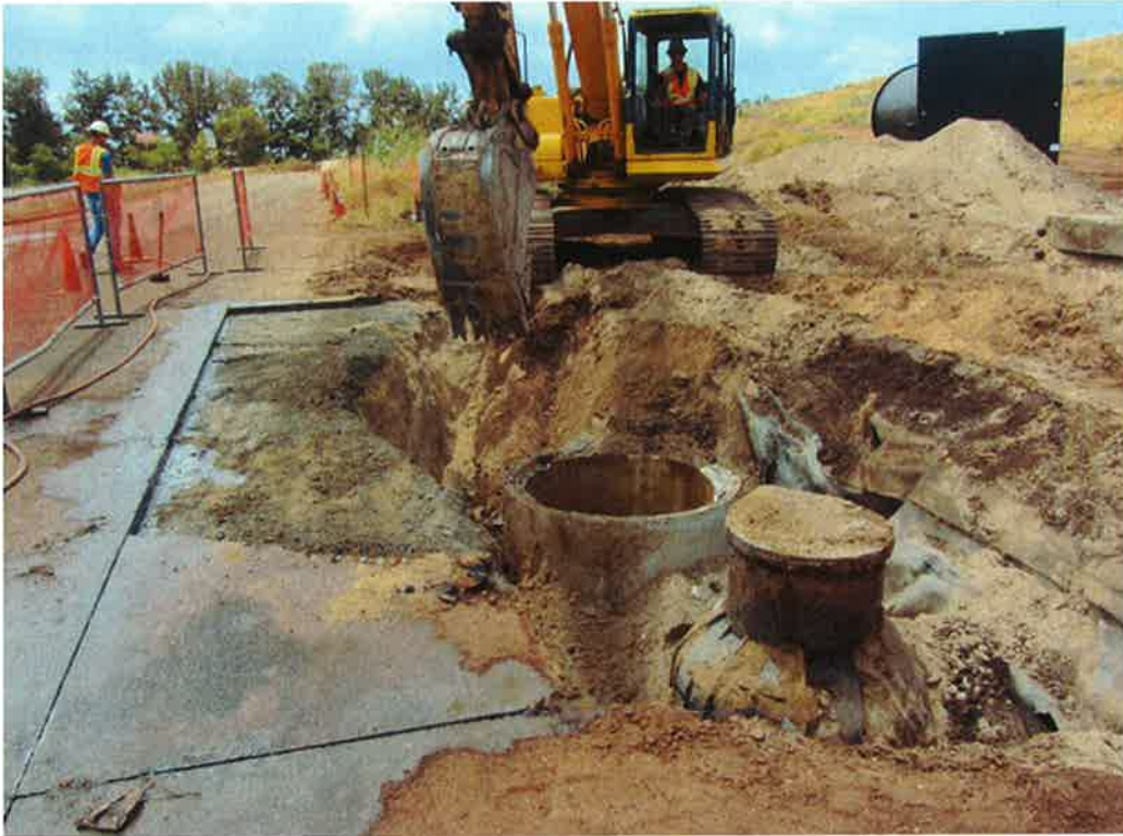
Photo 45. Excavation to remove the existing wet well and valve box assembly.
