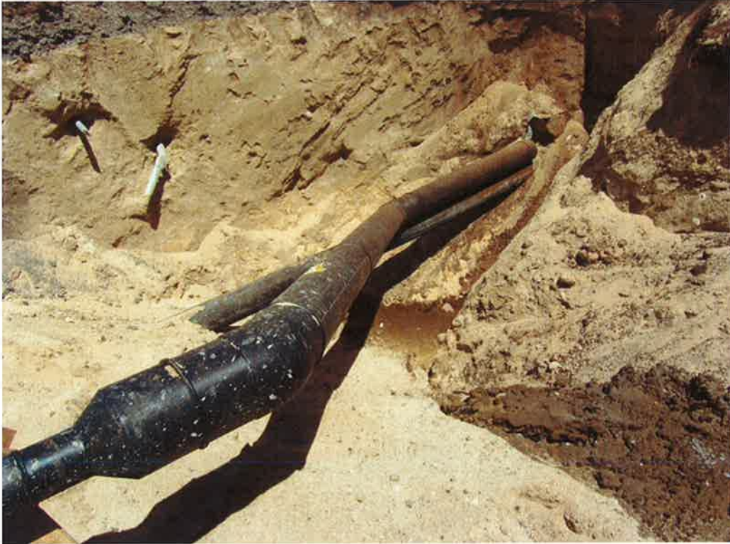
Photo 27. New meter valve box assembly tie-in location to existing discharge lines.
