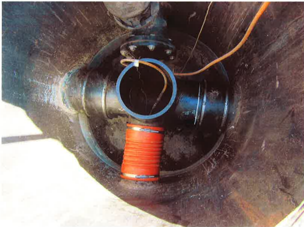
Photo 104. LCM 10 modification with isolation plug prior to installation of Fernco cap.
