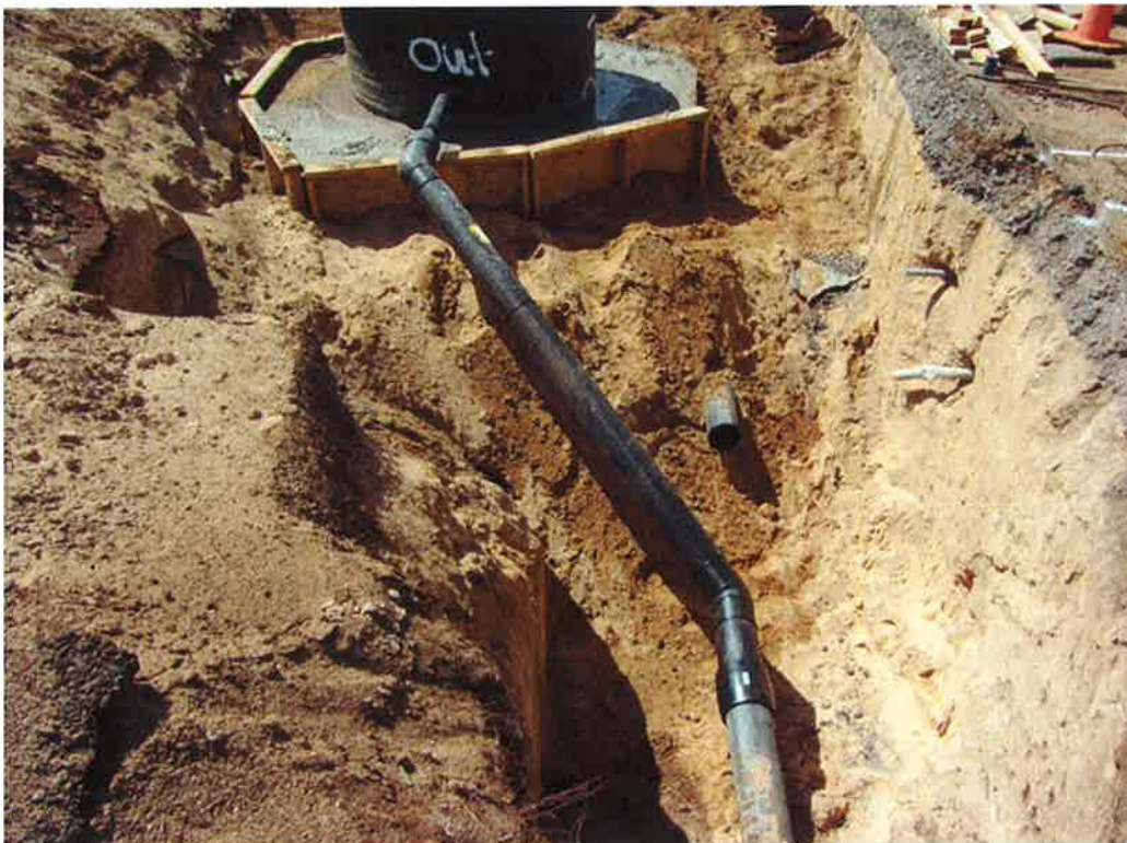
Photo 28. Electro-fusion coupler to join the new meter valve box assembly to the existing discharge line.
