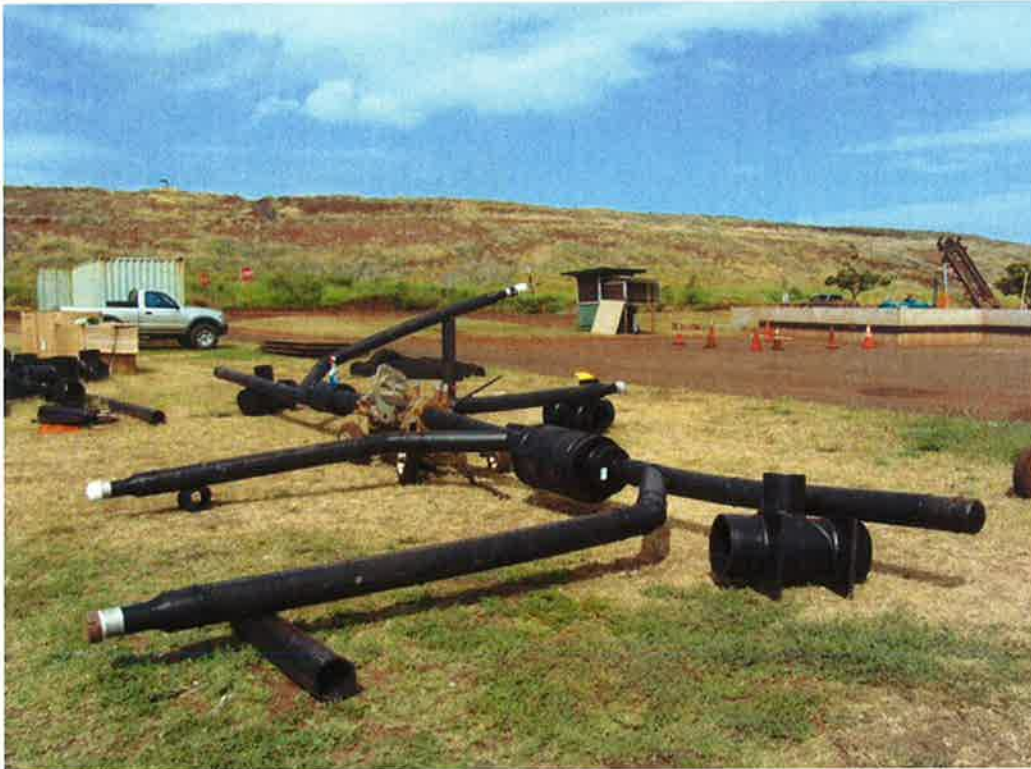
Photo 15. Various fusion welded components connected together to perform system air pressure tests.
