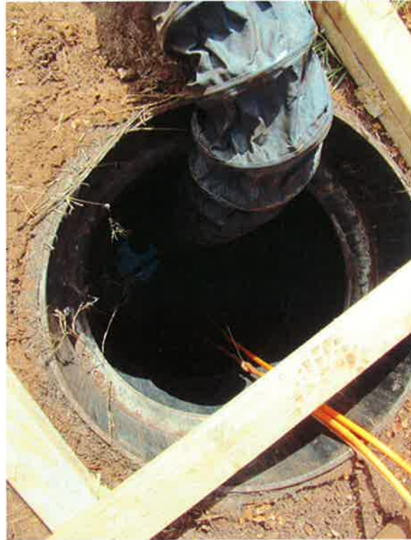
Photo 41. Positive pressure ventilation within the existing valve box in preparation for removal.
