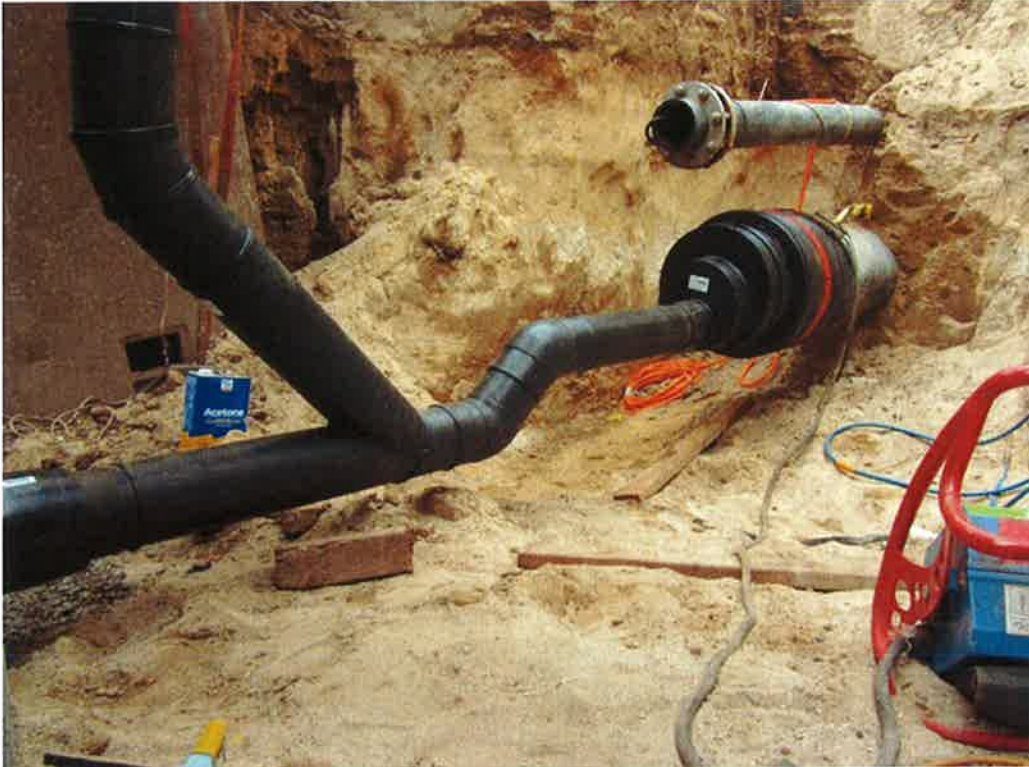
Photo 61. Wet Well #1 plumbing to connect the existing inlet to the cleanout riser assembly.
