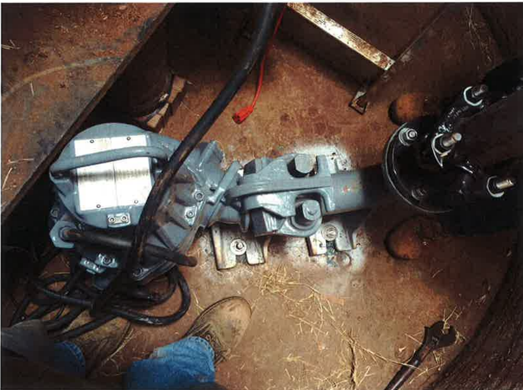
Photo 116. New Flygt pump, mounting system, and discharge piping installed in Wet Well #2 in 2015 (typical).
