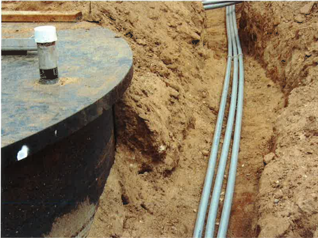
Photo 81. Wet Well #1 electrical conduit installation (later modified).
