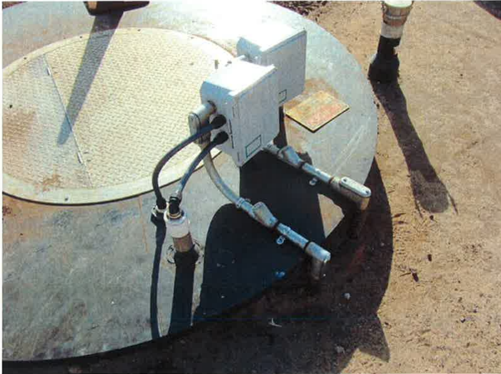
Photo 35 Completed Wet Well #2 electrical junction box (later modified).
