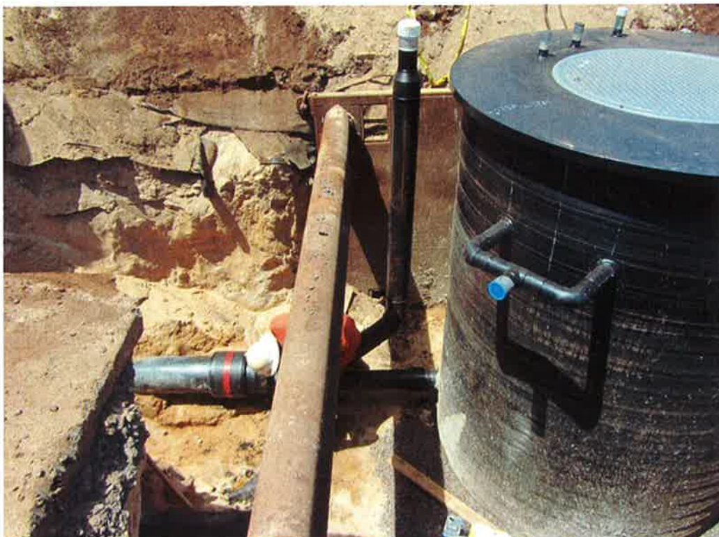
Photo 16. Electro-fusion coupler used to join existing plumbing to the new Wet Well #2 system.
