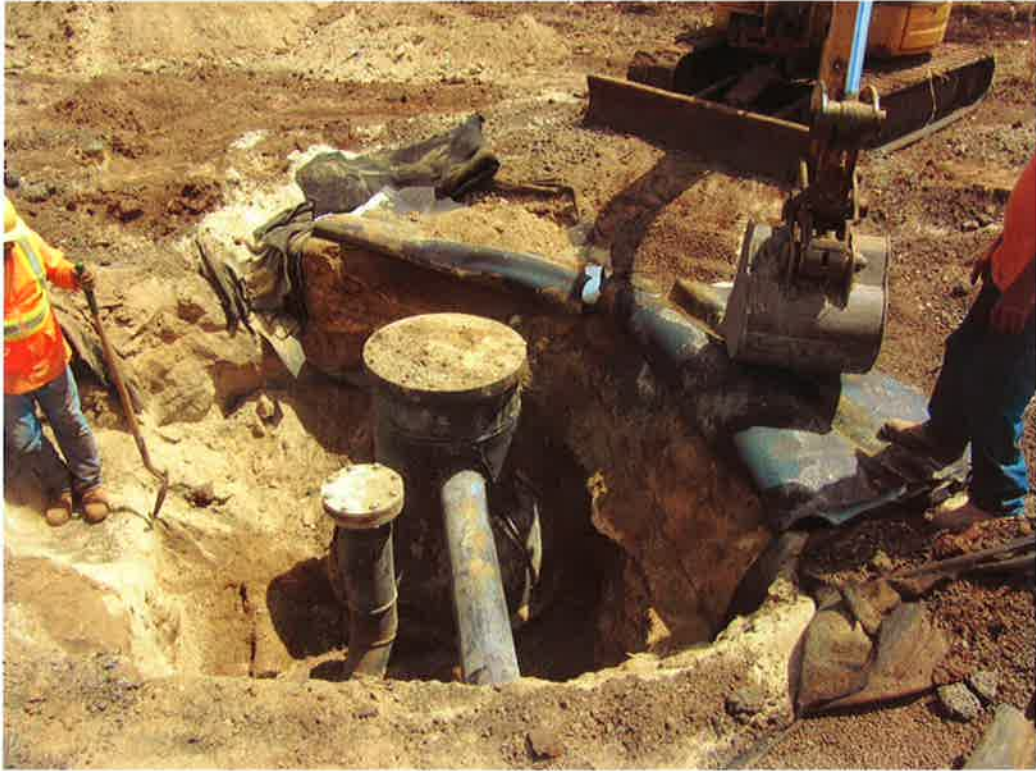
Photo 108. LCM 14 excavation to expose upper bell section to gain access for the modification.
