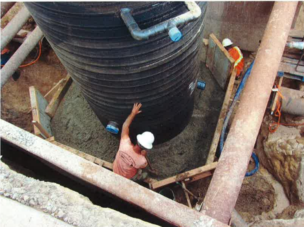
Photo 52. Concrete poured directly into the forms to construct the Wet Well #1 ballast system.
