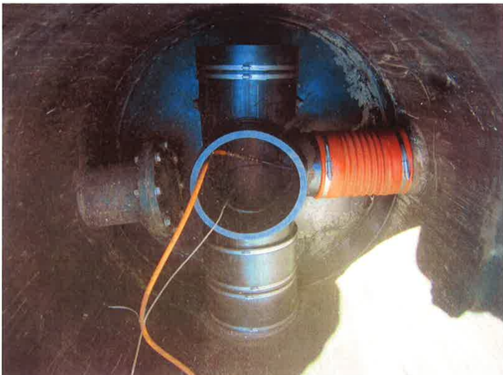
Photo 102. LCM 8 modification with isolation plug prior to installation of Fernco cap.
