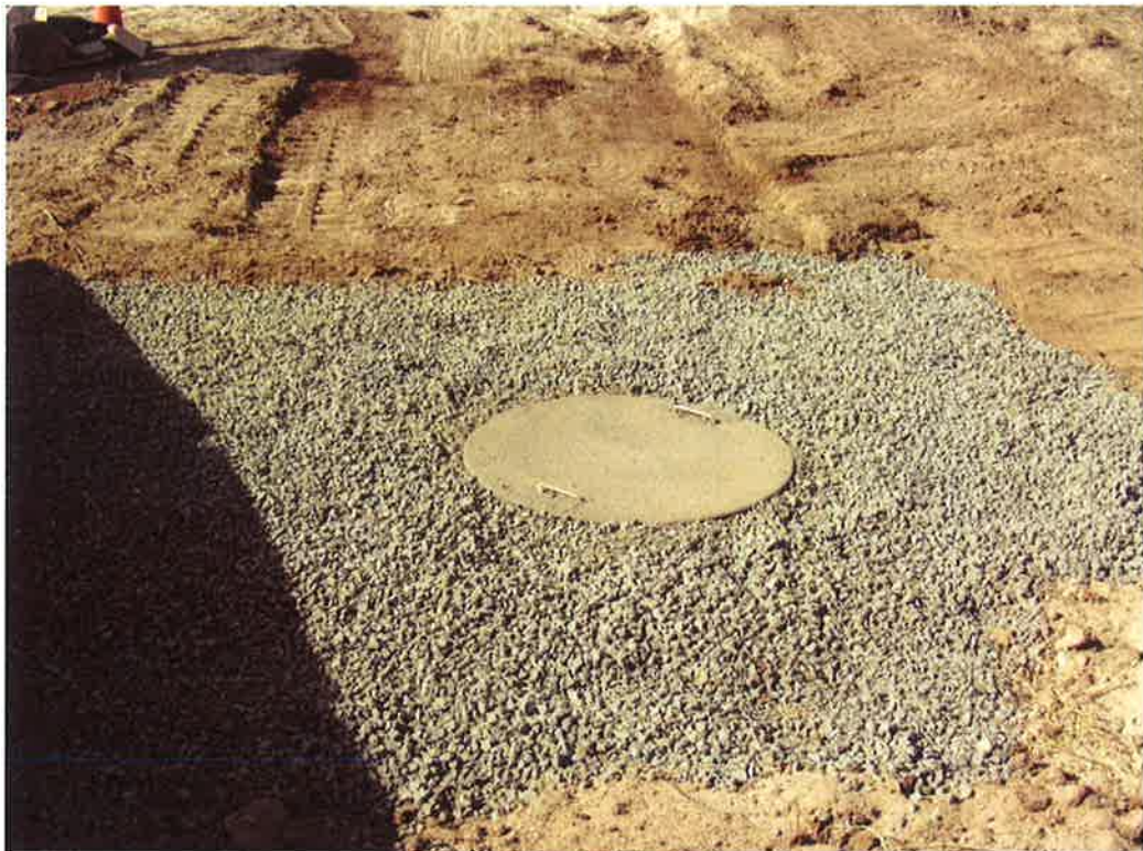
Photo 95 LCM 1 Surface completion.
