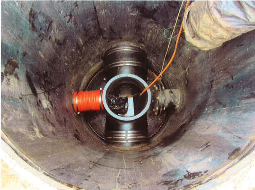
Photo 99. LCM 5 modification with isolation plug prior to installation of Fernco cap.
