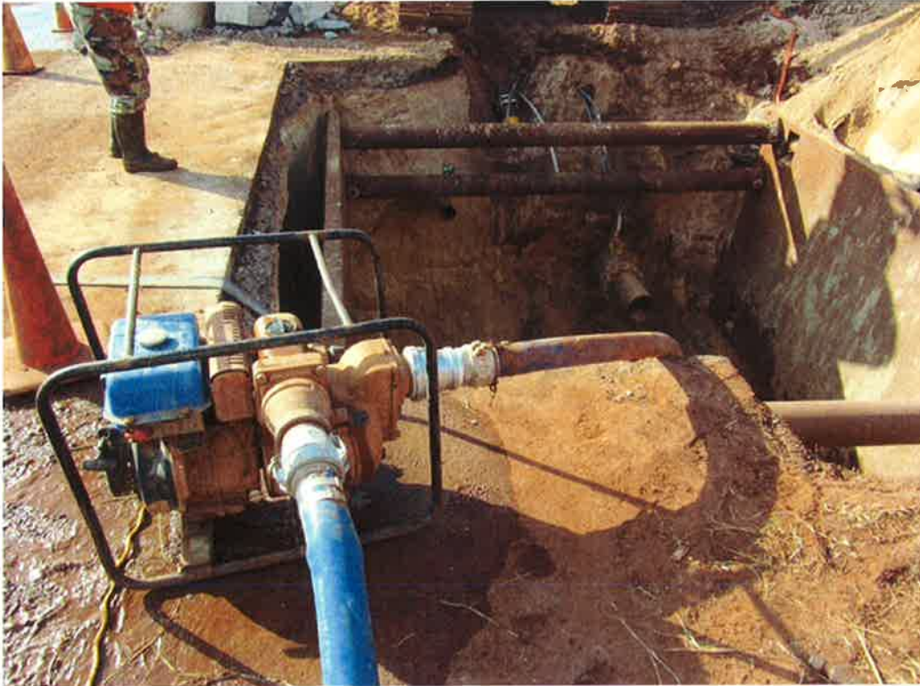
Photo 7. Dewatering excavation using a 3-inch trash pump.
