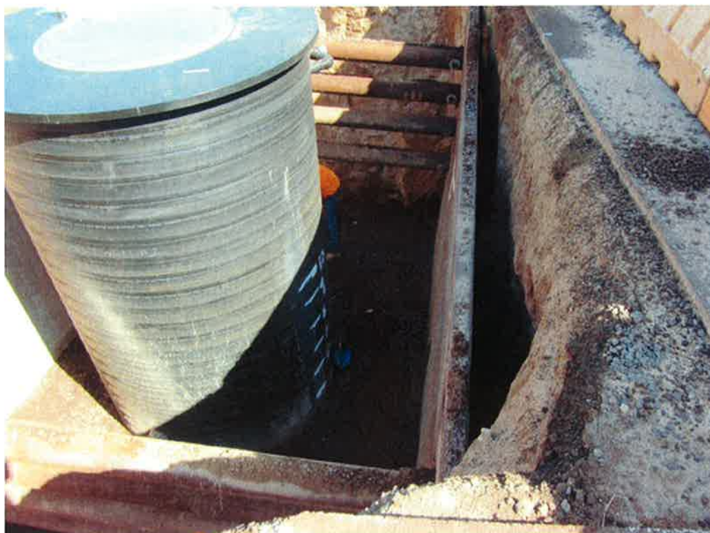
Photo 54. Backfill around ballast system using 3B course gravel.
