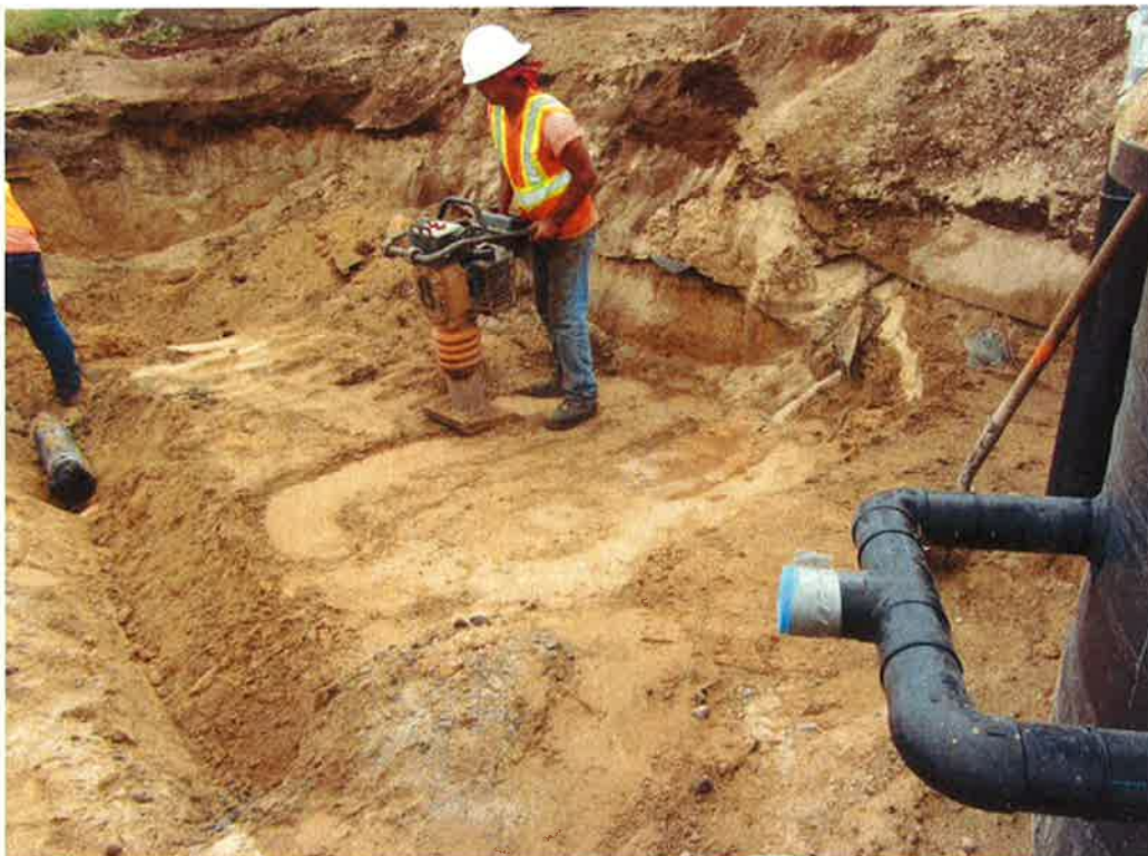
Photo 22. Backfill to construct the foundation for the new meter valve box assembly.
