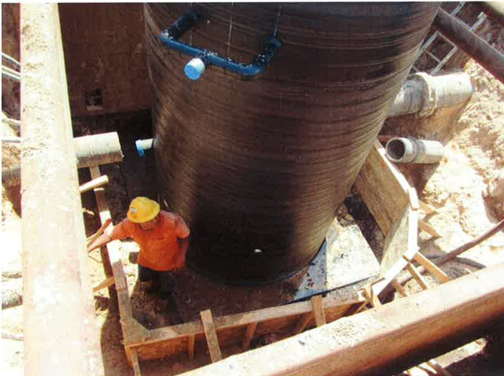
Photo 10. Form boards to construct new Wet Well #2 concrete ballast.
