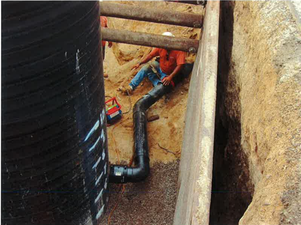
Photo 63. Existing 8-inch HDPE catch basin drain pipe installation to the new Wet Well #1
