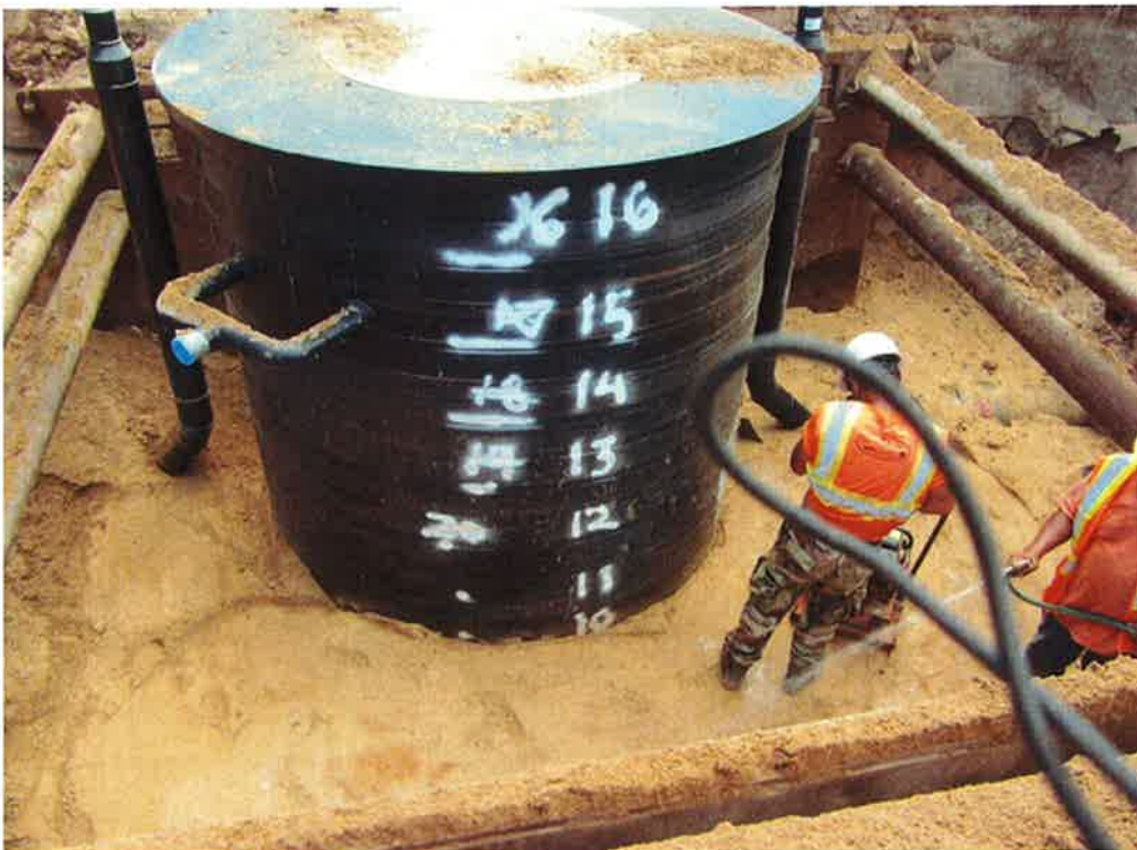
Photo 20. EP continues to backfill around Wet Well #2.
