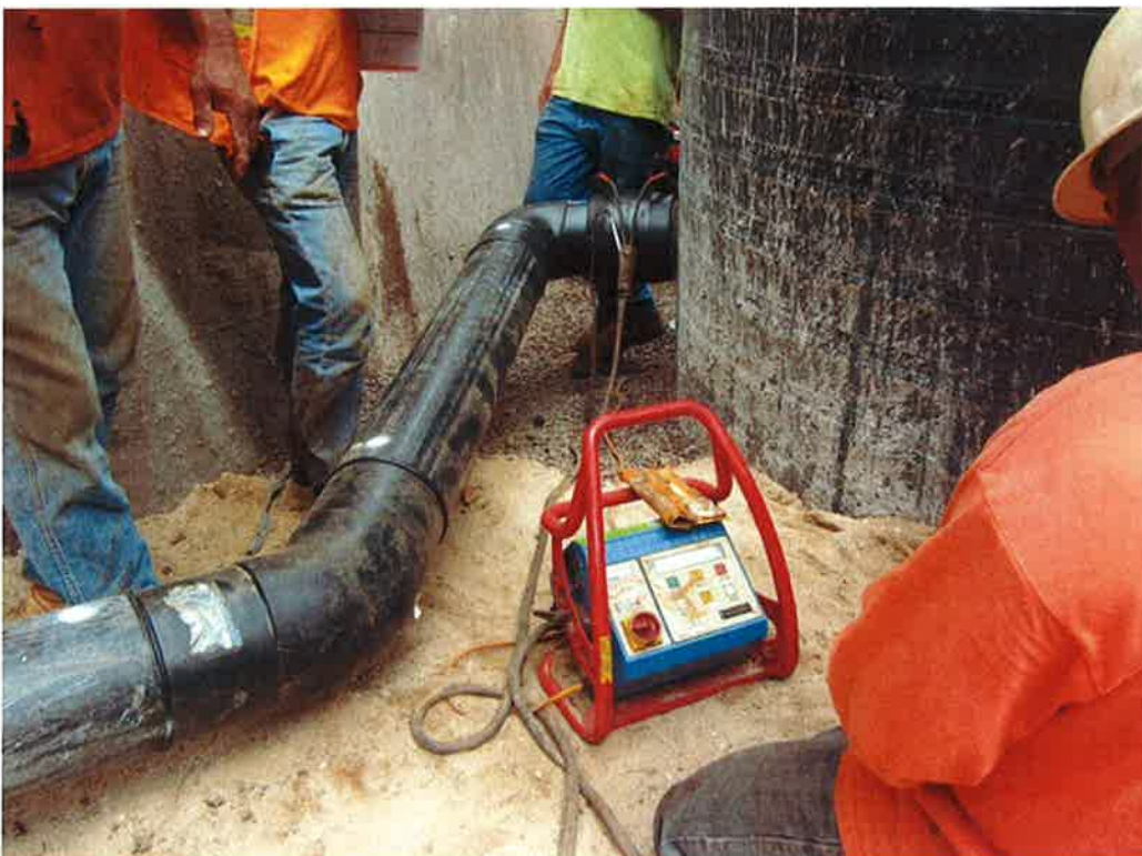
Photo 64. Final connection to complete the existing catch basin drain pipe assembly.
