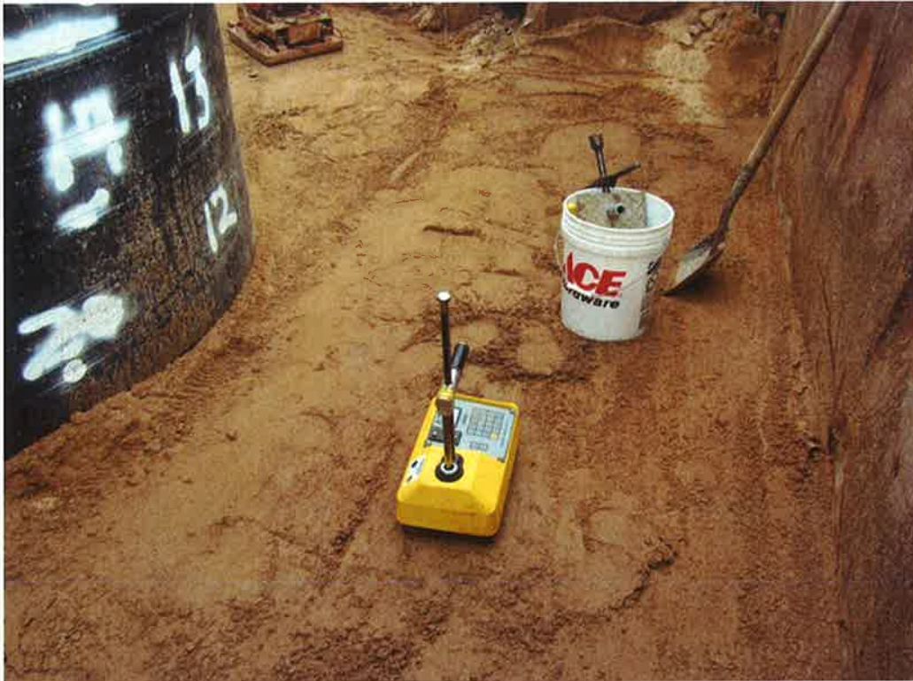
Photo 21. Field density testing using a Troxler portable moisture/density gauge.
