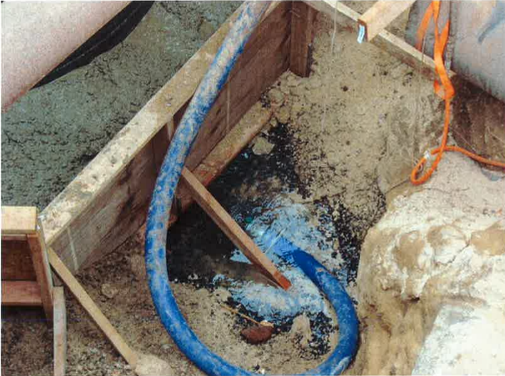
Photo 51. 3 inch suction pump to manage groundwater during construction.
