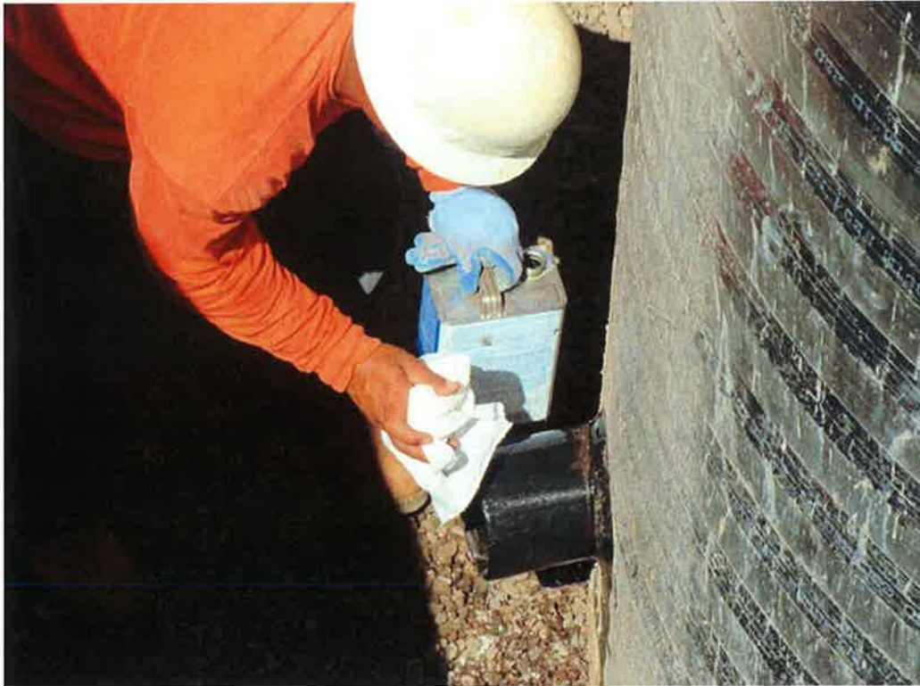
Photo 55. Cleaning plumbing connection in preparation for electro-fusion coupler installation.
