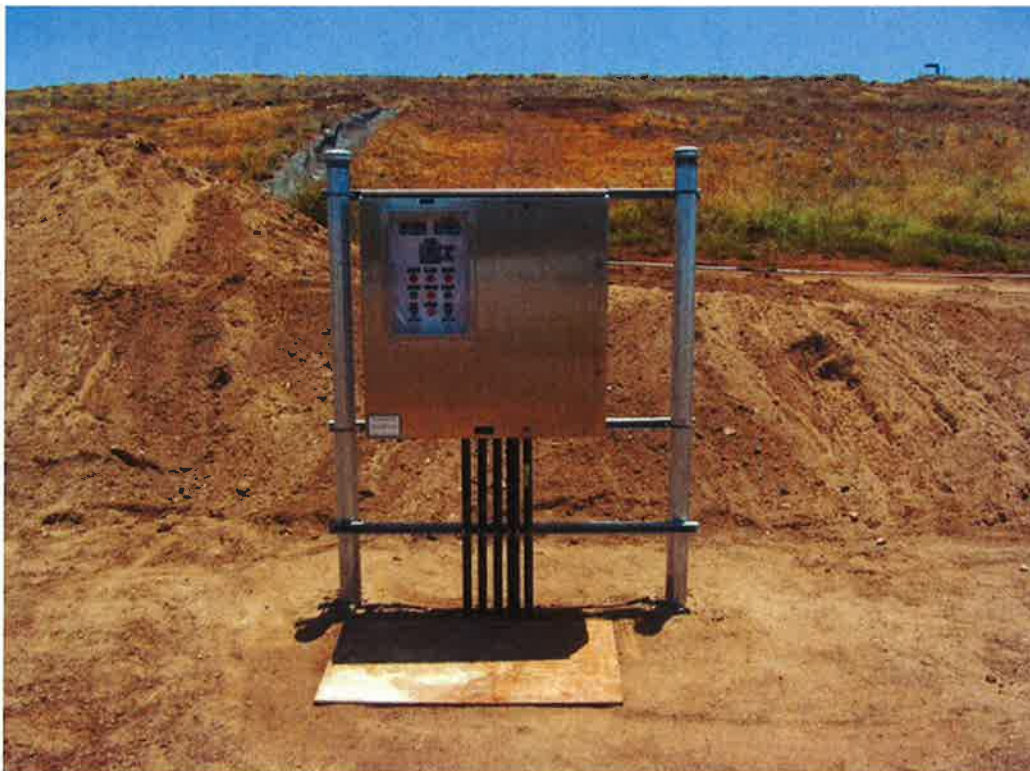
Photo 82. Completed Wet Well #1 EPG master control panel (later modified).
