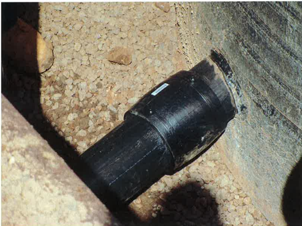
Photo 56. Electro-fusion coupler to connect cleanout riser assembly to the new Wet Well #1.
