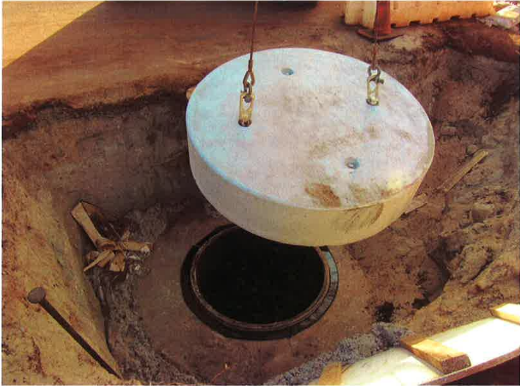
Photo 90. LCM 2-13 reinforced concrete protective cover installation, with water stop seal (typical).
