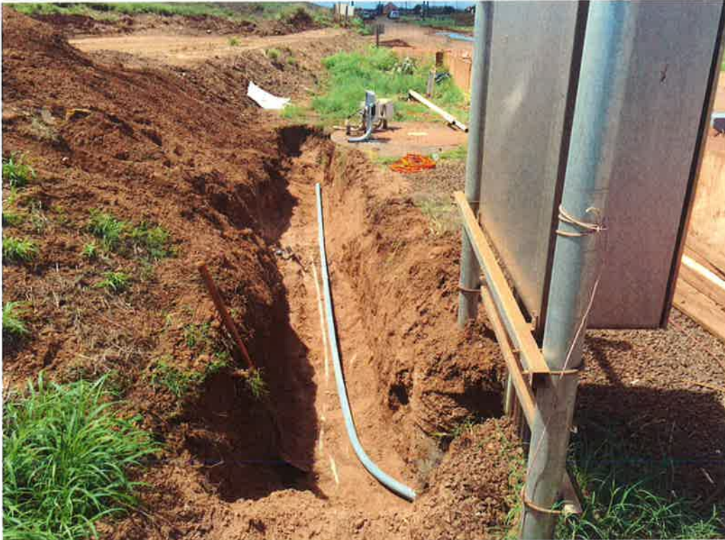
Photo 113. Additional conduit installed from control panel to wet wells in 2015 in preparation for pump replacement. (typical).
