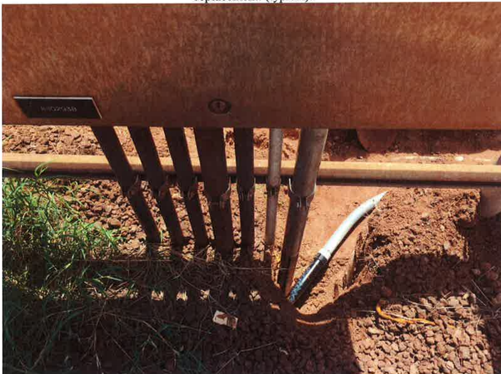
Photo 114. Additional conduit at base of panel (typical).
