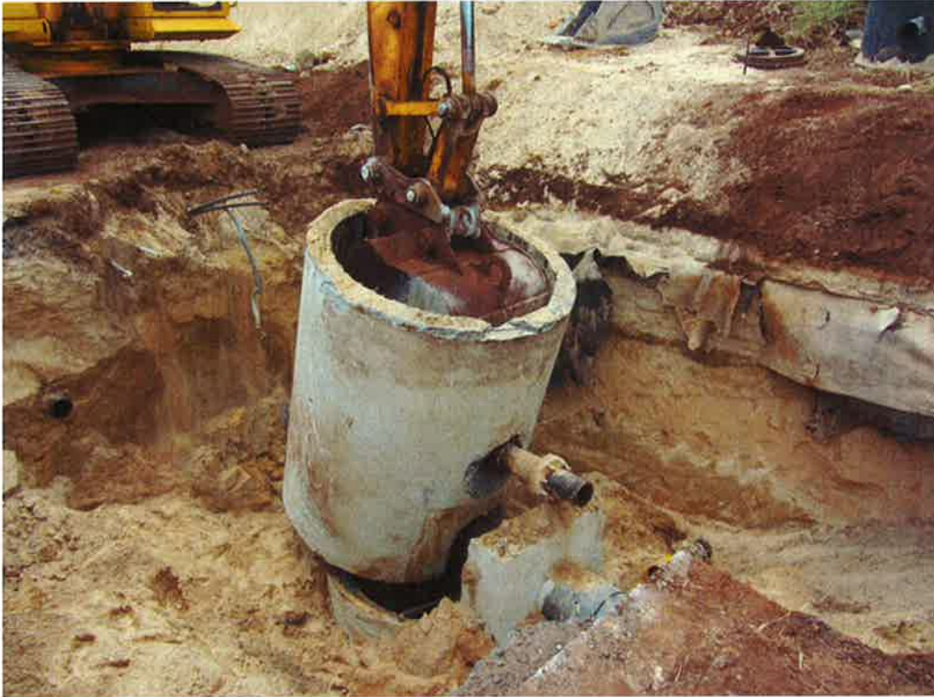
Photo 5. Removal of existing Wet Well #2.
