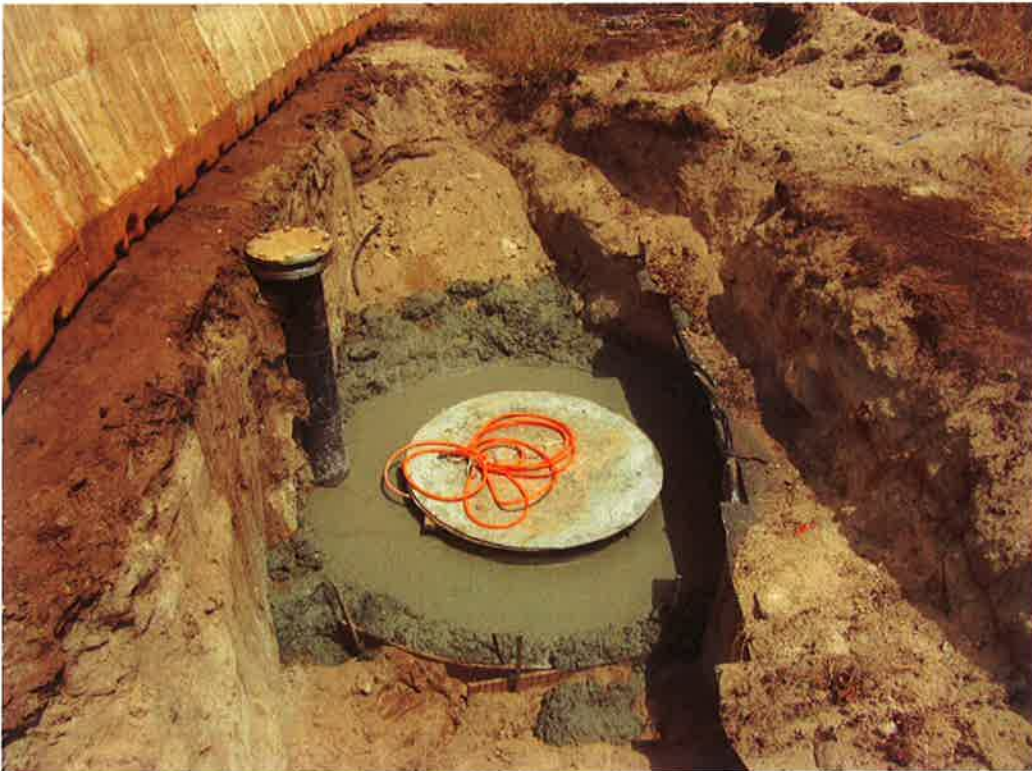
Photo 86. LCM 2-13 concrete foundation support (typical)..
