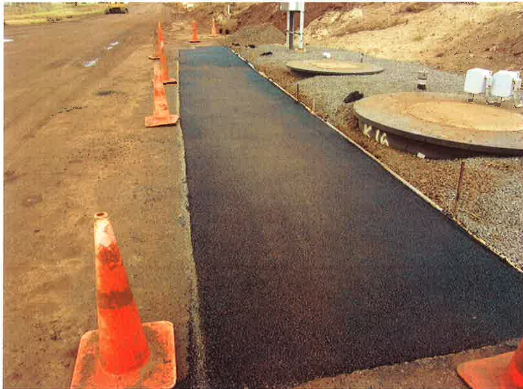
Photo 112. Completed asphalt surface.
