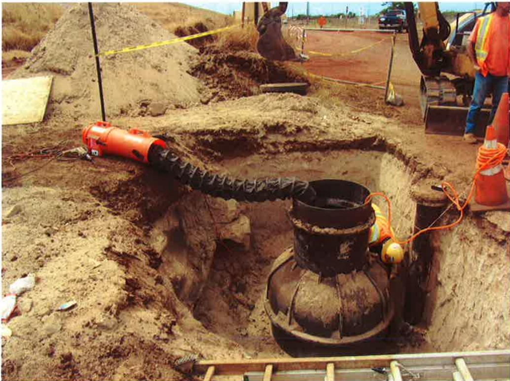
Photo 83. LCM 2-13 upper bell section removal for access to fittings (typical).
