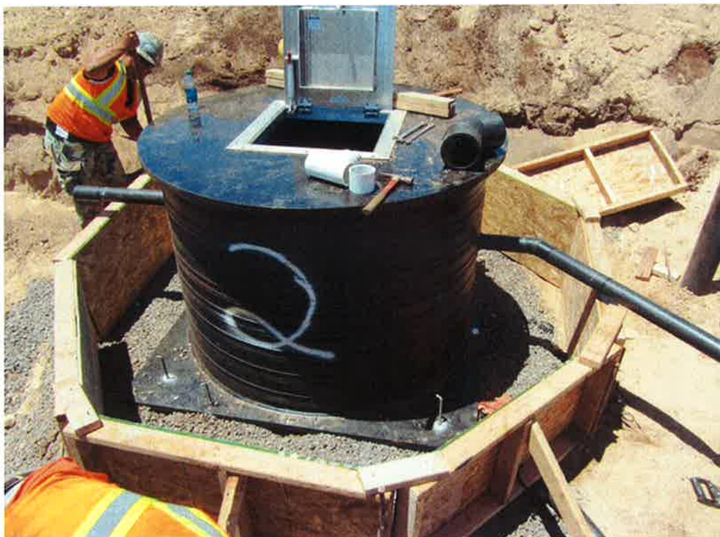
Photo 24. Form boards to construct the meter valve box #2 assembly ballast.
