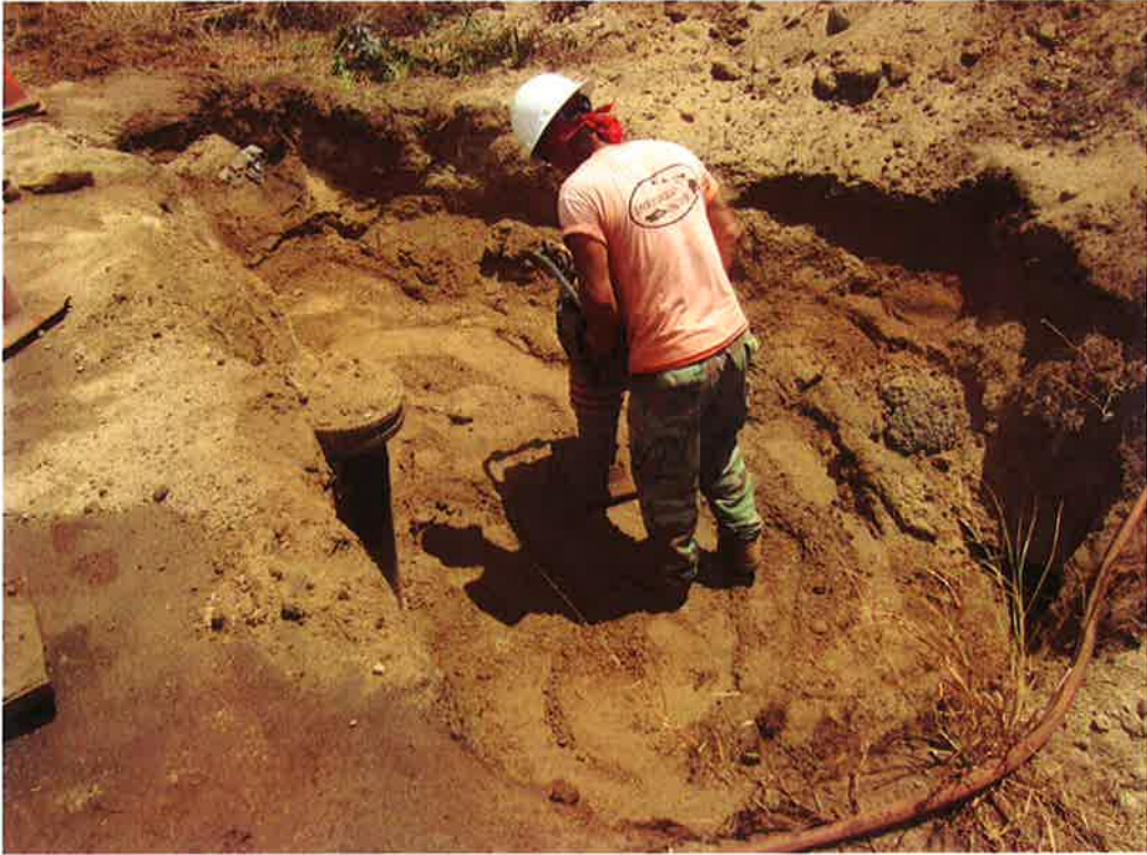
Photo 92. LCM 2-12 backfill using onsite sand (typical). Compaction effort using a “jumping-jack” compactor.
