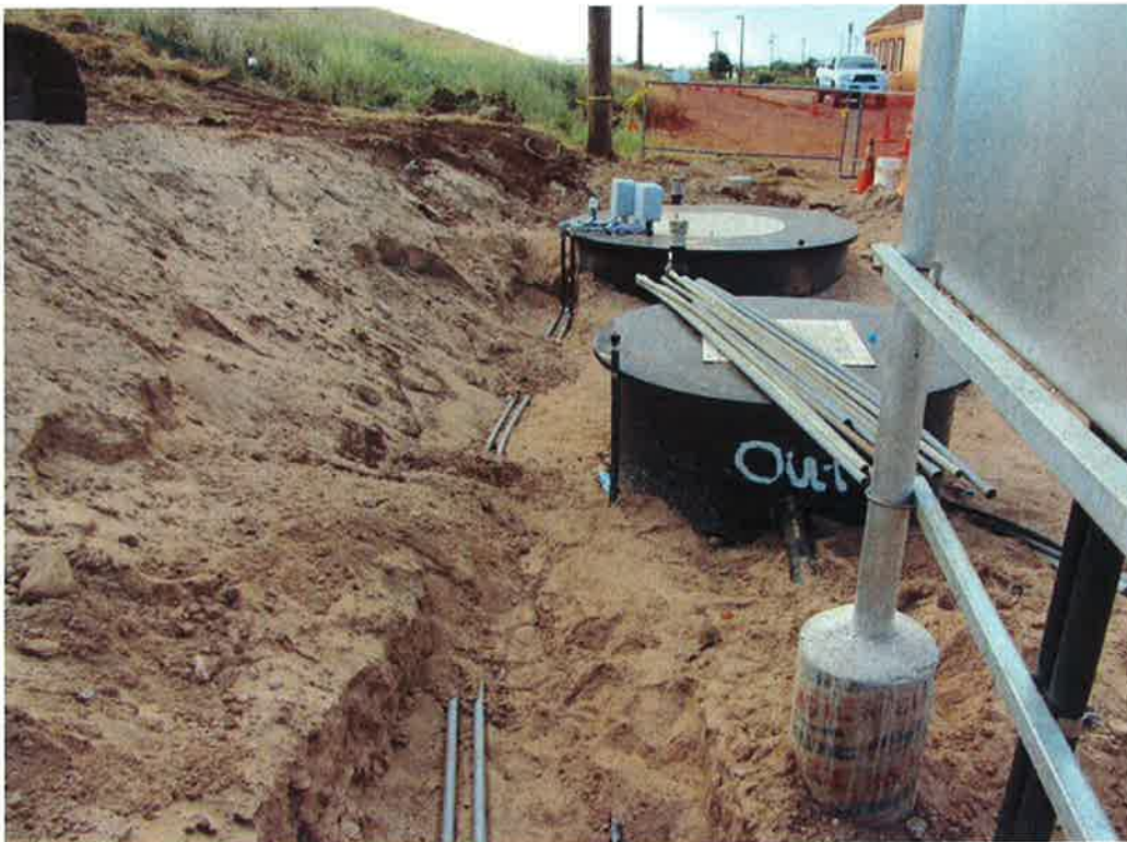
Photo 32. Wet Well #2 electrical system conduit location (later modified).
