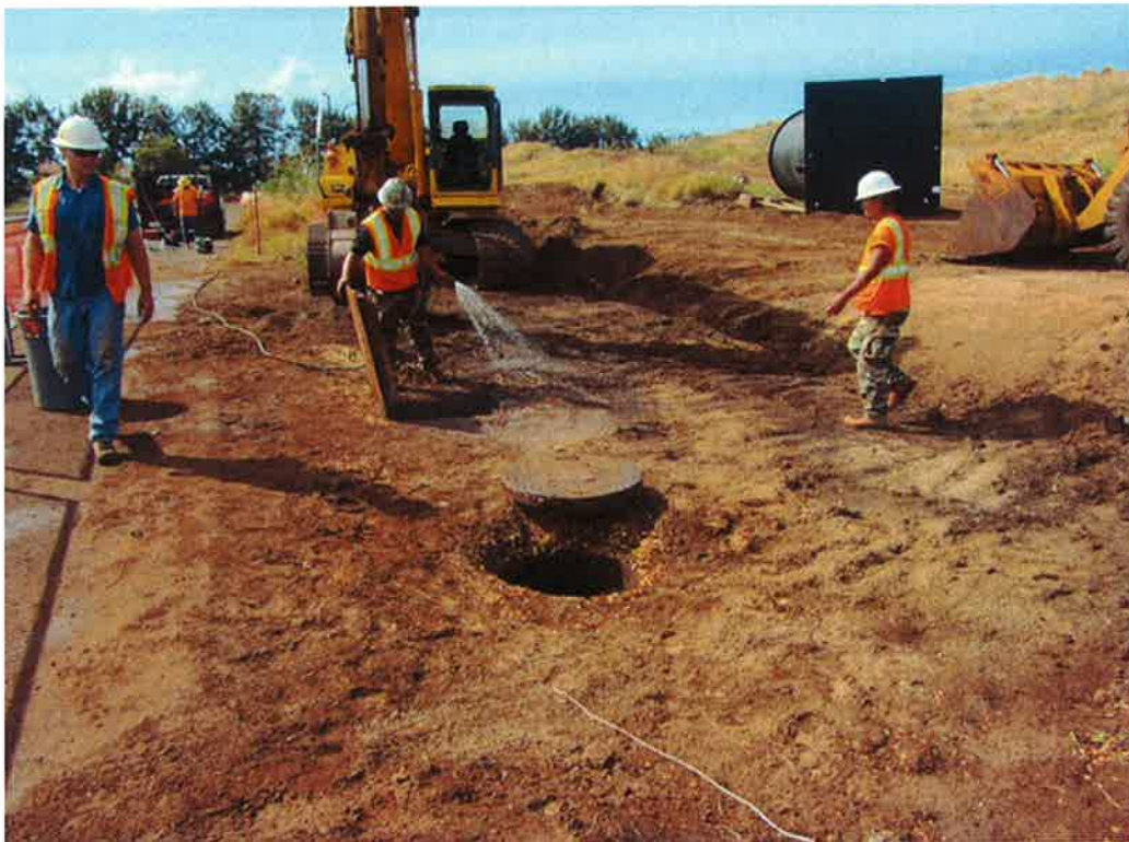
Photo 42. Dust suppression during excavation of the existing Wet Well #1 1.
