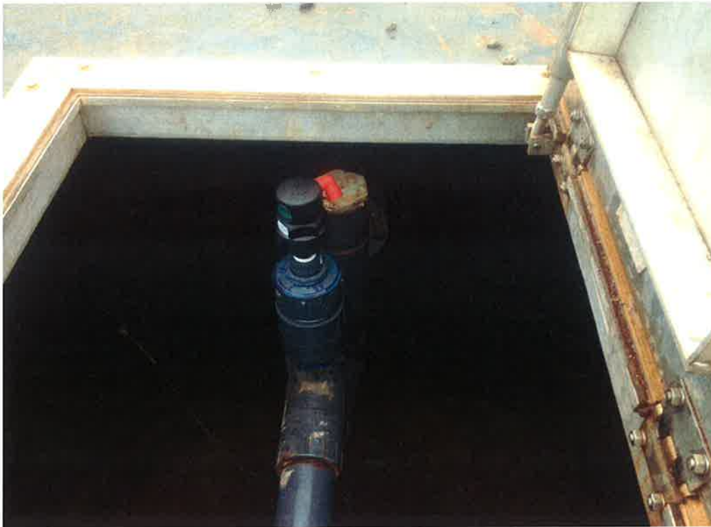
Photo 38. Air relief valve installed on the discharge piping within the meter valve box.
