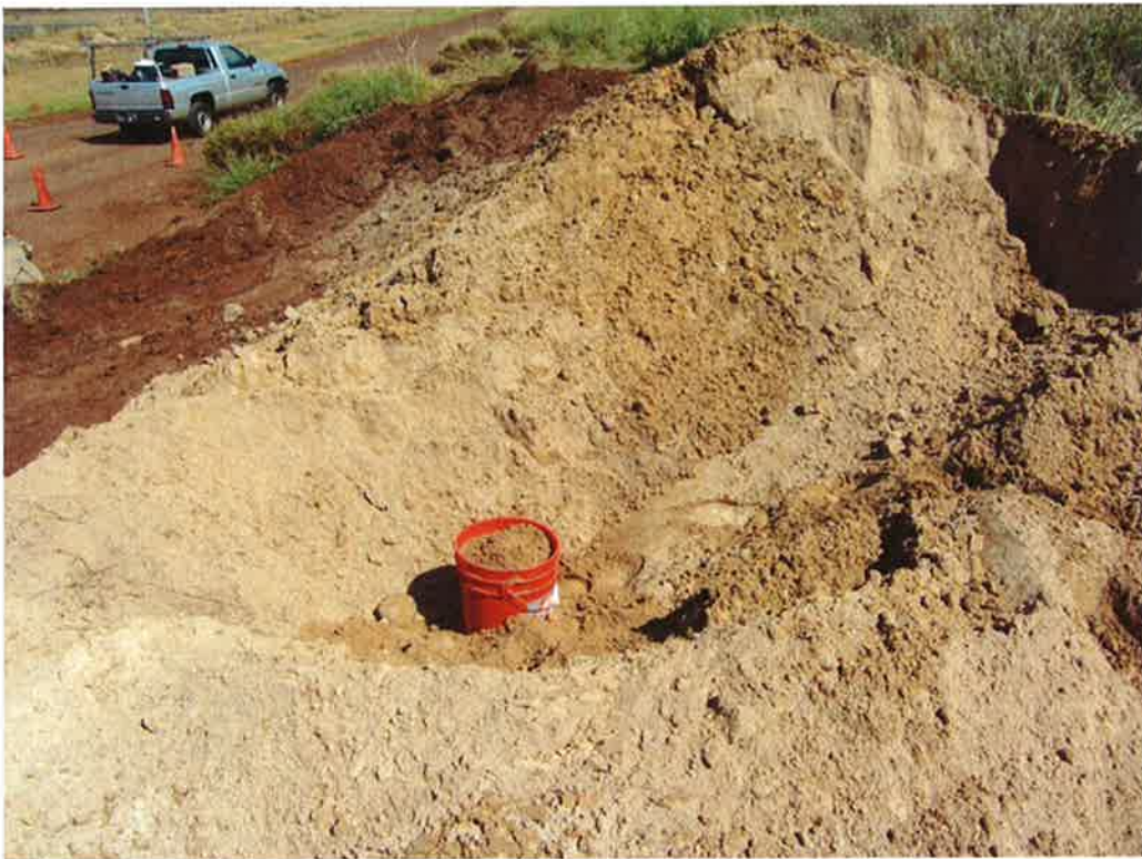
Photo 4. Sample of onsite backfill material.
