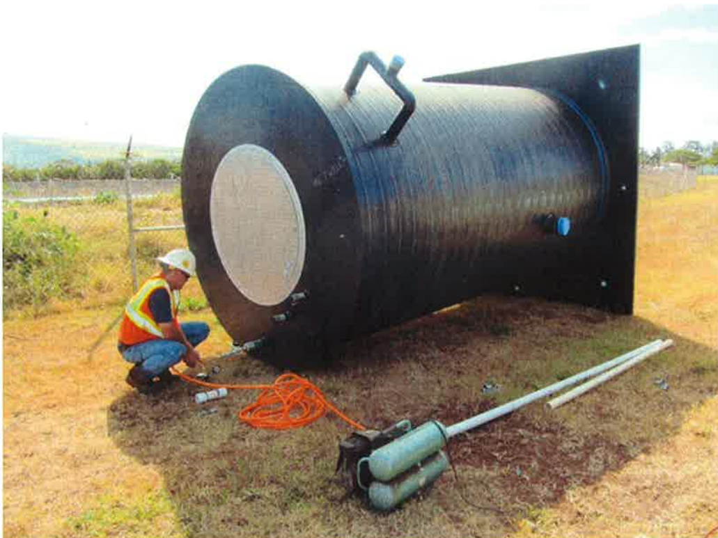
Photo 8. Pressure testing interstitial space to verify wet wells do not leak.
