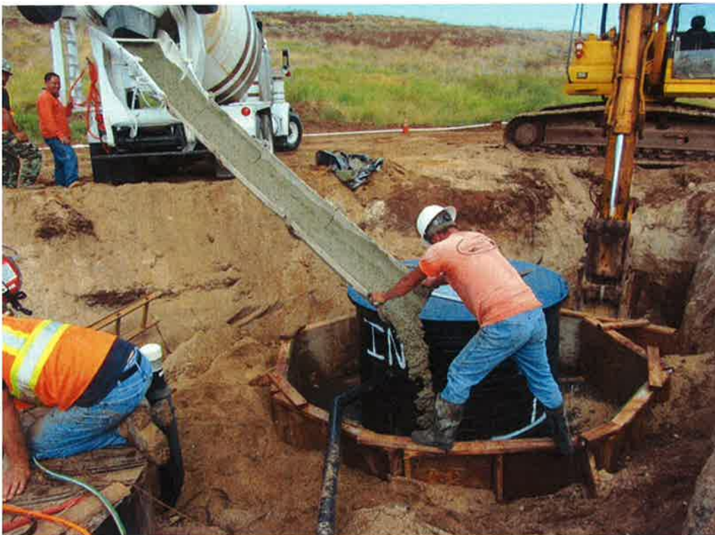
Photo 72. Concrete poured directly into prepared forms to construct the ballast system.
