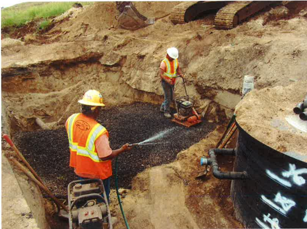
Photo 23. Gravel placement to support the meter valve box #2 assembly.
