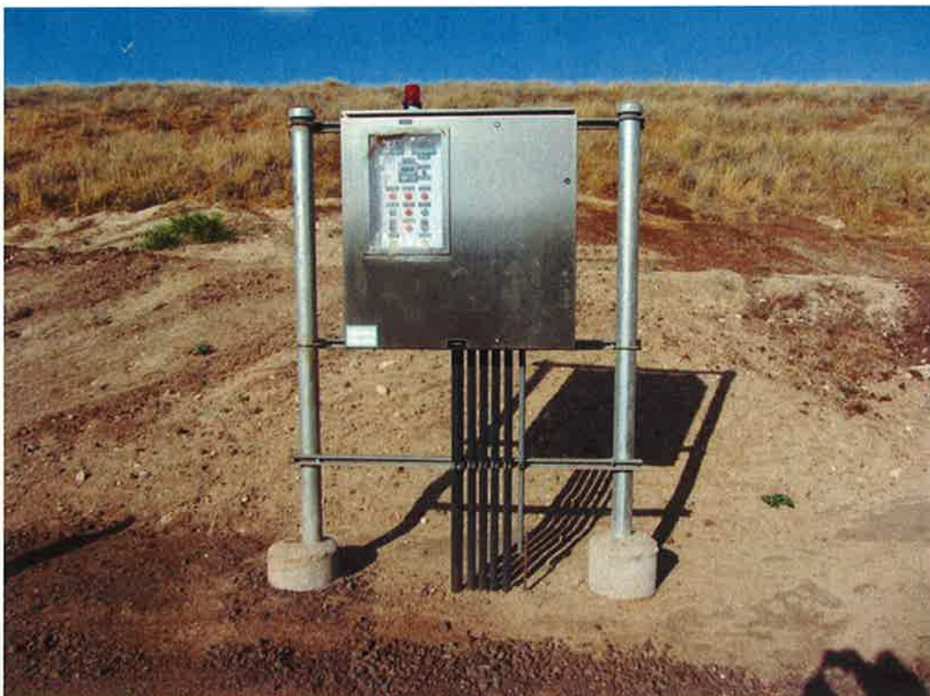
Photo 36. Completed Wet Well #2 control panel (later modified).
