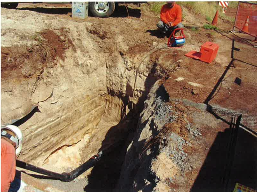
Photo 74. Final connection to complete the discharge piping connection.
