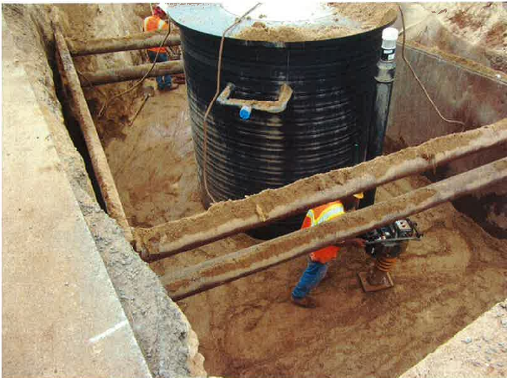
Photo 68. Compaction effort using a walk behind "jumping jack" compactor.
