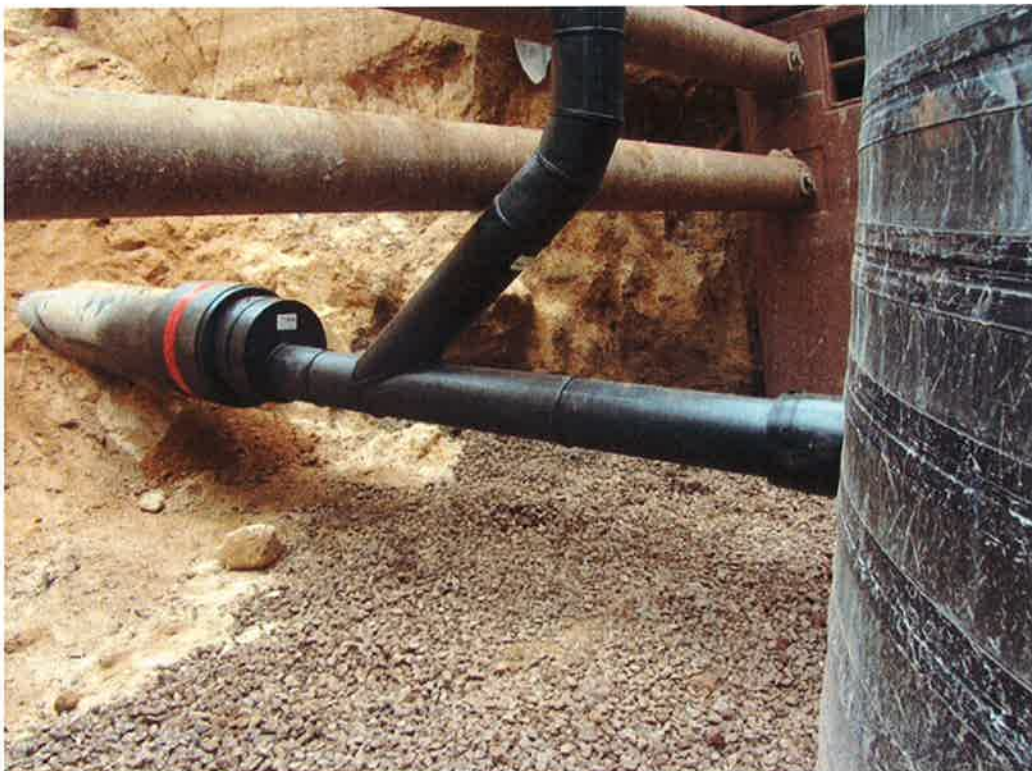
Photo 60. Completed assembly to connect the existing system to the new Wet Well #1 assembly.
