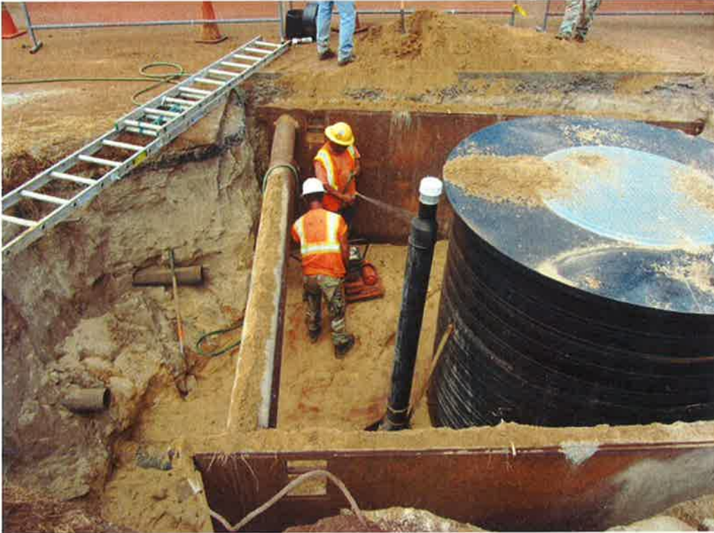
Photo 19. Moisture conditioning during backfill around the newly installed Wet Well #2.
