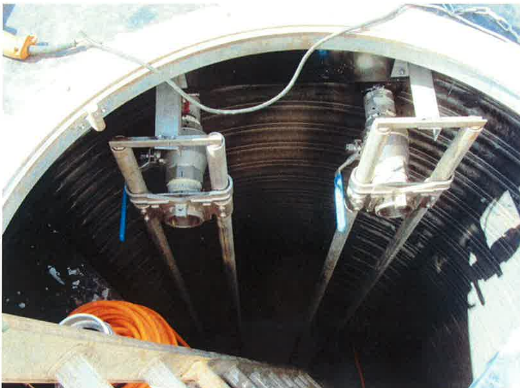
Photo 78. Wet Well #1 rail system pump support (later removed)..
