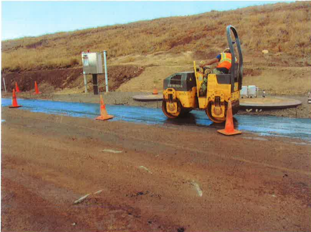
Photo 111. Asphalt surface restoration.
