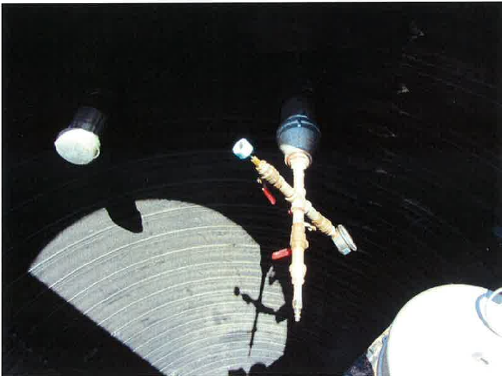
Photo 26. Air pressure test to verify Wet Well #2 discharge piping integrity.
