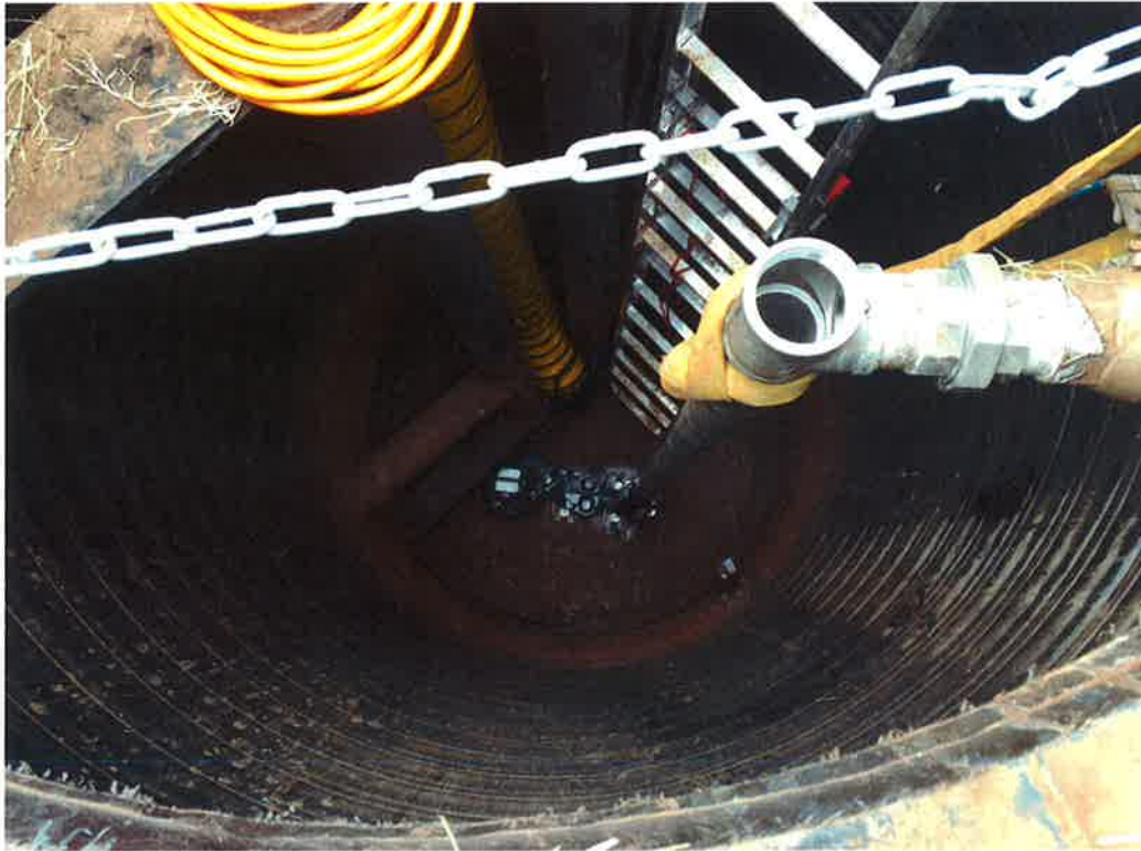
Photo 117. New Flygt pump, mounting system, and discharge piping installed in Wet Well #2 in 2015 (typical).
