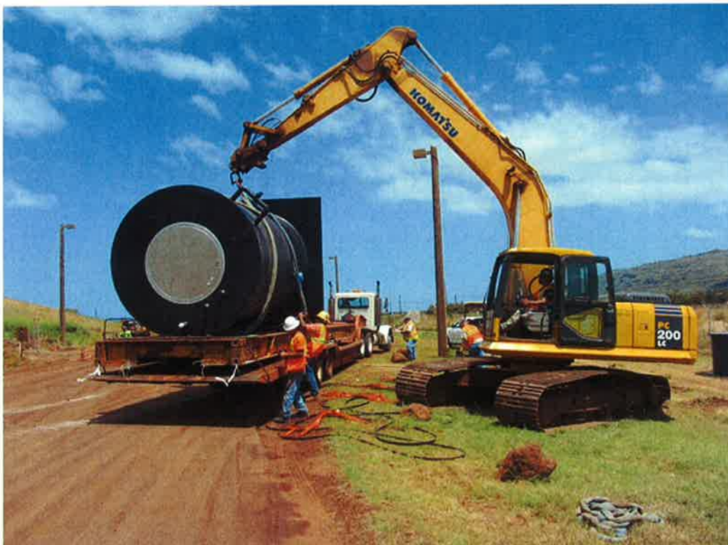
Photo 2. Offloading wet wells and meter valve boxes using an excavator.
