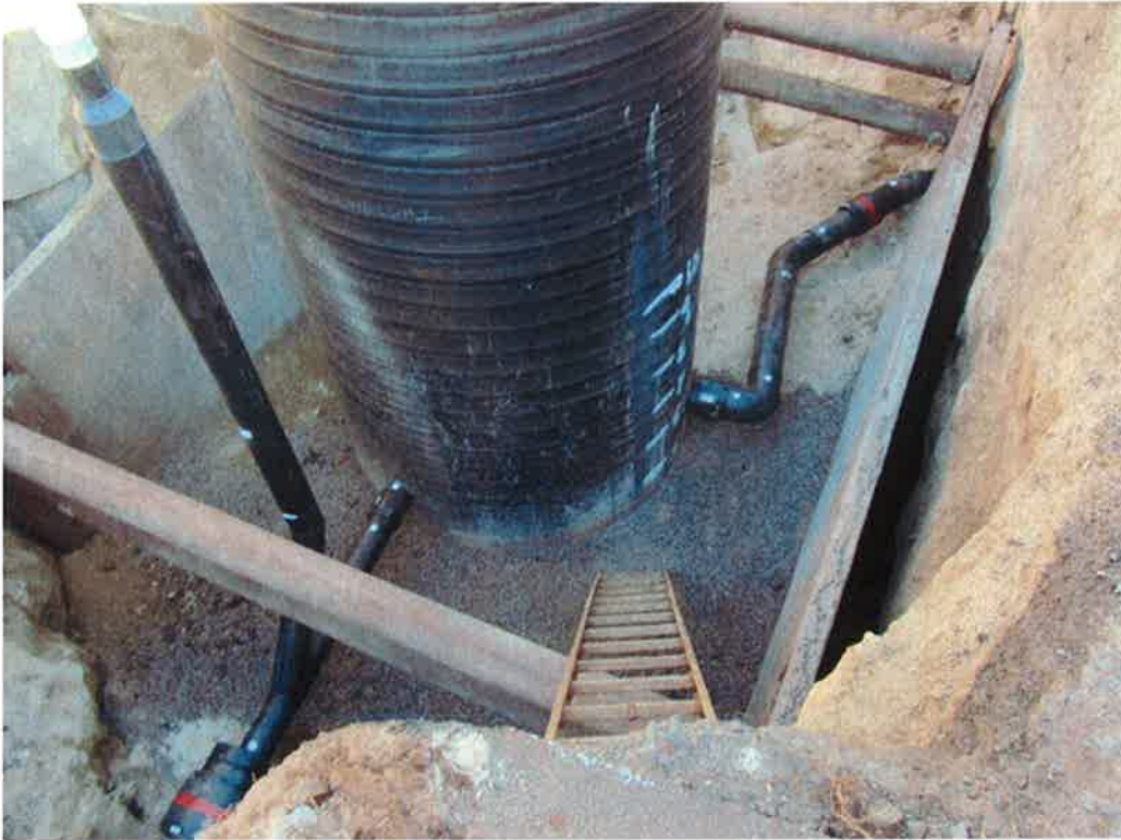
Photo 65. Completed Wet Well #1 plumbing assembly.
