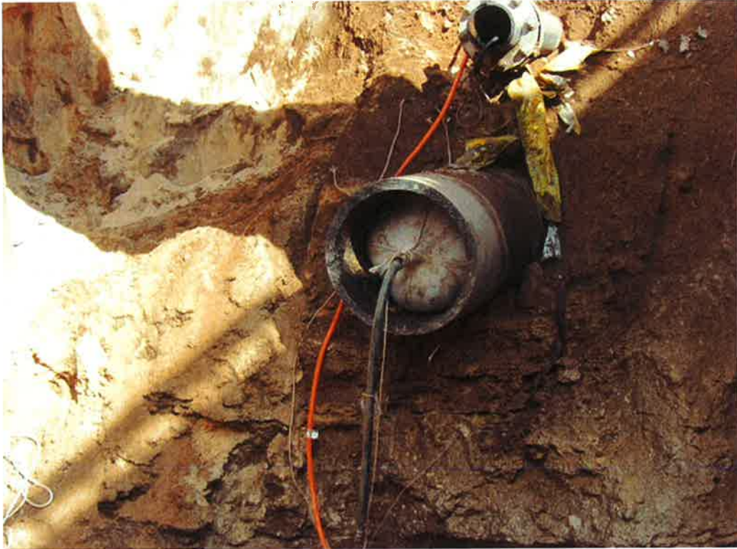
Photo 49. Inflatable isolation plug to manage leachate during construction.
