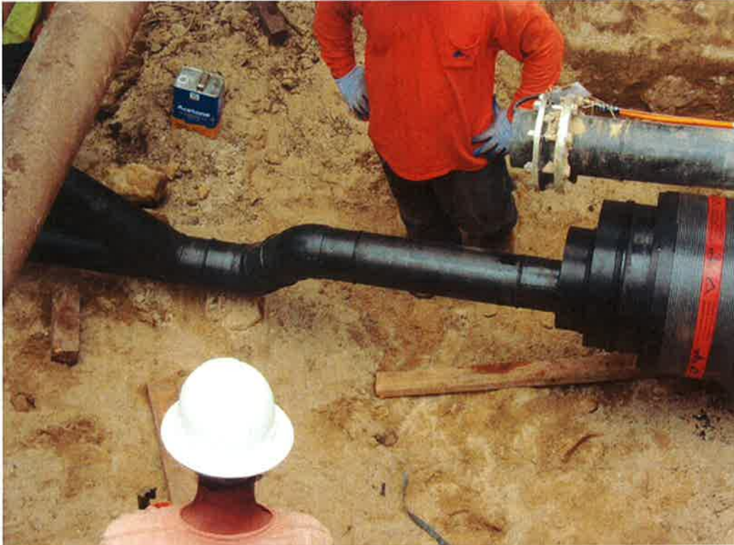
Photo 59. Existing 12-inch HDPE pipe inlet connection to the newly installed Wet Well #1 assembly.
