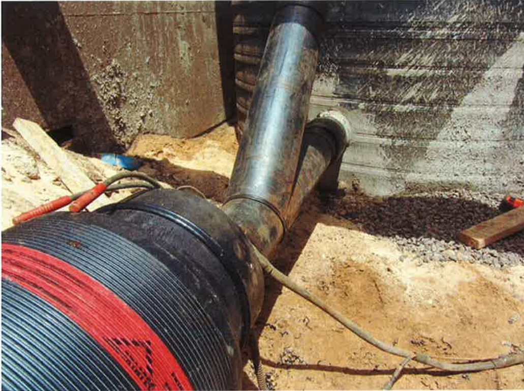
Photo 17. Completed connection to join the leachate collection manhole to the new wet well.
