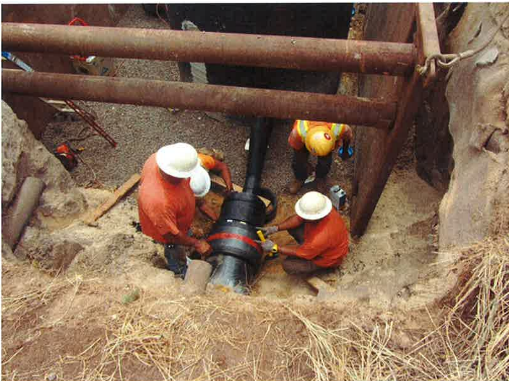
Photo 18. 18-inch electro-fusion coupler to join the existing plumbing to the new Wet Well 2 system.
