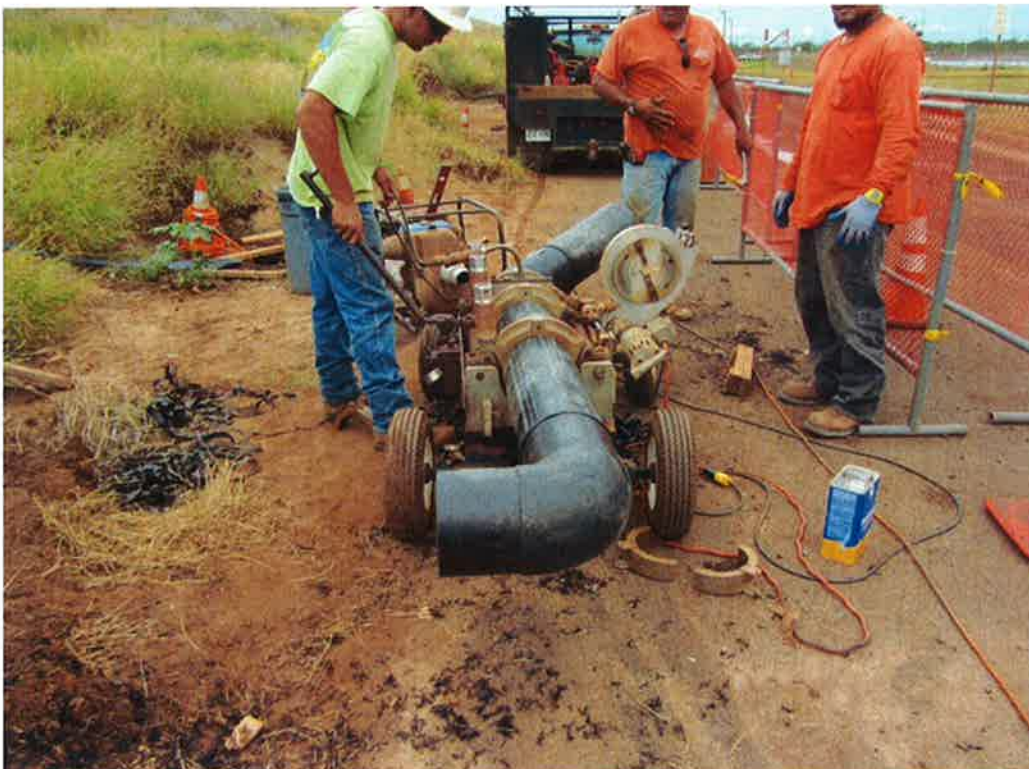
Photo 62. Prefabricated catch basin drain pipe connection.
