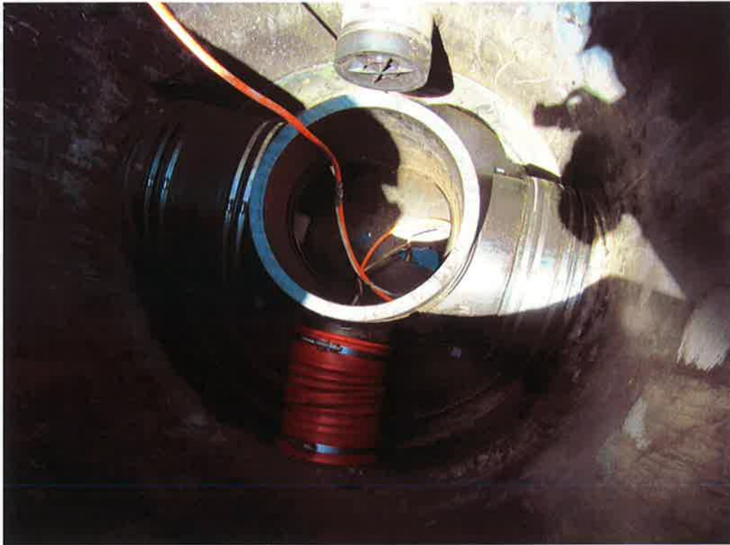
Photo 105. LCM 11 modification with isolation plug prior to installation of Fernco cap.
