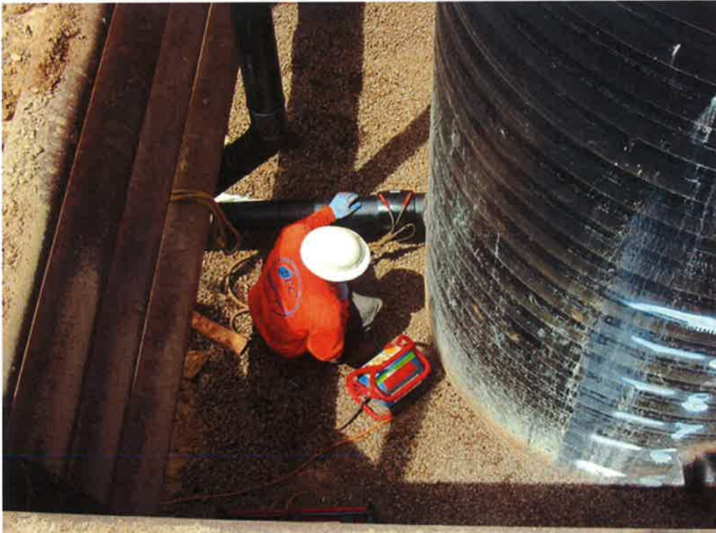
Photo 57. Electrofusion coupler installation using a Friatec electrofusion system
