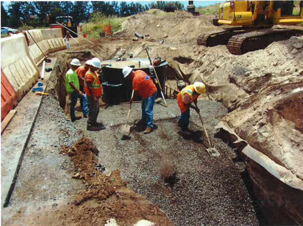
Photo 69. 3B course gravel used to construct the meter valve box foundation.
