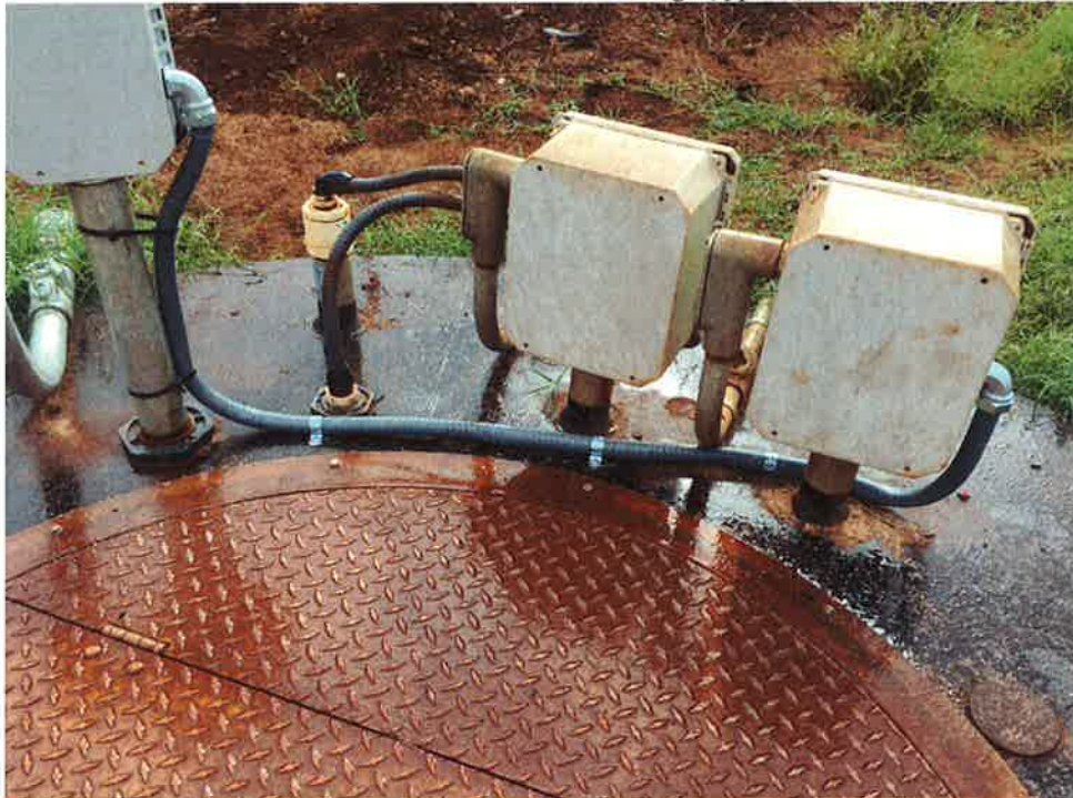
Photo 122. New flexible conduit installed at Wet Well#1 to replace faulty T1 and T2 temperature sensor wires.
