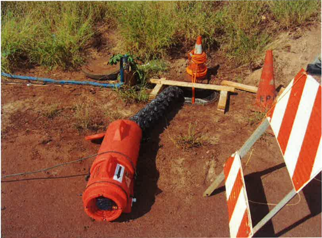
Photo 40. Leachate collection manhole isolation and ventilation during construction
