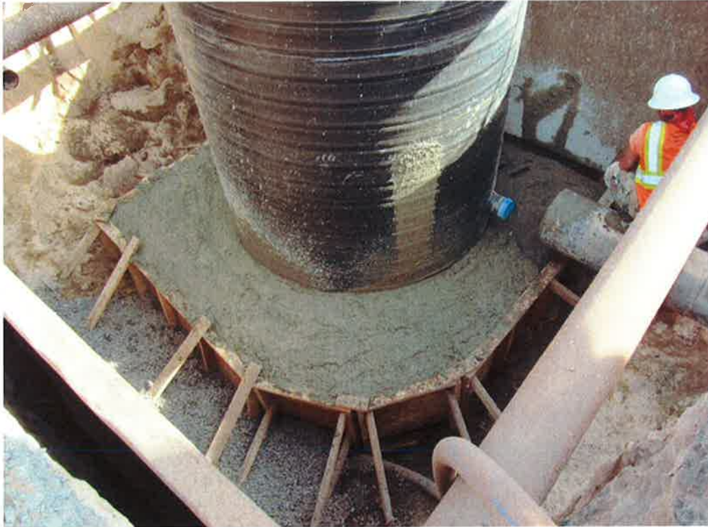
Photo 11. Concrete poured into prepared forms to construct the concrete ballast system.
