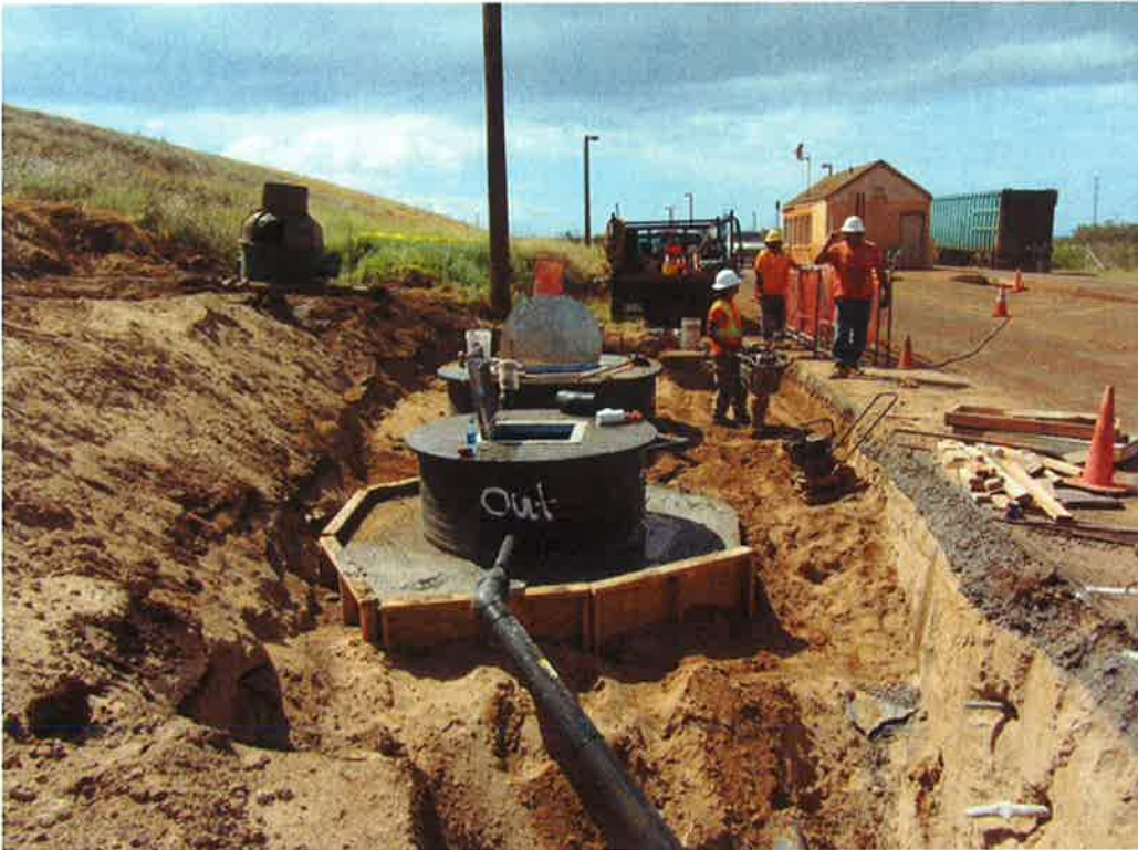
Photo 29. New Wet Well #2 system installation looking north.
