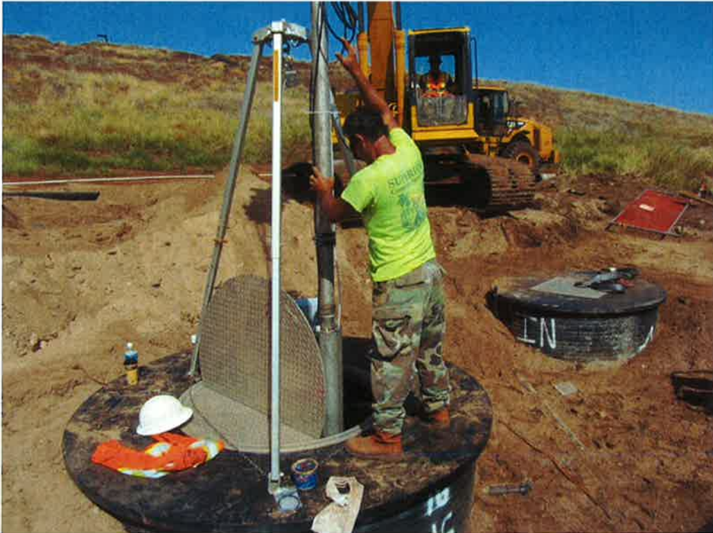
Photo 77. Wet Well #1 pumping system installation (later removed).
