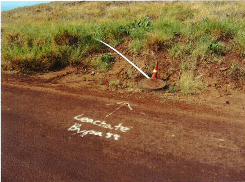
Photo 39. Leachate management via LCM 14 during construction of the new system
