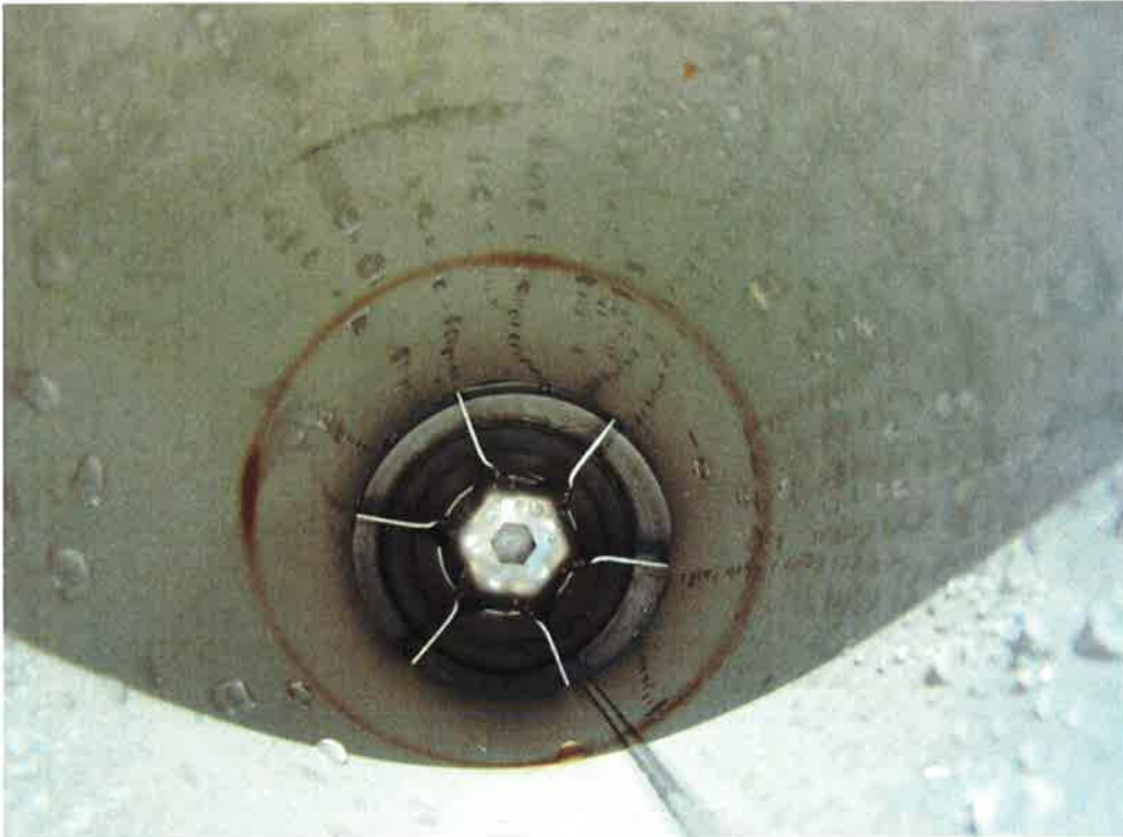
Photo 75. Stainless steel check valve assembly within the EPG pump system (later removed).
