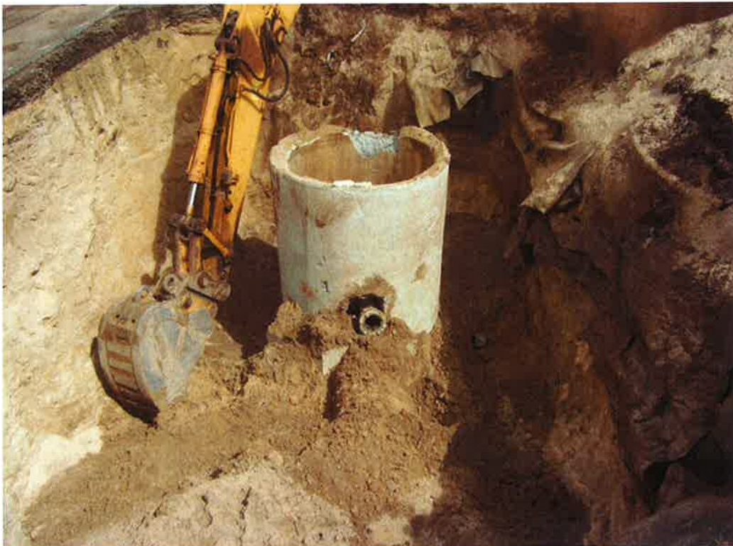
Photo 46. Excavation to remove the lower section of the existing Wet Well #1.
