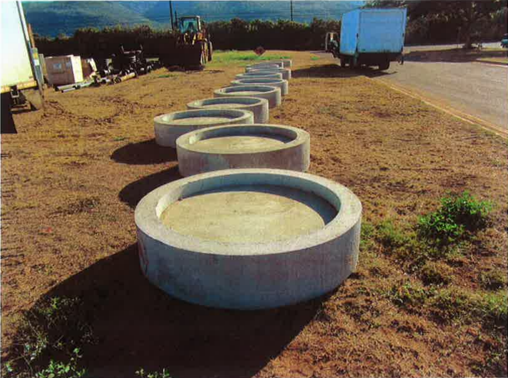
Photo 88. Prepared concrete lids ready for epoxy coating.
