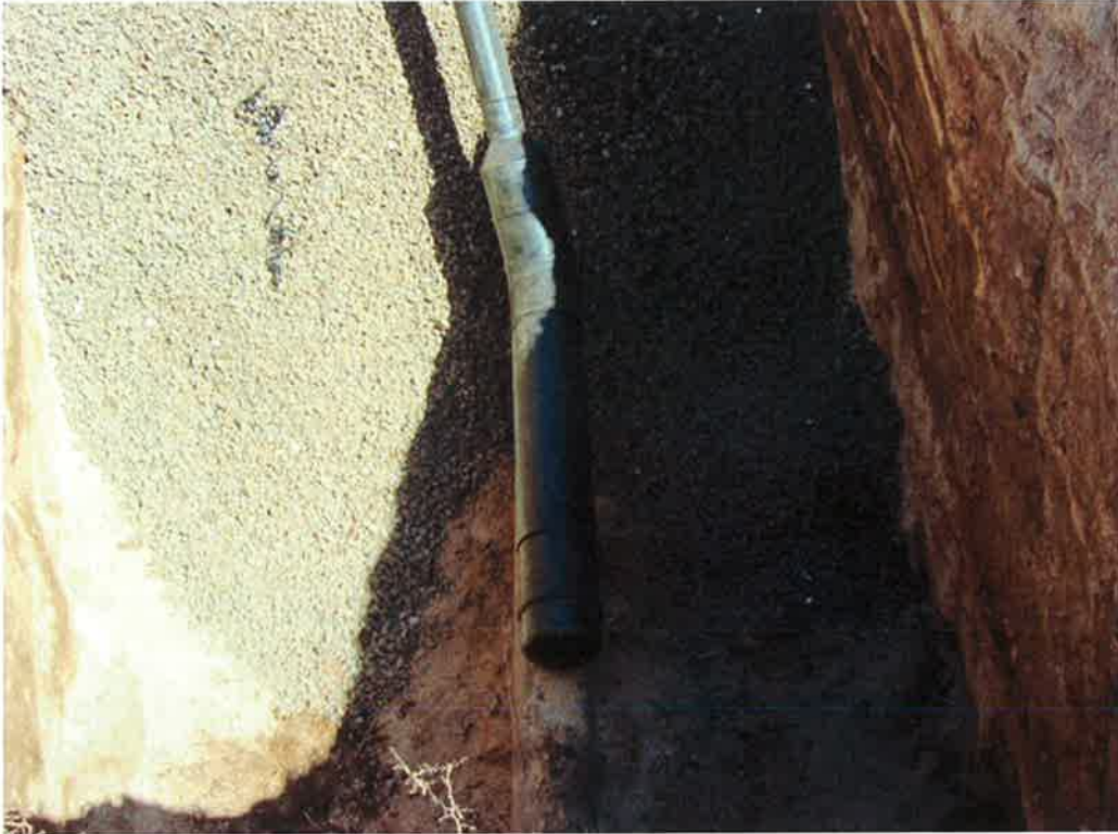
Photo 71. 6-inch HDPE pipe connection to connect the existing discharge to the new meter valve box.
