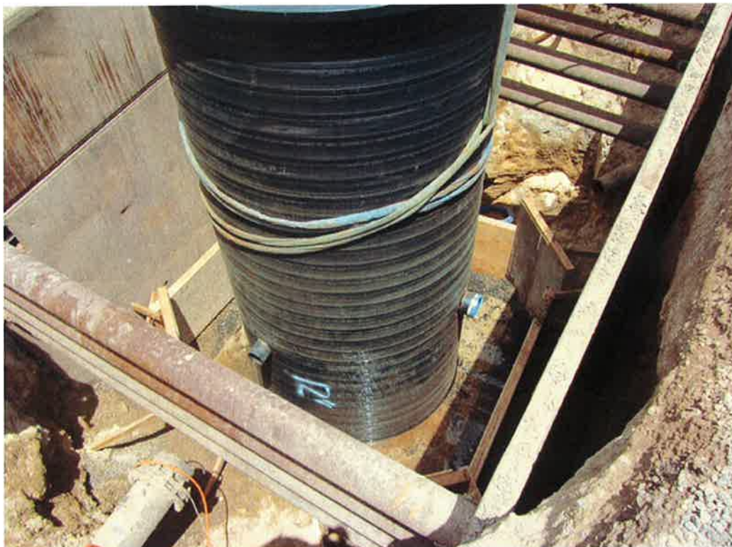
Photo 50. Installed form boards to construct the Wet Well #1 ballast system.
