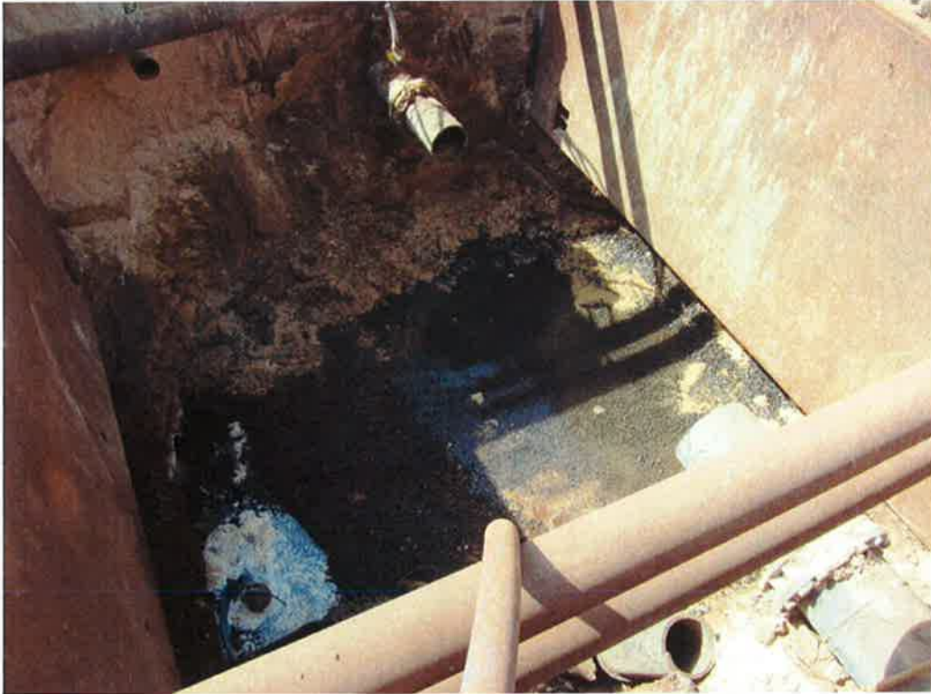
Photo 8. Gravel placement to achieve design grades for new Wet Well #2 placement.
