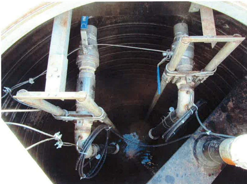
Photo 34. Installed pump and discharge piping in Wet Well #2 (later modified).
