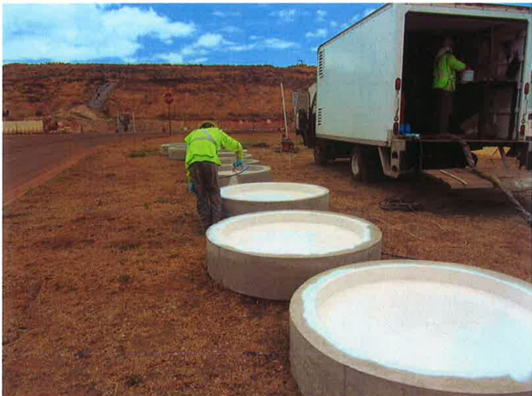
Photo 89. Epoxy coating to cover underside of the concrete lids.
