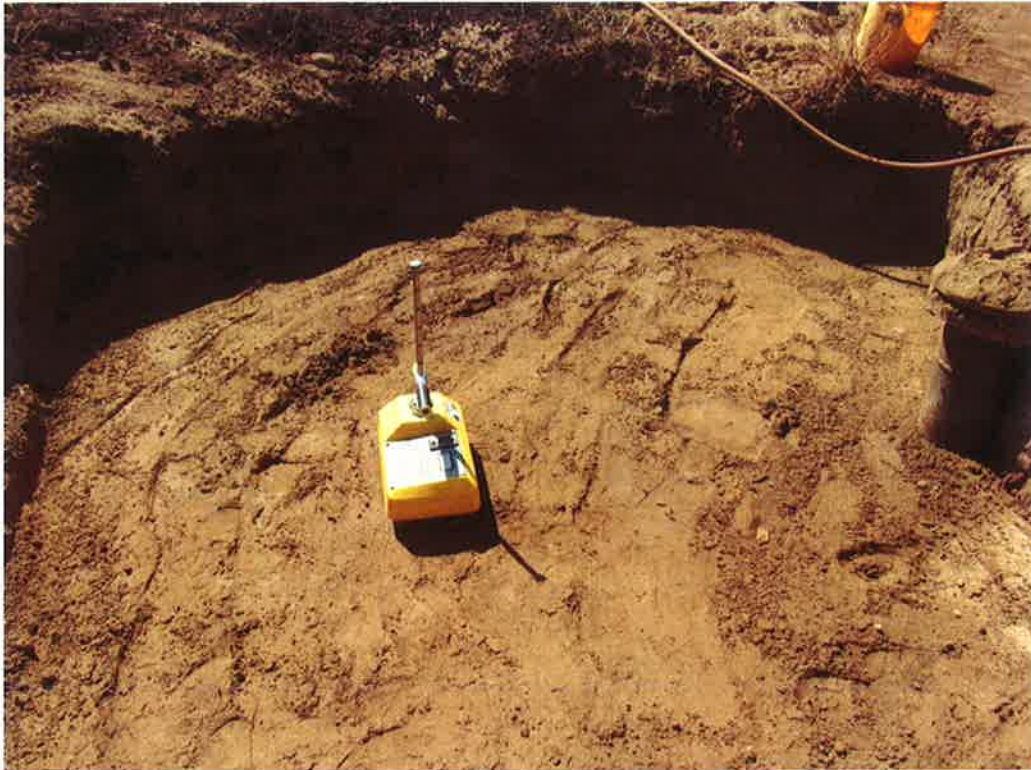
Photo 93. Troxler portable moisture/density gauge used to verify backfill above reinforced concrete lids
