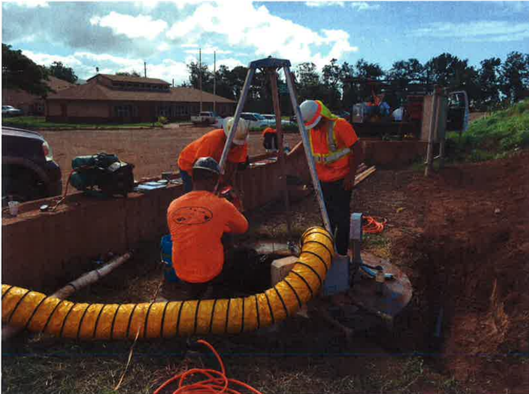
Photo 115. Preparing for confined space entry for pump replacement in Wet Well #2.
