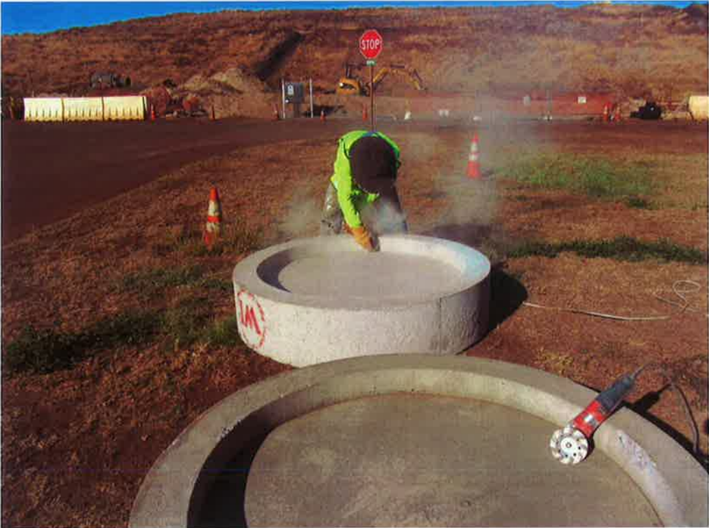
Photo 87. .Preparing precast concrete lids for epoxy coating.
