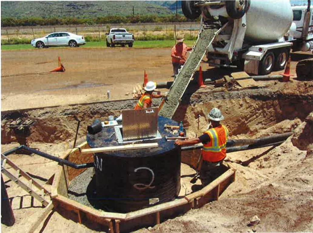
Photo 25. Concrete poured directly into prepared forms.
