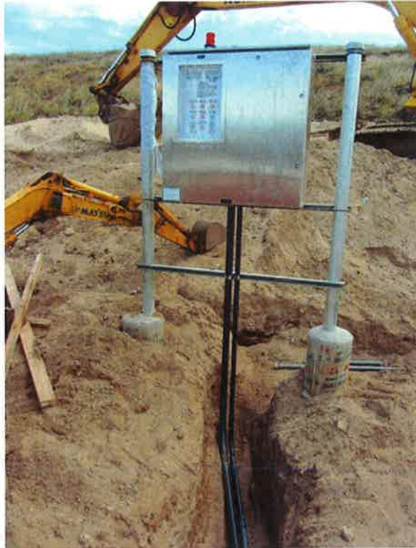
Photo 31. Newly installed Wet Well #2 control panel.
