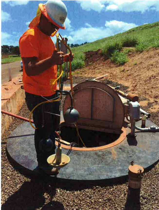
Photo 121. New float switch system installed in Wet Well #2 as back-up control for the High Alarm and Low Alarm/Shut-off transducer readings (typical).
