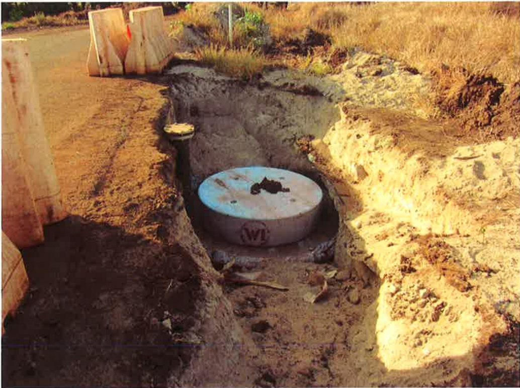
Photo 91. LCM 2-13 cover installation (typical).
