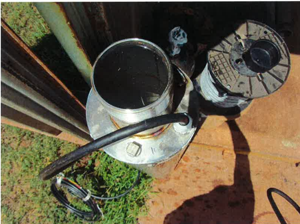
Photo 76. Check valve system verified within EPG pump system before installation (later removed)..
