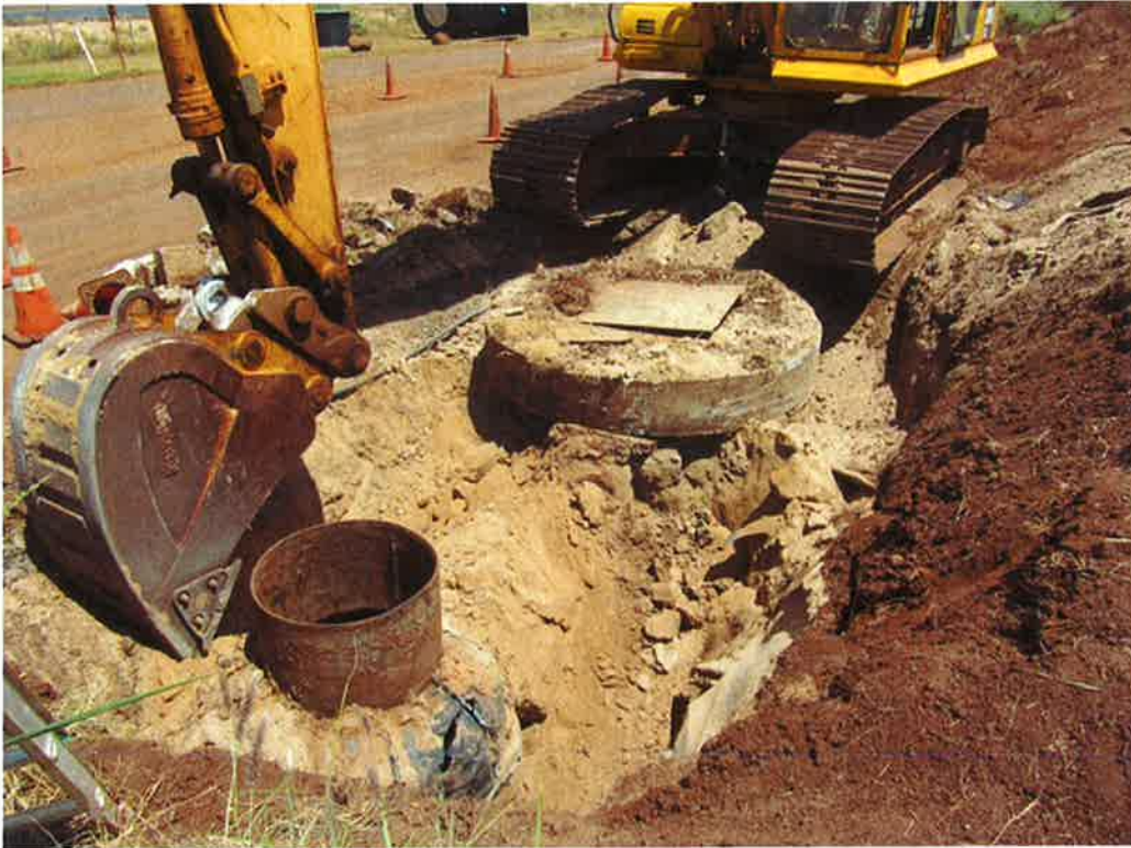
Photo 3. Excavation to remove existing Wet Well #2 and valve box.
