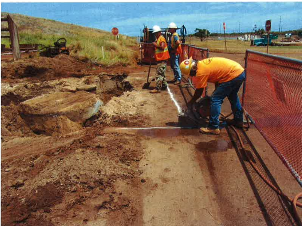
Photo 44. Saw cutting to remove existing asphalt paving to allow for access of the trench box shoring.
