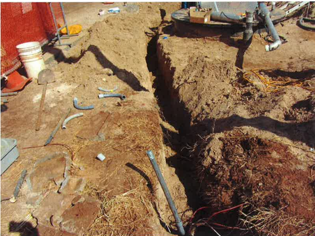
Photo 30. Electrical conduit and trenches for the new Wet Well #2 control panel.
