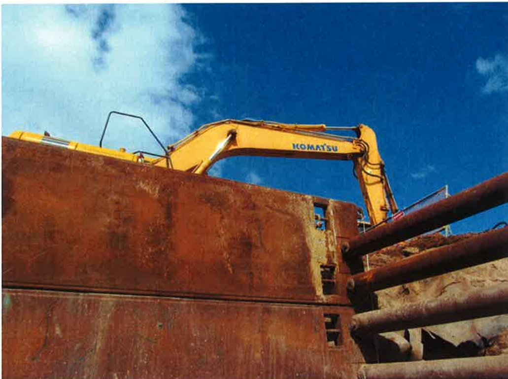
Photo 48. Trench box shoring to provide access during installation of the new Wet Well #1.
