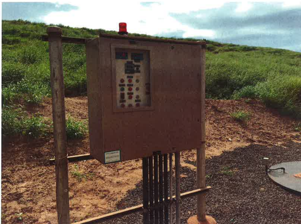
Photo 120. Exterior of Wet Well #2 control panel (typical).
