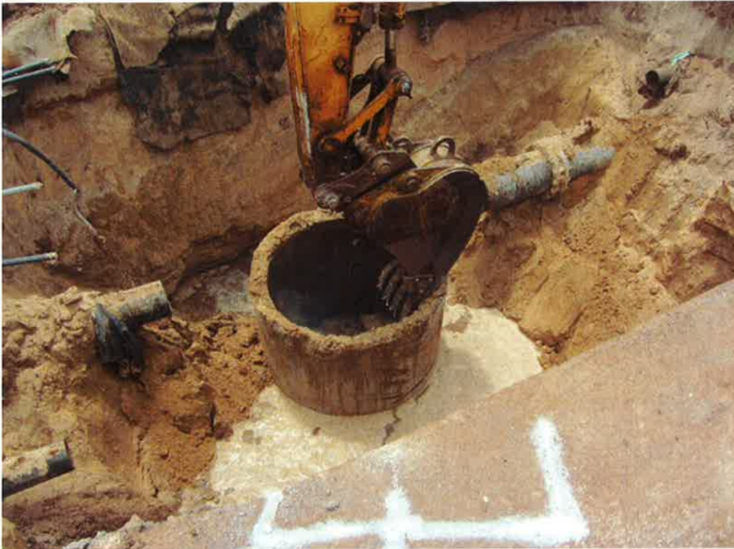
Photo 6. Removal of the existing lower section of Wet Well #2.
