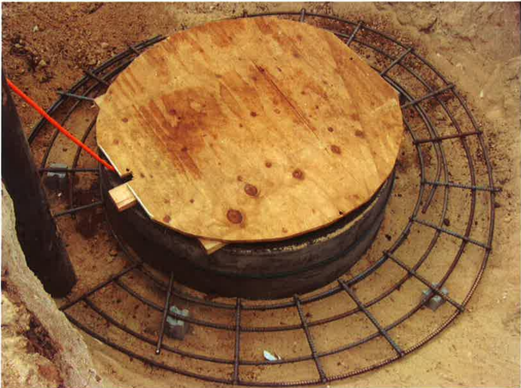
Photo 84. . LCM 2-13 foundation footing reinforcing and water stop to support precast concrete cap (typical).
