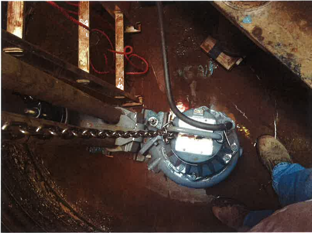
Photo 118. Stainless steel lifting chain connected to new Flygt pump in Wet Well #1 (typical).
