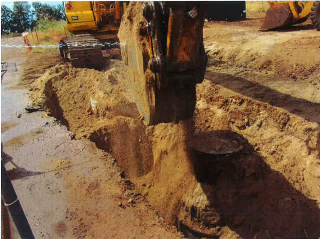
Photo 43. Excavation to remove the existing Wet Wet#1 and existing valve box.
