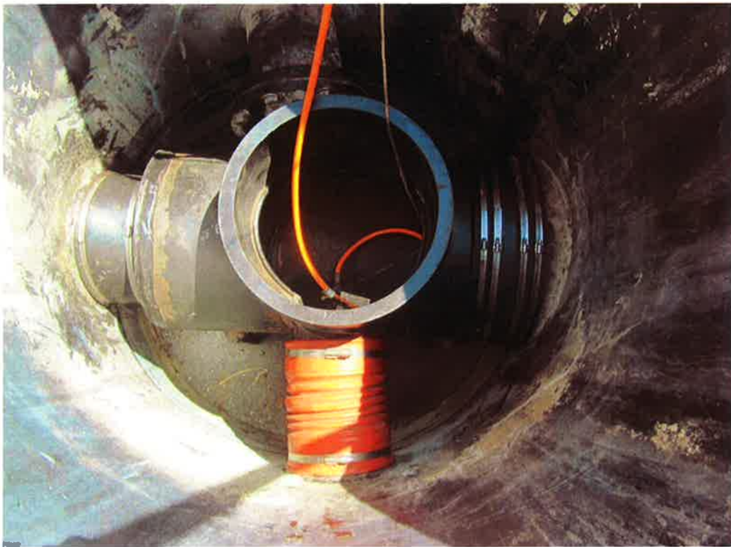
Photo 106. LCM 12 modification with isolation plug prior to installation of Fernco cap.
