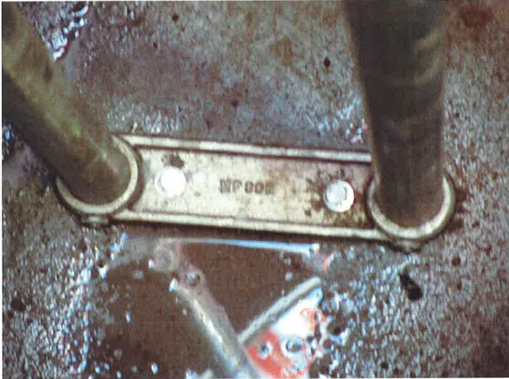
Photo 33. Wet Well #2 lower rail system support bracket bolted to poured concrete floor (later removed)
