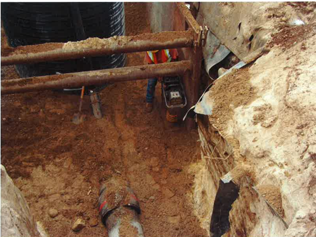
Photo 66. Wet Well #1 backfill using onsite sand.
