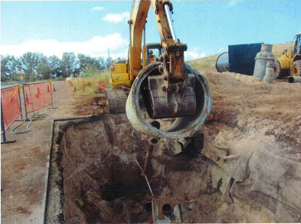
Photo 47. Removal of the existing concrete Wet Well #1 assembly using an excavator.
