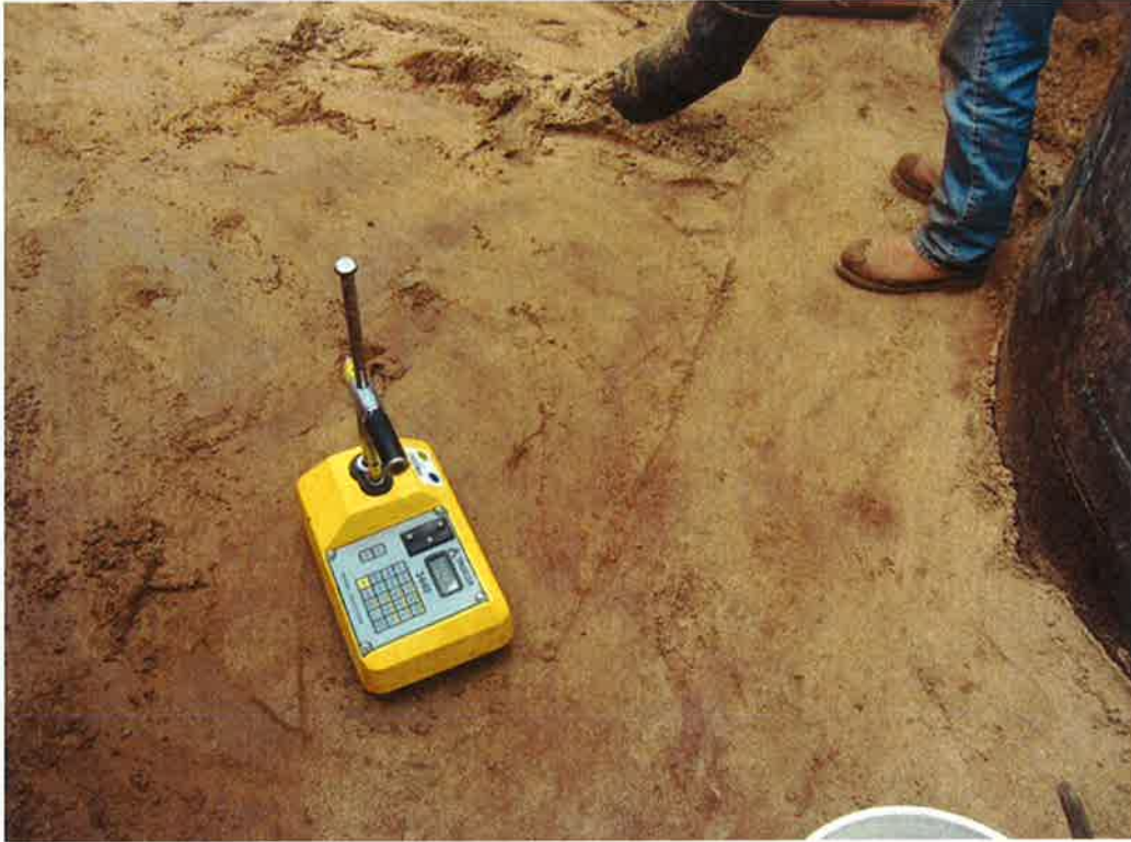
Photo 67. Field density tests using a Troxler portable moisture/density gauge.
