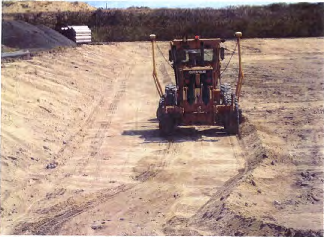
Photo 5. Motorgrader removes the approximate top 6 inches of subgrade soils (looking south)
