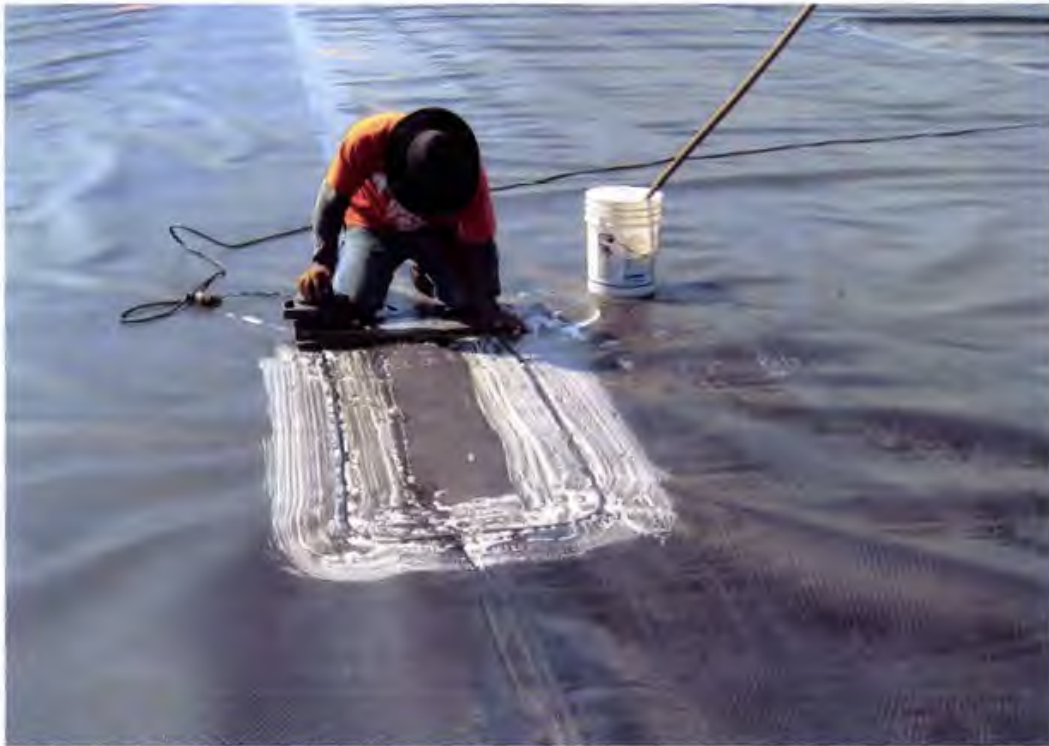
Photo 113. Non-destructive vacuum box testing the extrusion seam of a repair patch for a destructive seam sample locations
