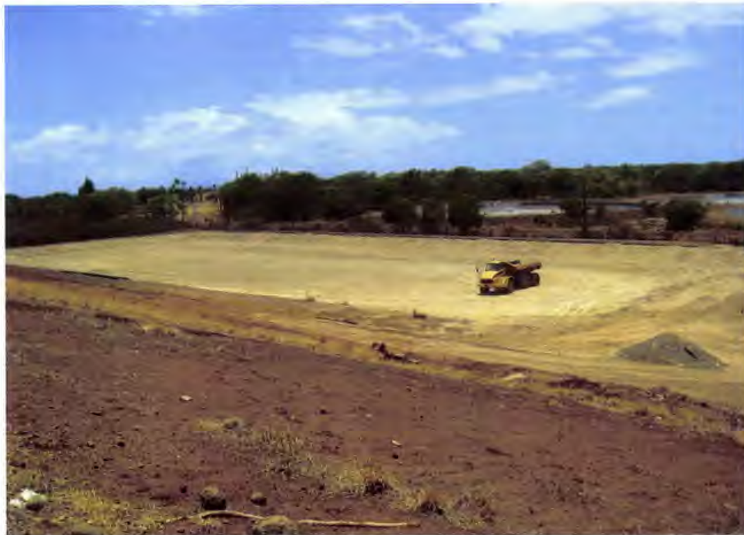
Photo 2. Cells 1A/1B existing subgrade, after demolition of the former leachate pond (looking southwest)
