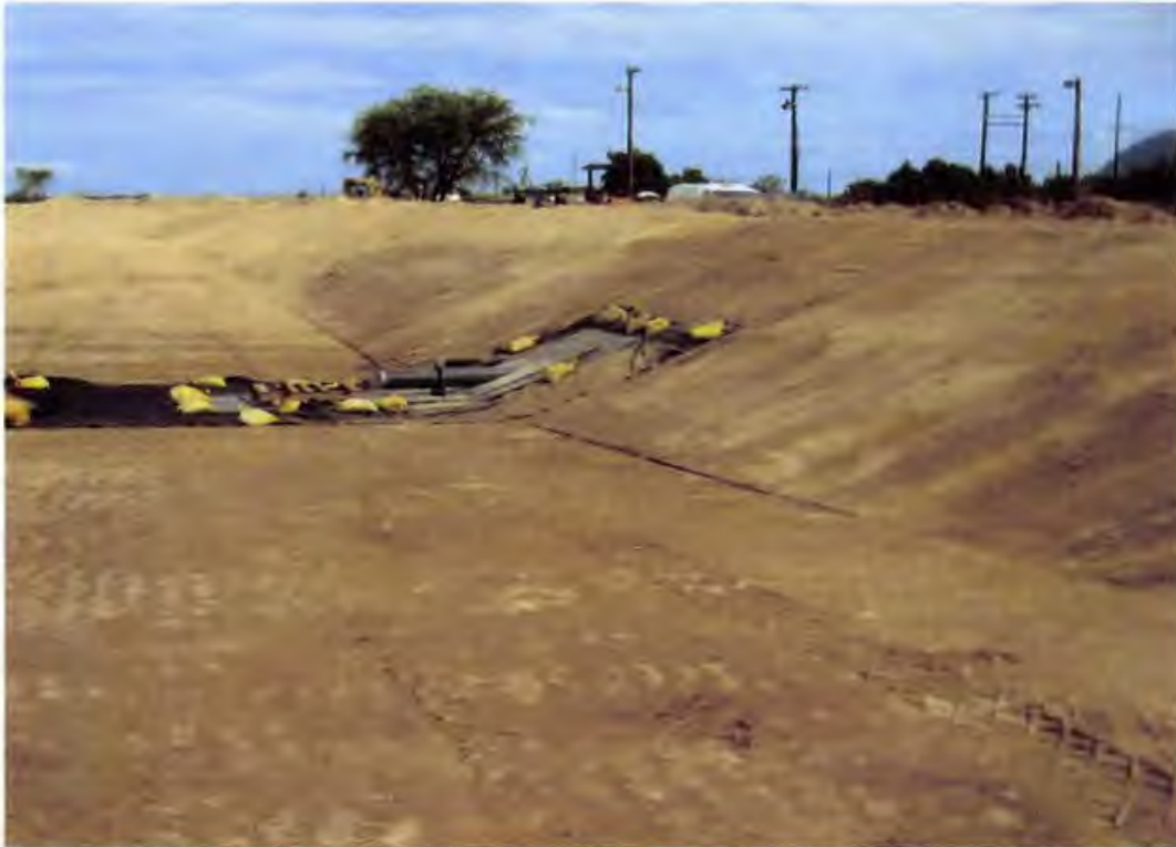
Photo 73. Prepared subbase on side slopes (looking west along Cell 1D north sideslope)
