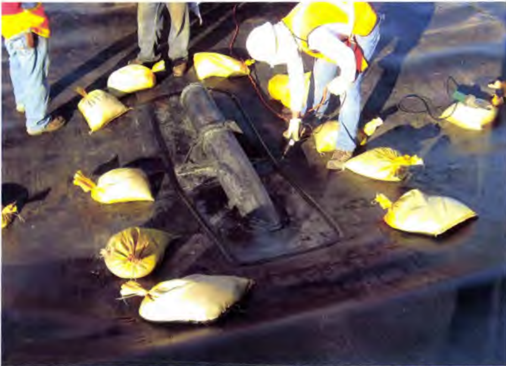
Photo 111. The embedded copper wire provides a mean to spark test the weld to verify integrity
