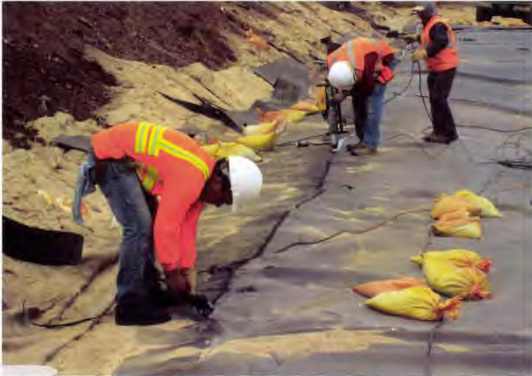
Photo 109. Extrusion welding the primary 60 mil HDPE geomembrane to the existing Phase II geomembrane; the seam is abraded prior to applying the extrusion bead (looking south)
