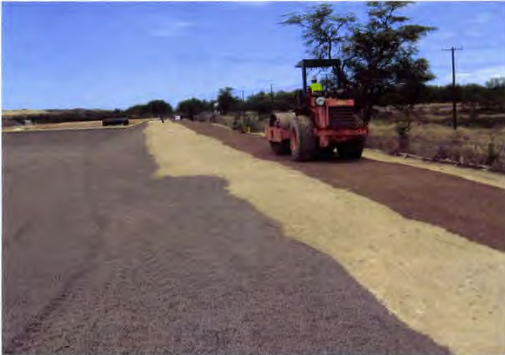
Photo 133. Compacting 9-inch-thick crushed aggregate for perimeter access road using a HAMM smooth drum vibratory compactor (looking south)
