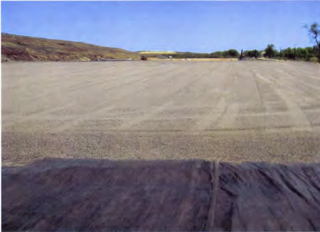
Photo 129. Completed operations layer material (looking south)
