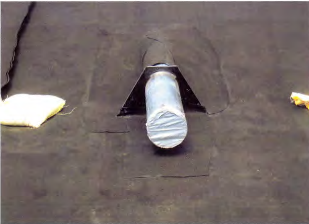
Photo 118. 16 oz/sy nonwoven cushion geotextile around sump pipe penetration
