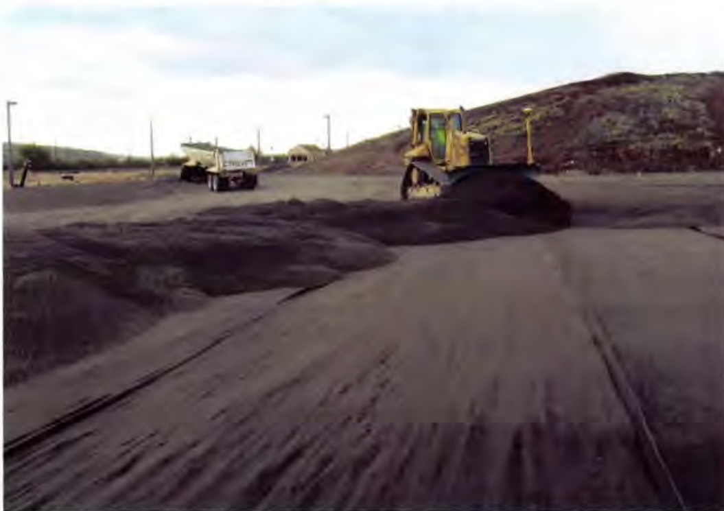
Photo 128. An LGP D5 dozer spreads and grades the placed operations layer material to 2-ft thick (looking east)
