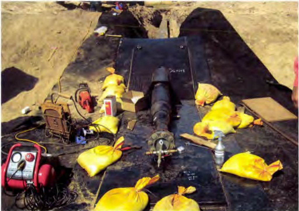
Photo 48. All connected penetrating pipes are pressure tested prior to final connection to Wet Well #3 or LCM-14
