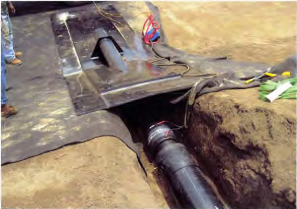
Photo 47. The dual containment (8"φ x 12"φ) pipes are connected to the sump pipe penetration using electro-fusion couplers
