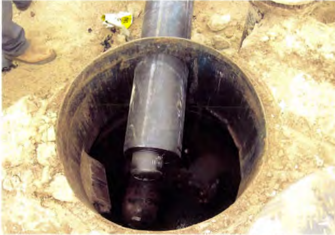
Photo 57. The dual containment (4"φ x 8"φ) forcemain pipe penetrates LCM-14 above the Cell 1D dual containment (8"φ x 12"φ) pipe
