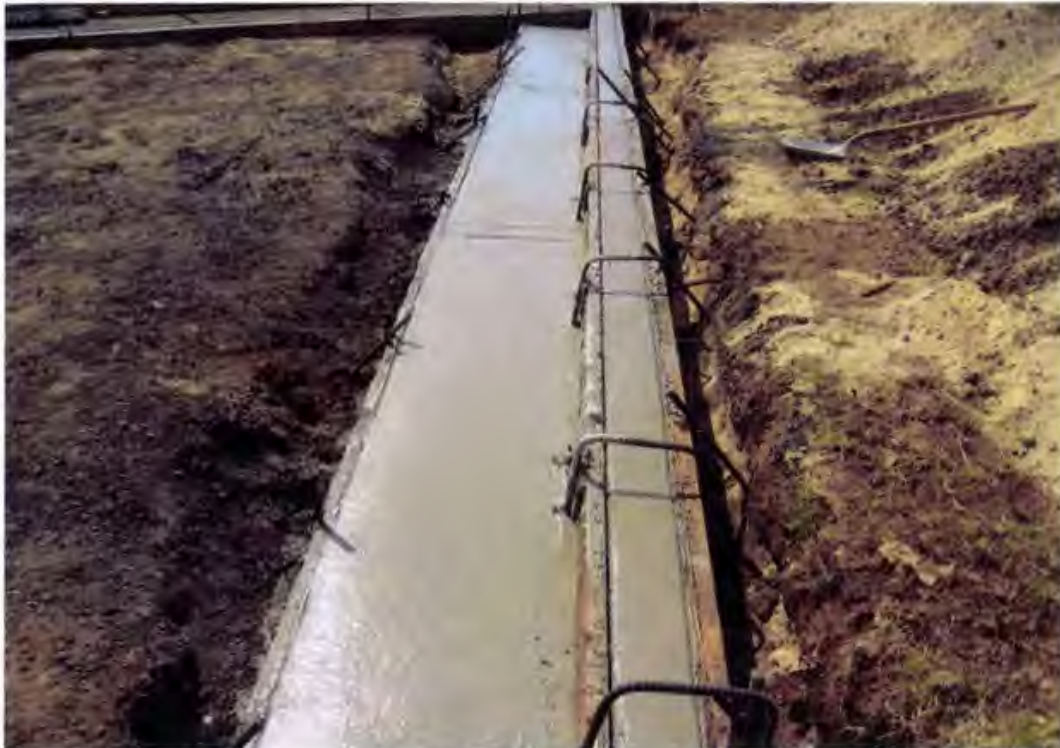
Photo 147. New concrete curb
