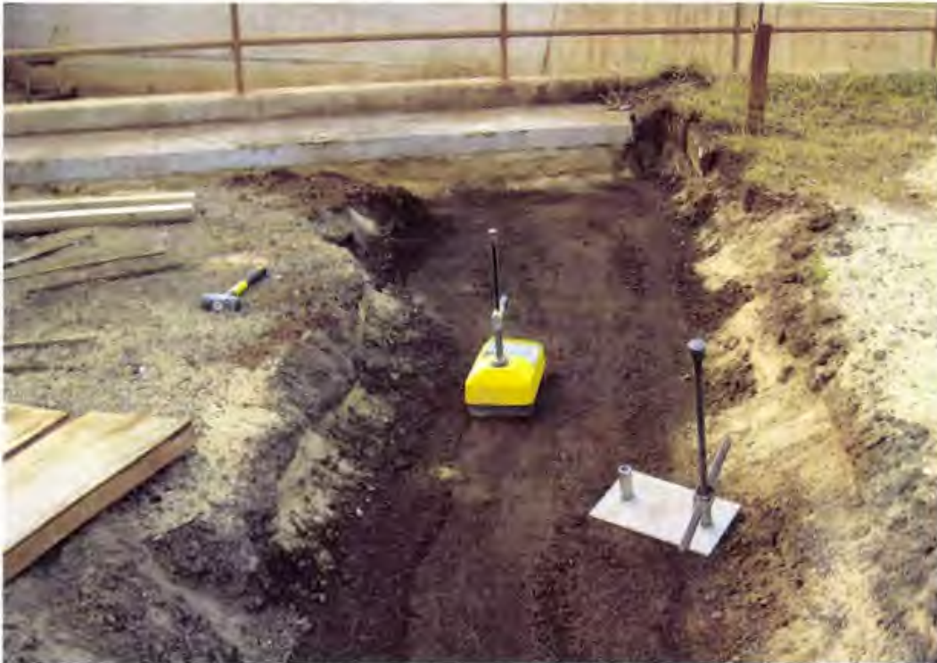
Photo 145. Field tests performed using a nuclear moisture density gauge verifies the compaction effort of 18" aggregate base course
