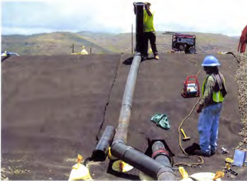
Photo 123. Sump pipe penetrations are connected to the wye assemblies and cleanout risers using an electro-fusion coupler. Wye assemblies are fusion-welded to the perforated LCRS pipes
