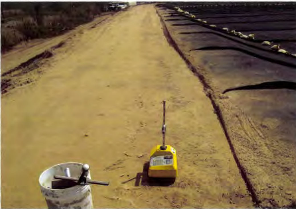
Photo 120. Verifying anchor trench backfill compaction effort using a nuclear moisture density gauge (looking north)
