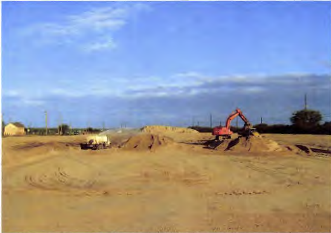
Photo 7. Onsite trimmings from the new leachate evaporation pond (NLEP) construction are also used to construct the Cell 1 subbase grades (looking west)
