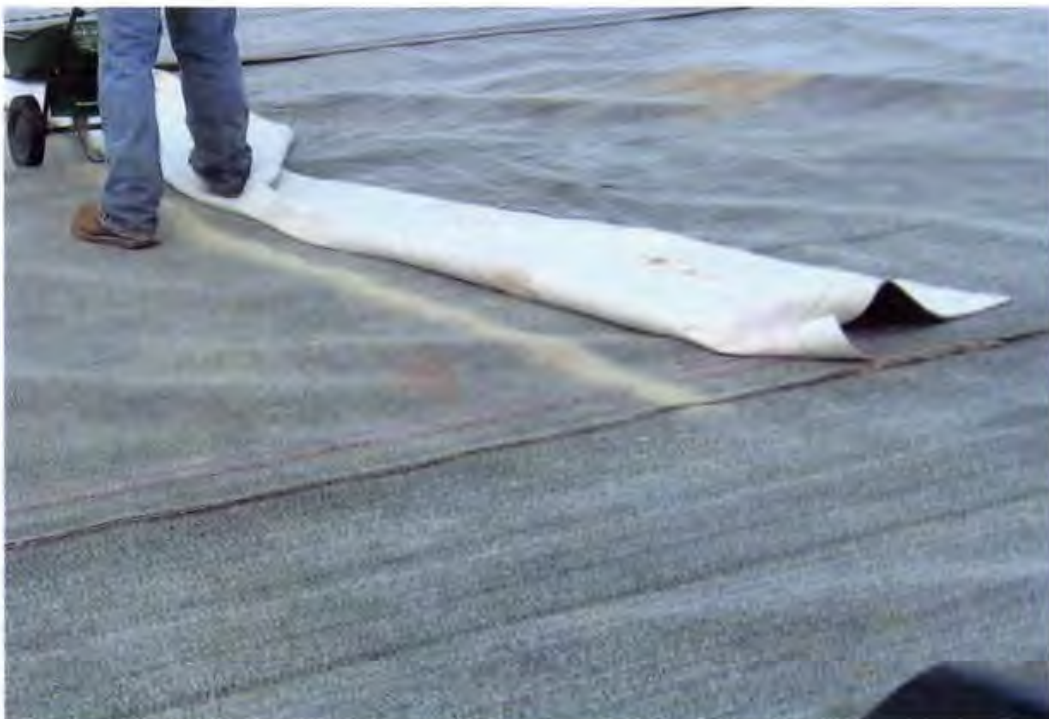
Photo 104. GCL panels are overlapped 12 inches minimum along the width and 6 inches minimum along the length. Granular bentonite is placed along the width (butt) seam, and a "super-groove" factory seam is along the length seam
