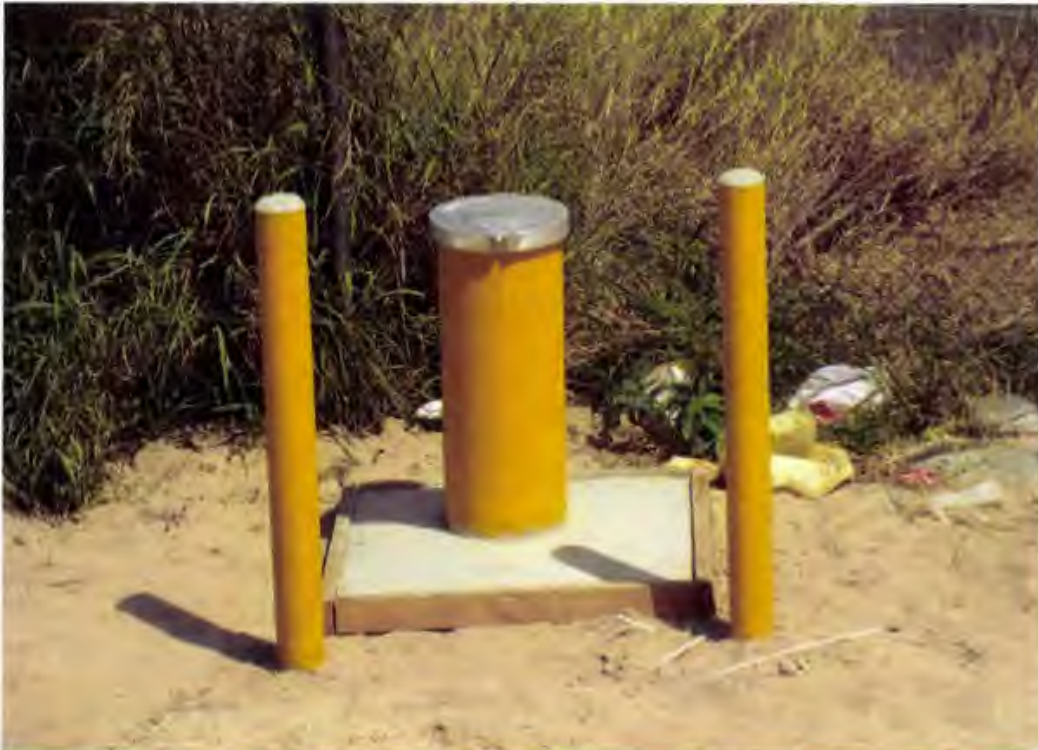
Photo 137. Completed gas monitoring probe with concrete pad and protection posts
