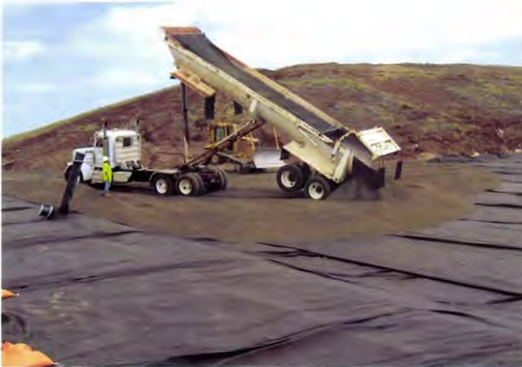
Photo 127. 3/8-inch minus operations layer material (from Kauai Aggregate Quarry) is placed directly onto the floor above the completed 6 oz/sy nonwoven separator geotextile (looking southeast)
