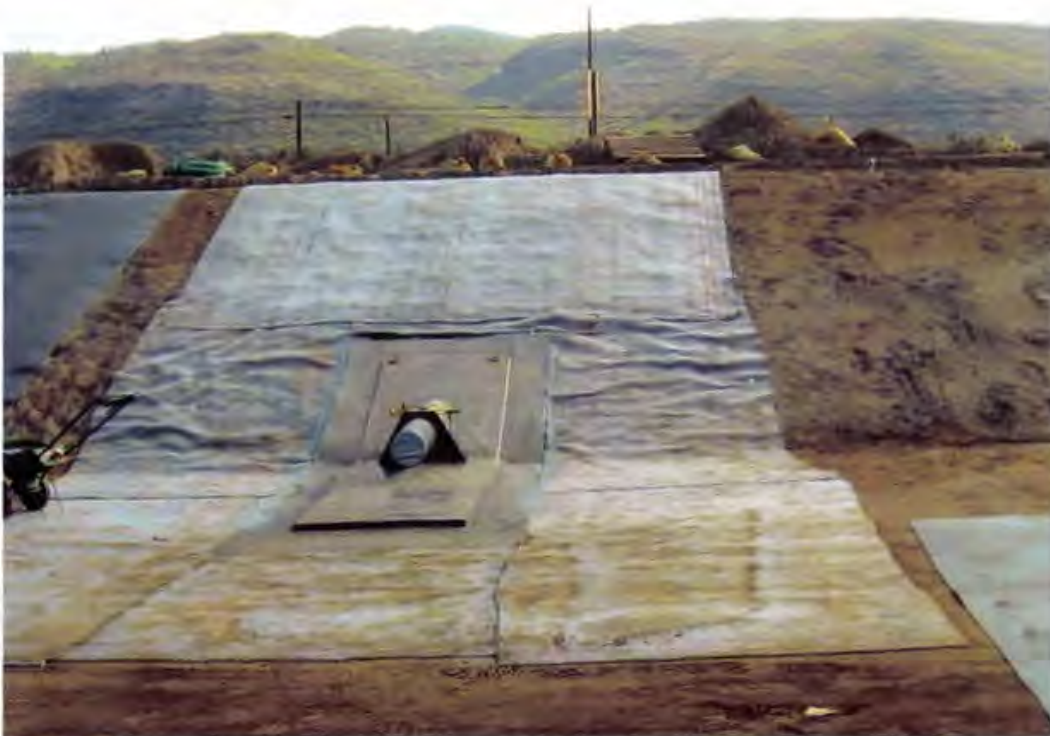
Photo 54. A layer of GCL is installed around the pipe penetration assemblies, below the subbase HDPE geomembrane for transition to pipe penetration flatstock (looking north)
