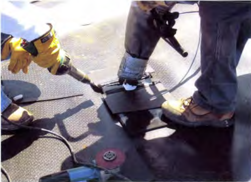
Photo 85. Preparing an extrusion trial weld of textured 80 mil HDPE geomembrane to 1/2-inch thick HDPE flatstock
