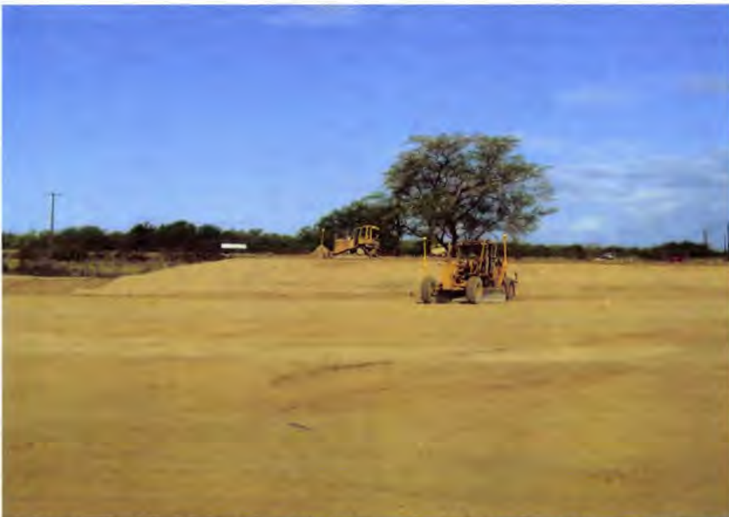
Photo 20. The Cat. 140H motor grader and Cat. D5 dozer (both with GPS control) fine grade Cells 1C/1D (looking west)
