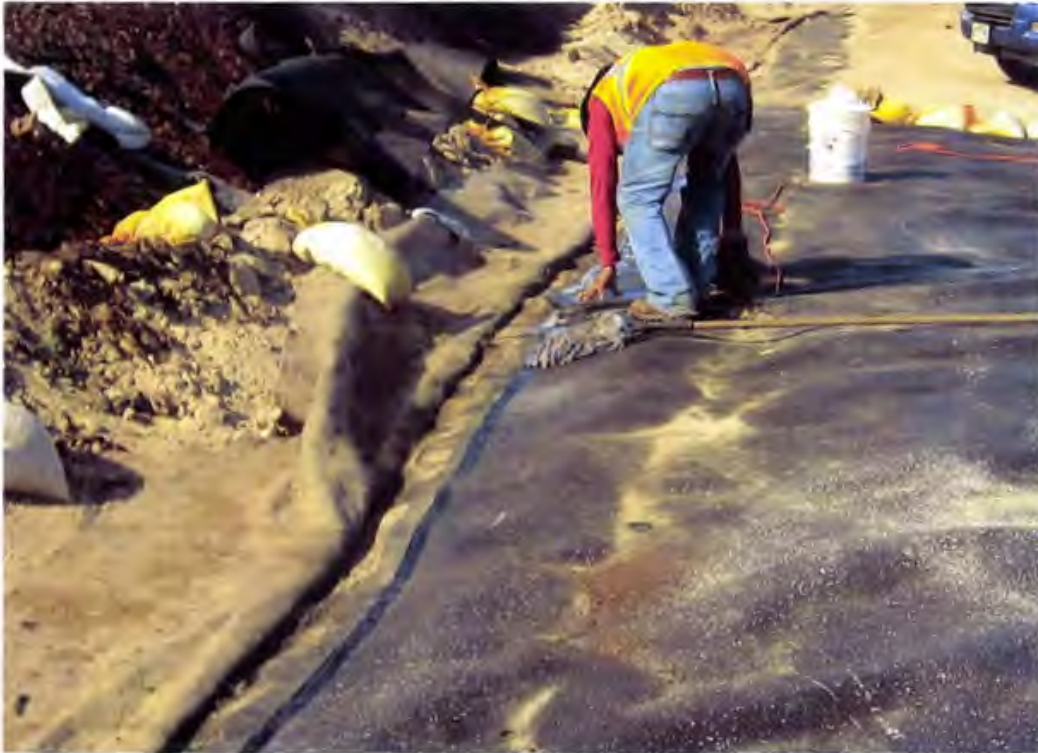
Photo 93. Non-destructive vacuum box testing extrusion welded seams
