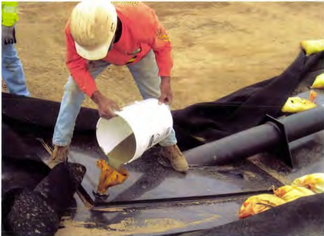
Photo 53. Bentonite grout is used to fill the 1-inch void within the penetration assemblies
