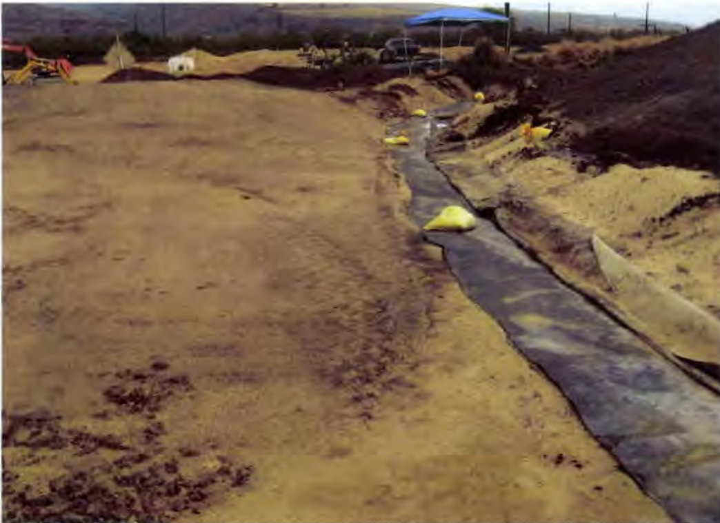
Photo 70. Northwest corner of existing Phase II containment system exposed for tie-in (looking north)
