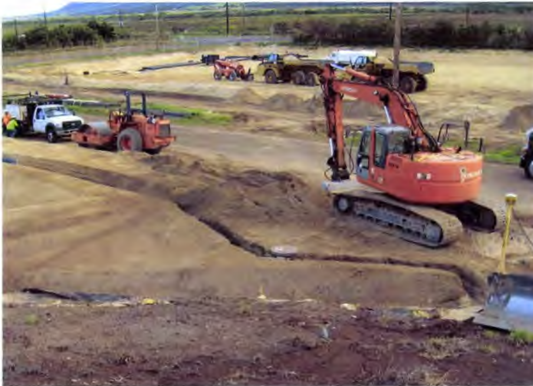
Photo 75. Field fitting subbase grades at far northeast corner of Cell 1D (looking northwest)
