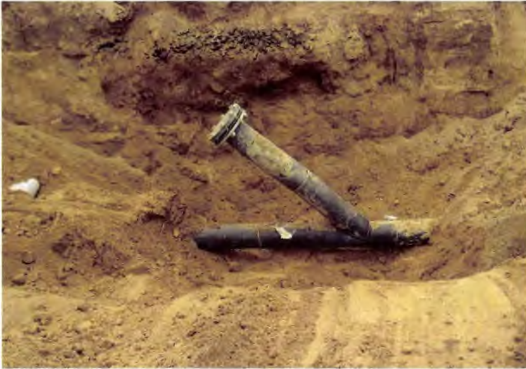
Photo 21. Existing forcemain cleanout located at the northeast end of Cell 1D (as shown on Drawing 2 of the Construction Drawings)
