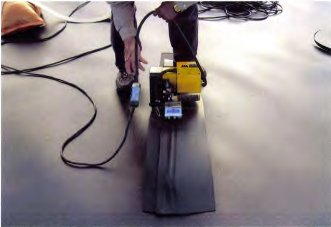
Photo 83. Trial welds are prepared at the start of the day and at midday for each welding apparatus and material combination used that day (fusion welding textured-to-textured 60 mil HDPE geomembrane shown above)
