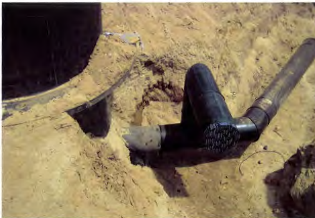
Photo 42. Dual containment (8"φ x 12"φ) HDPE pipe from Wet Well #3 to connect to Cell 1B sump
