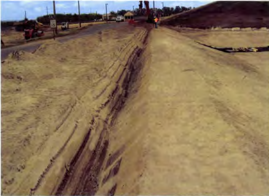
Photo 77. V anchor trench along Cells 1C/1D perimeter berm (looking south)
