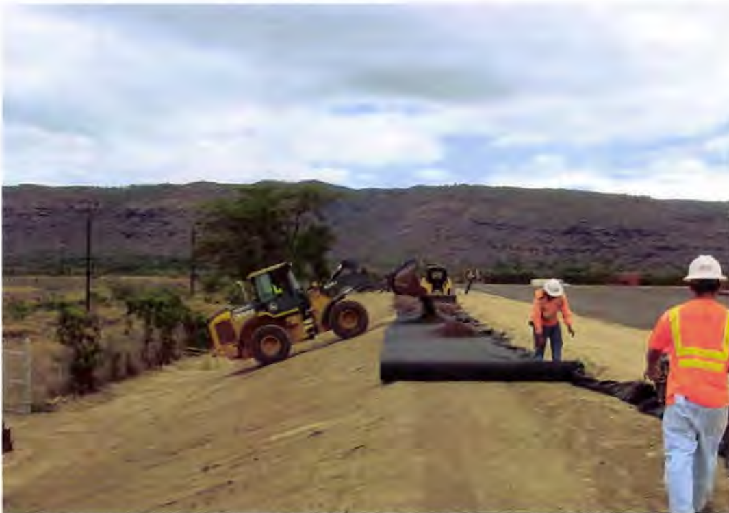
Photo 132. Separator geotextile for the perimeter access road is placed along the outer portion of the berm before placement of the crushed aggregate base course for the perimeter maintenance road (looking north)
