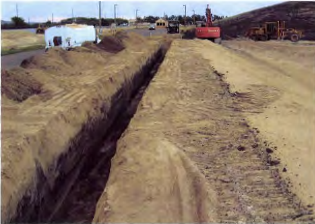
Photo 55. Trench along Cells 1C/1D perimeter berm for the dual containment (4"φ x 8"φ) HDPE forcemain pipe from the new Wet Well #3 to LCM-14 (looking east along Cell 1D north berm)
