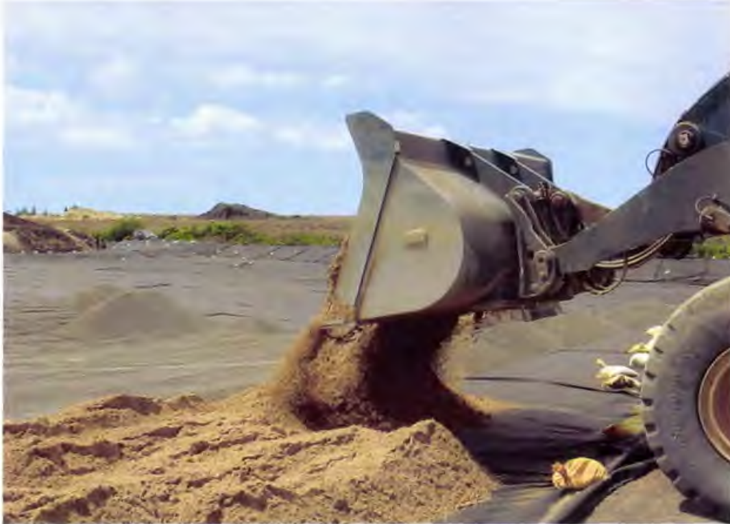
Photo 131. General fill (onsite soils) is placed along the inner crest of the Cell 1 perimeter berm (looking southwest)
