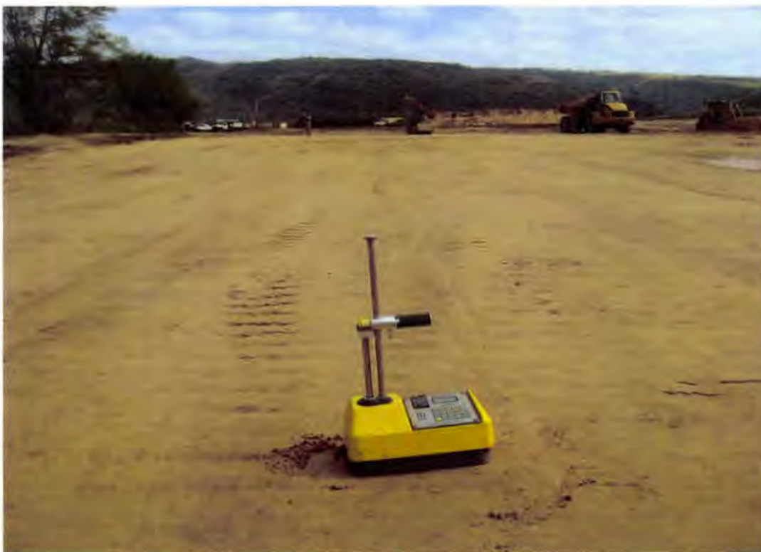
Photo 12. Verifying compaction effort using a Troxler portable nuclear moisture density gauge (looking north)
