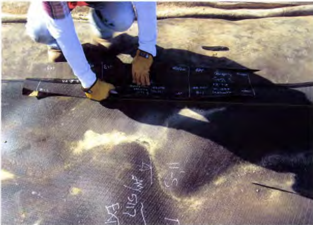
Photo 95. Destructive seam sample collected on the subbase tie-in to Phase II containment system
