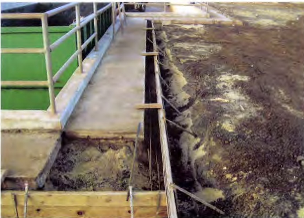
Photo 146. Form work and reinforcing steel bars are constructed in preparation for new concrete
