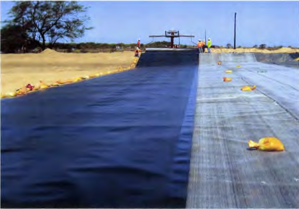
Photo 107. Primary 60 mil HDPE geomembrane is deployed over GCL panels
