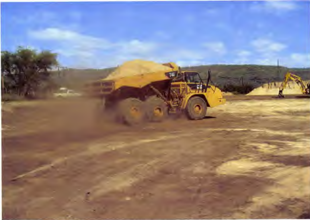
Photo 5. A fully loaded Caterpillar (Cat.) 740 haul truck drives over the existing subbase to verify that the subbase is firm and non-yielding (looking north)
