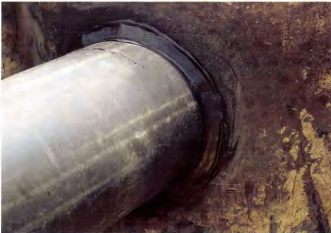
Photo 58. Dual containment (4"φ x 8"φ) forcemain pipe connects to LCM-14. Outer pipe is extrusion welded to the manhole
