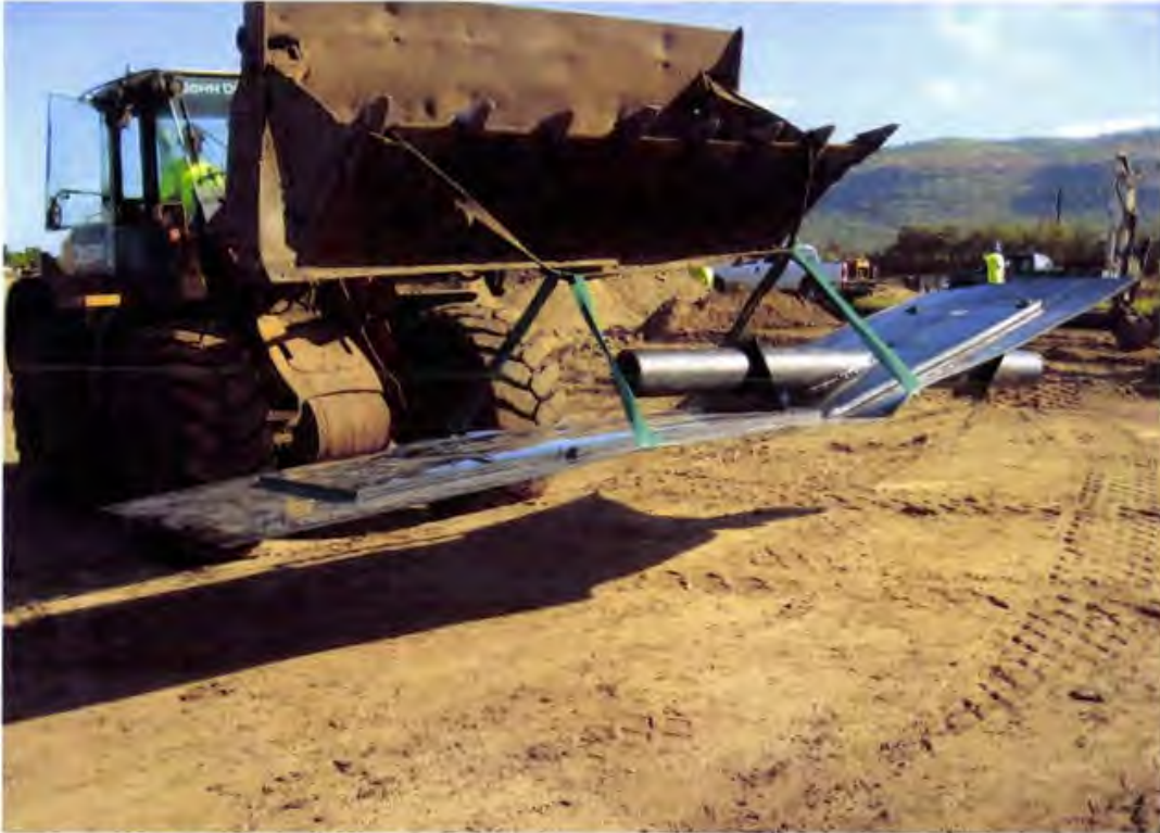
Photo 35. Typical factory-welded HDPE pipe penetration assembly used for each of the Cells 1A through 1D sumps
