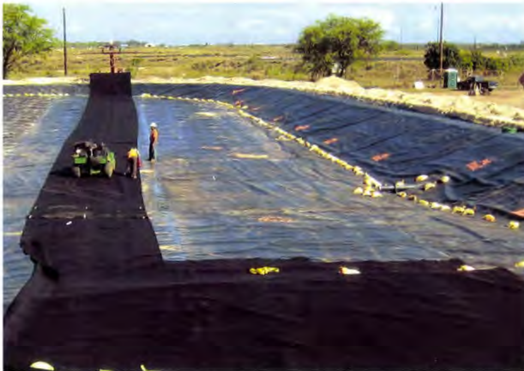
Photo 114. Installing 16 oz/sy nonwoven cushion geotextile above the approved primary 60 mil HDPE geomembrane (looking west)
