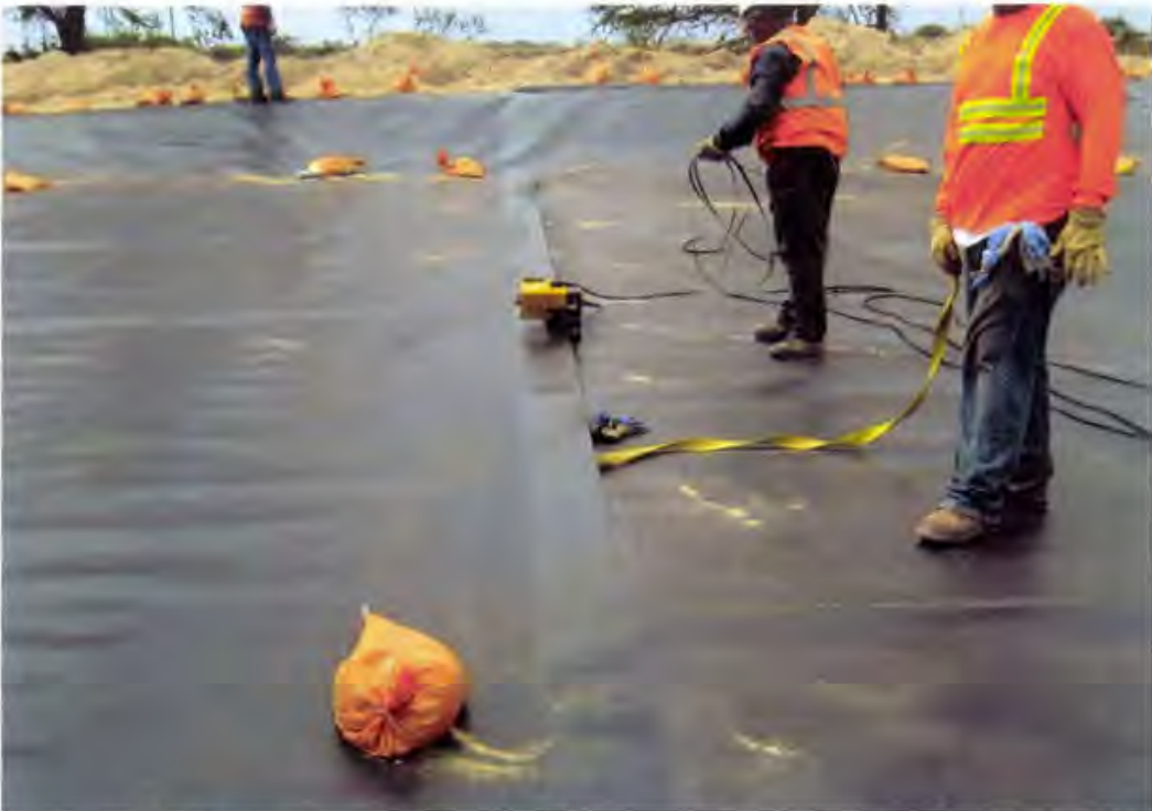
Photo 88. Production seaming subbase 60 mil HDPE geomembrane using a double-fusion wedge welder
