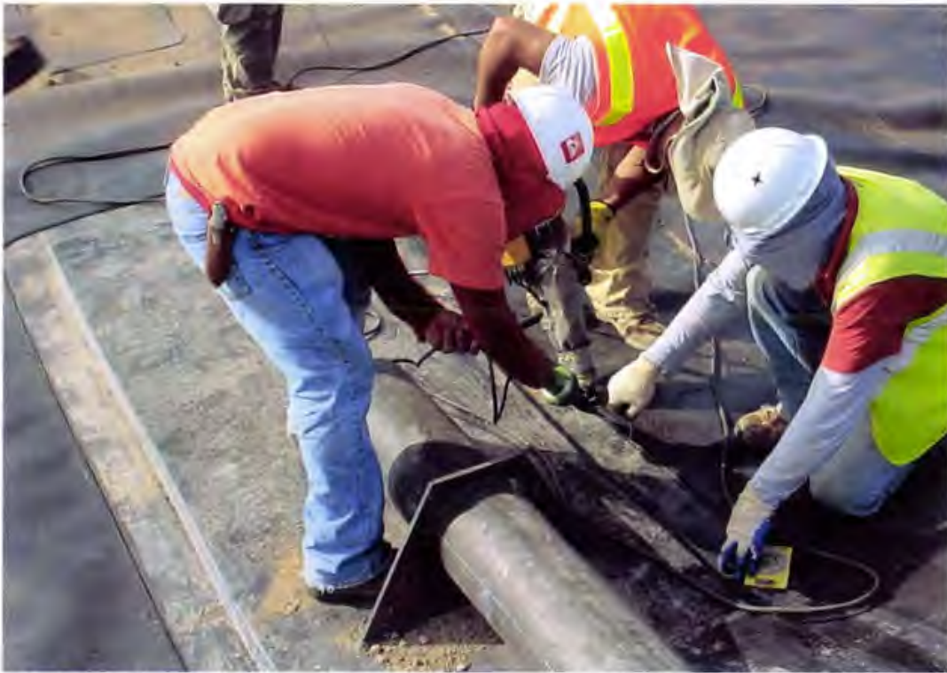
Photo 91. Subbase 80 mil HDPE geomembrane panels are extrusion welded, with an embedded copper wire (for spark testing), to the ½-inch thick HDPE flatstock of the pipe penetration assemblies
