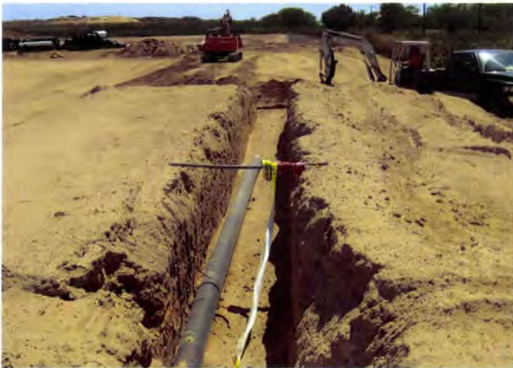
Photo 56. Installed dual containment (4"φ x 8"φ) forcemain pipe (looking south)
