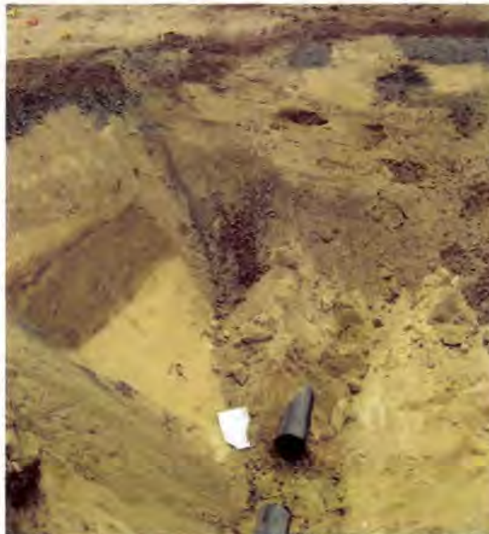
Photo 24. The existing forcemain pipe (from former leachate pond to existing valve box #2) cut at southwest end before Cell 1B (shown above) and at east end before valve box #2
