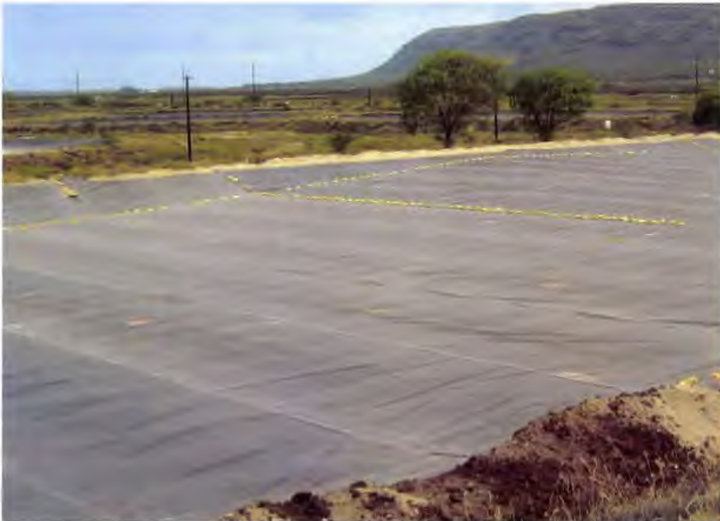
Photo 99. Completed subbase HDPE geomembrane (looking northwest)
