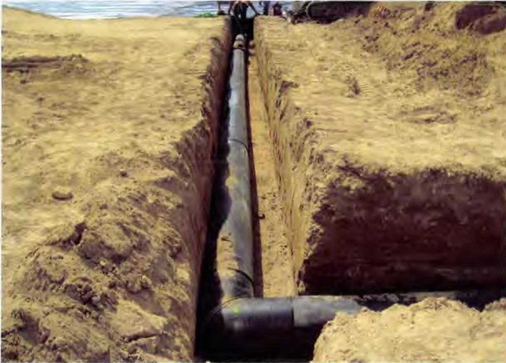
Photo 43. Installing the dual containment (8"φ x 12"φ) HDPE conveyance pipe from Cell 1C sump penetration to new Wet Well #3 (looking east)
