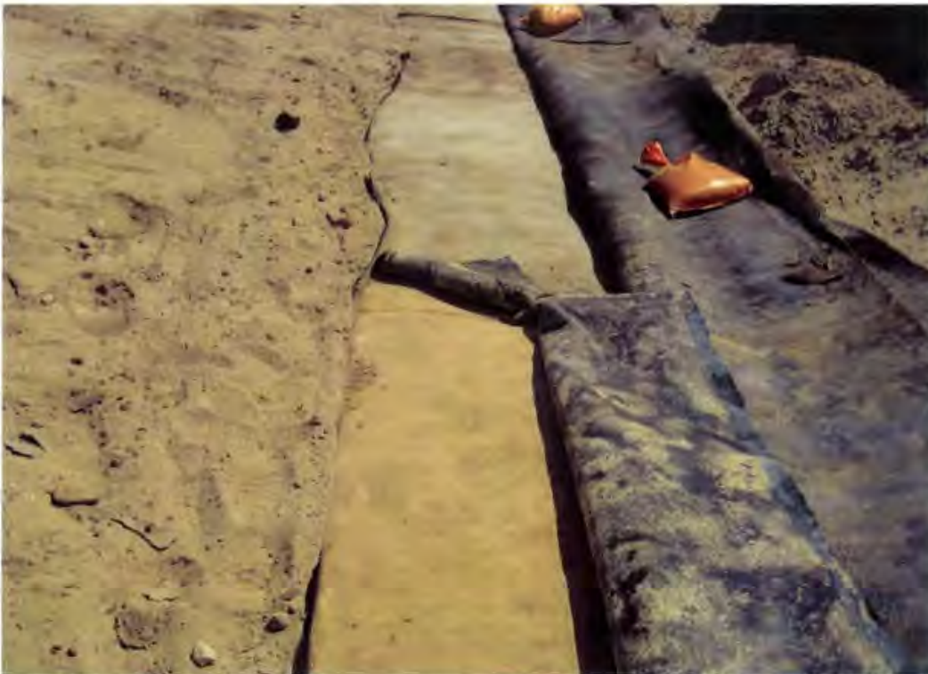
Photo 68. Existing Phase II containment system consists of 60 mil HDPE geomembrane overlying GCL (bentonite layer with geomembrane carrier, carrier side down)
