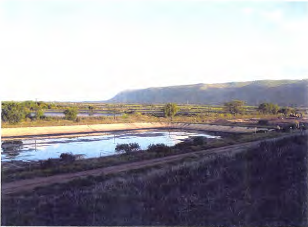
Photo 1. Existing leachate evaporation pond area prior to removal of leachate (looking northwest)
