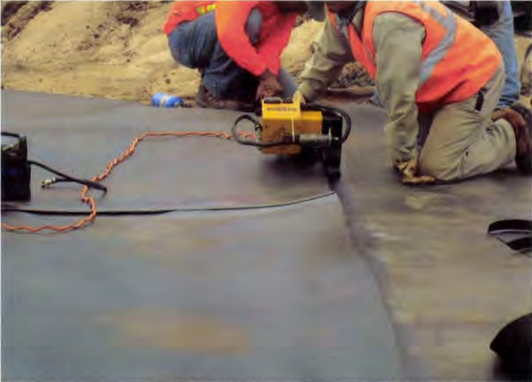
Photo 108. Production seaming primary 60 mil HDPE geomembrane using a double-track fusion wedge welder
