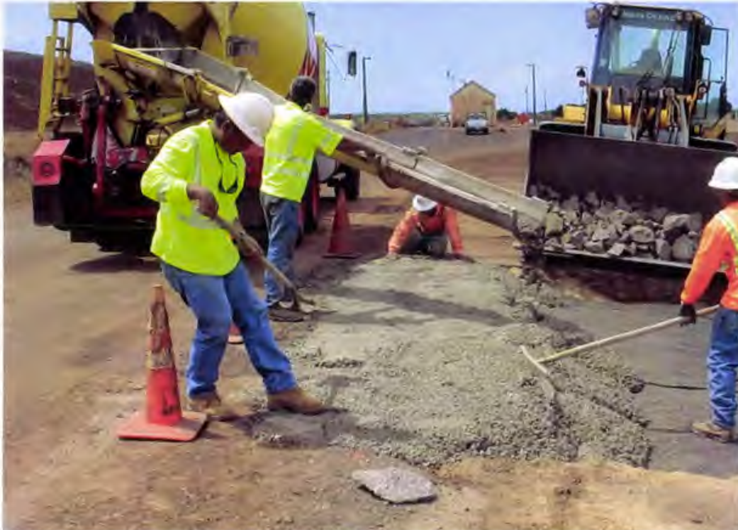
Photo 135. Concrete and rip rap being installed near south end of the infiltration ditch (looking west)
