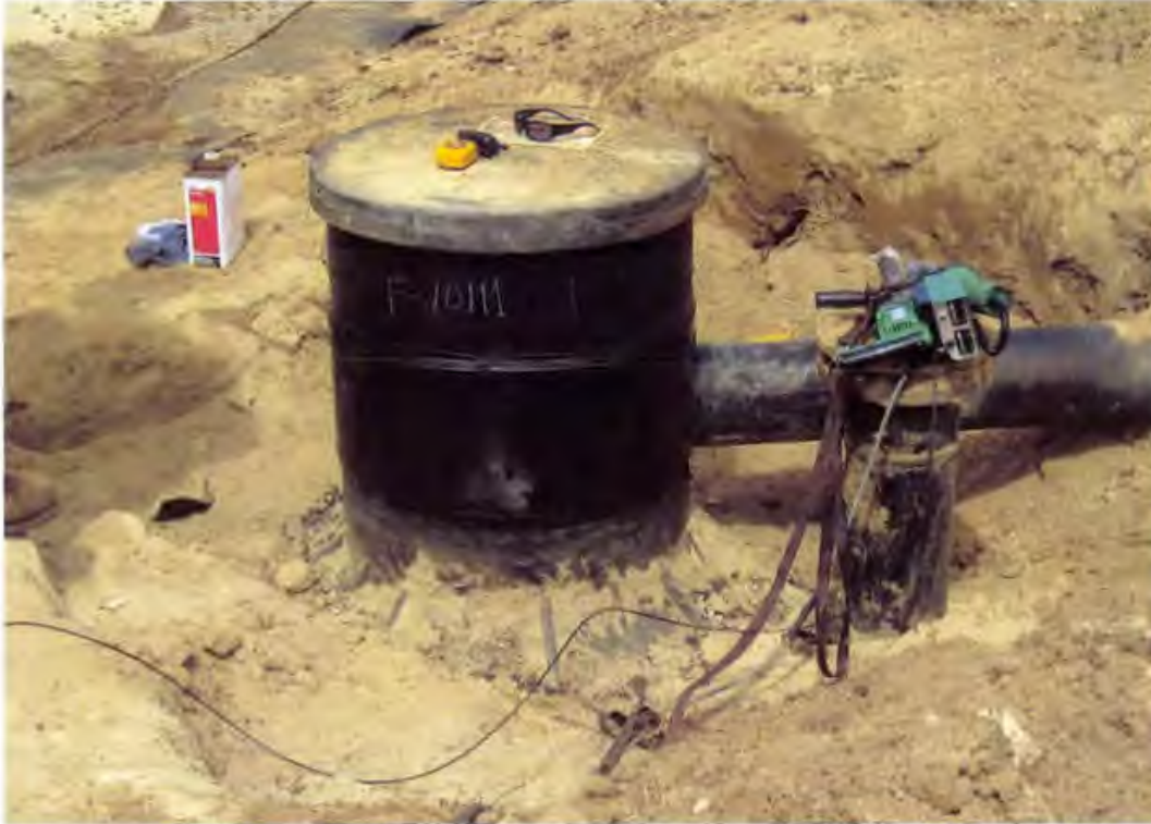
Photo 59. A prefabricated manhole section is extrusion welded to LCM-14 to extend the manhole above design grades
