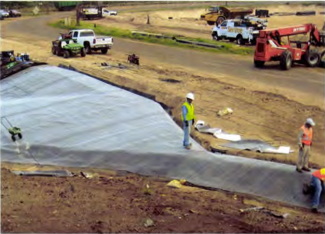
Photo 106. GCL panels at Cell 1D northeast corner (looking northwest)
