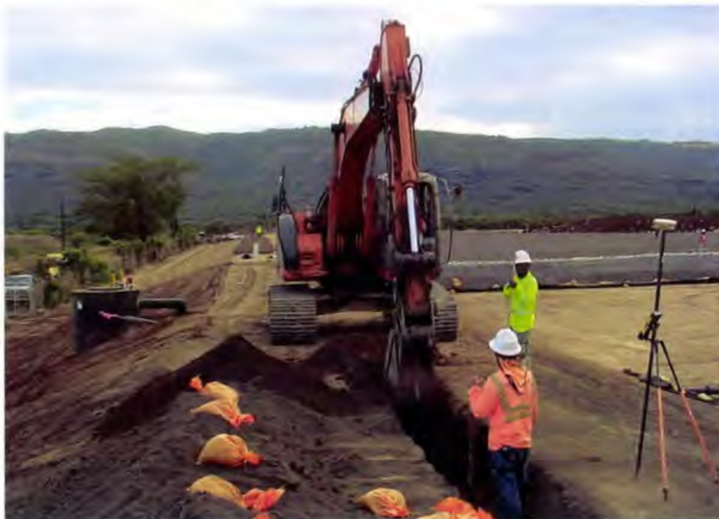
Photo 76. A Hitachi 450LC excavator constructs the 2'x2' square anchor trench along Cells 1A/1B perimeter berm (looking north)
