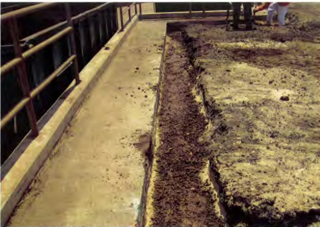
Photo 144. The excavation is backfilled with compacted new aggregate base course
