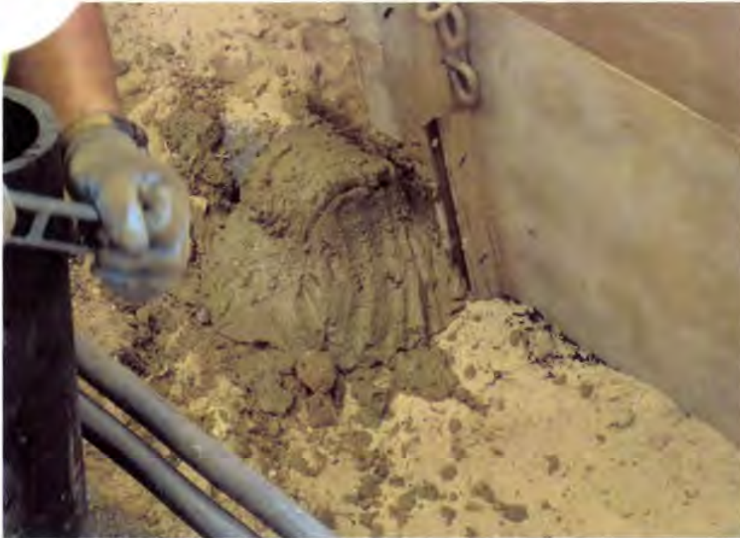
Photo 26. Ends of the existing forcemain pipe are plugged with cement grout
