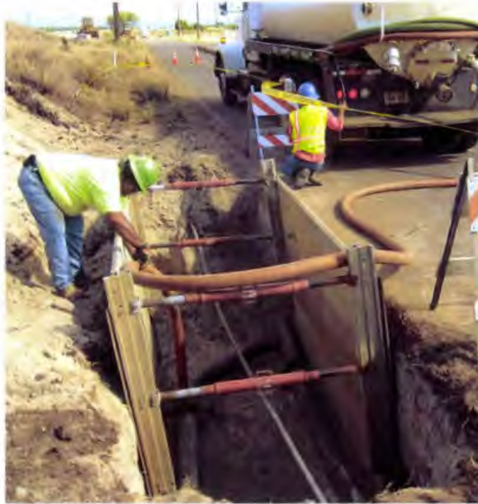
Photo 25. Residual fluid from the existing forcemain pipe is pumped out using a vacuum truck (looking west at valve box #2)
