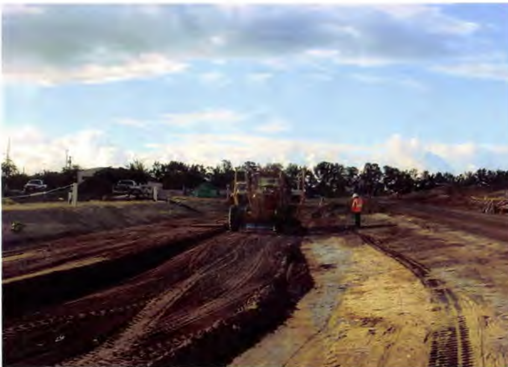
Photo 134. The Cat. 140H motor grader fine grades the infiltration ditch (looking east)
