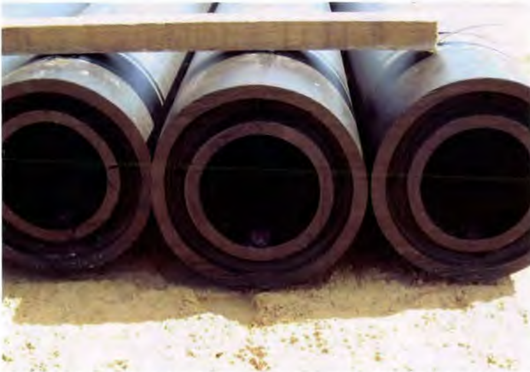
Photo 29. New dual containment, 8-inch diameter SDR 11 inside 12-inch diameter SDR 17 (8" \square x 12" \phi ), HDPE pipe sections
