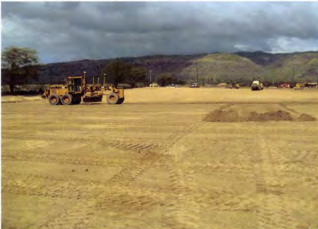
Photo 14. Fine grading the Cell 1 floor subbase with a Cat. 140H motor grader (looking north)
