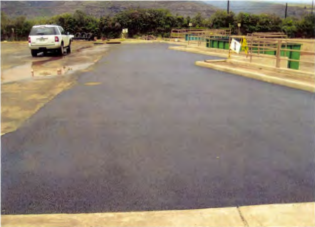
Photo 151. New AC pavement and curb and gutter at MDOF
