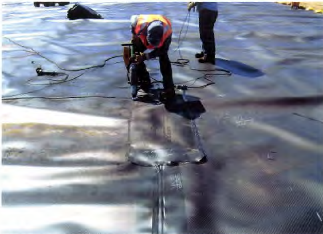
Photo 96. A repair patch is constructed over each destructive seam sample location once the sample is removed
