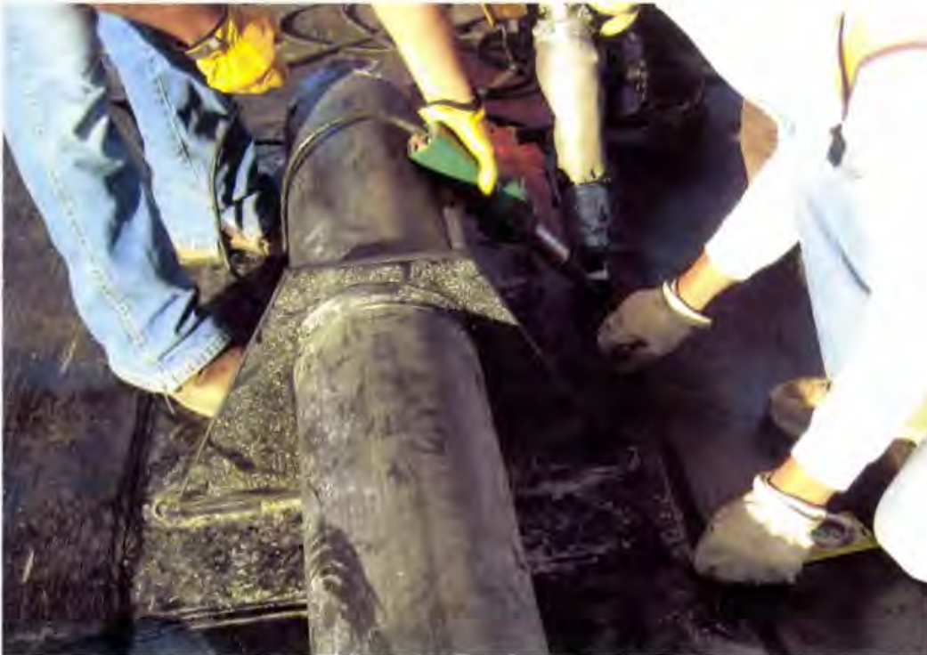
Photo 110. Primary 80 mil HDPE geomembrane panels are extrusion welded (with an embedded copper wire) to the ½-inch thick HDPE flatstock of the pipe penetration assemblies
