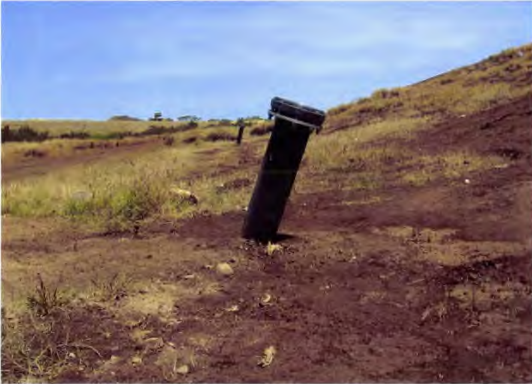
Photo 141. Completed and backfilled modified cleanout riser (typical)
