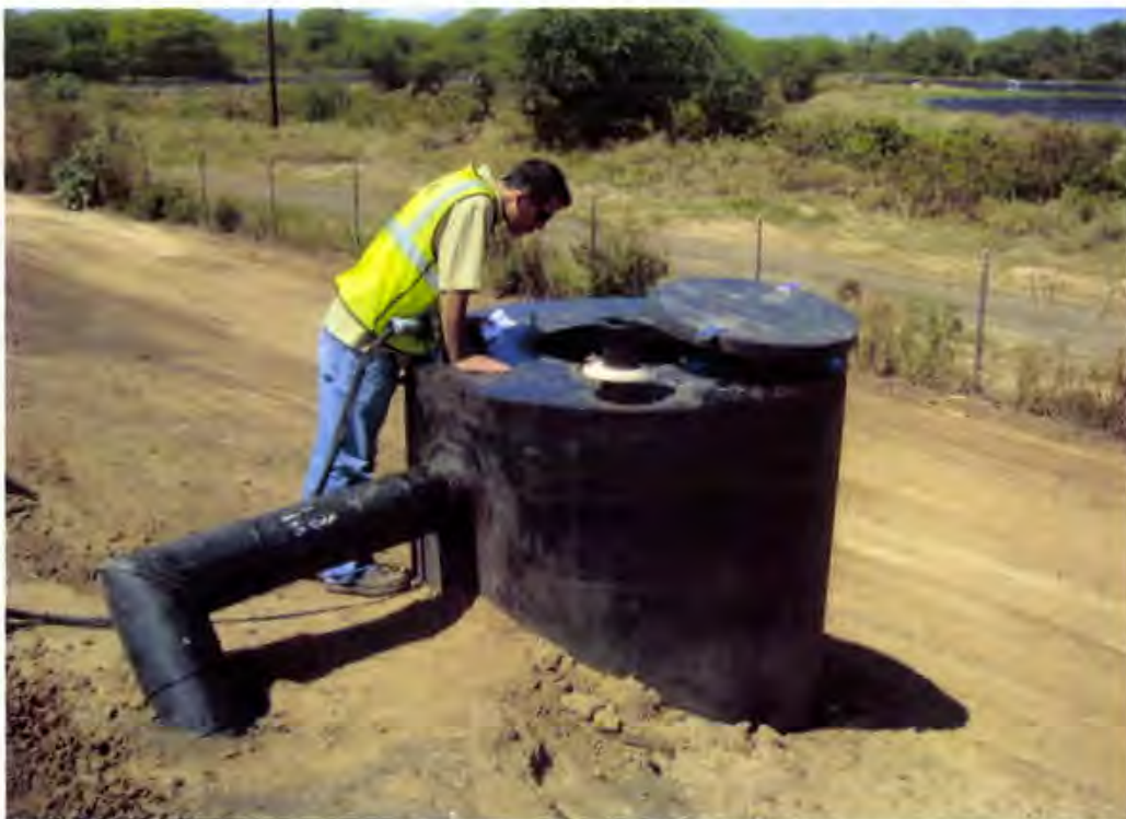
Photo 66. Wet Well #3 system demonstration was performed once the leachate conveyance system was completed
