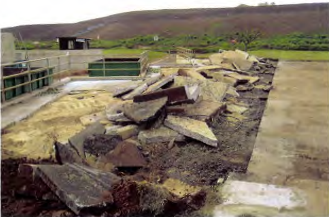
Photo 142. Sawcutting and demolition of existing concrete sidewalk and pavement at the Material Drop Off Facility (MDOF) (looking south)
