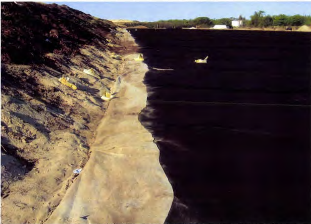
Photo 117. 16 oz/sy nonwoven cushion geotextile heat bonded along existing Phase II tie-in (looking south)
