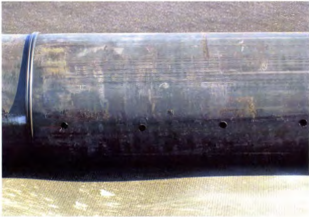
Photo 122. Perforations along the the LCRS pipe
