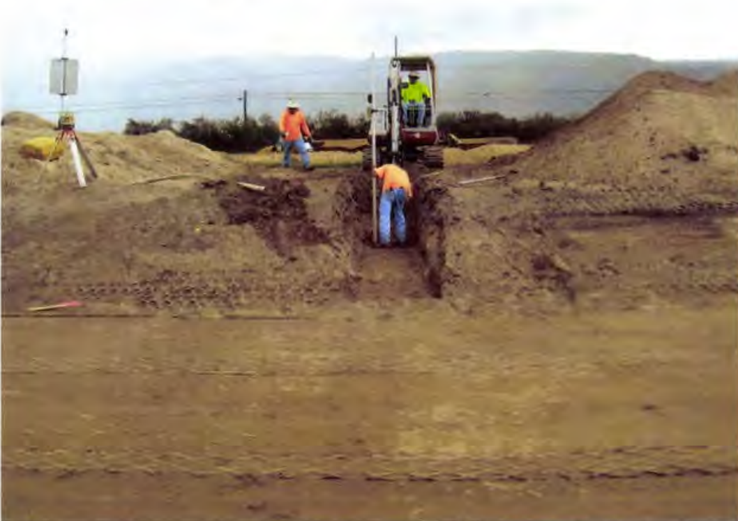
Photo 38. Typical trenches cut at each of Cells 1A-1D sumps, through the sideslopes, for the leachate conveyance pipes
