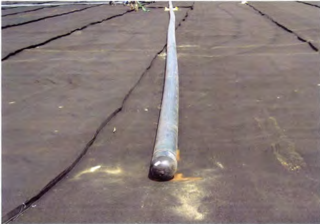
Photo 121. 8"φ perforated HDPE leachate collection and removal system (LCRS) pipes are installed with end caps above the 16 oz/sy nonwoven cushion geotextile
