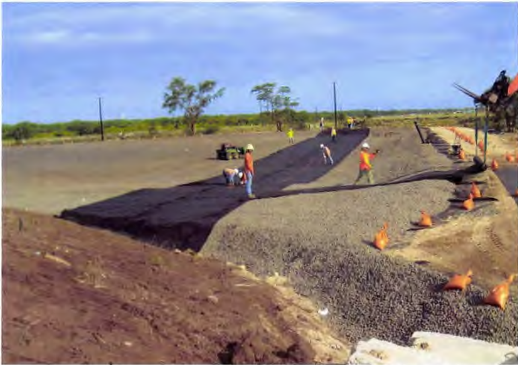
Photo 125. Installing 6 oz/sy nonwoven separator geotextile above the completed granular drainage layer (looking west)
