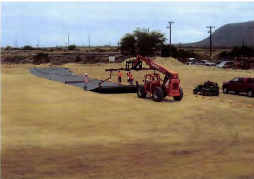
Photo 82. Deploying subbase 60 mil double-sided textured (DST) HDPE geomembrane using a Skytrac hi-lift fork lift over approved subbase (looking northwest)
