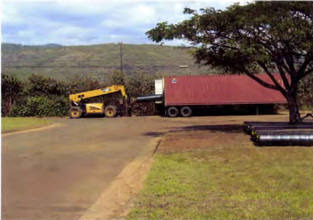
Photo 79. Unloading and stockpiling 16 oz/sy nonwoven geotextile rolls near the administrative office area
