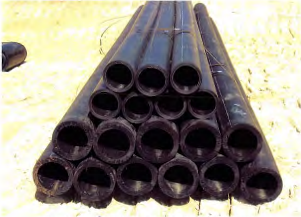
Photo 27. New 6-inch \phi SDR 11 and 8-inch \phi SDR 9 HDPE pipe sections
