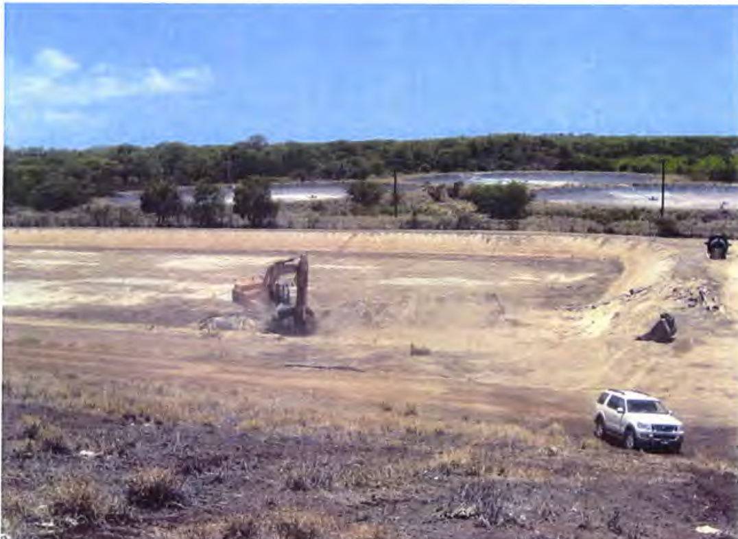
Photo 2. Hitachi 450 LC excavator removing existing leachate pond materials (looking west)
