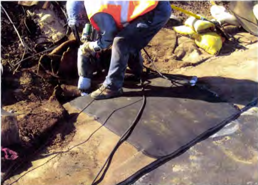
Photo 97. Extrusion welding a repair patch on the existing Phase II geomembrane
