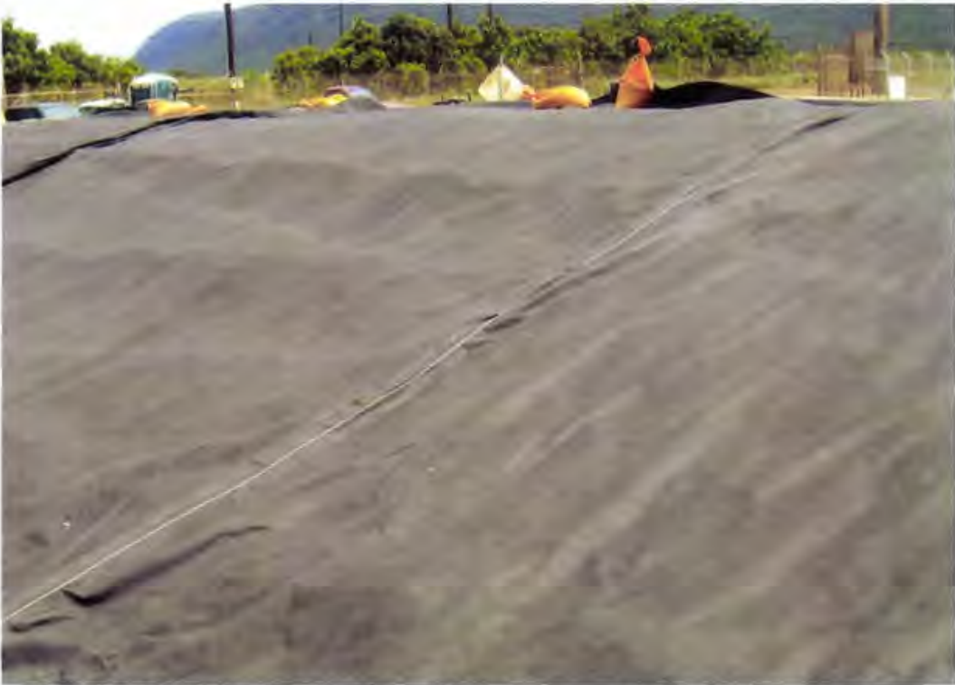
Photo 126. 6 oz/sy nonwoven separator geotextile panels seams sewn using single-prayer seams
