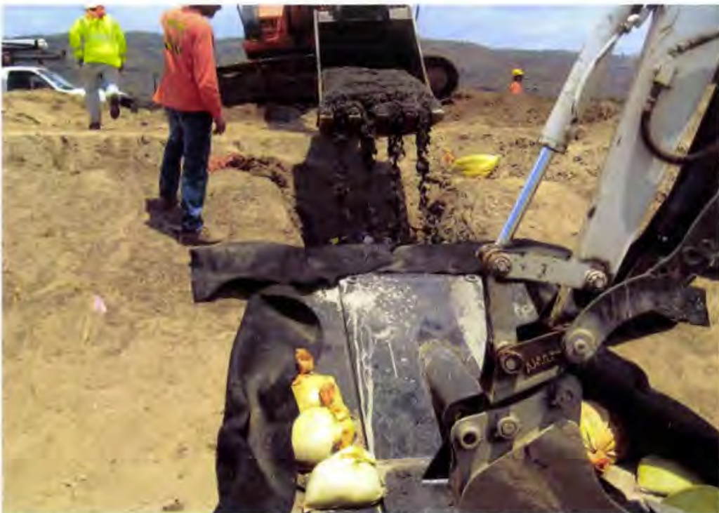
Photo 50. A controlled low-strength material (CLSM) slurry is used to backfill the void space below the pipe penetration assemblies (looking north at Cell 1D penetration)
