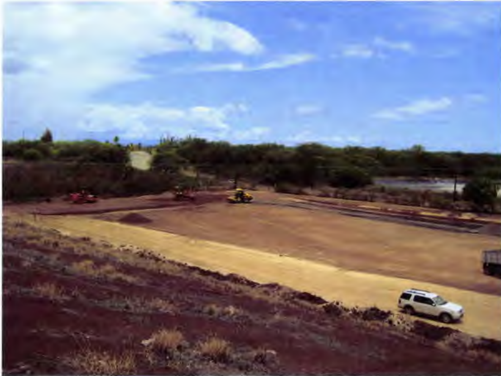
Photo 15. Cells 1A/1B perimeter berm material being spread with a Cat. D5 dozer and compacted with smooth drum rollers (looking southwest)
