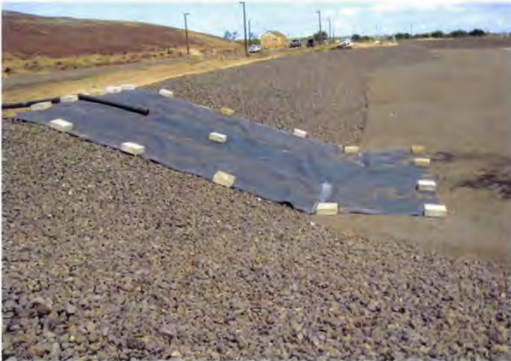
Photo 65. End of discharge pipe in NLEP underlain by HDPE rubsheet weighed down with concrete blocks (looking west)
