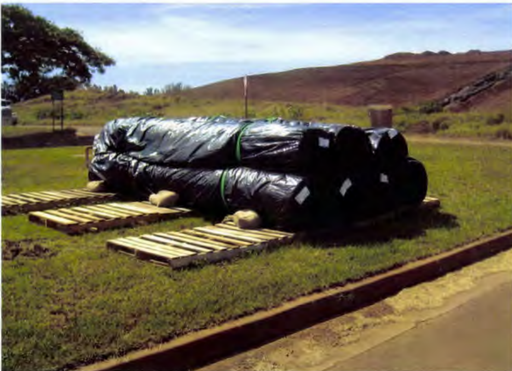
Photo 78. GCL rolls stockpiled on pallets near the administrative office area
