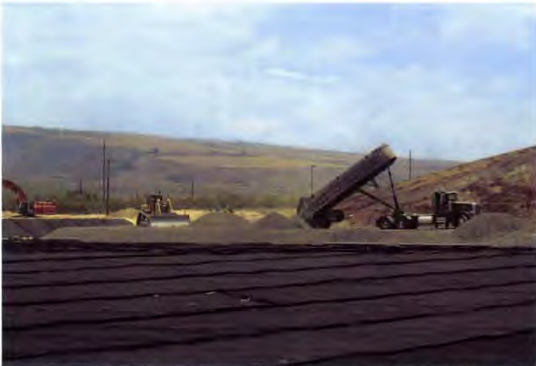
Photo 124. 1.5-inch minus granular drainage layer material (from Kauai Aggregate Quarry) is placed the floor, and is spread and graded using an LGP D6 dozer (looking northeast)
