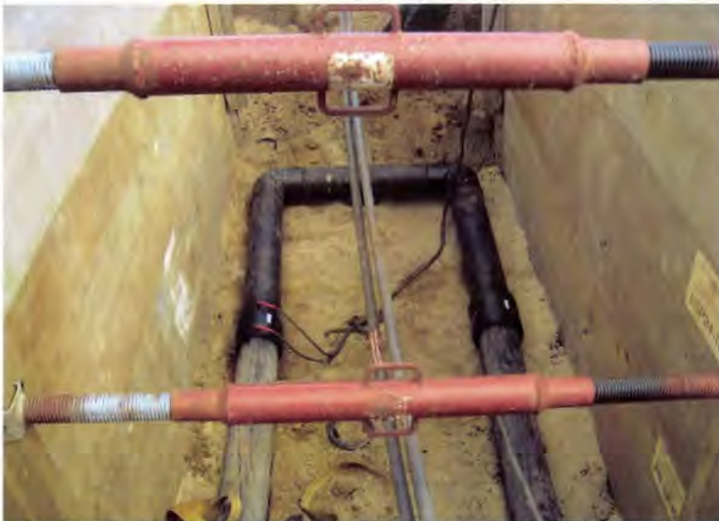
Photo 62. Modified piping near valve box #2 to direct leachate flow to NLEP and new forcemain valve box
