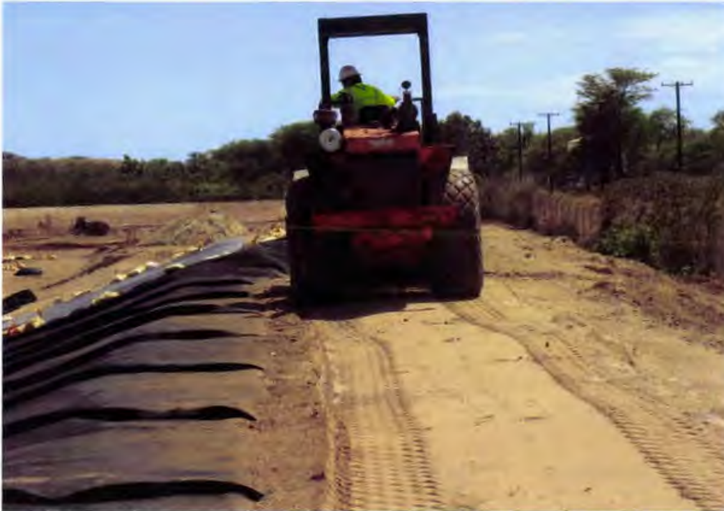
Photo 119. The Cell 1 perimeter anchor trench is backfilled using with a sand fill (onsite soils) and compacted (looking south)
