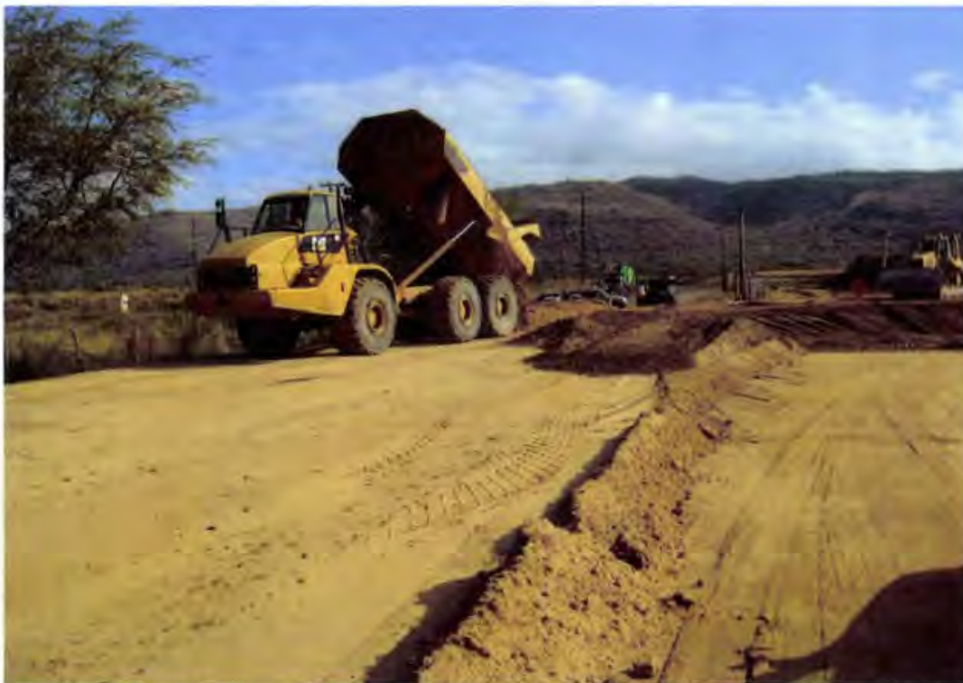
Photo 16. Cat. articulated haul trucks place the fill material along the Cells 1C/1D perimeter berm (looking north)
