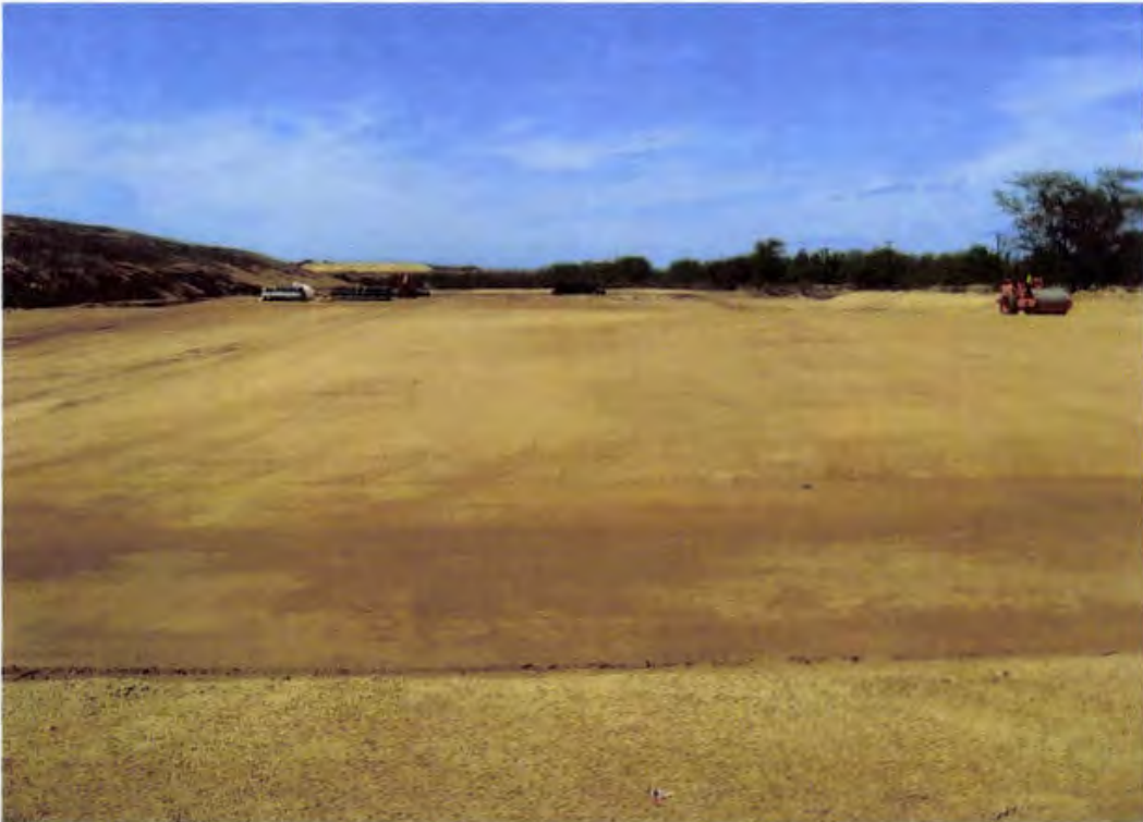
Photo 72. Cells 1C/1D prepared subbase (looking south)
