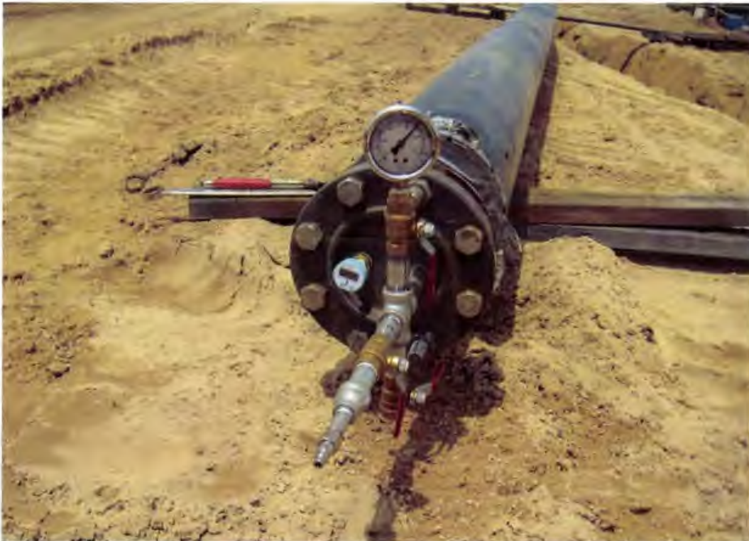
Photo 33. Air pressure tests were performed for all production welded HDPE pipe sections prior to installation
