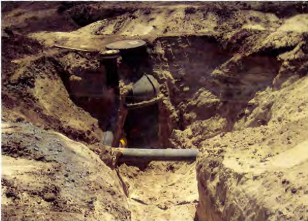
Photo 45. Existing manhole LCM-14 is exposed for the pipe connections (looking east)
