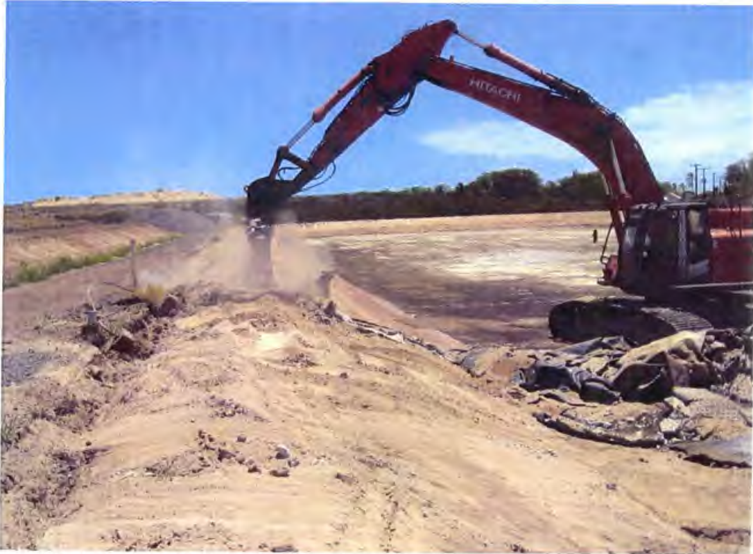
Photo 3. Hitachi 450 LC excavator removing existing leachate pond materials (looking south)
