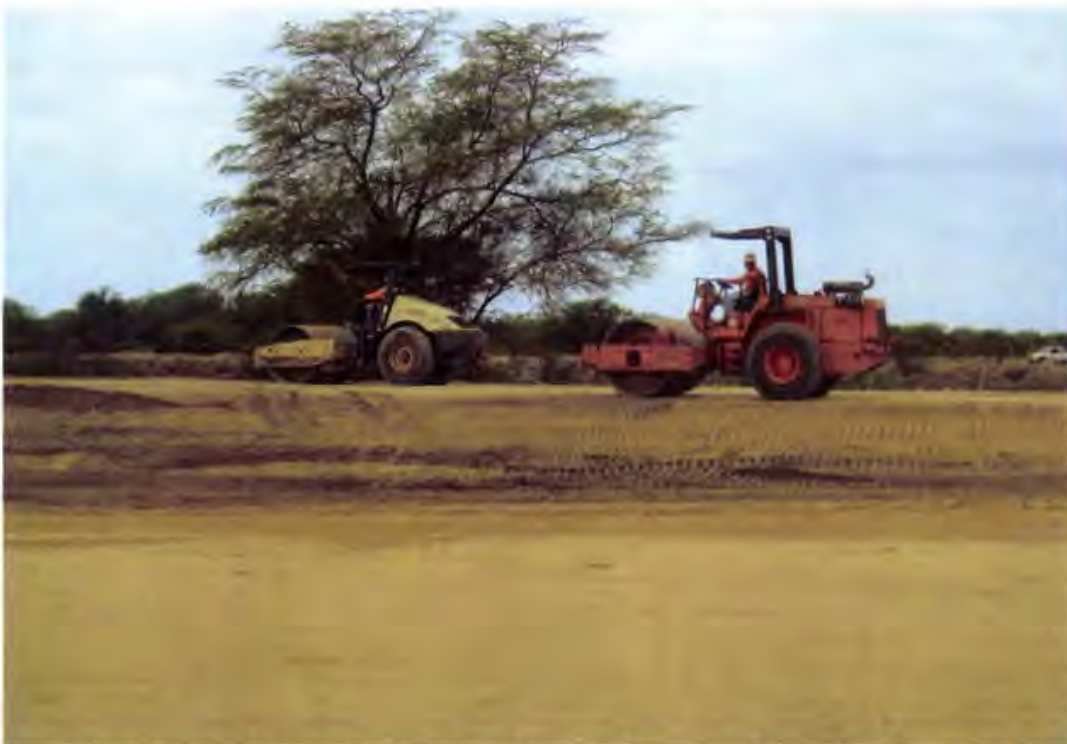
Photo 18. A HAMM 2420 rubber tire smooth drum vibratory compactor assists to compact the perimeter berm (looking west)
