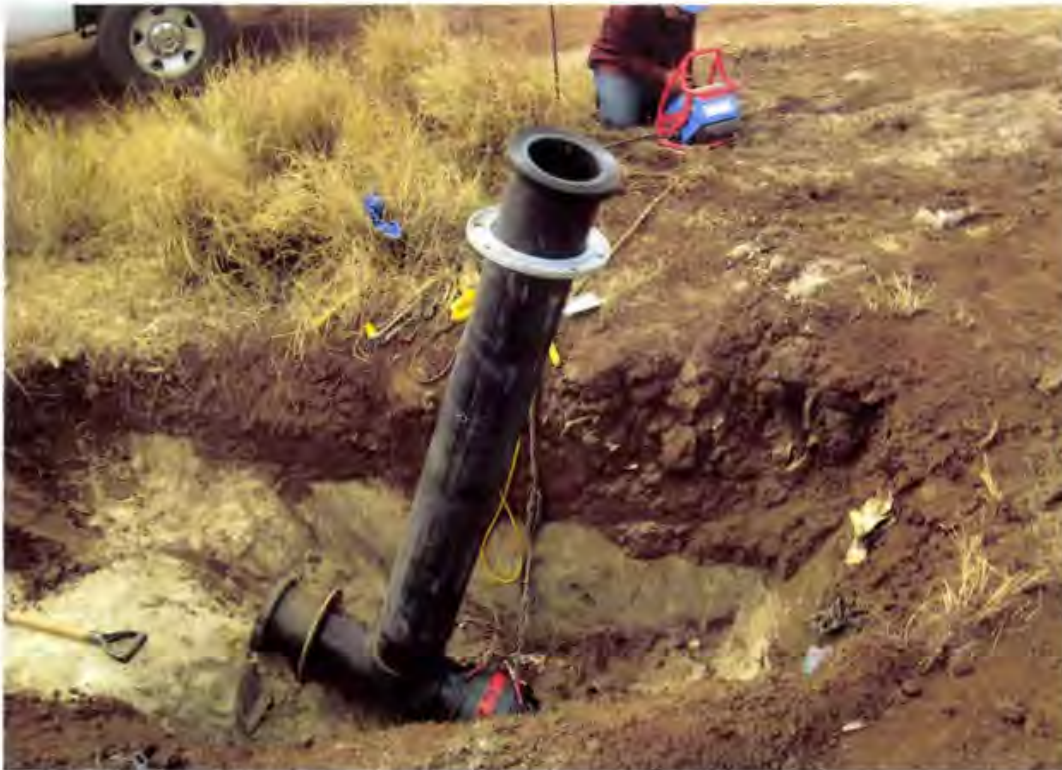
Photo 140. Existing cleanout modified with new HDPE end section connected using an electro-fusion coupler (typical)
