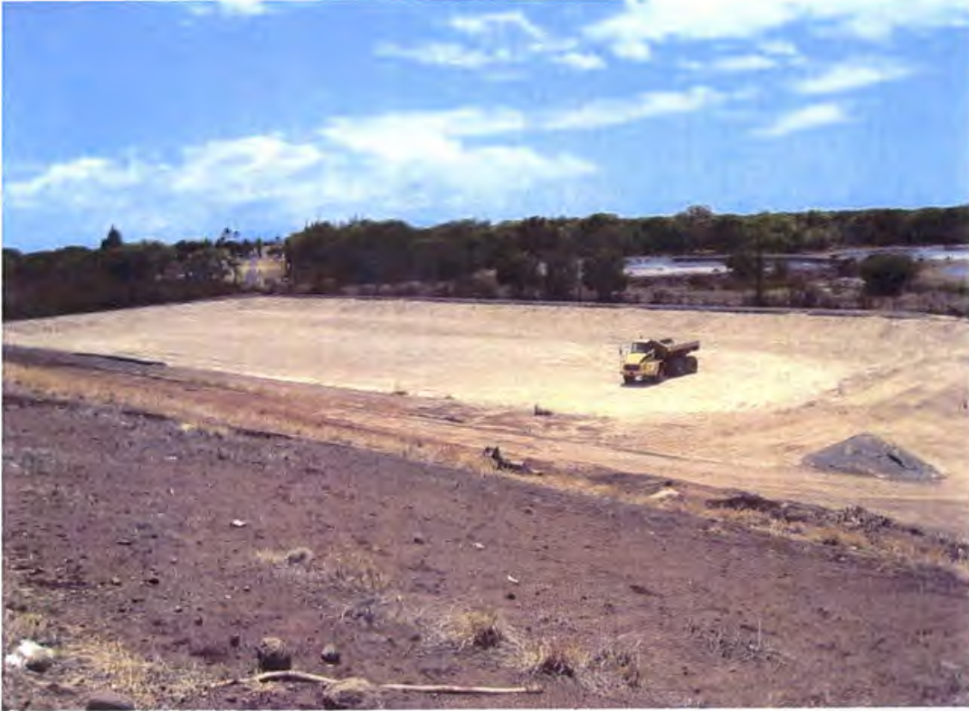
Photo 7. Existing leachate pond subgrade (looking southwest)
