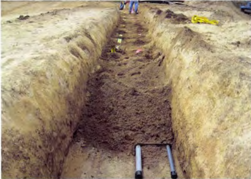
Photo 61. Two electrical conduits are installed above the buried forcemain pipe, and the trench is backfilled with compacted fill (onsite soils) and marked for future identification (looking west)
