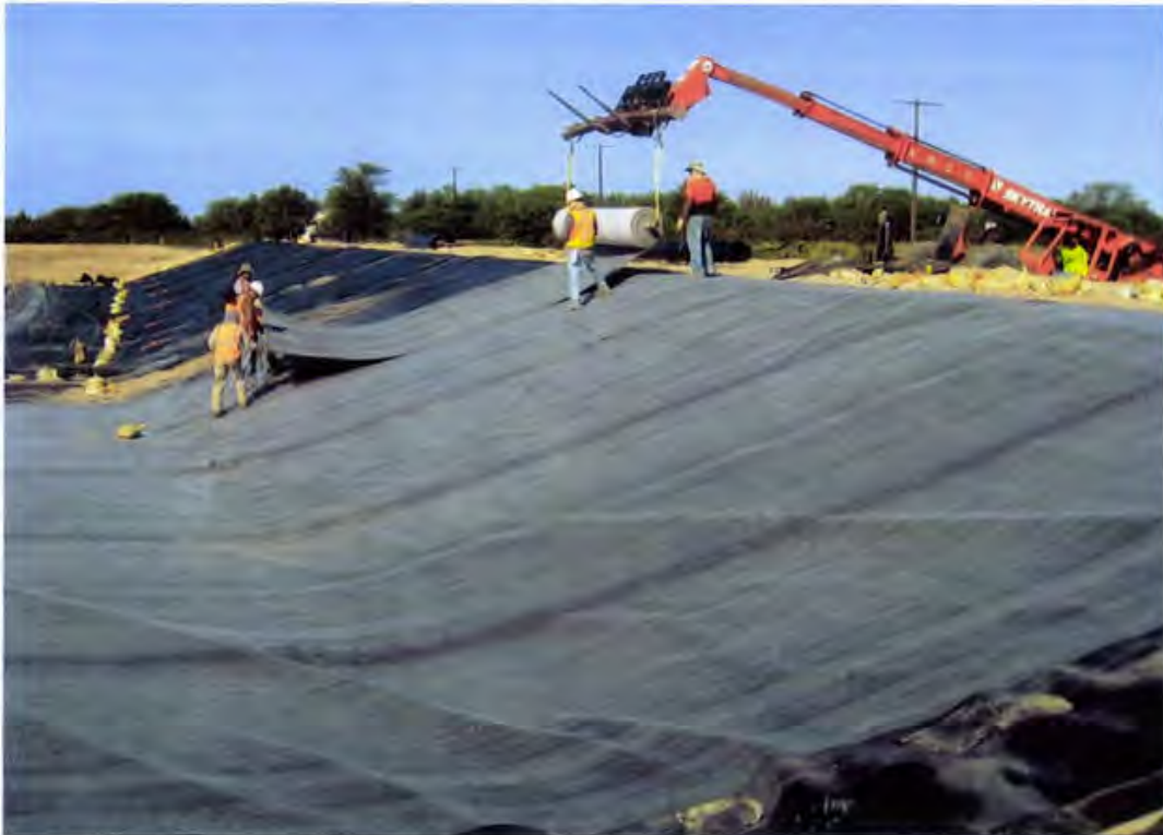
Photo 102. Deploying GCL above the approved subbase 60 mil HDPE geomembrane on the sideslopes (looking south)
