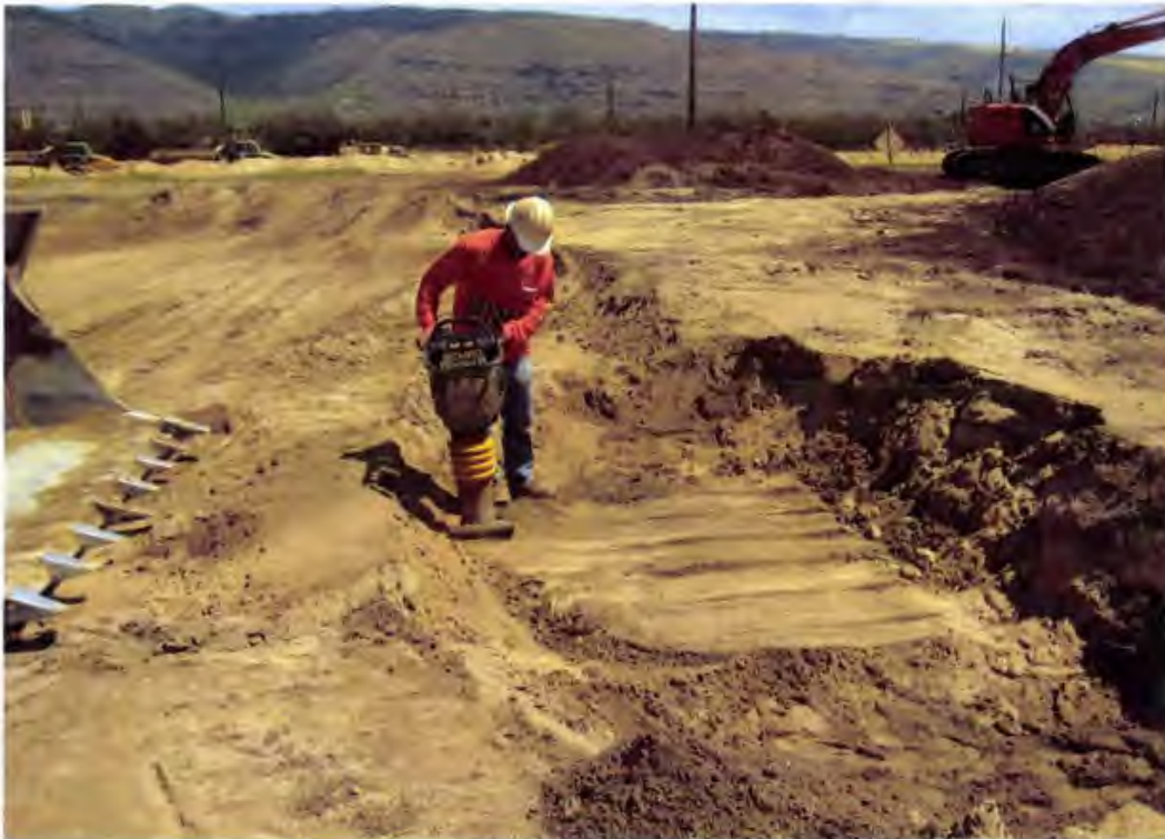
Photo 23. The existing cleanout is backfilled with hand-compacted sand fill (onsite soils) (looking north)
