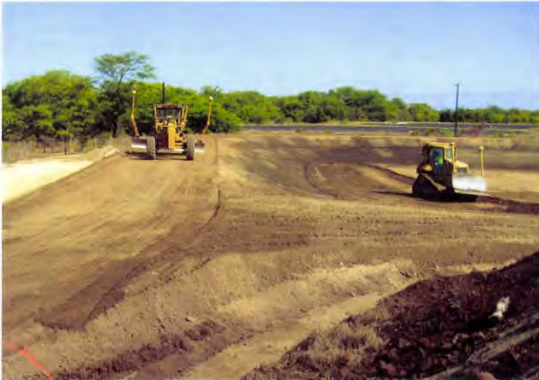
Photo 19. A Cat. 140H motor grader and Cat. D5 dozer (both with GPS control) fine-grade Cells 1A/1B (looking west)
