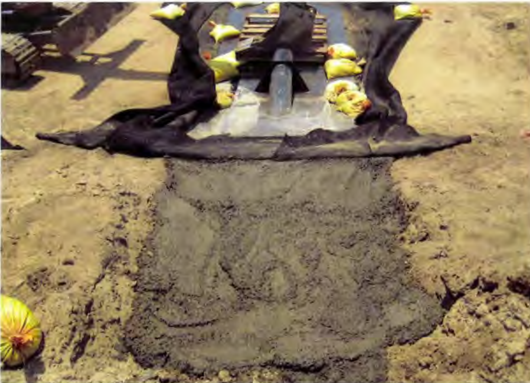
Photo 52. Typical completed CLSM backfill at the pipe penetration
