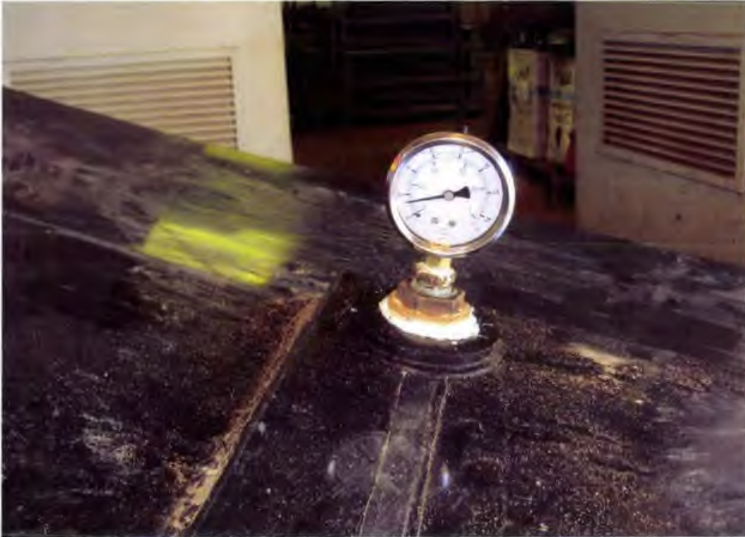
Photo 37. Air pressure of 1.5 psig is applied to the penetration assemblies and sustained for 1 hr minimum
