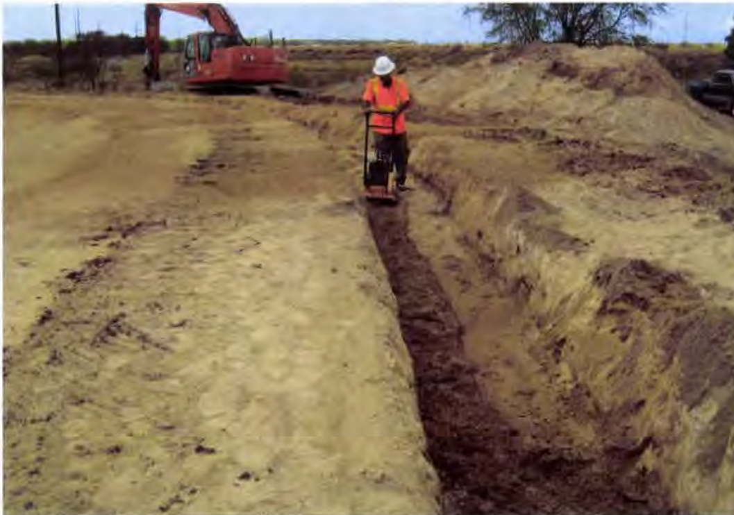
Photo 60. Six inches of compacted fill (onsite soils) is backfilled over the forcemain pipe and compacted using a walk-behind vibratory compactor (looking west)
