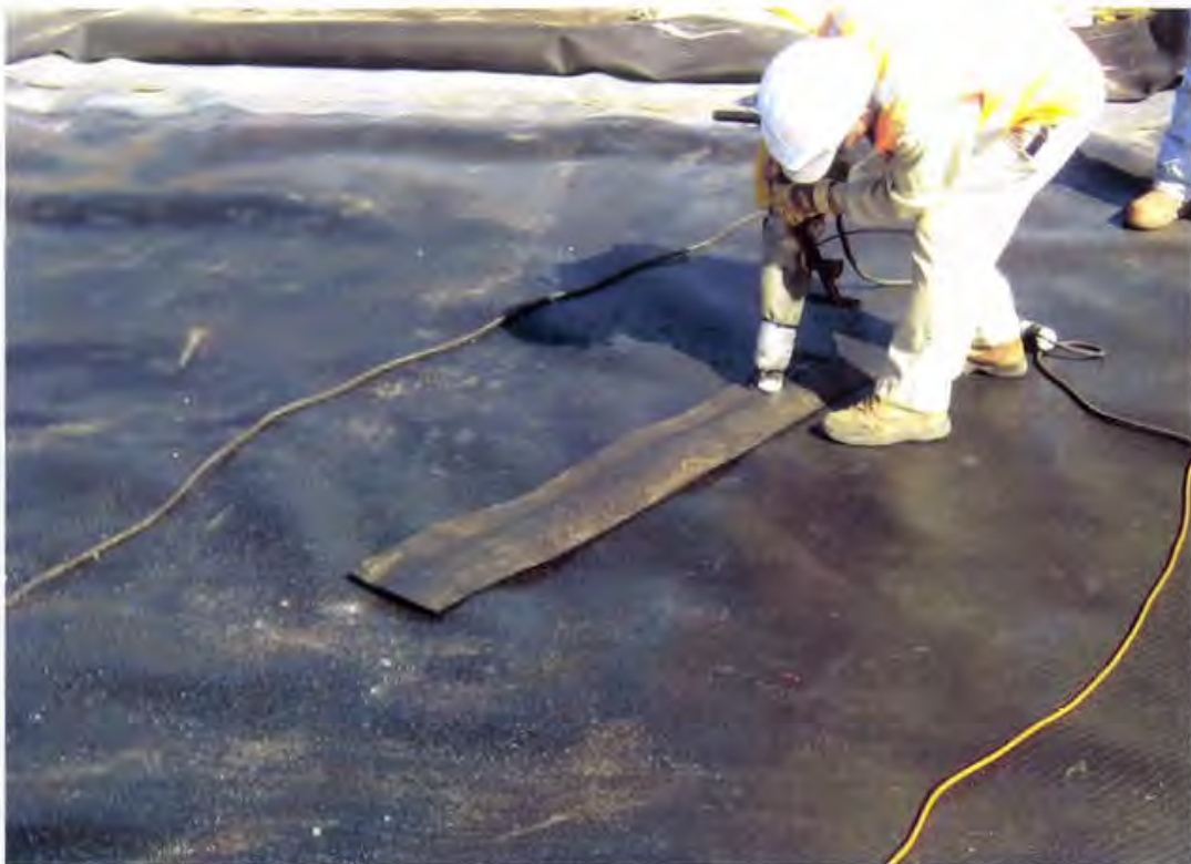
Photo 84. Preparing an extrusion trial weld of textured-to-textured 60 mil HDPE geomembrane
