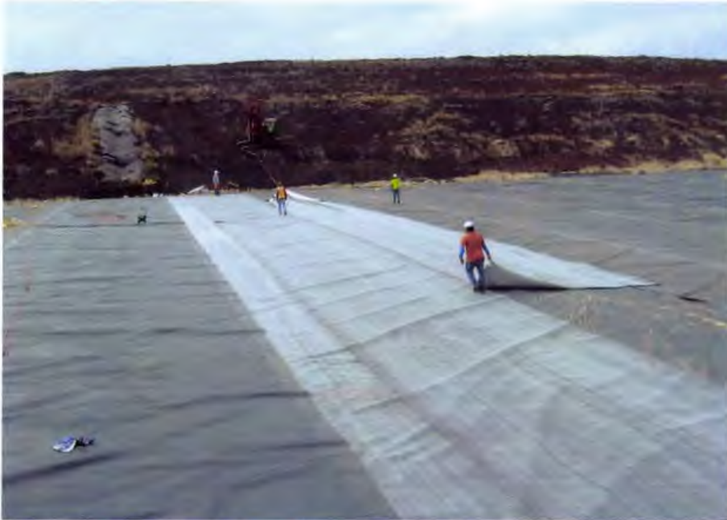
Photo 101. Deploying GCL above the approved subbase 60 mil HDPE geomembrane on the floor (looking east)
