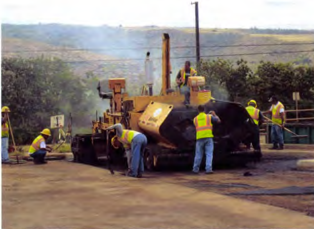
Photo 149. HMA Mix IV AC pavement placed with a hot asphalt spreader and hand spread (looking north)
