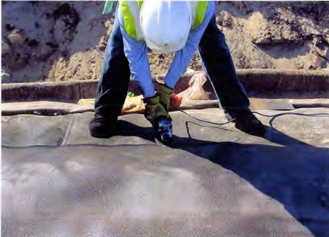
Photo 89. A grinder is used to abrade the surface of the geomembrane prior to extrusion welding.
