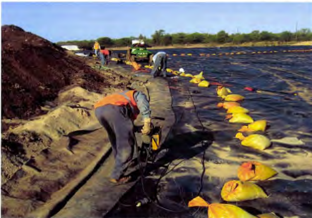
Photo 90. Extrusion welding the subbase 60 mil HDPE geomembrane to the existing Phase II geomembrane (looking southwest)
