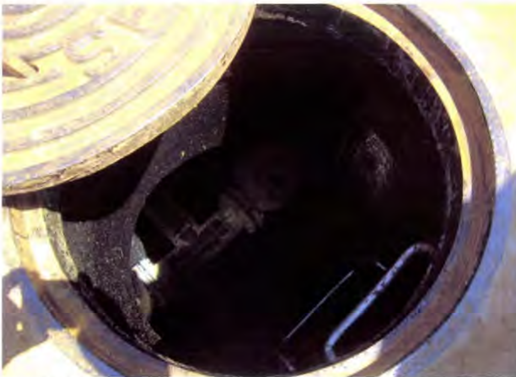
Photo 64. Installed concrete valve box completed with interior coating for waterproofing
