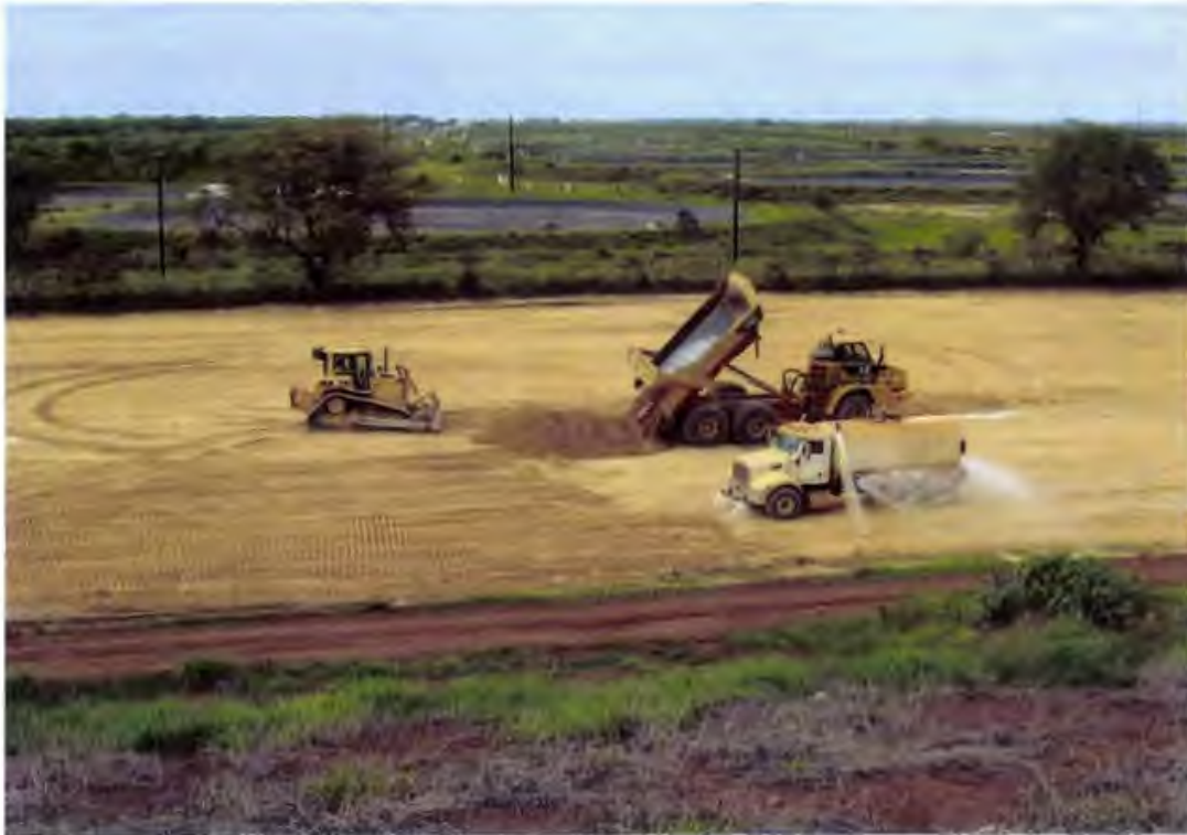
Photo 9. The compacted fill (onsite soils) materials are hauled to Cell 1 using Cat. articulated haul trucks, spread with a Cat. D6 LGP dozer, and then moisture conditioned with the water truck (looking west)
