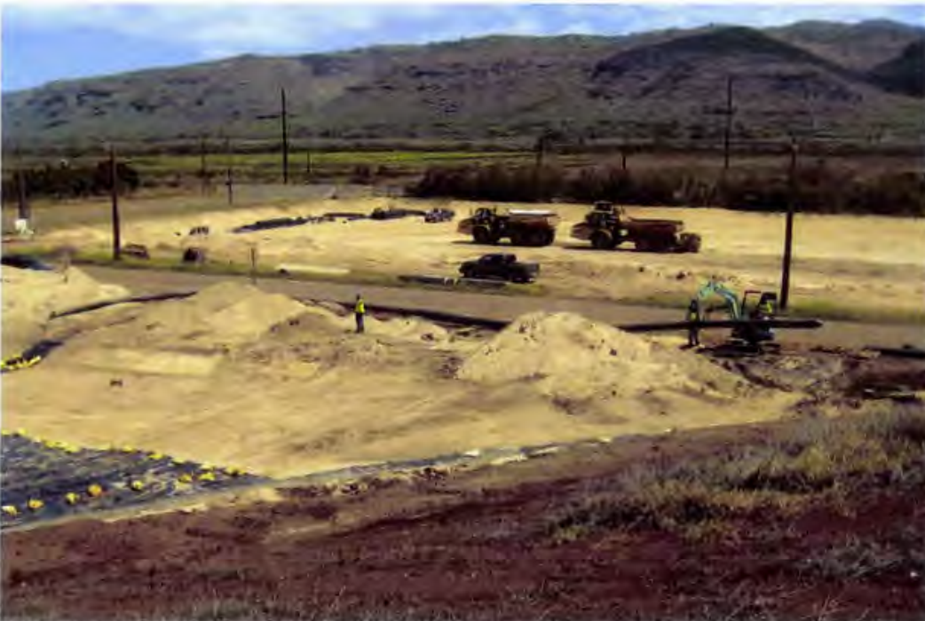
Photo 44. Installing the dual containment (8"φ x 12"φ) HDPE pipe from Cell 1D sump penetration to existing manhole LCM-14 (looking northwest)
