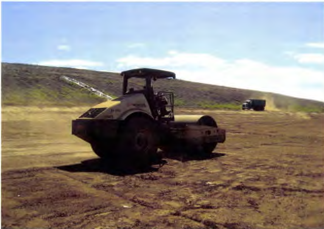
Photo 4. Proof-rolling the existing Cell 1 subbase using a 13-ton Ingersoll-Rand SD122DX rubber tire smooth drum vibratory compactor (looking southeast)
