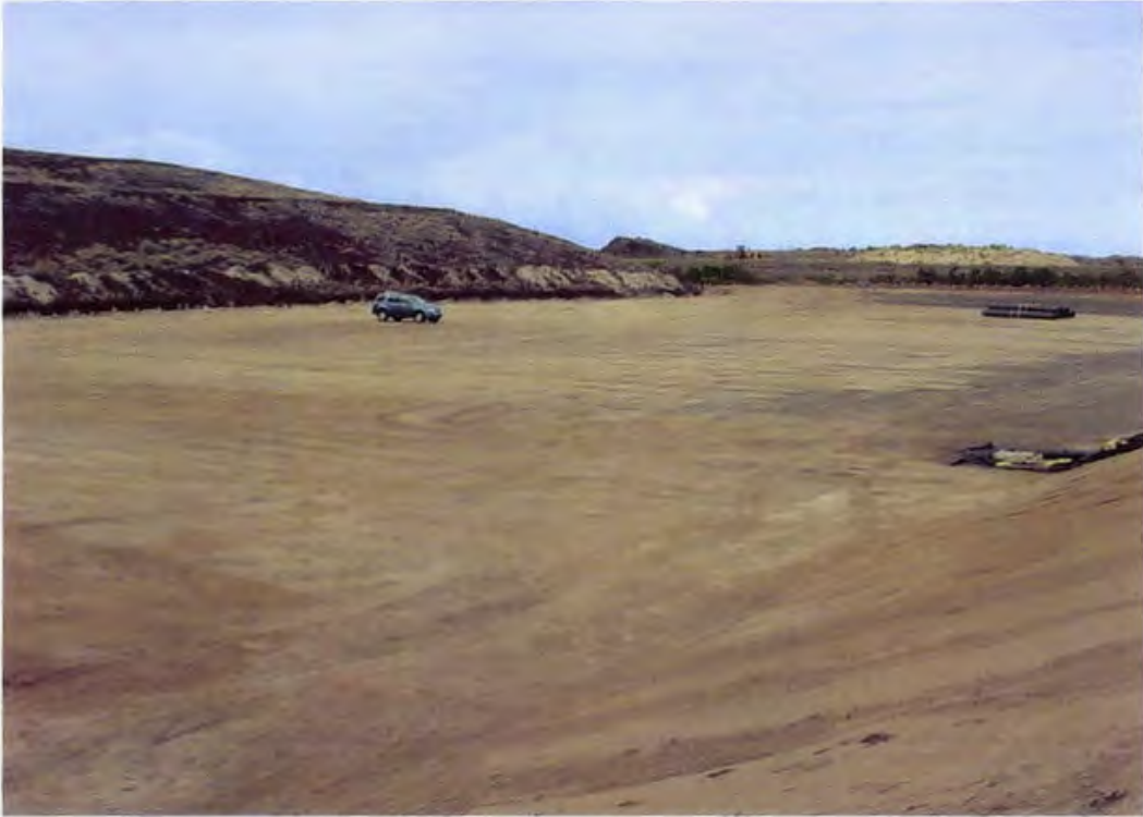
Photo 71. Cells 1A/1B prepared subgrade (looking south)
