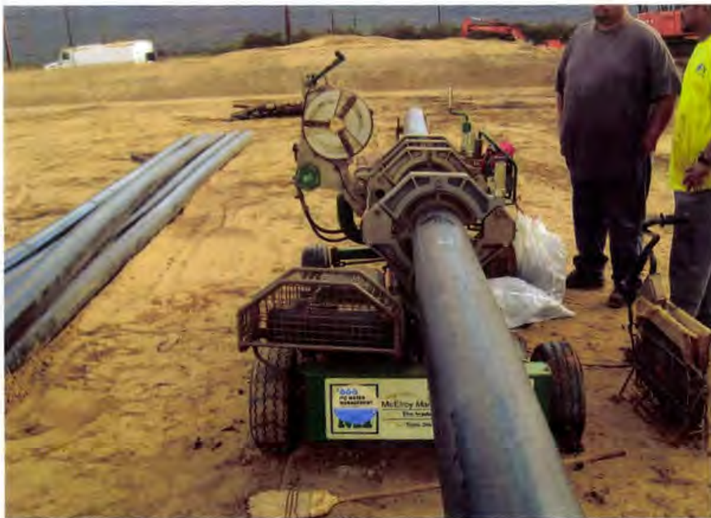
Photo 30. ITC Water Management production welds the various HDPE pipe sections
