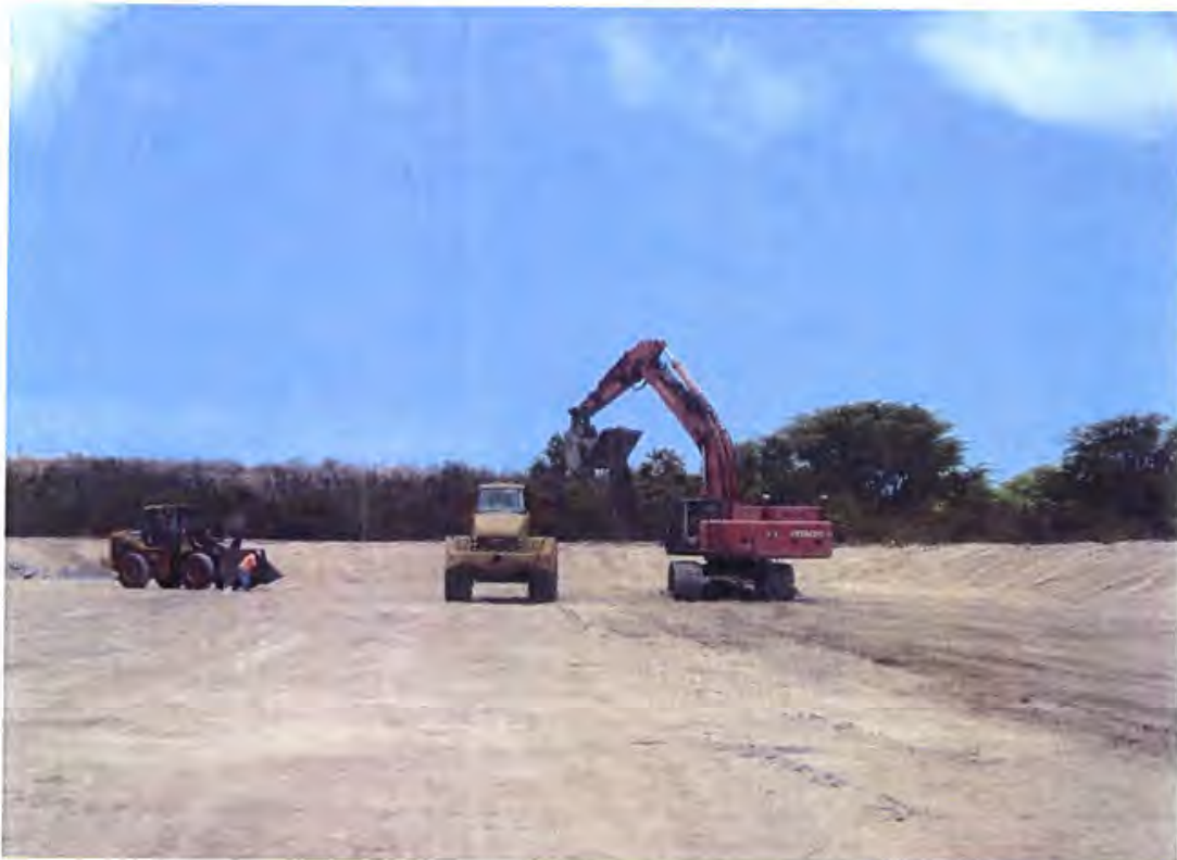
Photo 6. A Caterpillar 740 haul truck transports the removed pond materials to the Phase II landfill for disposal (looking south)
