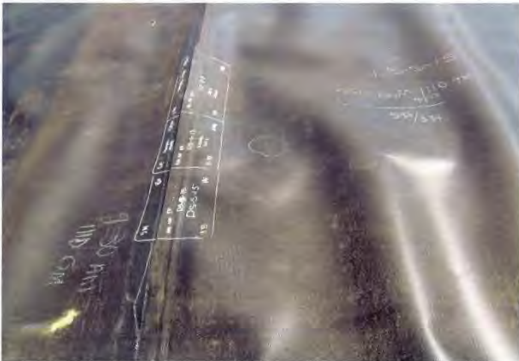
Photo 94. Destructive seam sample location marked within production seam. Each seam sample consists of three parts: one part for the Installer, one part for CQA conformance testing, and one part for the Owner's archive
