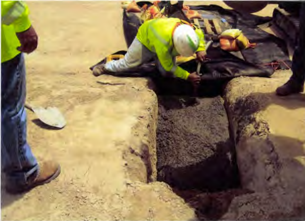
Photo 51. The CLSM slurry is vibrated to remove voids and produce a more homogenous backfill
