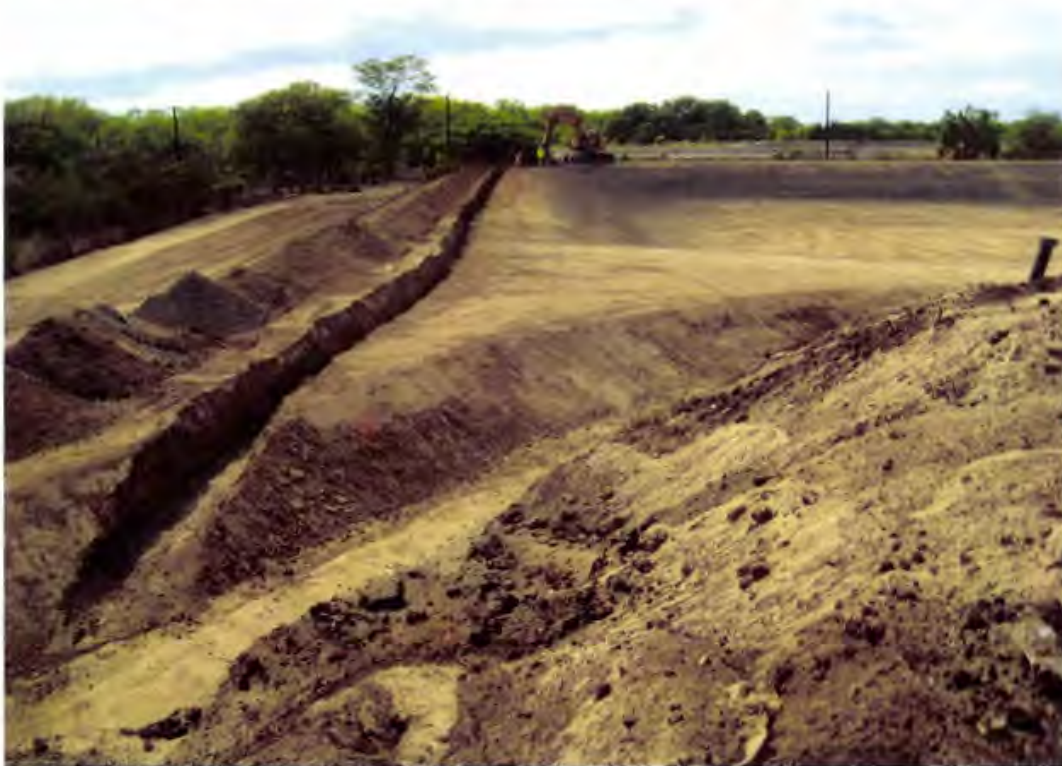
Photo 74. Field adjusted subbase grades at far southeast corner of Cell 1A (looking west)
