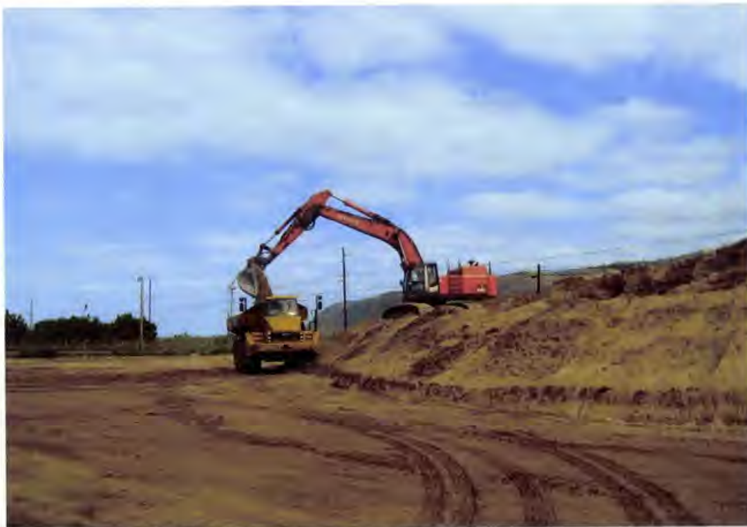
Photo 6. Compacted Fill (onsite soils) material is hauled from the existing sand stockpile and the new infiltration basin (NIB) to construct the Cell 1 subbase grades (looking northwest)
