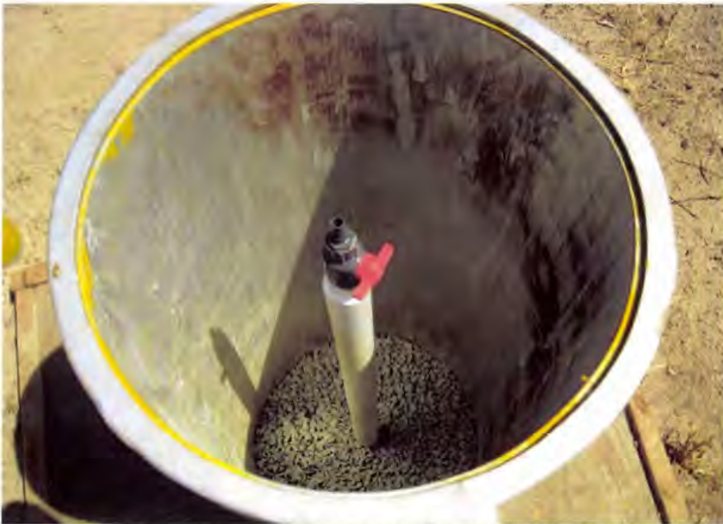
Photo 136. Two new gas monitoring probes were installed (GP-II-6 and GP-II-7)
