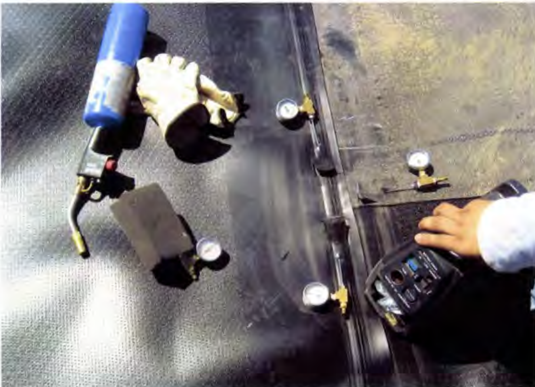
Photo 112. Non-destructive air pressure testing the fusion welded production seams of the primary geomembrane
