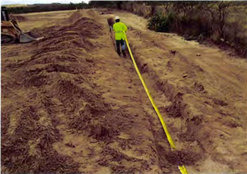
Photo 49. The dual containment pipe trenches are backfilled with compacted fill (onsite soils) and marked with tape for future identification (looking south)
