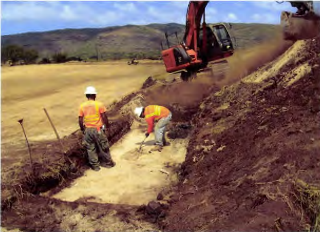
Photo 67. Exposing the existing Phase II containment system tie-in (looking north)
