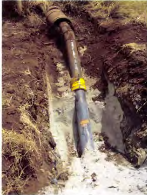
Photo 139. Exposed existing Phase II cleanout riser (typical)
