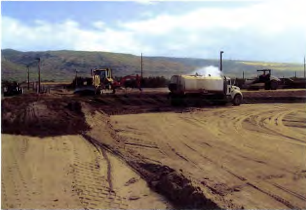
Photo 17. A Cat D5 dozer with GPS control spreads the fill material to uniform 8- to 10-inch thick loose lifts across the berm width, a water truck moisture conditions the lifts, and the Ingersoll-Rand SD122DX vibratory compactor provides compactive effort (looking north)
