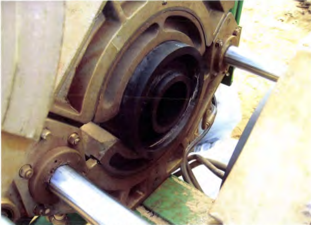
Photo 31. Fusion (butt) welding dual containment HDPE pipe sections
