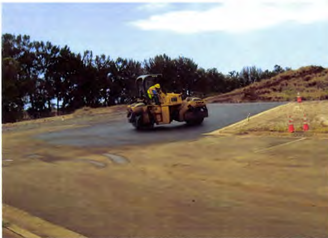
Photo 150. A smooth drum roller rolls the surface of the placed AC pavement (looking southeast)
