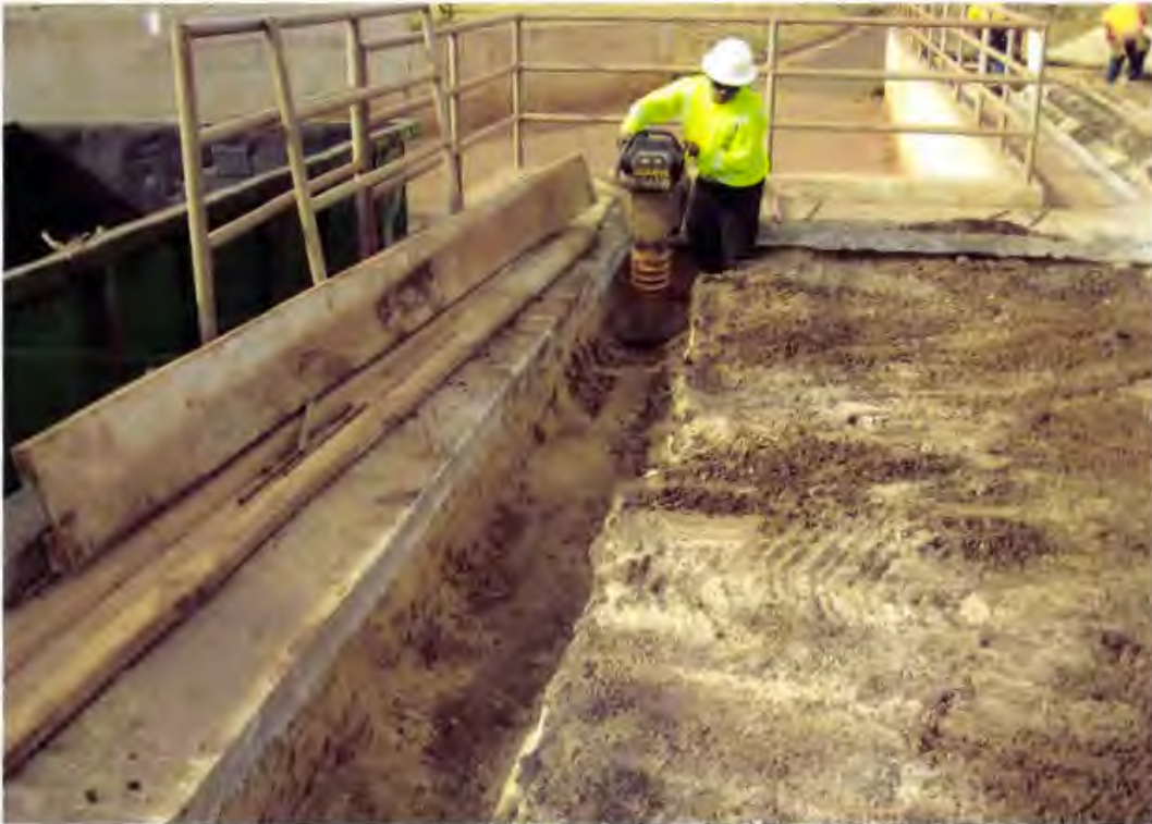
Photo 143. Existing perimeter curb and gutter transition is over-excavated 18 inches, and existing subgrade is hand compacted (looking south)
