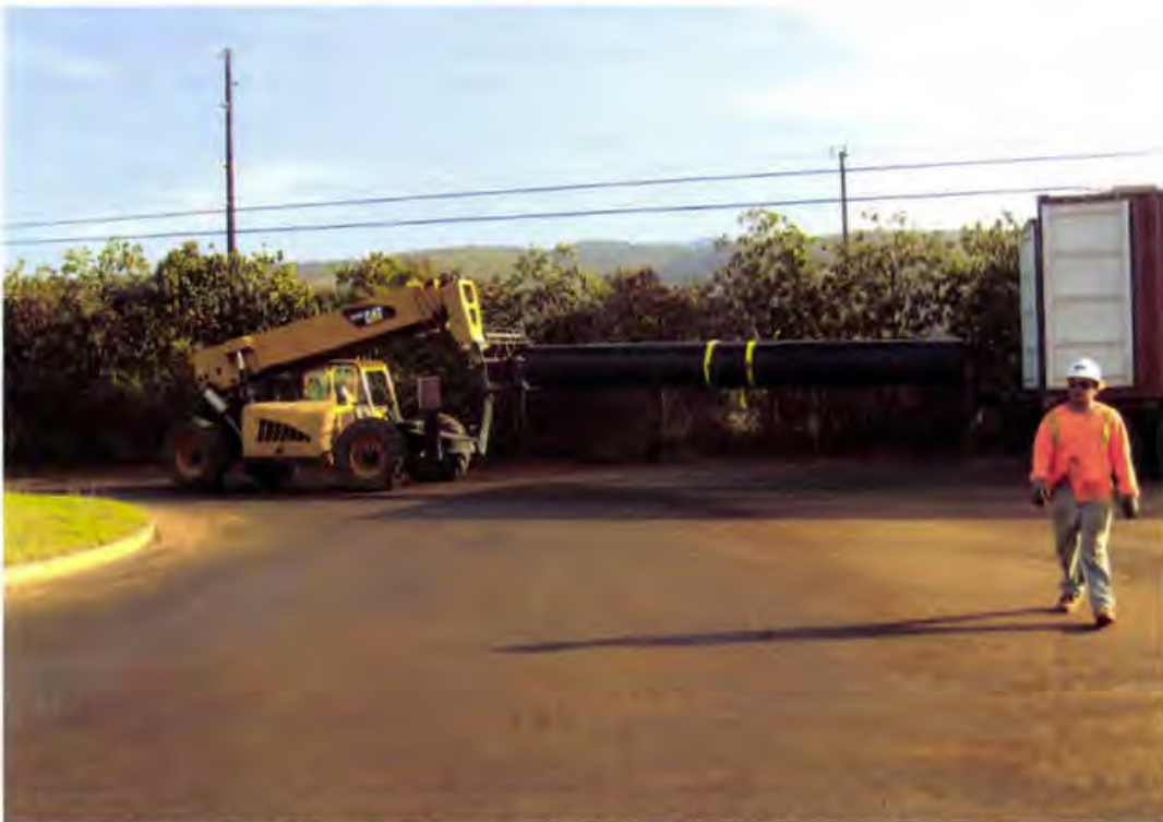
Photo 80. Unloading Agru 60 mil double-sided textured HDPE Microspike geomembrane rolls
