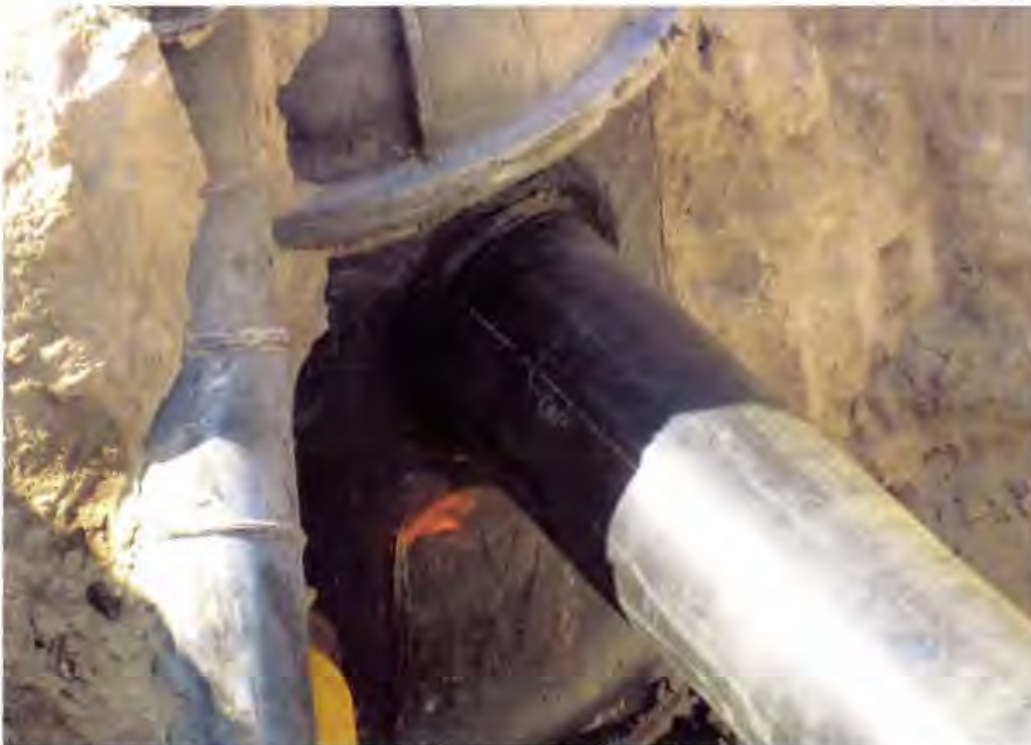
Photo 46. Cell ID dual containment (8"φ x 12"φ) connection to LCM-14. Outer pipe is extrusion welded to the manhole
