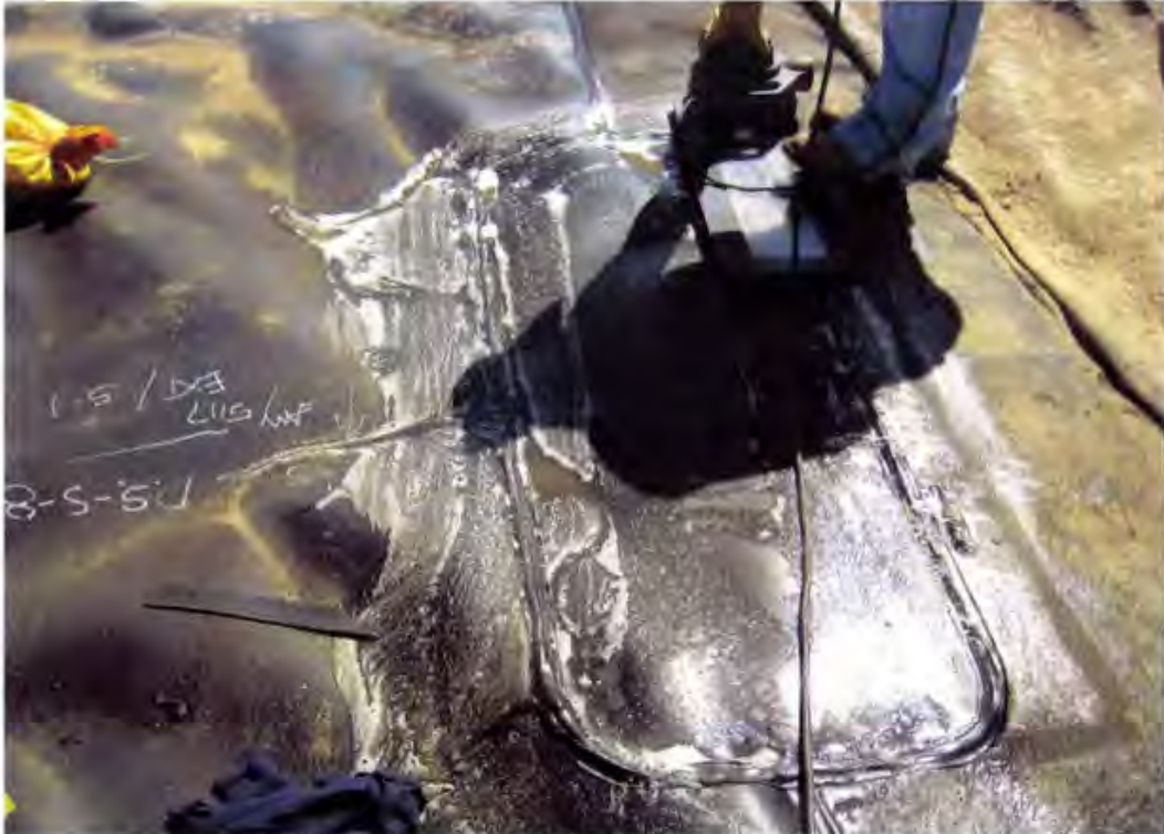
Photo 98. Non-destructive vacuum box testing the extrusion seam of a repair patch
