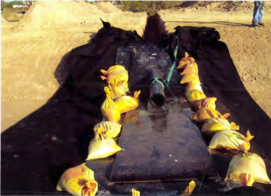
Photo 39. Typical installed pipe penetration assembly underlain by nonwoven geotextile and aligned with pipe trenches
