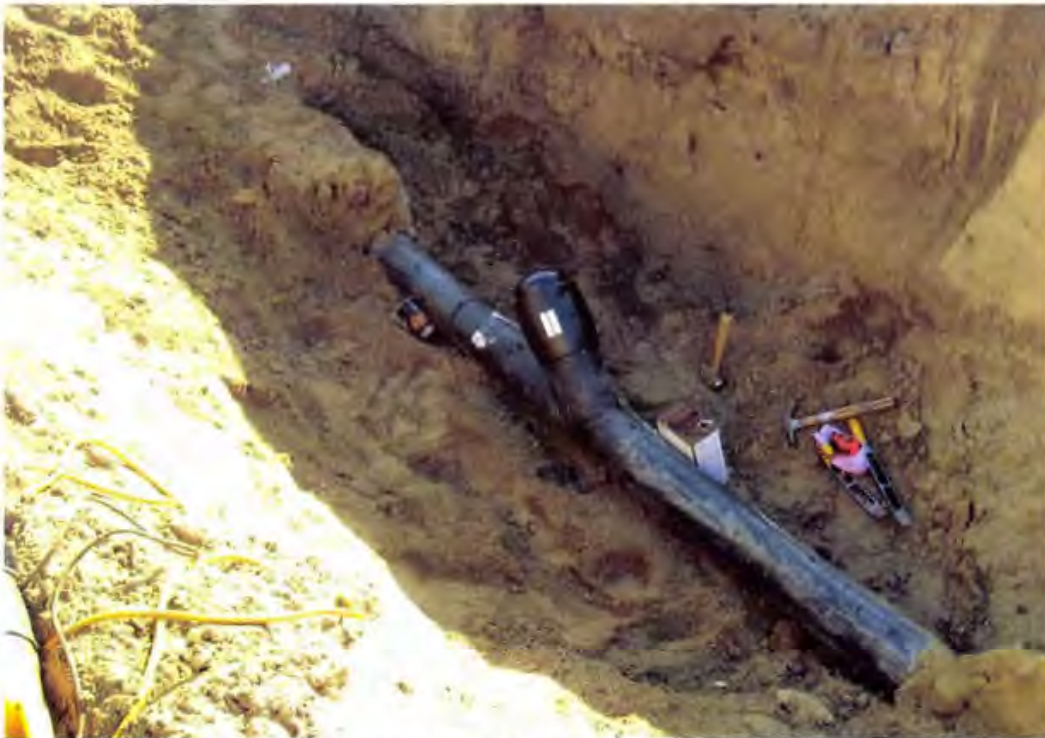
Photo 22. End section of existing cleanout is cut and capped using an HDPE cap with electro-fusion coupler (in accordance with RFI #7)
