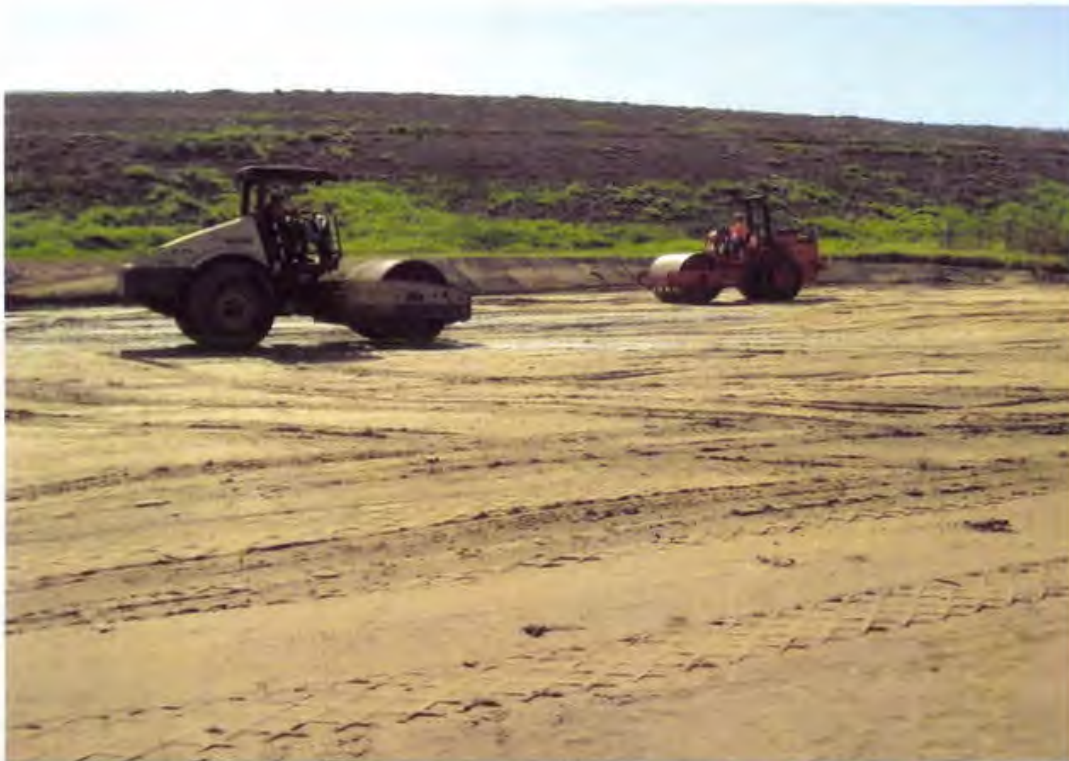
Photo 11. An Ingersoll-Rand SD122DX rubber tire smooth drum vibratory compactor and Bomag smooth drum vibratory roller applies compaction effort to the lifts (looking northwest)
