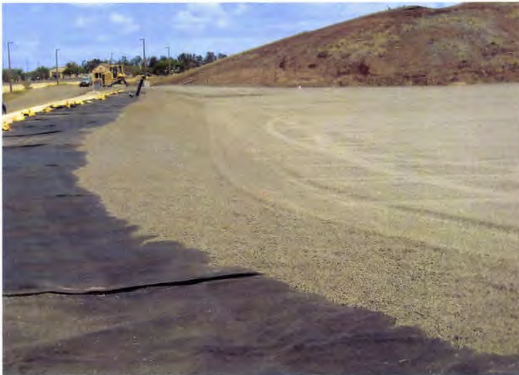
Photo 130. Completed operations layer material (looking east along Cell 1D north berm)
