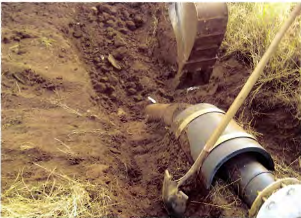
Photo 138. Carefully exposing 14 existing cleanout risers along southern perimeter of Phase II landfill for modifications (typical)
