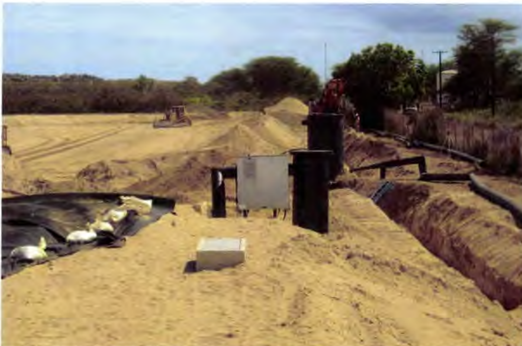
Photo 40. During Cell 1A/1B construction, the temporary wet well (foreground well) was removed and the new Wet Well #3 (background well) was installed (looking south)
