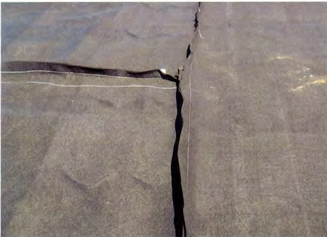
Photo 116. 16 oz/sy nonwoven cushion geotextile panels seams sewn using single-prayer seams
