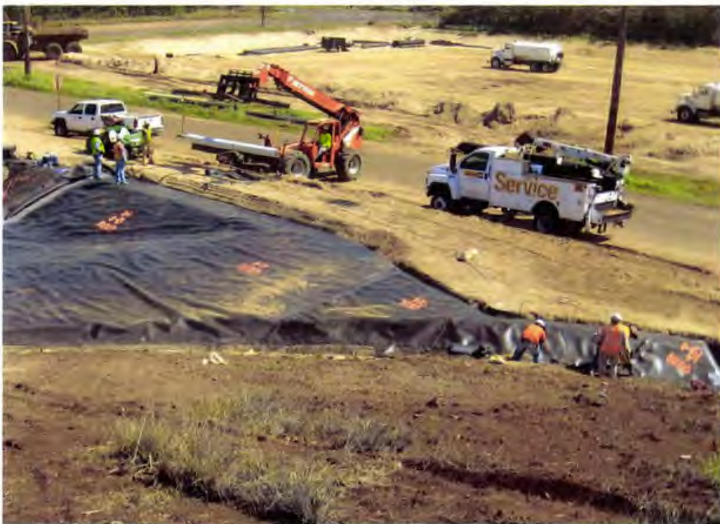
Photo 100. Completed subbase HDPE geomembrane at Cell 1D northeast corner (looking northwest)
