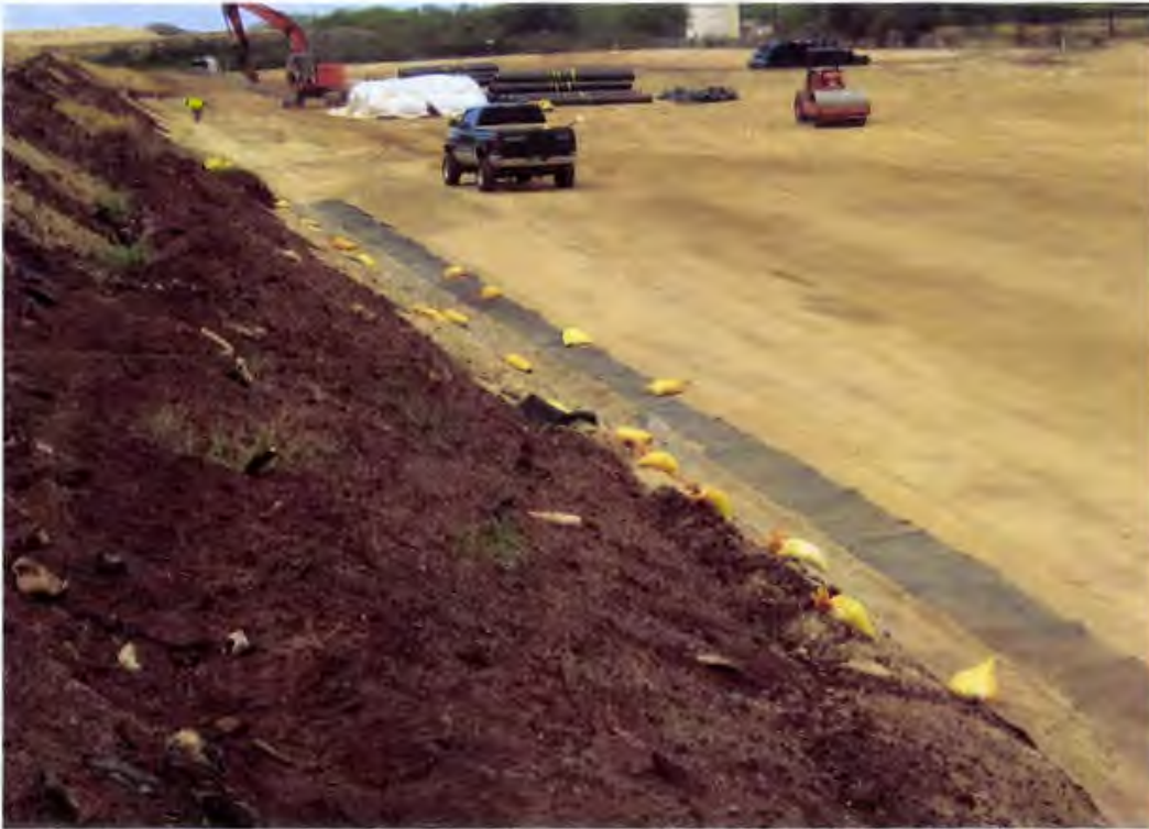
Photo 69. West edge of existing Phase II containment system exposed for tie-in (looking south)
