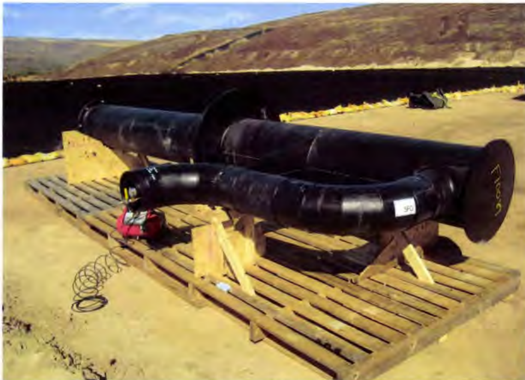
Photo 34. Air pressure tests were also performed for the prefabricated, factory-welded HDPE temporary wet well and Wet Well #3 assemblies prior to installation
