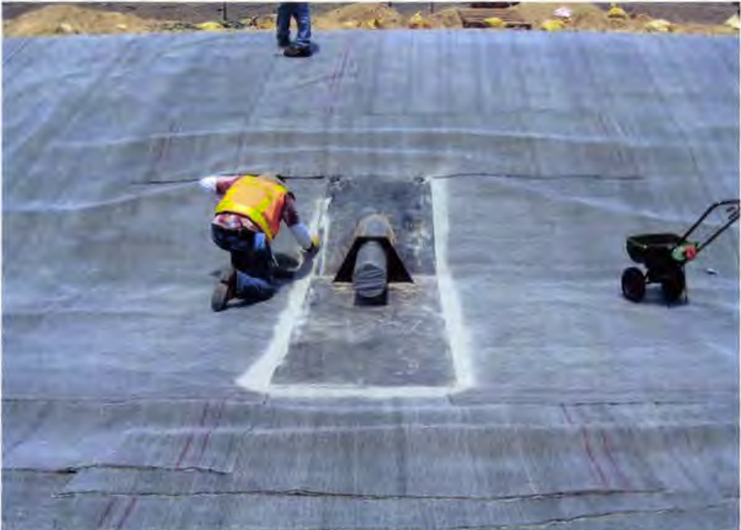
Photo 105. Granular bentonite is placed along the edge of GCL around the pipe penetration assemblies (looking north at Cell 1D penetration)
