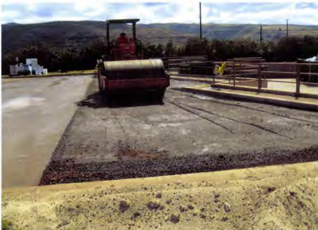
Photo 148. Compacting new 18-inch aggregate base course using a HAMM 2420 smooth drum vibratory compactor for new pavement around MDOF and entrances/exits to administration area (looking south at MDOF)
