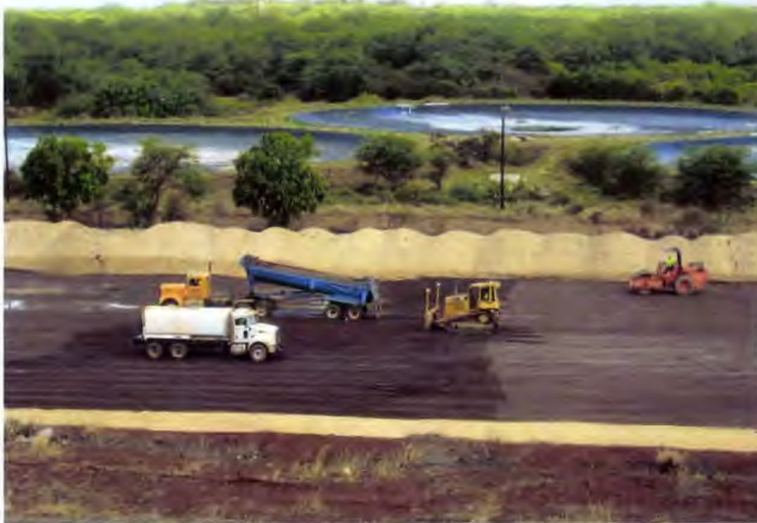
Photo 10. The compacted fill (offsite soils) materials are imported to Cells 1A/1B from the Kauai Aggregates quarry using end-dump trucks, spread with a Cat. D5 dozer, and moisture conditioned with the water truck (looking west)
