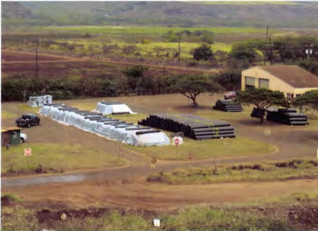
Photo 81. Complete geosynthetic inventory stockpiled adjacent to the administrative office area
