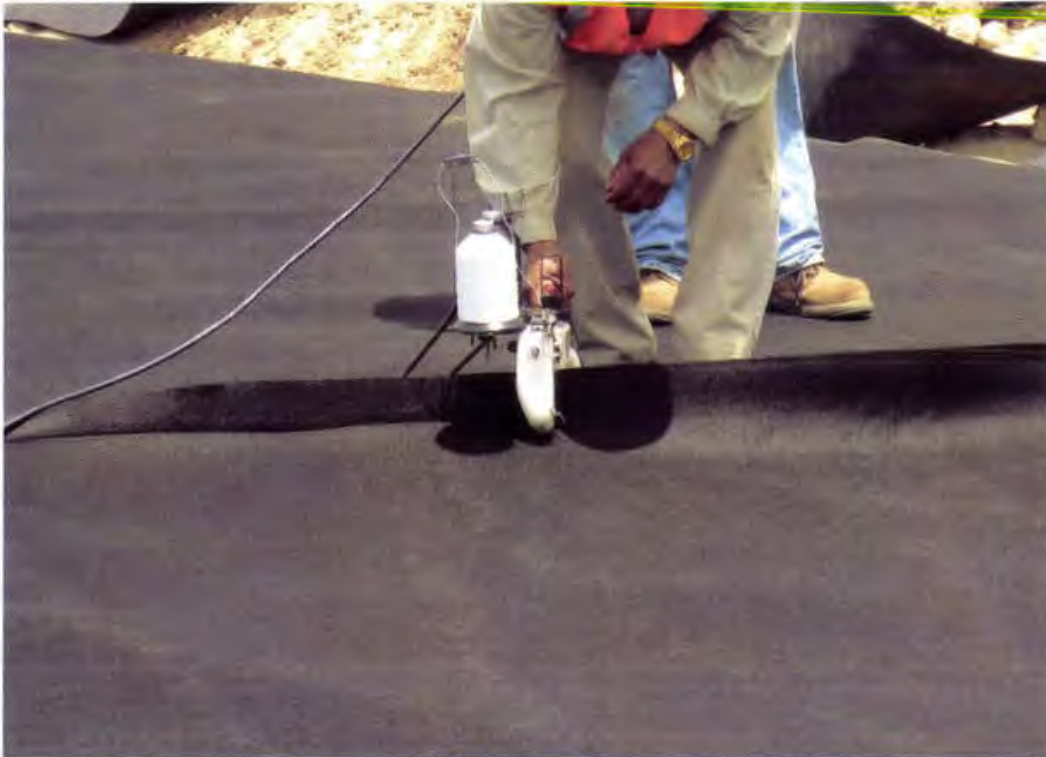
Photo 115. Sewing 16 oz/sy nonwoven cushion geotextile panels using single-prayer seams
