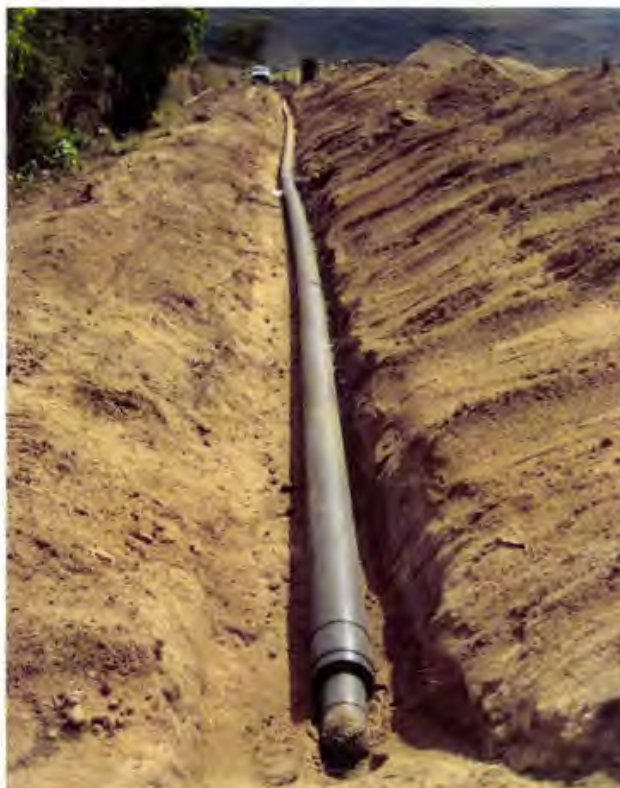
Photo 41. Dual containment (8"φ x 12"φ) HDPE conveyance pipe from the southern stubout (for future expansion) to Wet Well #3 (looking north)
