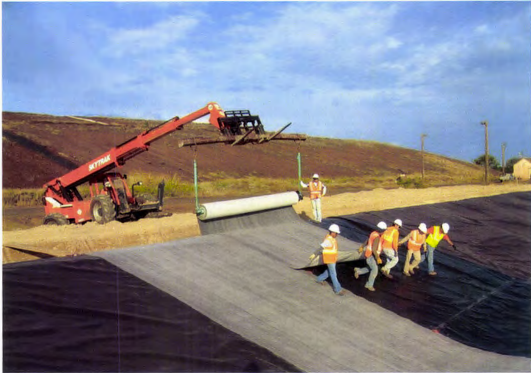
Photo 39. Deploying secondary GCL above the approved subbase 60 mil HDPE geomembrane
