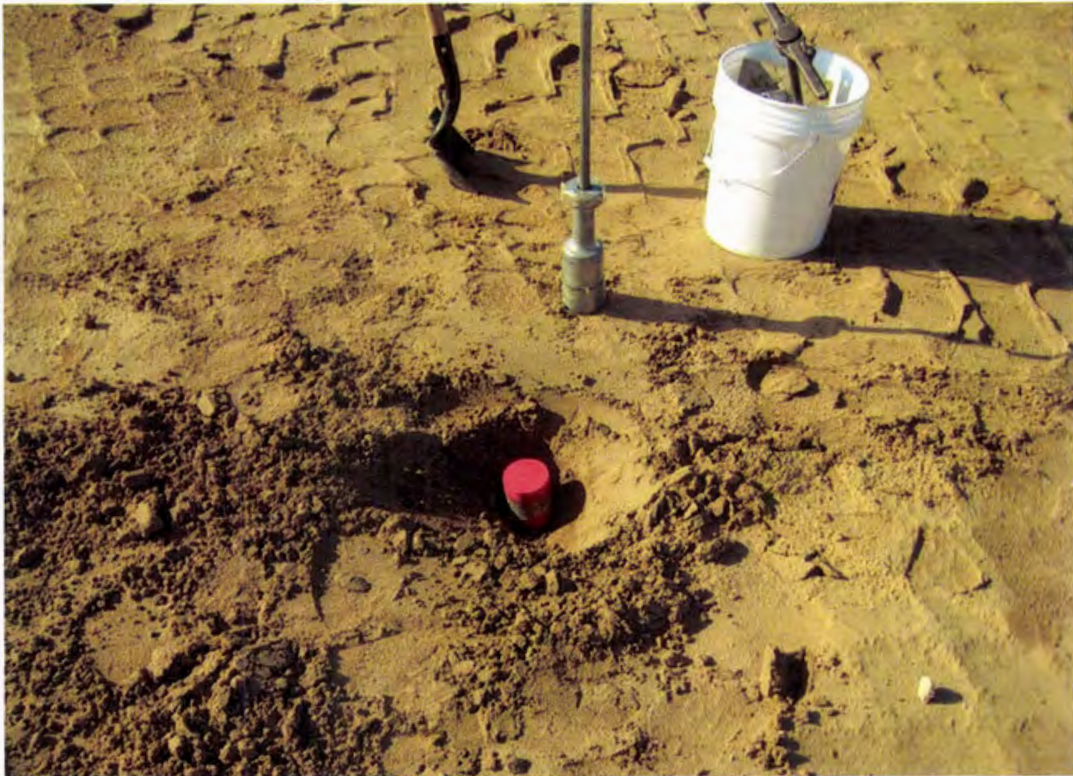
Photo 7. Collecting thin-wall Shelby tube samples for moisture-density determination by the drive cylinder method
