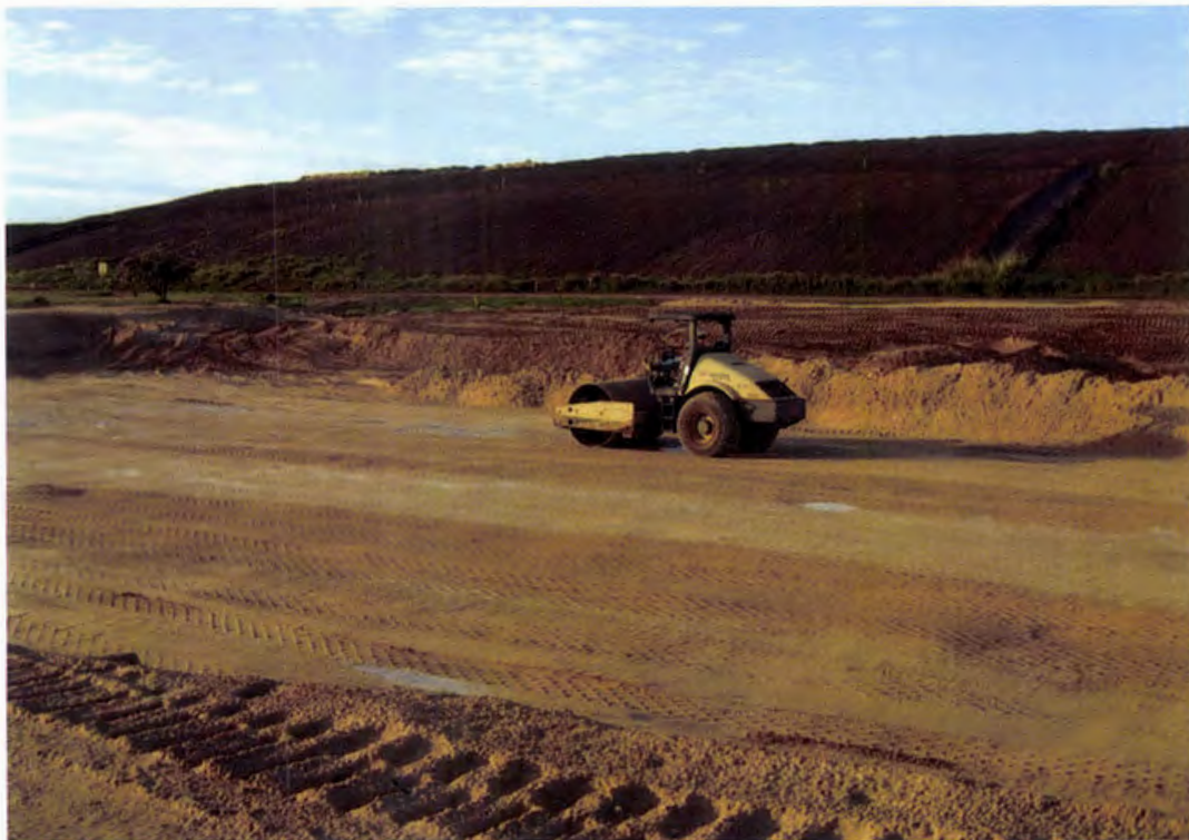
Photo 12. An Ingersoll-Rand SD122DX rubber tire smooth drum vibratory compactor rolls the subbase to maintain a suitable subbase surface (looking south)
