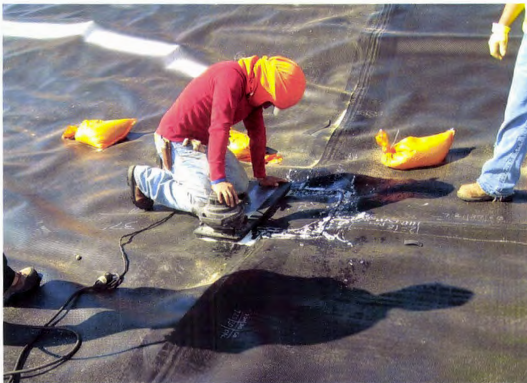
Photo 37. Non-destructive vacuum box testing the extrusion seam of a repair patch
