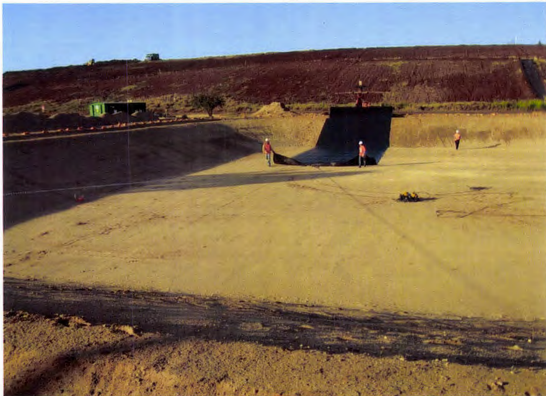
Photo 24. Deploying subbase 60 mil double-sided textured (DST) HDPE geomembrane over the prepared subbase (looking south)
