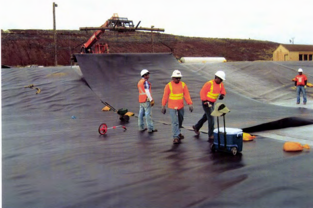
Photo 42. Secondary 60 mil HDPE geomembrane is deployed over the GCL panels to ensure all GCL is covered by the end of the each day.
