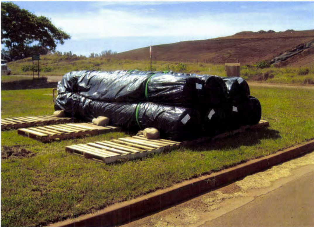
Photo 20. GCL rolls stockpiled on pallets near the administrative office area
