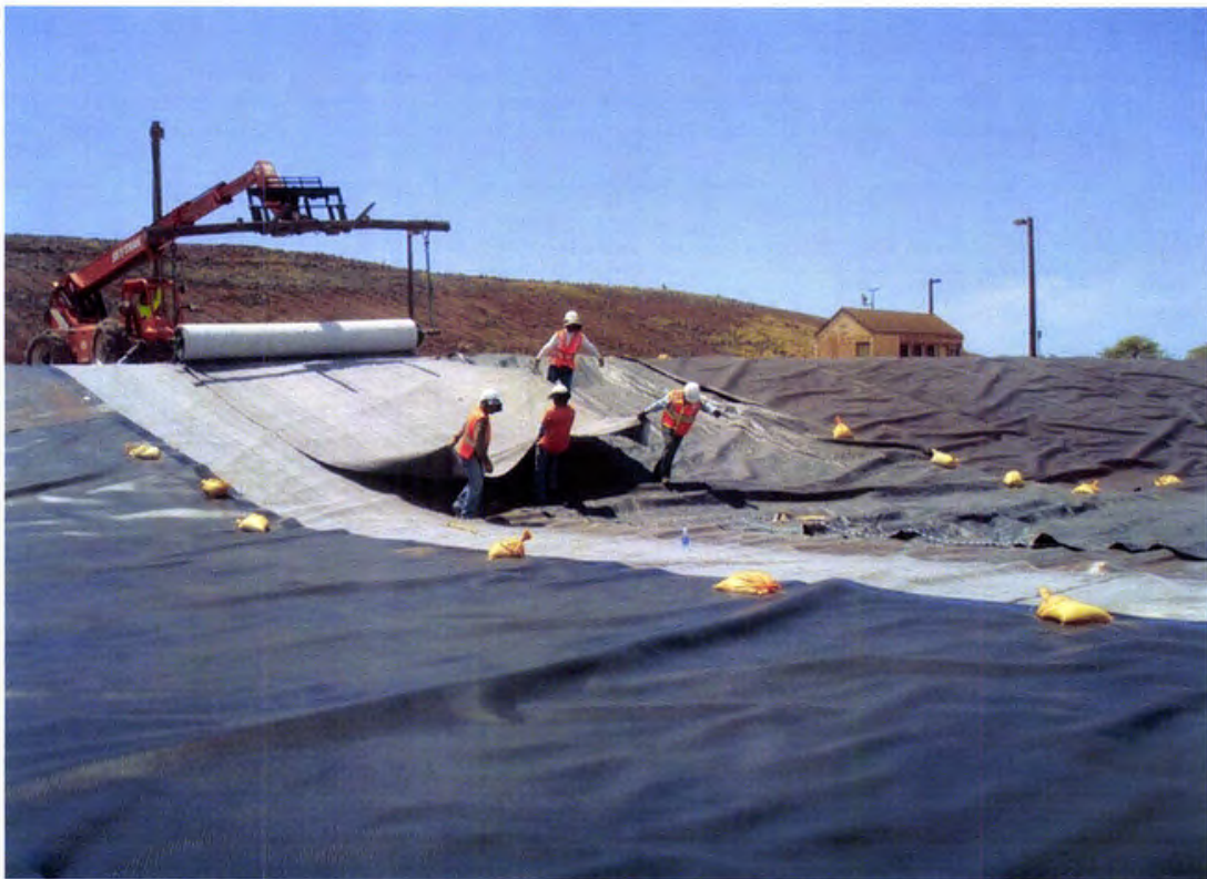
Photo 48. Deploying primary GCL above the approved secondary 60 mil HDPE geomembrane
