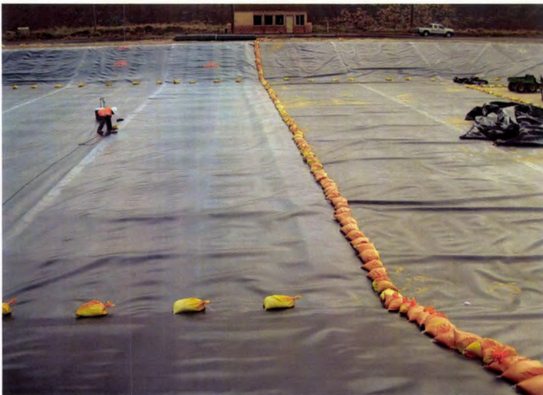
Photo 46. Leading edge of the secondary 60 mil HDPE geomembrane is sealed (extrusion welded and sandbagged) at the end of the day to protect the underlying GCL from premature hydration
