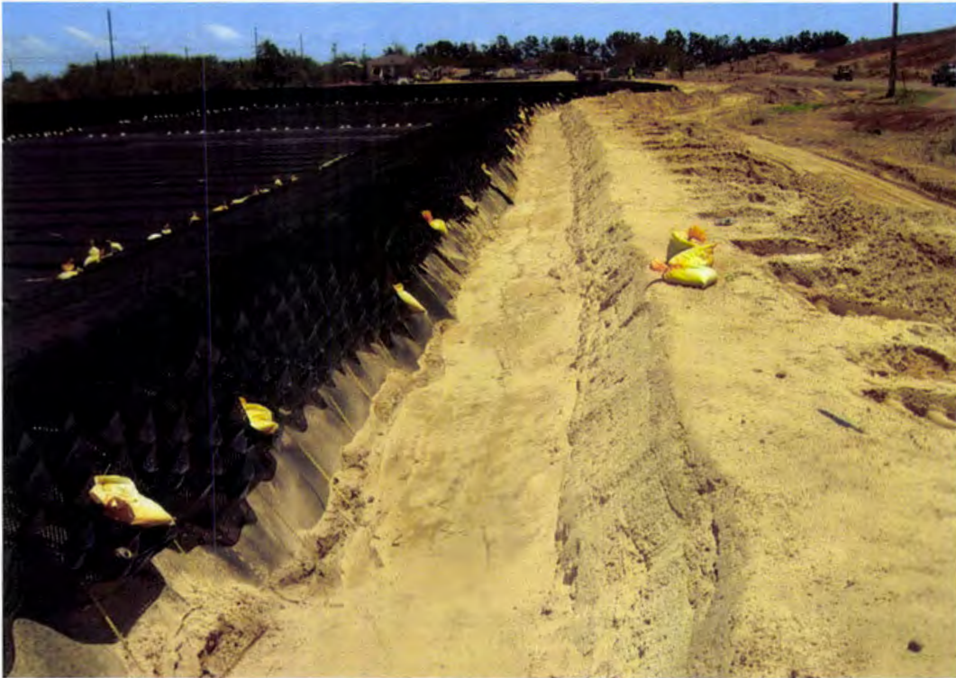
Photo 67. Partially backfilled and compacted perimeter anchor trench with a sand backfill (onsite soils) (looking east along south berm)
