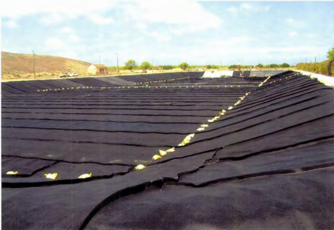
Photo 61. Majority of 16 oz/sy nonwoven cushion geotextile installed (with exception of west berm) (looking west)
