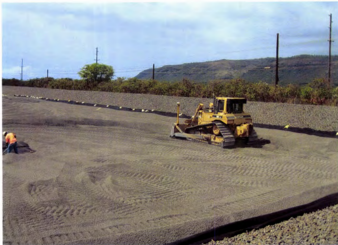
Photo 80. A Caterpillar LGP D6 dozer with GPS grade control grades the granular operations layer to a final 12-inch thick layer over the NLEP floor
