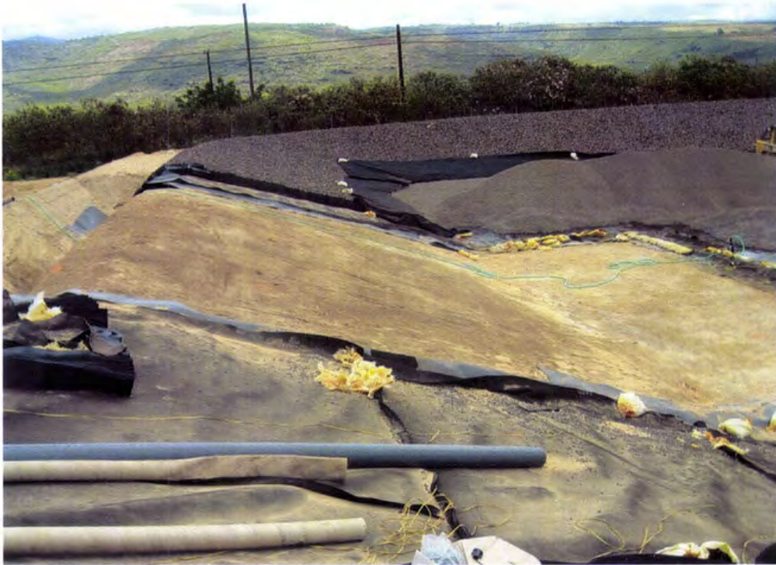
Photo 99. Completed NLEP west berm subbase and perimeter anchor trench (looking north)
