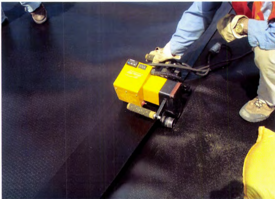
Photo 44. Production seaming secondary 60 mil HDPE geomembrane using a double-fusion wedge welder
