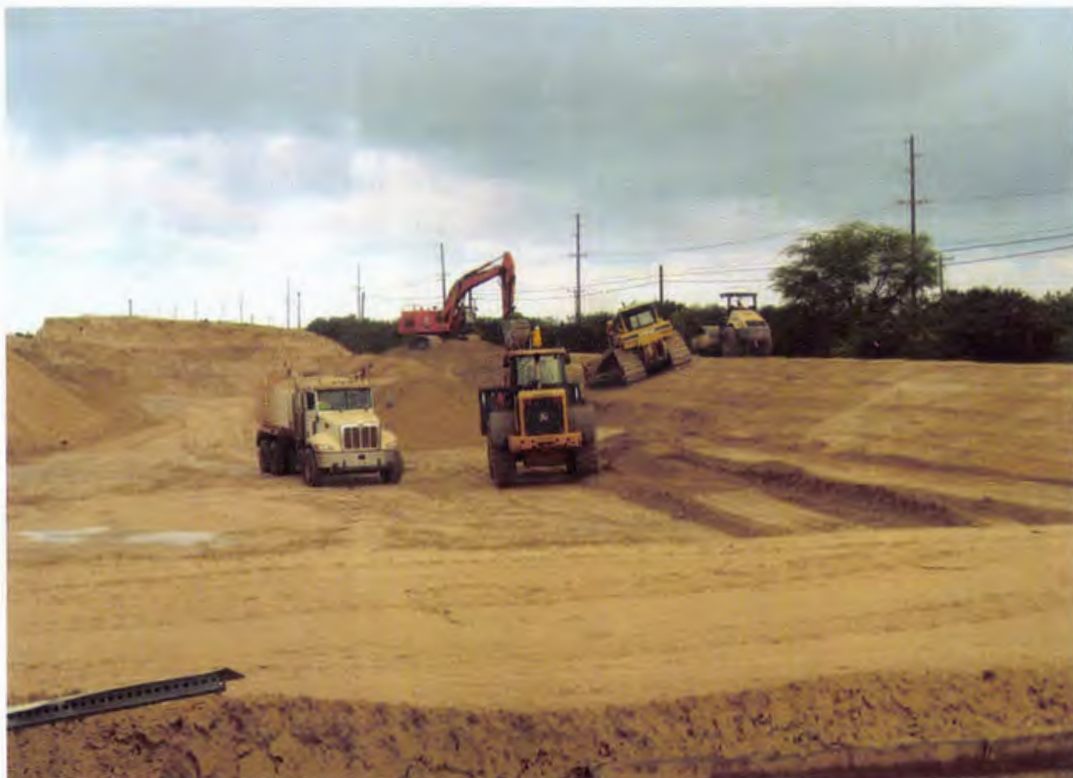
Photo 8. Grading and compacting the NLEP perimeter berm (looking west)
