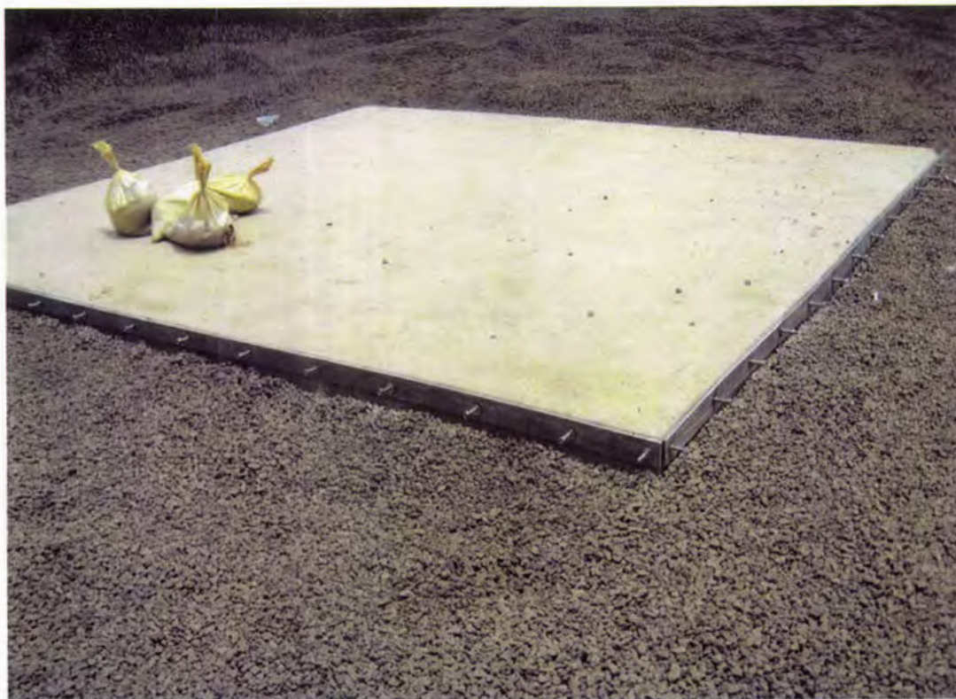
Photo 92. Completed concrete aerator pad
