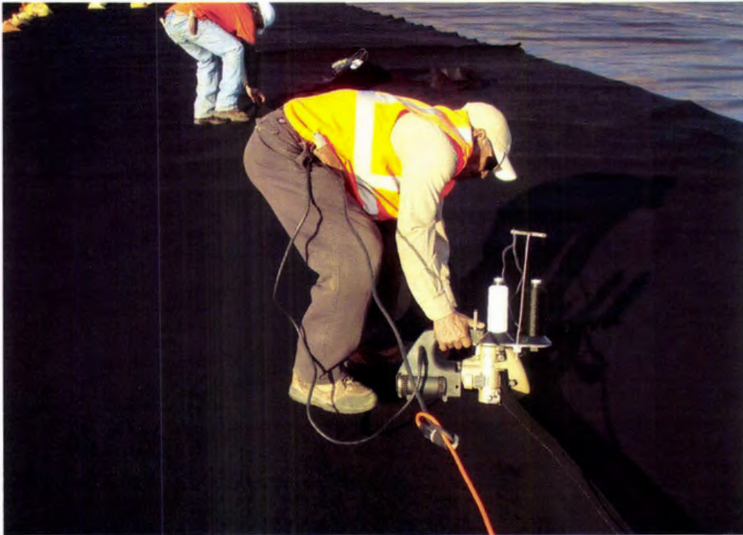
Photo 59. Sewing 16 oz/sy nonwoven cushion geotextile panels using single-prayer seams
