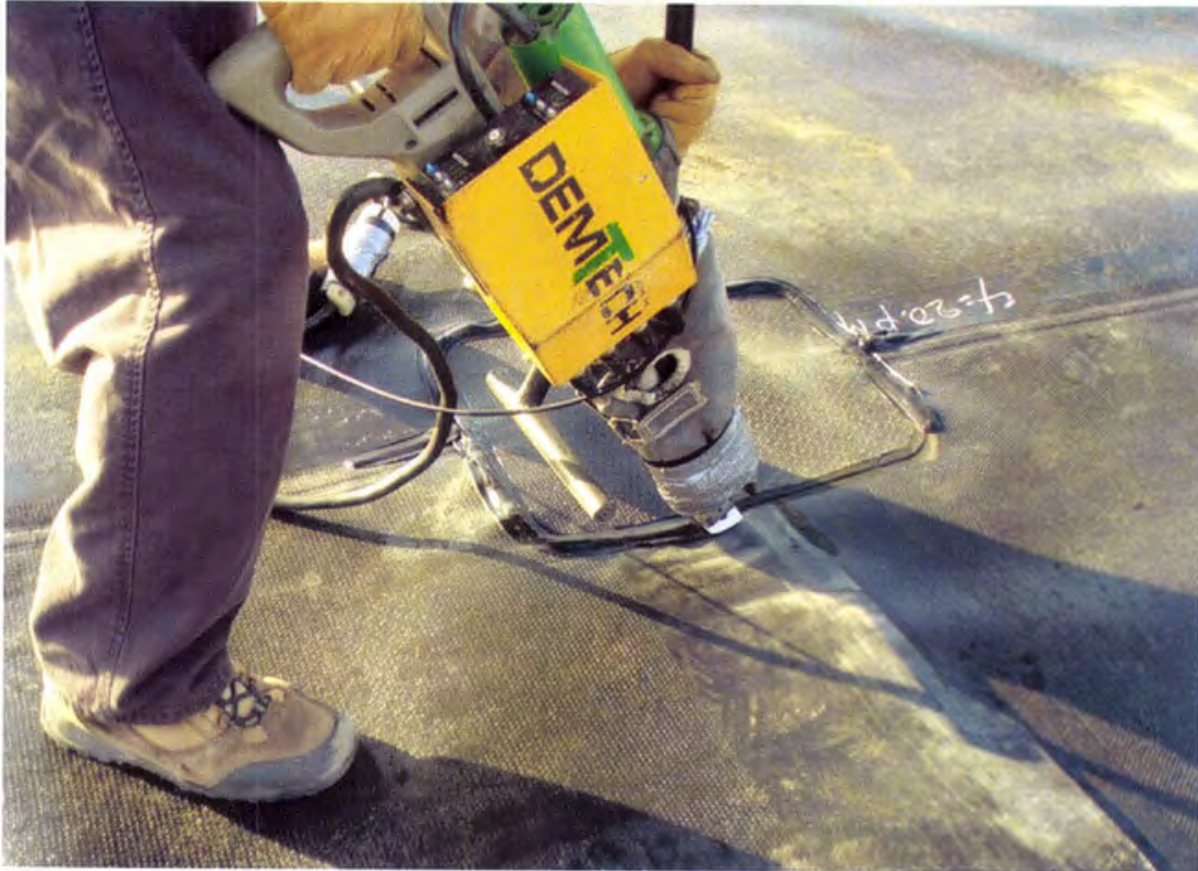
Photo 55. Extrusion welding a repair patch on the primary 60 mil HDPE geomembrane
