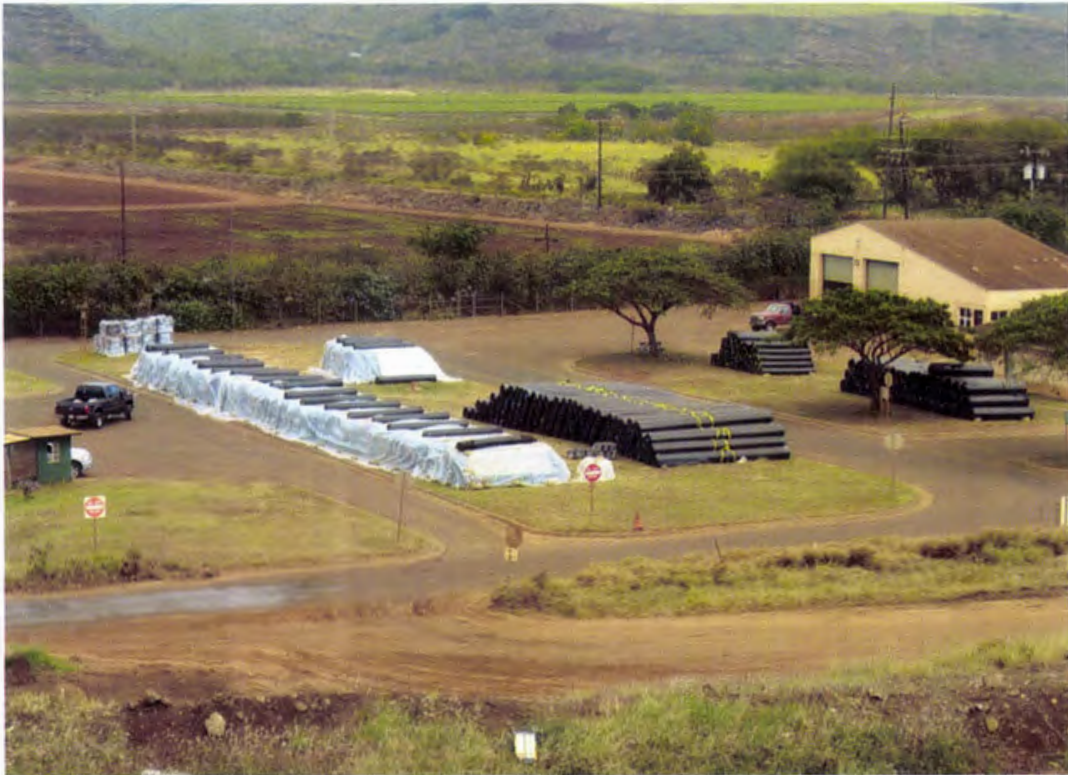
Photo 23. Complete geosynthetic inventory stockpiled adjacent to the administrative office area
