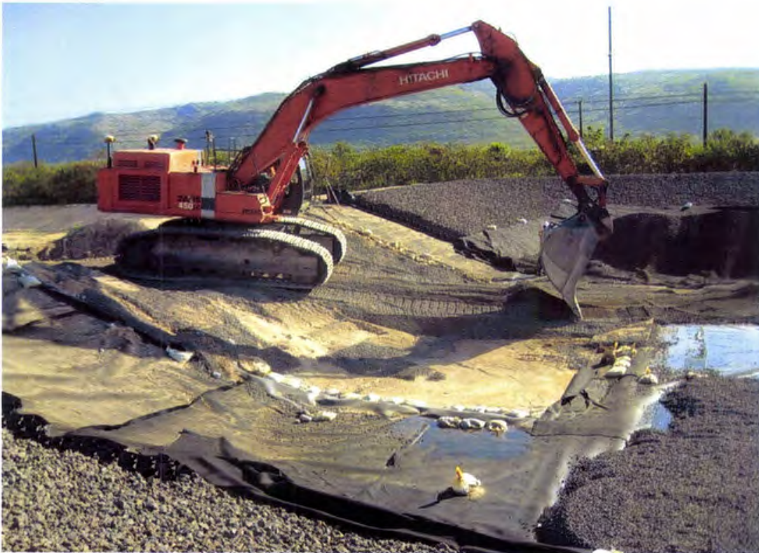
Photo 95. Once the majority of the granular protection layer is installed, the western temporary ramp area is cleaned in preparation for completion of the west berm construction (looking northwest)
