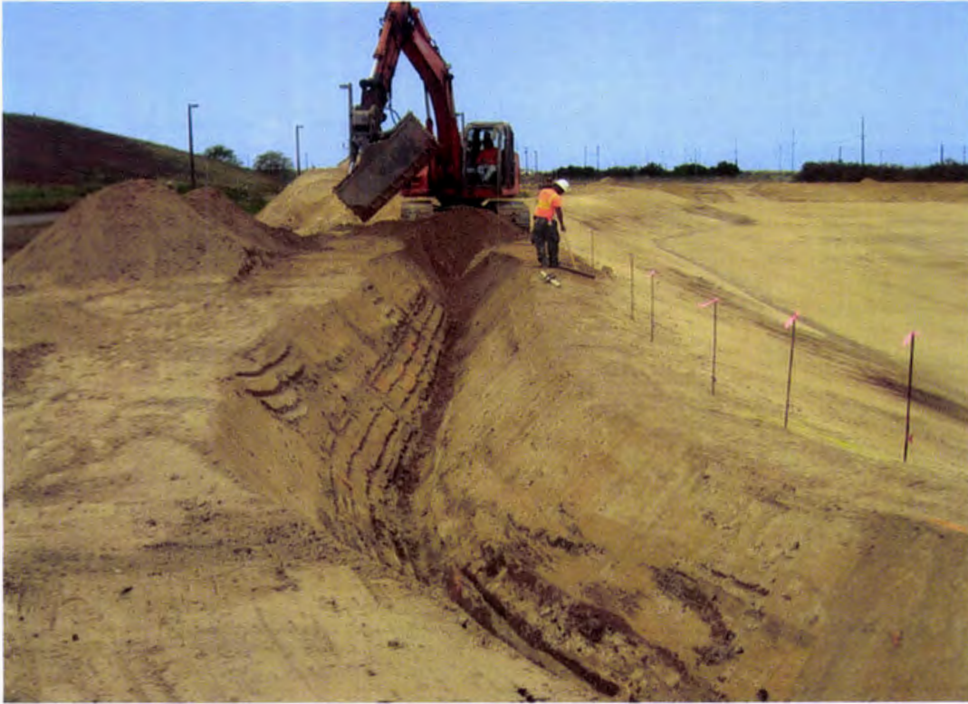
Photo 15. Constructing the perimeter anchor trench along the south berm (looking west)
