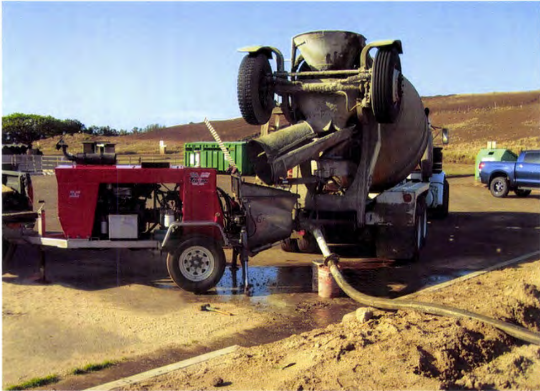
Photo 89. Concrete pump delivering concrete to the aerator pads
