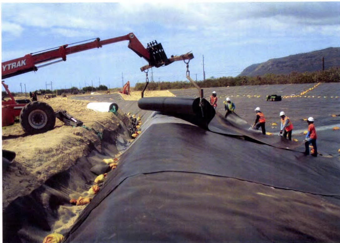
Photo 50. Deploying primary 60 mil HDPE geomembrane over completed secondary GCL
