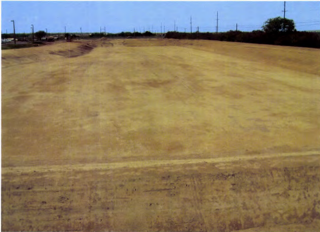
Photo 19. NLEP finished subbase with temporary west ramp left in place (looking west)
