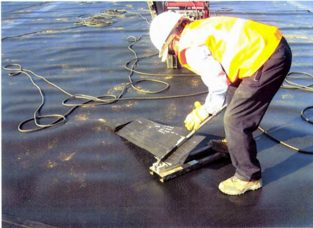
Photo 27. Coupons cut from the trial welds are tested (peel and shear) using a field tensiometer
