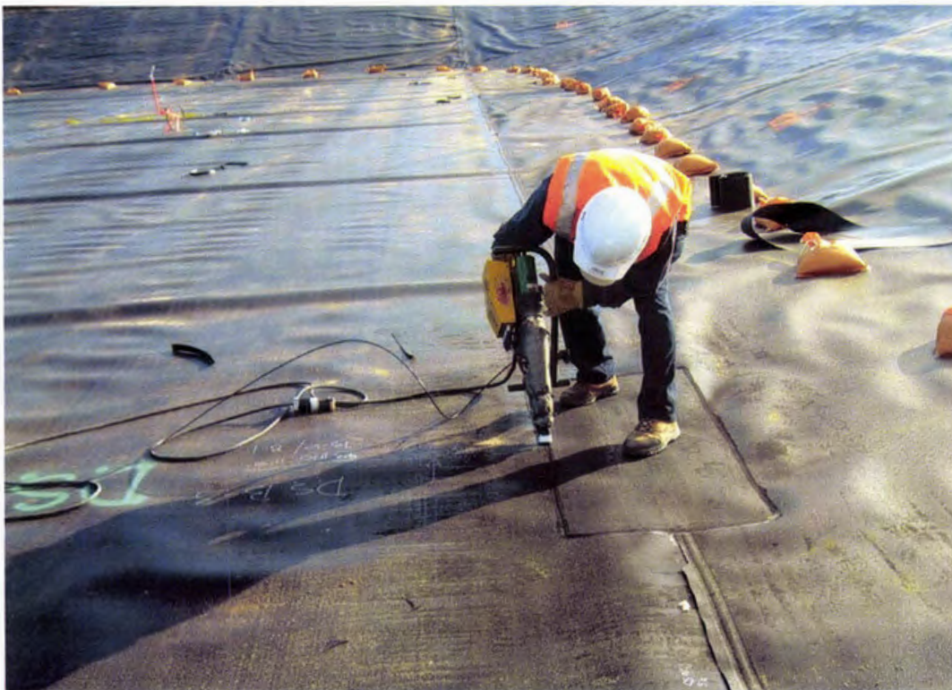
Photo 36. Extrusion welding a destruct repair patch within the subbase 60 mil HDPE geomembrane
