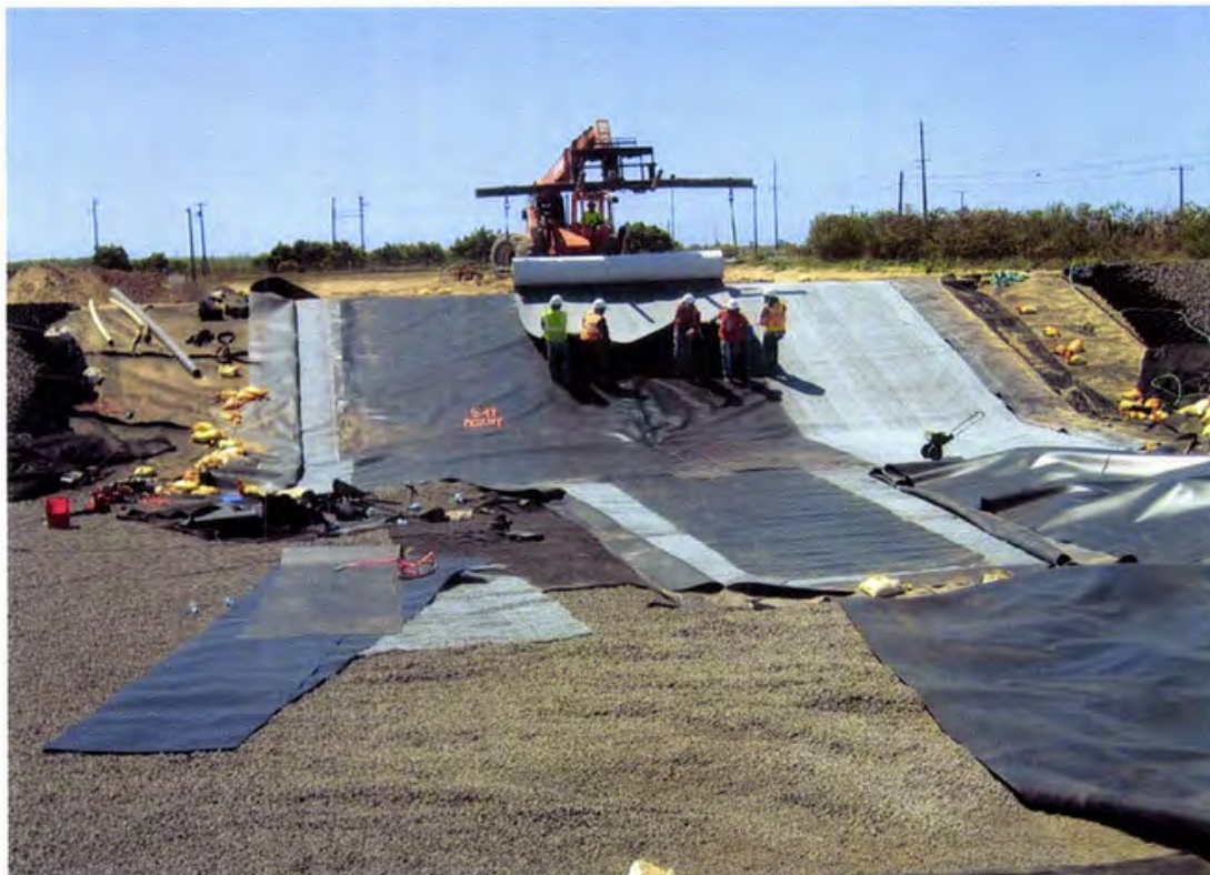
Photo 104. Deploying primary GCL above the approved secondary 60 mil HDPE geomembrane (looking west)
