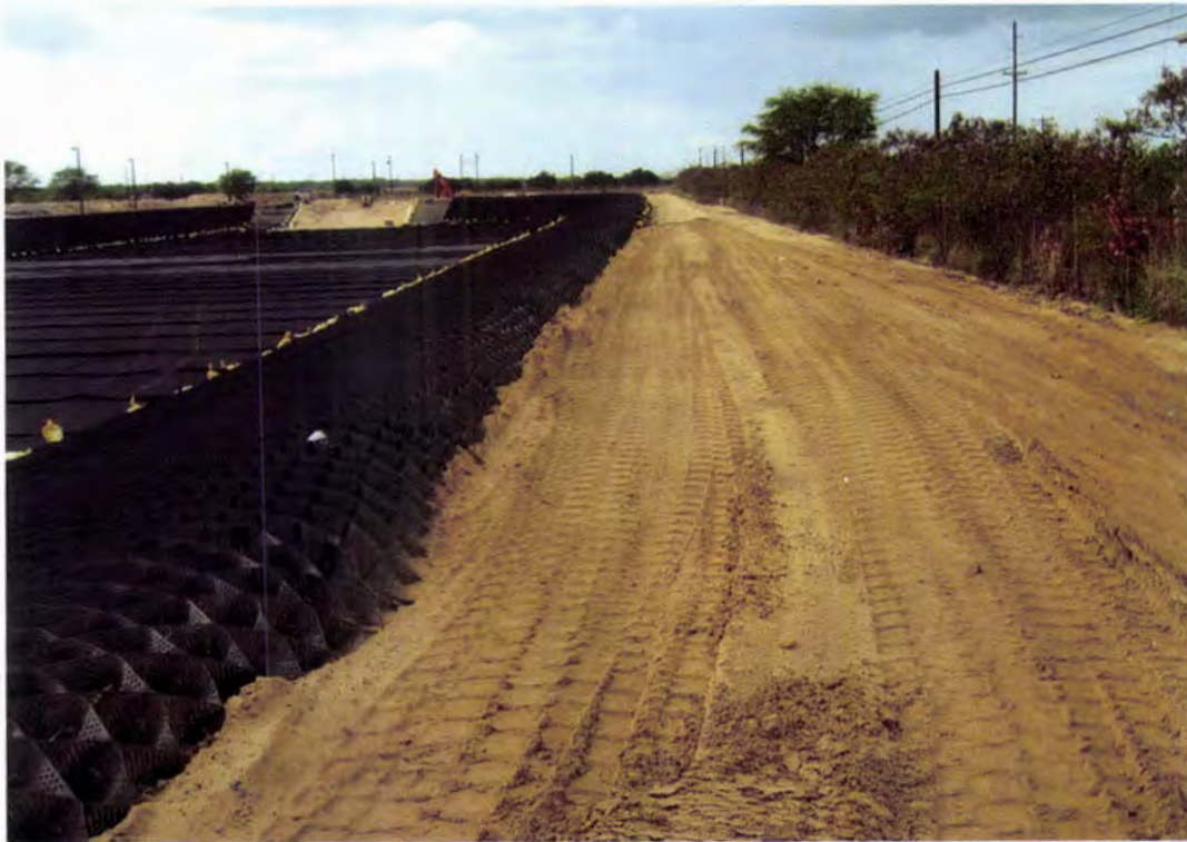
Photo 69. The perimeter anchor trenches are backfilled and compacted to the top with a sand backfill (onsite soils) (looking west)
