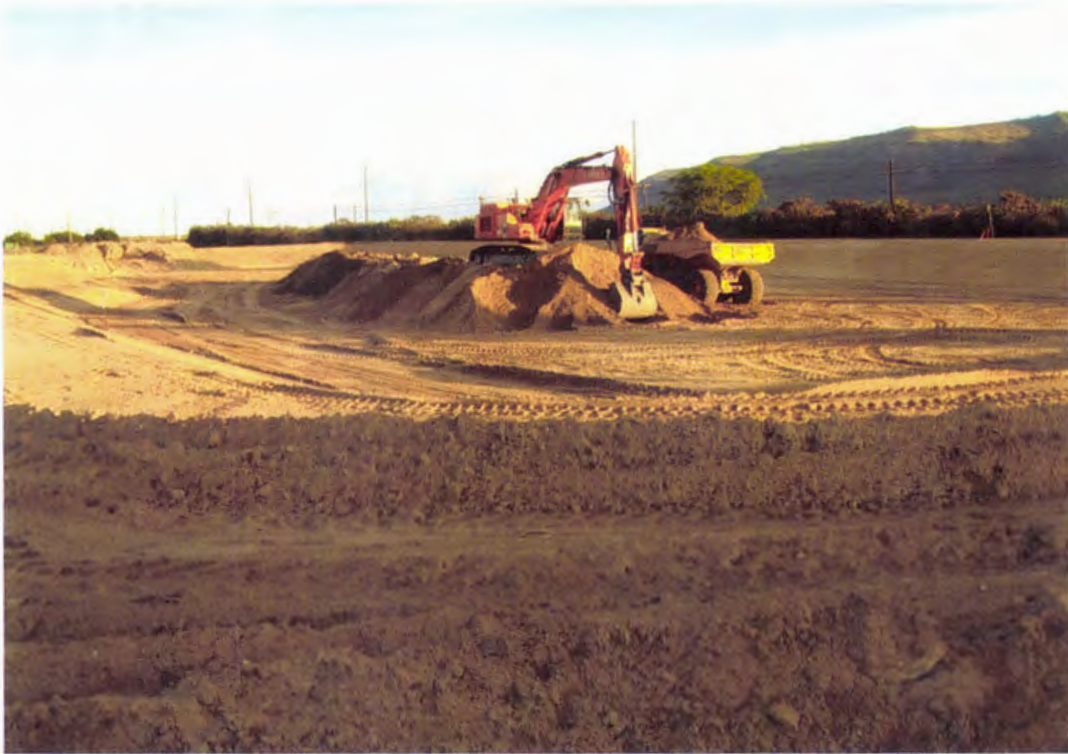
Photo 11. Trimmings from fine grading are loaded into an articulated haul truck and hauled to Cell 1 for use as compacted fill (onsite soils) (looking north)
