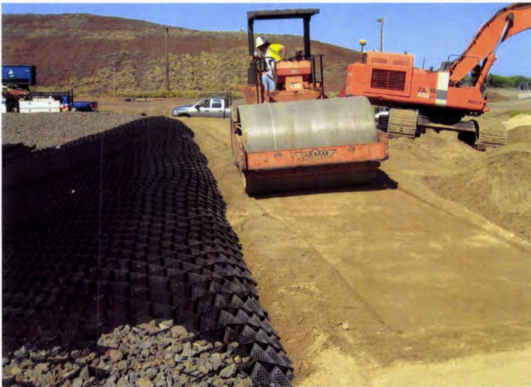
Photo 110. A HAMM 2420 rubber tire smooth drum vibratory compactor performs final compaction and rolling of the west perimeter berm (looking south)
