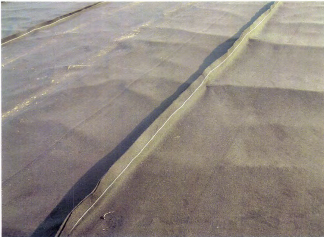
Photo 60. 16 oz/sy nonwoven cushion geotextile panels seams sewn using single-prayer seams
