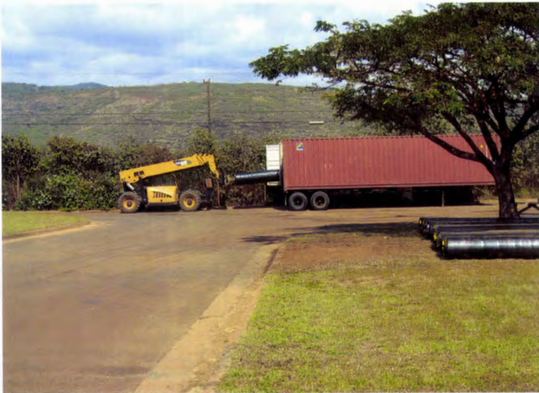
Photo 21. Unloading and stockpiling 16 oz/sy nonwoven geotextile rolls near the administrative office area
