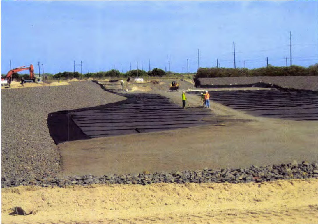
Photo 93. Installing the 2-inch thick granular protection layer above the 6 oz/sy nonwoven separator geotextile using a rubber tire track drive "skid steer" and manual hand raking (looking west)
