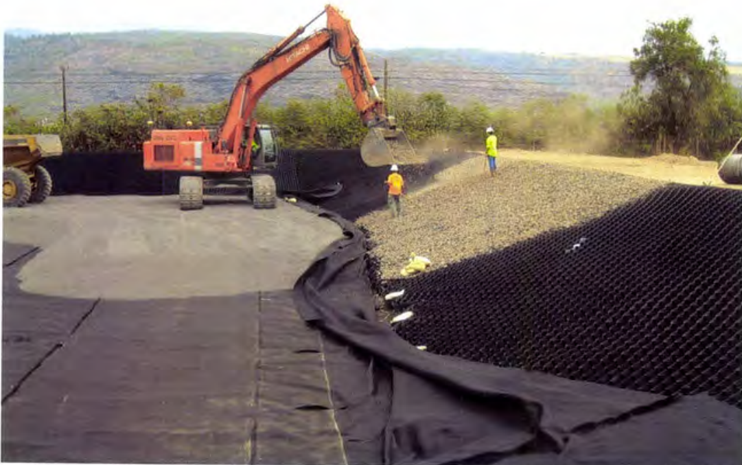
Photo 76. A Hitachi excavator and articulated haul truck work above a 3-ft to 4-ft thick granular operations layer road to bring and place 3-inch minus granular fill on the the NLEP sideslopes (looking north)
