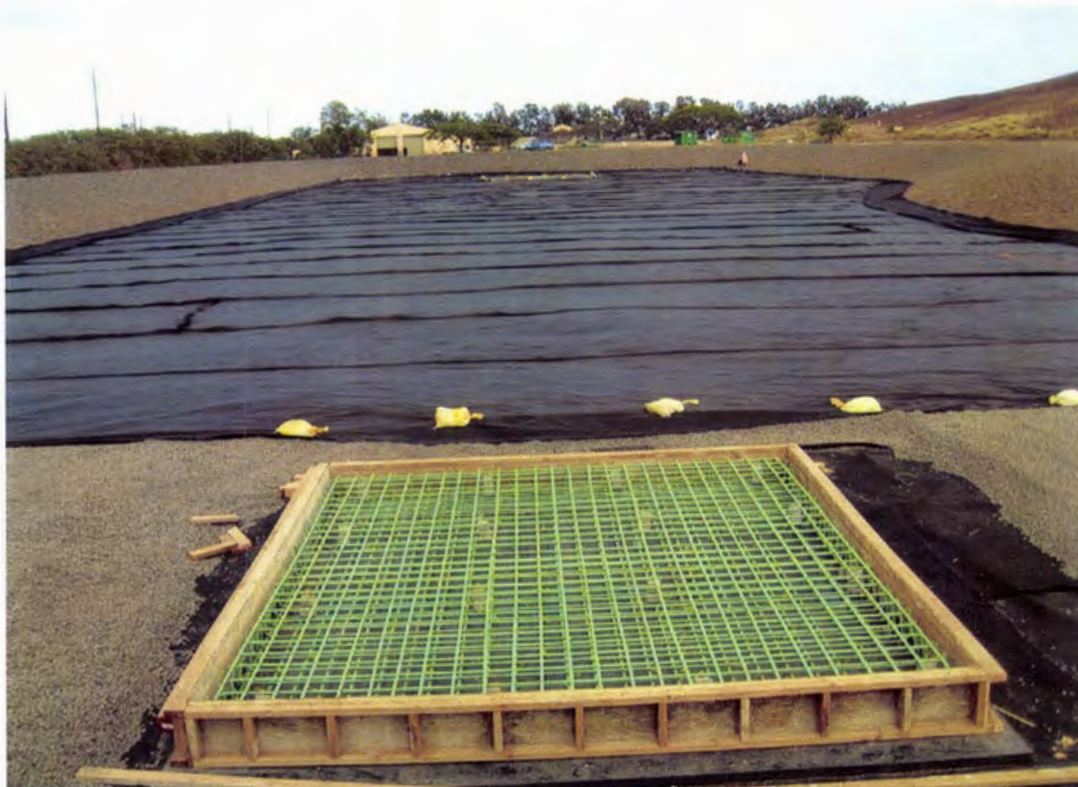
Photo 88. 6 oz/sy nonwoven separator geotextile installed above the granular operations layer (looking east)
