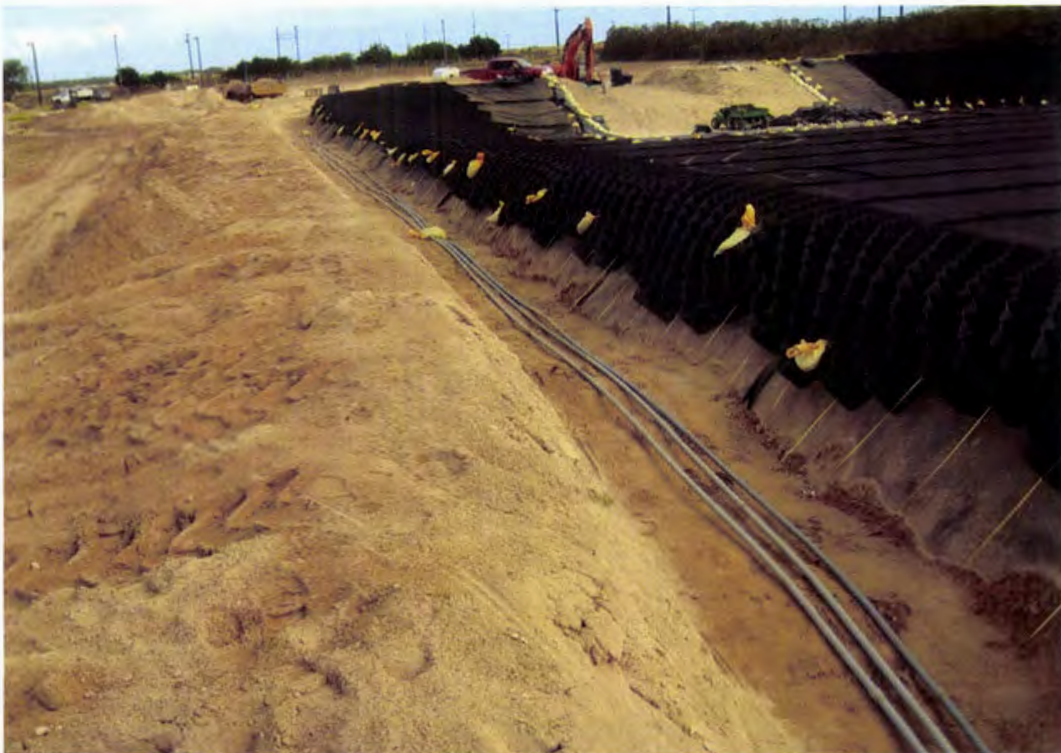
Photo 68. Three 2-inch diameter PVC electrical conduits are installed with marker tape within the southern perimeter anchor trench (looking west)
