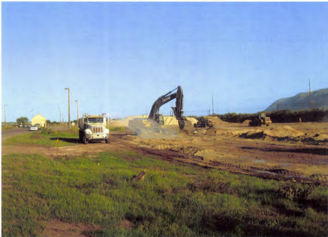
Photo 4. A water truck provides moisture conditioning during compacted fill placement (looking west)
