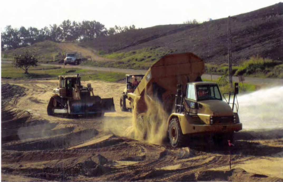
Photo 3. The excavated material is placed as compacted fill (onsite soils) to construct the NLEP berms and graded to uniform 8-inch loose lifts using a Caterpillar D6 LGP dozer
