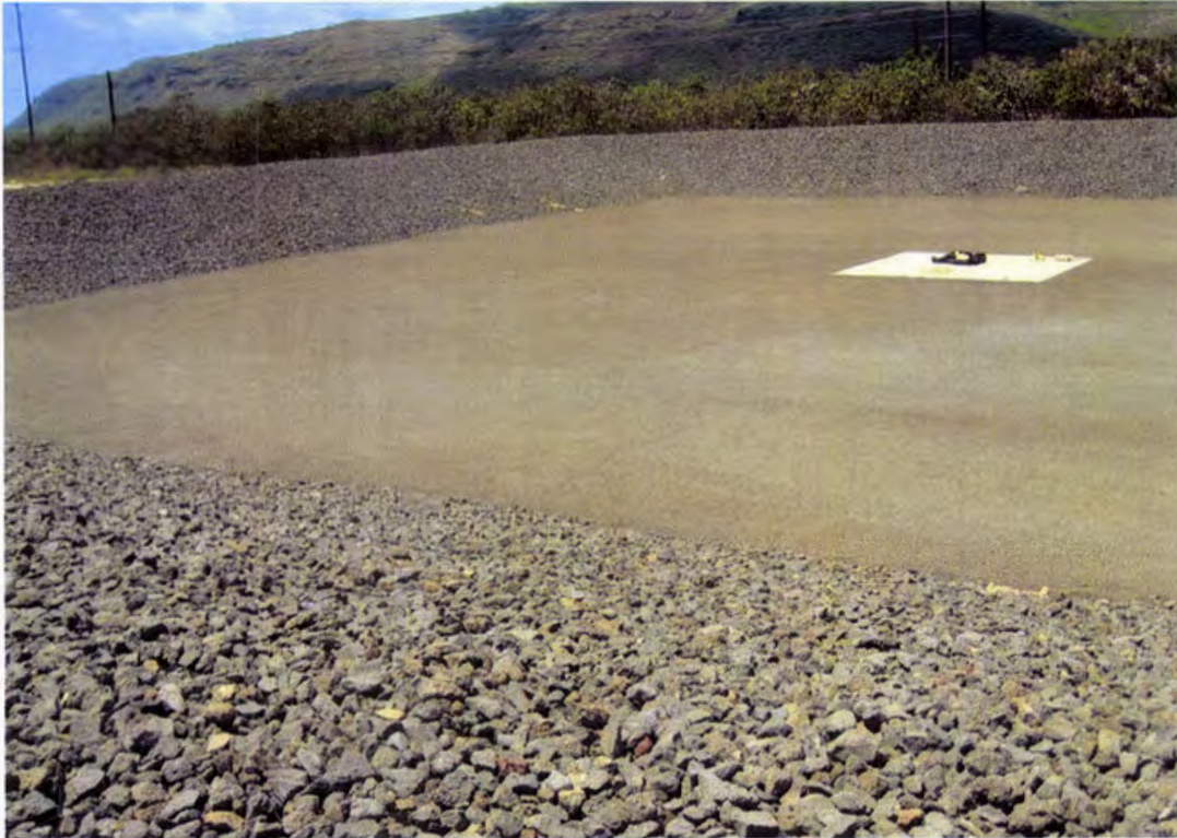
Photo 113. 2-inch thick granular protection layer is installed and graded over the 6 oz/sy nonwoven separator geotextile (looking northwest)
