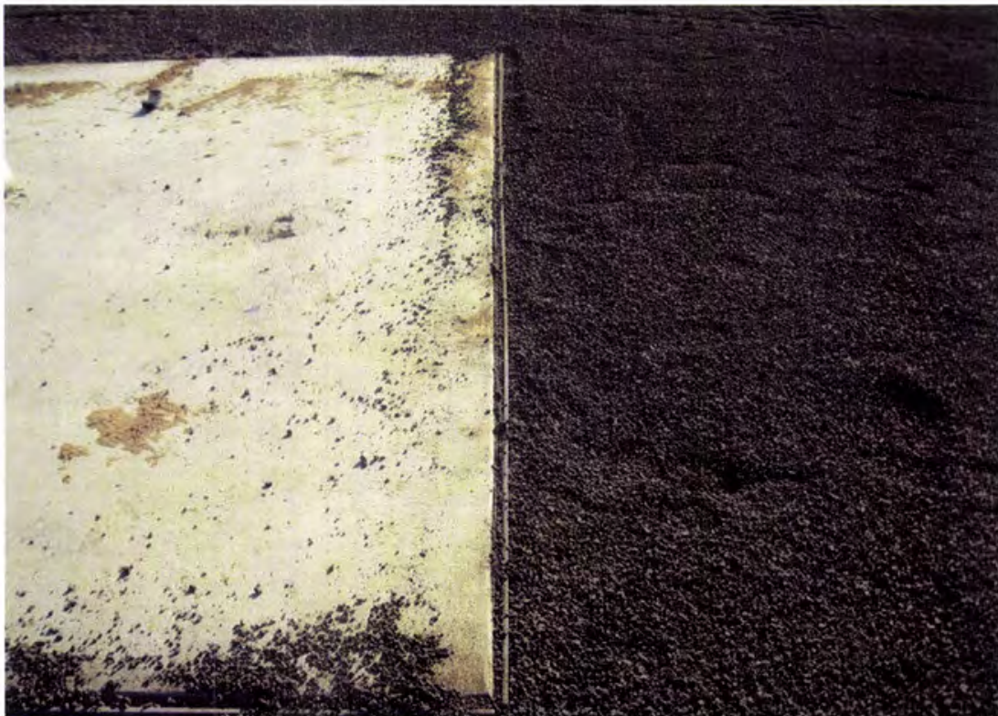
Photo 94. The 2-inch thick granular protection layer is installed flush with the aerator pads with rubber seal and batten strip installed
