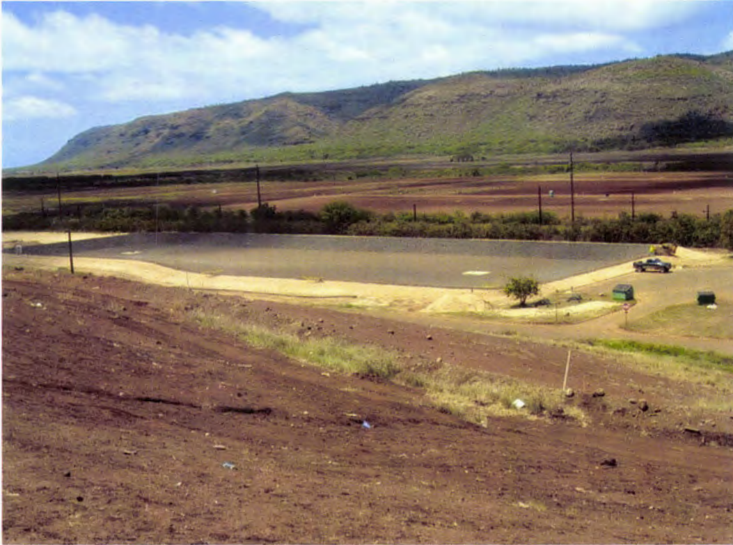
Photo 115. Completed NLEP containment system and aerator concrete pads (looking northwest)
