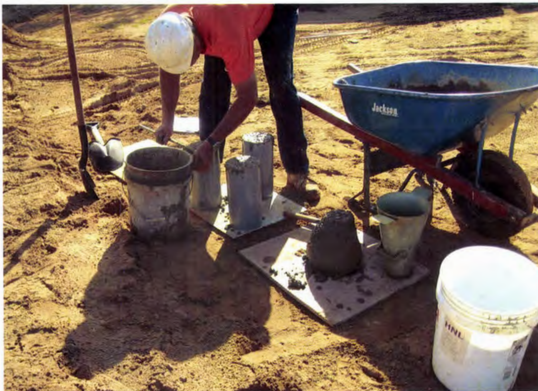
Photo 91. Hirata & Associates performs the slump cone test and collects cylinders for the concrete mix
