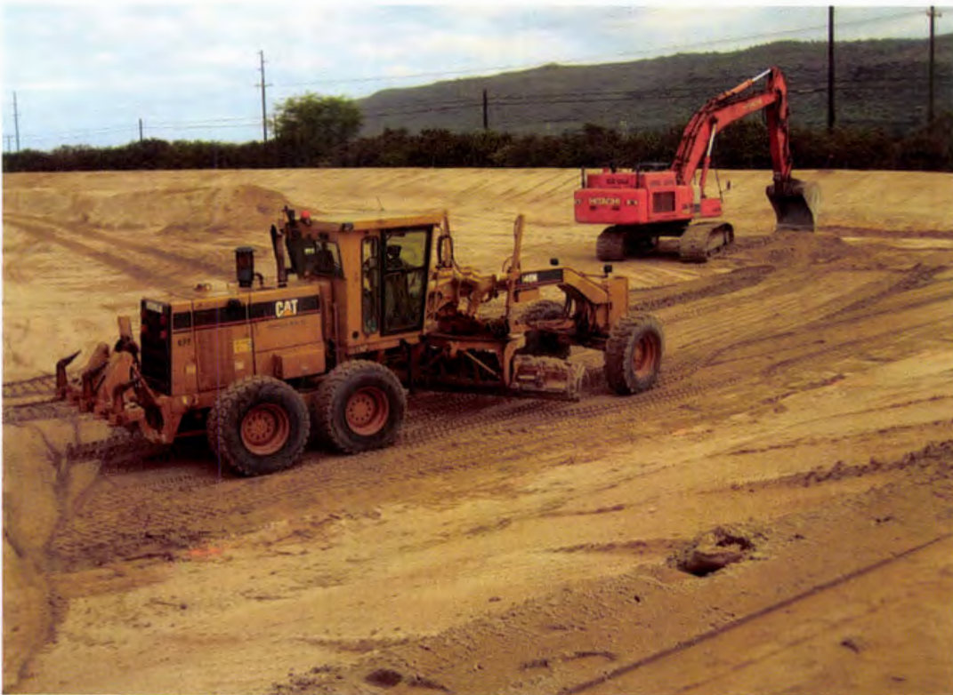
Photo 10. Fine grading the floor and sideslope subbase using a Caterpillar 140H motor grader with GPS grade control (looking north)
