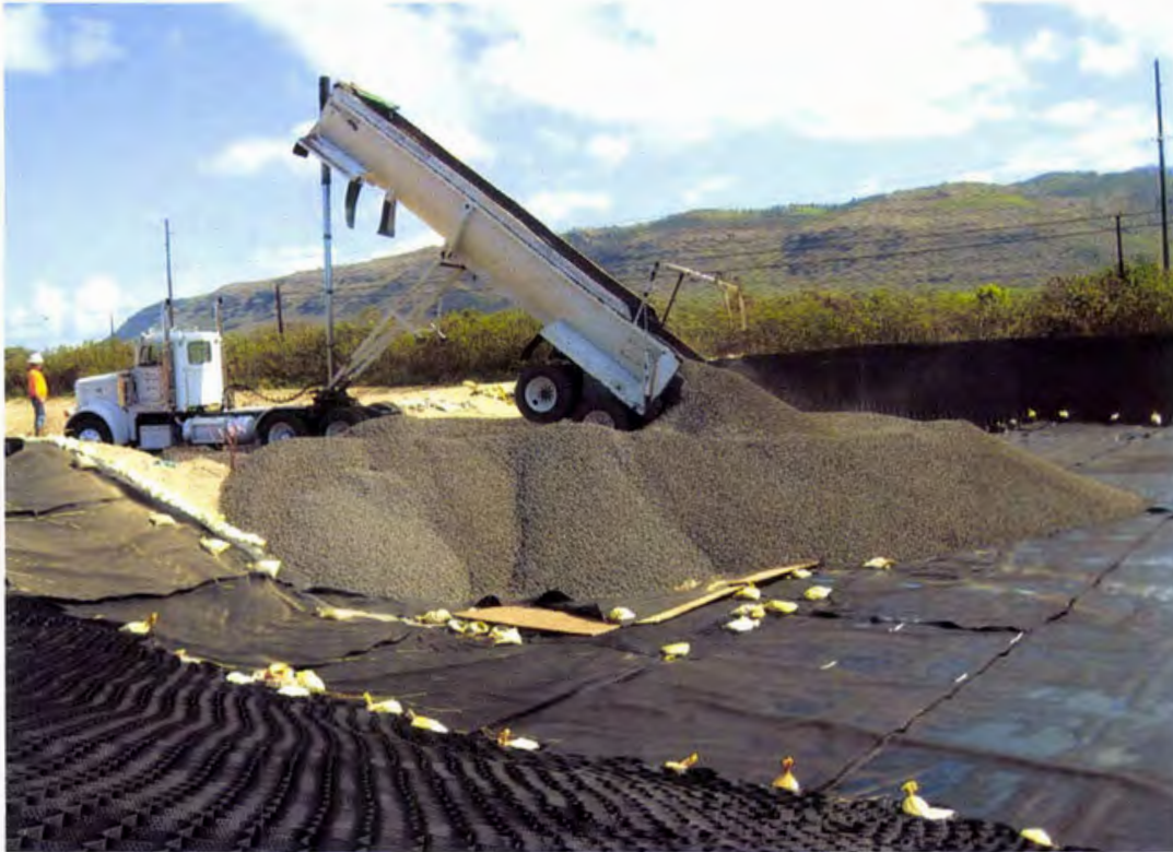
Photo 73. Imported 3/8-inch minus granular operations layer material is stockpiled directly in the NLEP
