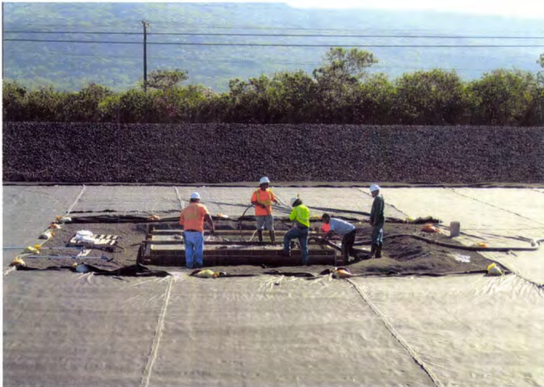
Photo 90. Concrete is pumped into aerator pad forms (looking north)
