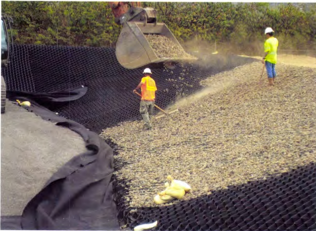
Photo 77. The 3-inch minus granular fill is backfilled and spread in the Geocell using hand tools
