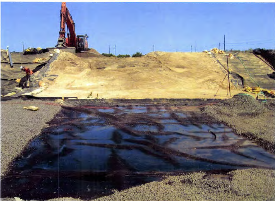
Photo 96. Trimmings from the NLEP exterior south berm is used to construct the west berm (looking west)
