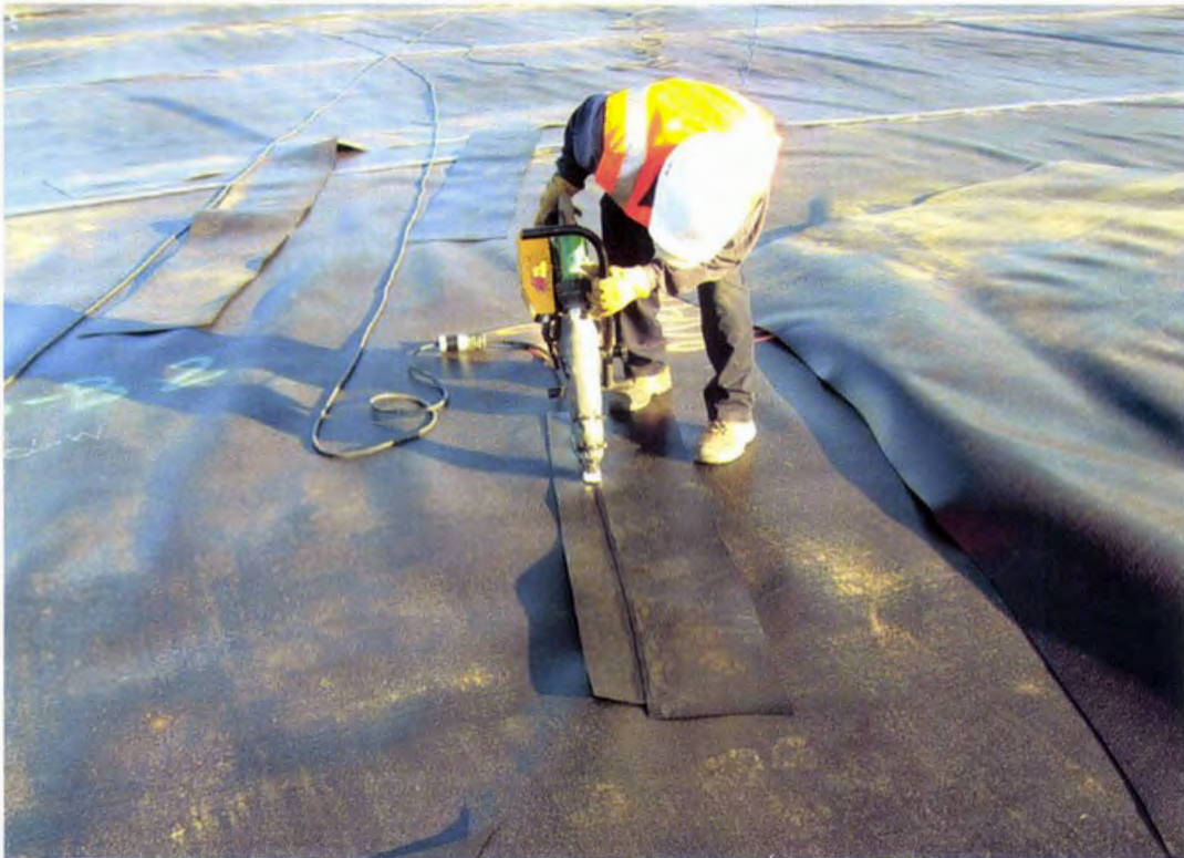
Photo 25. Trial welds are prepared at the start of the day and at midday for each welding apparatus and material combination used that day (extrusion welding textured-to-textured 60 mil HDPE geomembrane shown above)
