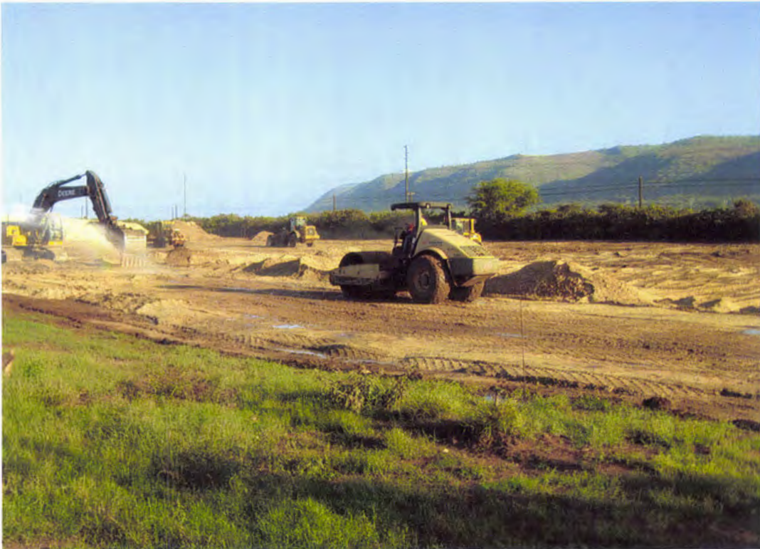
Photo 5. NLEP subbase is compacted using an Ingersoll-Rand SD122DX rubber tire smooth drum vibratory compactor (looking west)
