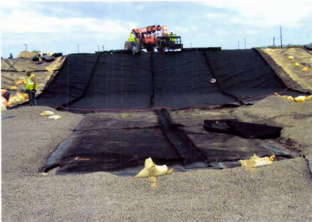
Photo 107. 16 oz/sy nonwoven cushion geotextile installed above the primary geomembrane (looking west)
