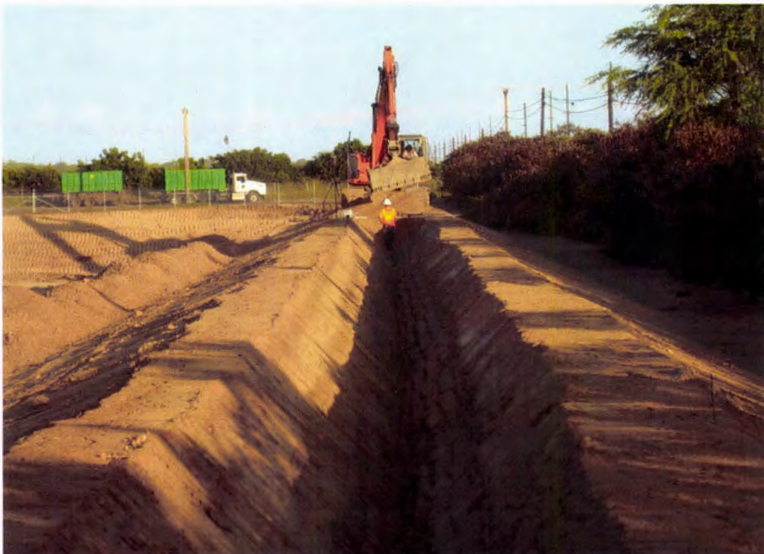
Photo 14. Constructing the perimeter anchor trench using a Hitachi BH278 excavator (looking west)
