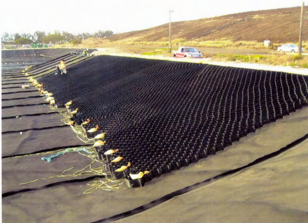
Photo 62. Installing Presto-manufactured Geoweb® GW30V8 Geocell on the NLEP sideslopes above the completed 16 oz/sy nonwoven cushion geotextile (looking east)
