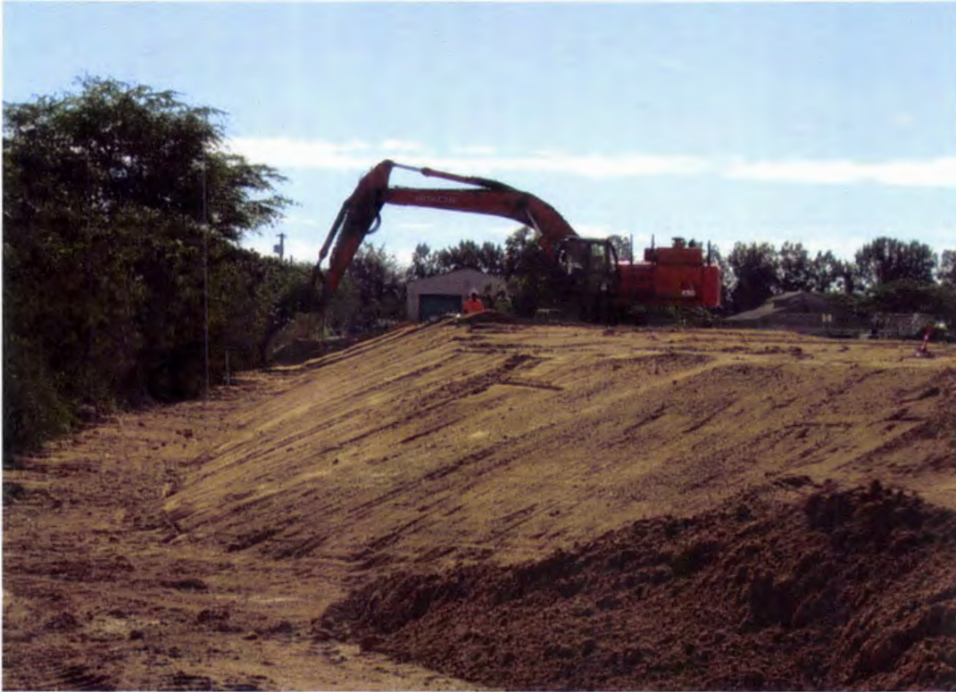
Photo 9. Grading the exterior slopes of the perimeter berms using a Hitachi 450 LC excavator (looking south)
