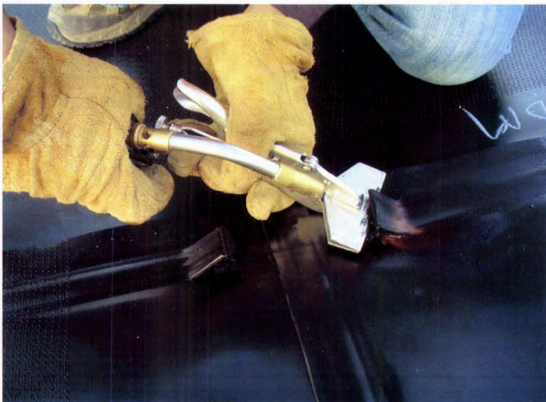
Photo 52. Sealing a double-fusion welded production seam in preparation for a non-destructive air test
