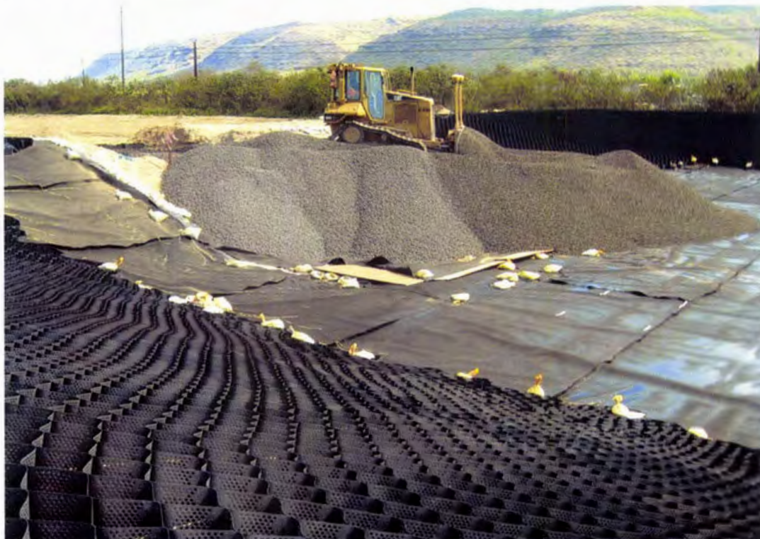
Photo 74. A Caterpillar LGP D6 dozer with GPS grade control pushes the stockpiled 3/8-inch minus granular operations layer material across the NLEP floor
