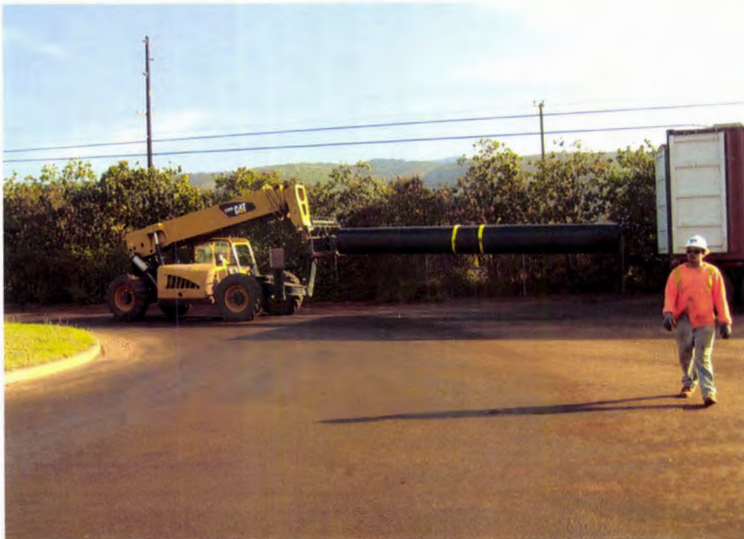
Photo 22. Unloading Agru 60 mil double-sided textured HDPE Microspike geomembrane rolls
