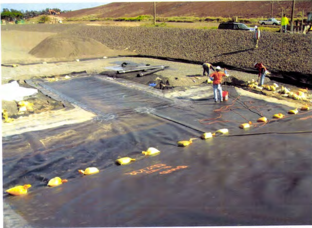
Photo 105. Completed primary 60 mil HDPE geomembrane installed above the primary GCL (looking southeast)
