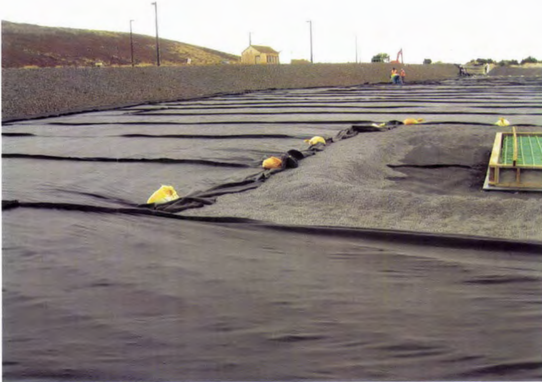
Photo 87. Sewing 6 oz/sy nonwoven separator geotextile above the 12-inch thick granular operations layer (looking west)
