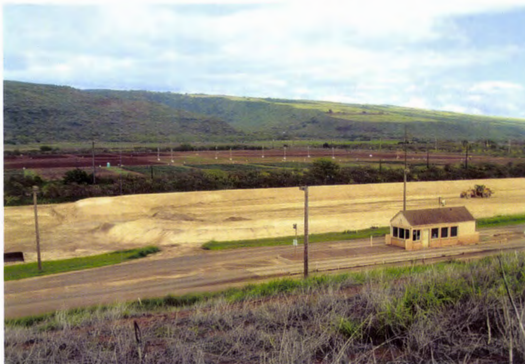
Photo 18. Temporary ramp (later removed) through west berm is left to allow import of granular drainage materials into NLEP
