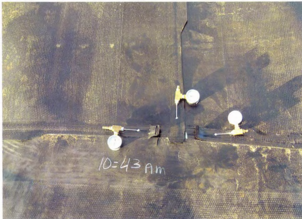
Photo 32. Non-destructive air pressure testing of double-fusion welded production seams
