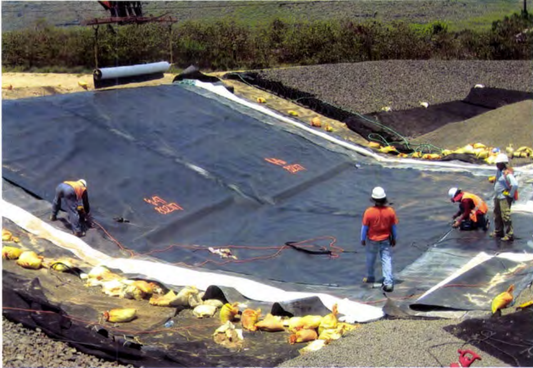
Photo 103. Production seaming and air testing the fusion welded production seams of the deployed secondary 60 mil HDPE geomembrane above the secondary GCL (looking northwest)
