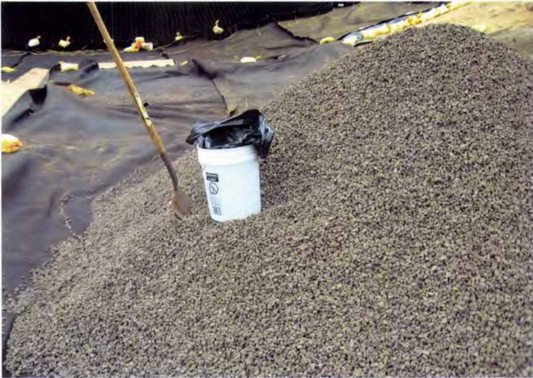
Photo 71. Collecting a sample of 3/8-inch minus granular operations layer material (imported from Kauai Aggregate Quarry) for conformance testing
