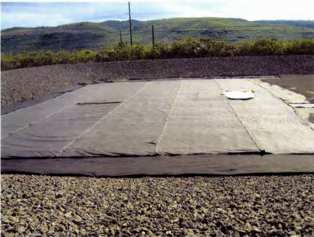
Photo 112. 6 oz/sy nonwoven separator geotextile is completed on the NLEP floor (looking north)
