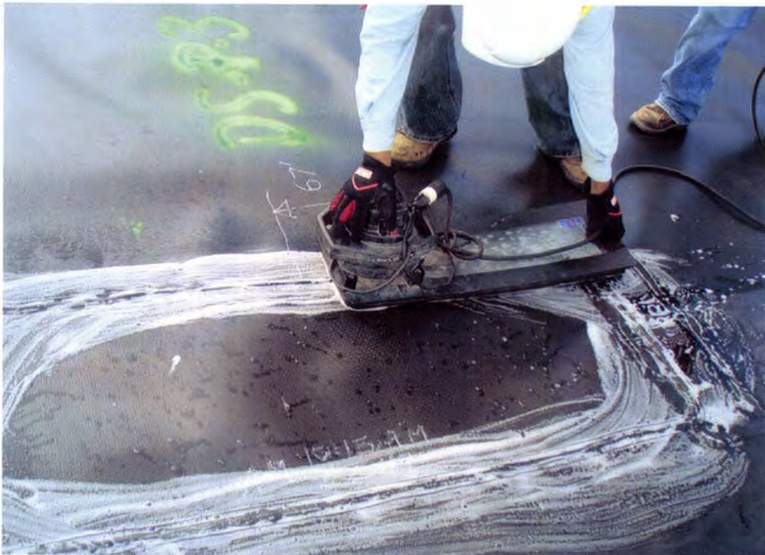
Photo 56. Non-destructive vacuum box testing the extrusion seam of a repair patch
