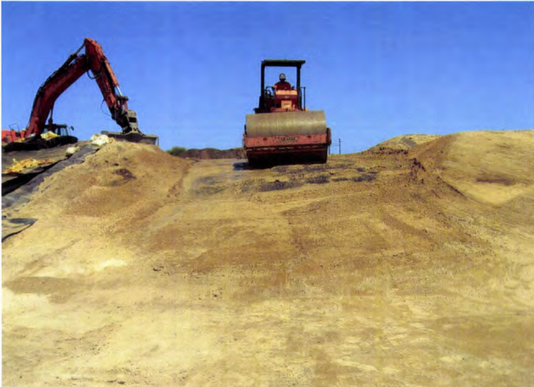
Photo 97. A HAMM 2420 rubber tire smooth vibratory compactor applies effort to the placed, moisture-conditioned compacted fill (onsite soils) (looking west)
