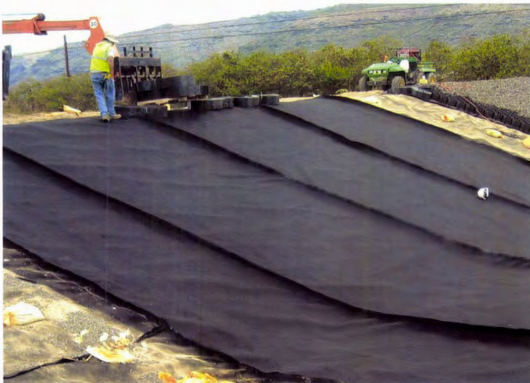
Photo 108. Installing the Geocell system above the 16 oz/sy nonwoven cushion geotextile (looking northwest)
