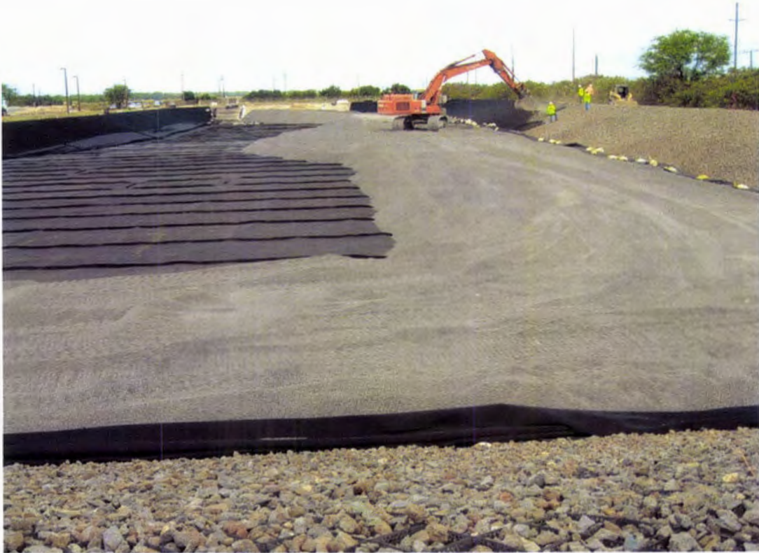
Photo 79. Backfilling Geocell on north sideslope with 3-inch minus granular fill (looking west)
