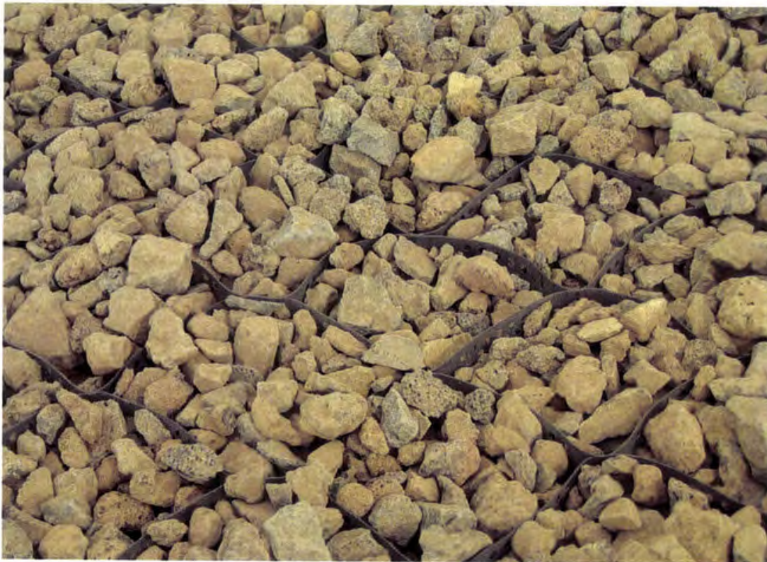
Photo 78. Geocell backfilled with 3-inch minus granular fill
