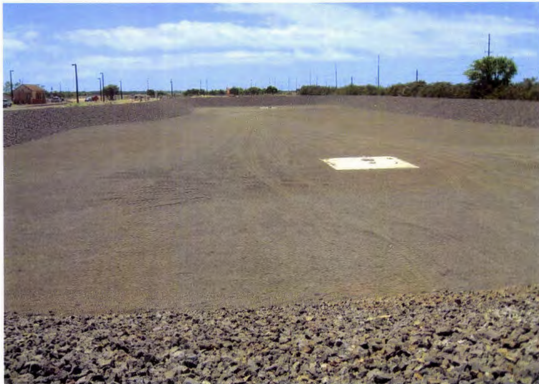
Photo 114. Completed NLEP containment system and aerator concrete pads (looking west)
