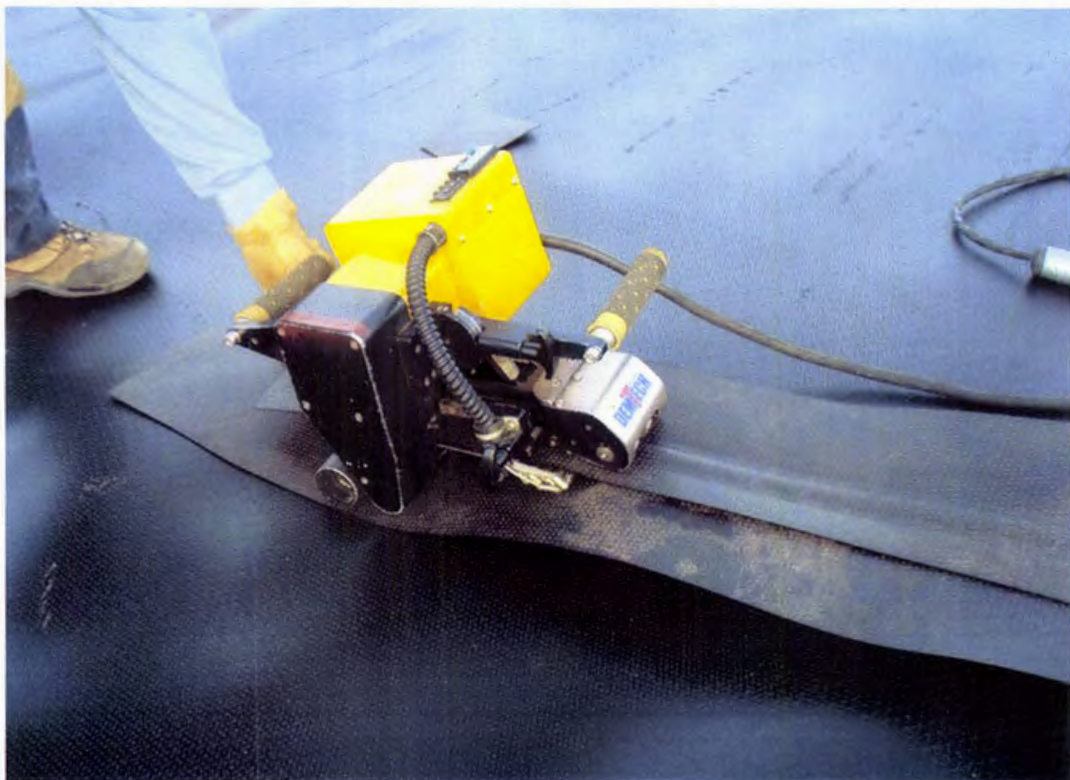
Photo 26. Preparing a double-fusion trial weld of textured-to-textured 60 mil HDPE geomembrane
