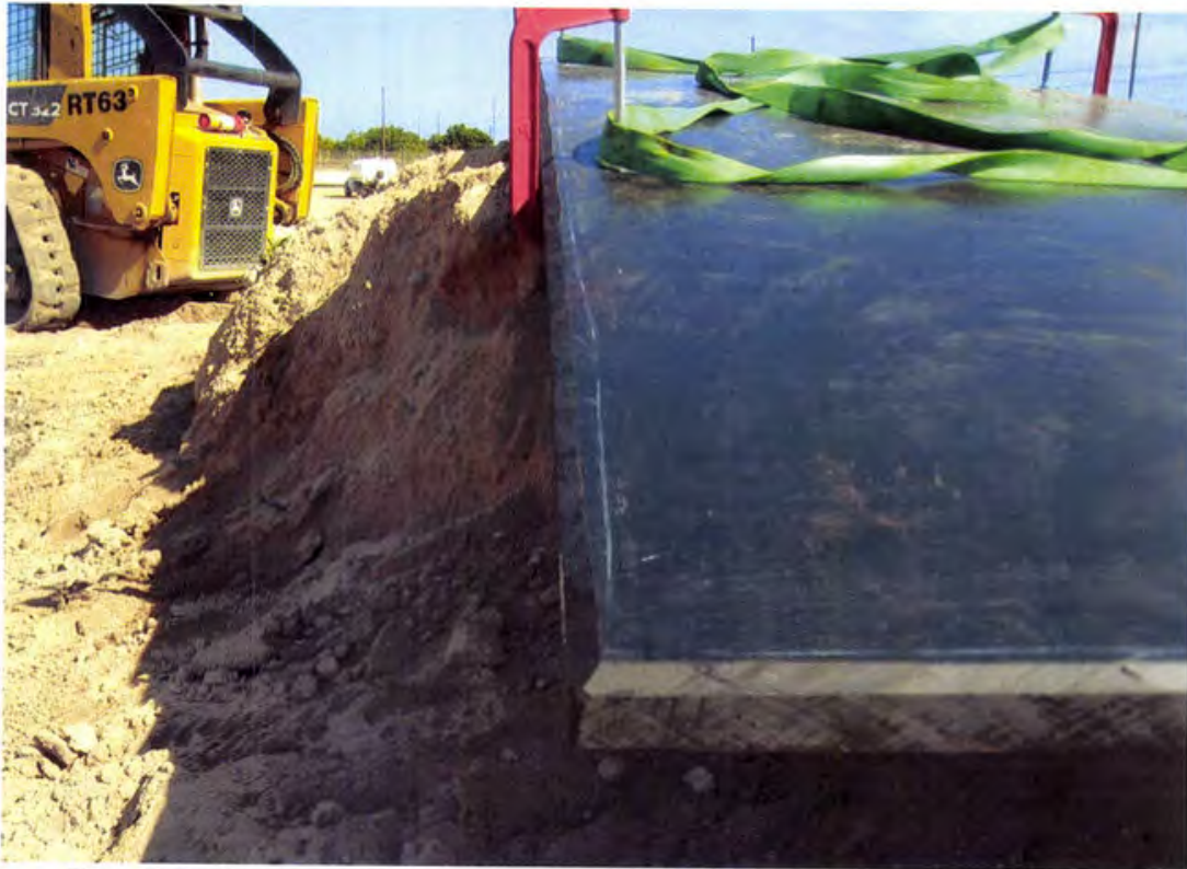
Photo 83. Half-inch chamfers are cut along edges of adjoining 2-inch thick HDPE flatstock panels prior to fillet extrusion welding
