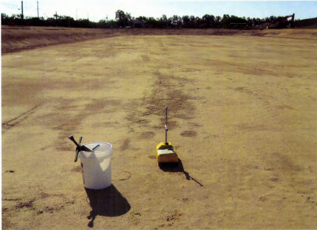
Photo 17. Conducting field density tests of the final subbase compacted fill lift to verify compaction effort (looking east)
