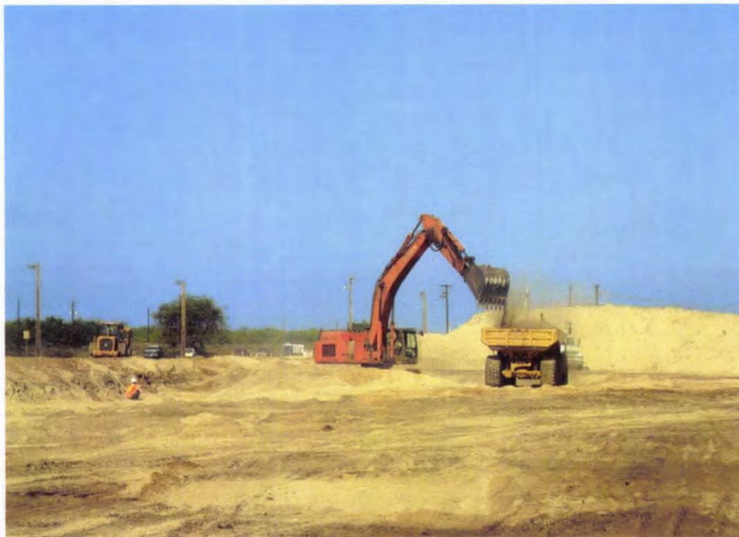
Photo 2. A Hitachi 450 LC excavator is used to excavate the NLEP area to design grades
