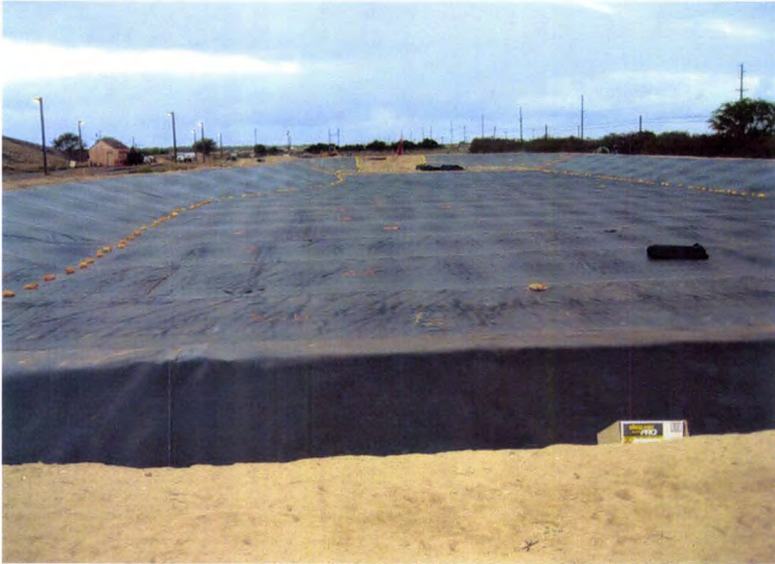
Photo 47. Majority of installed secondary 60 mil HDPE geomembrane
