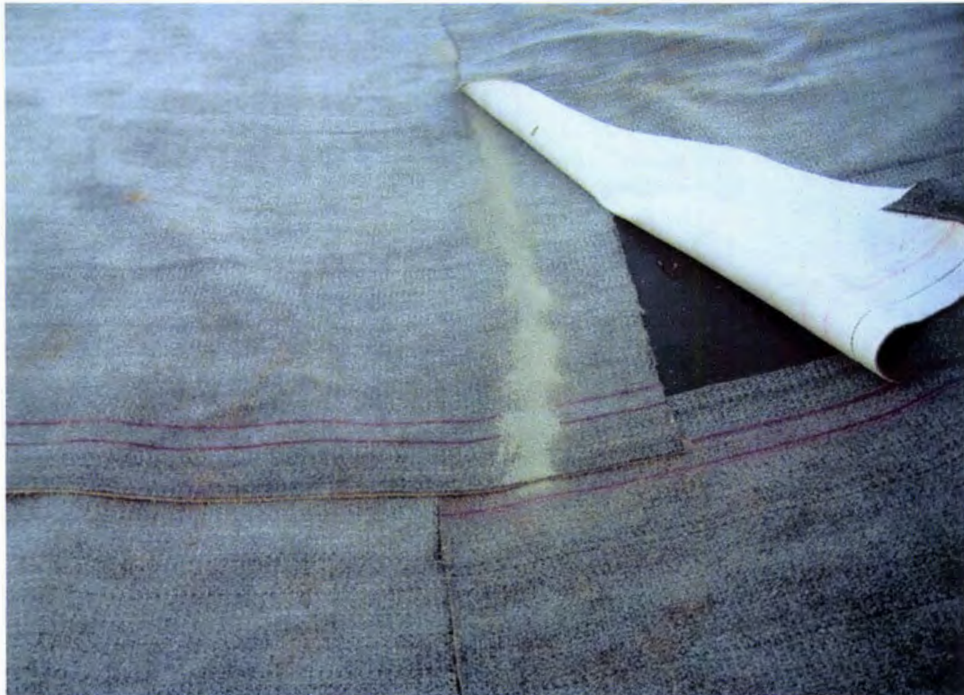
Photo 40. Secondary GCL panels are overlapped 12 inches minimum along the width and 6 inches minimum along the length; granular bentonite is placed along the width (butt) seam
