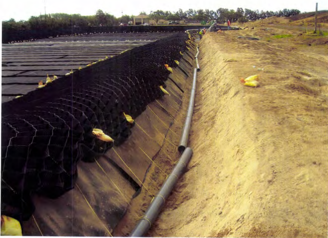
Photo 65. Geoweb System's tendons are tied to a deadman anchor (6-inch PVC pipe) placed within the perimeter anchor trench
