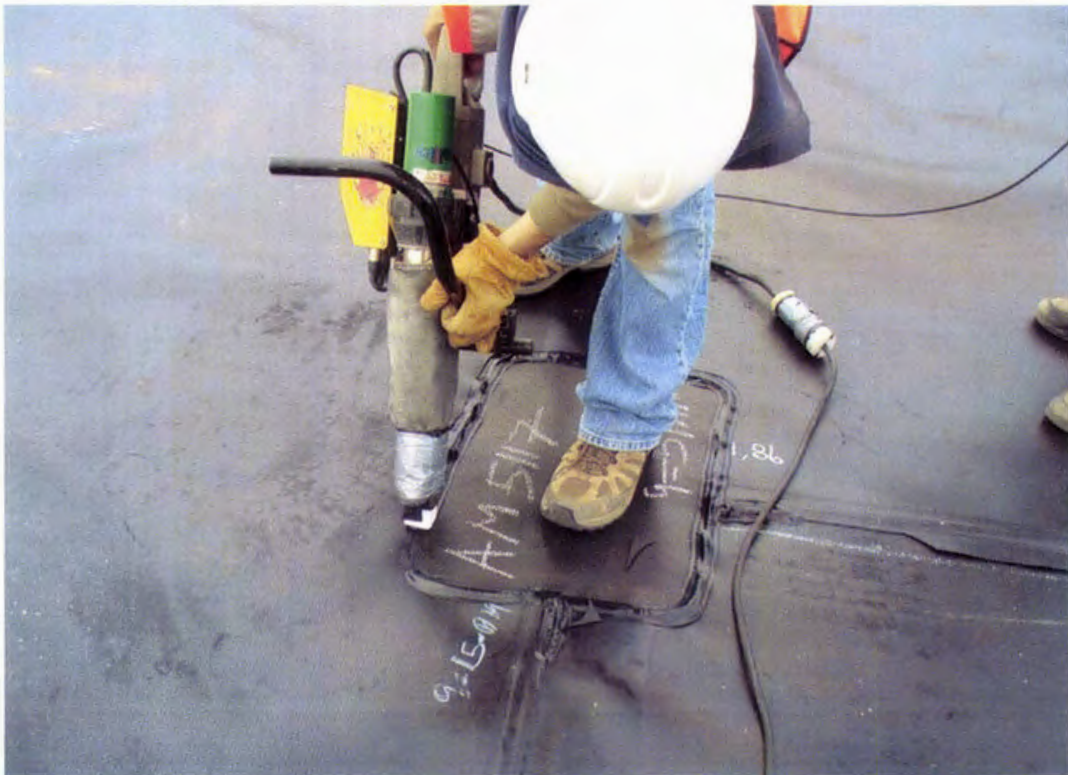
Photo 45. Extrusion welding a repair patch within the secondary 60 mil HDPE geomembrane
