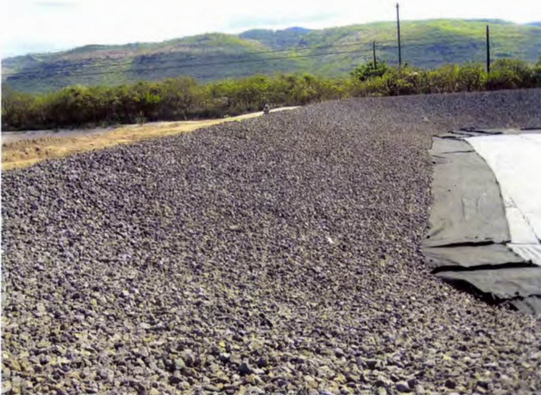
Photo 111. Granular fill installation in the Geocell system is complete on the west slope (looking north)
