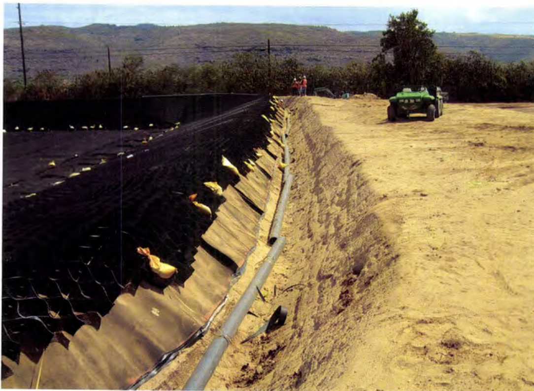
Photo 66. Geoweb System's deadman anchor along the east berm (looking north)
