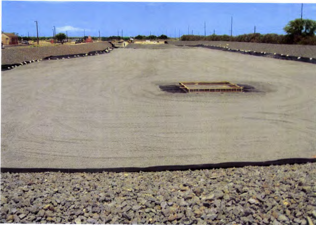
Photo 85. Form boards are constructed over the welded flatstock in preparation for the concrete pad construction. (Aerator Pad 3C shown in front) (looking west)
