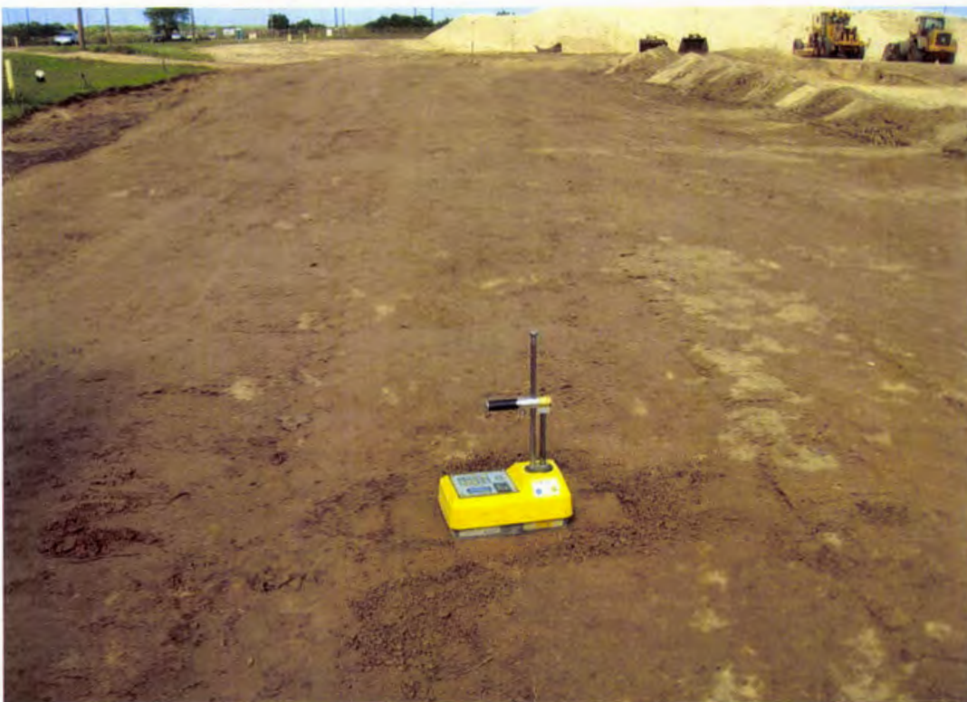
Photo 6. Field density tests using a portable nuclear density gauge to verify compaction effort
