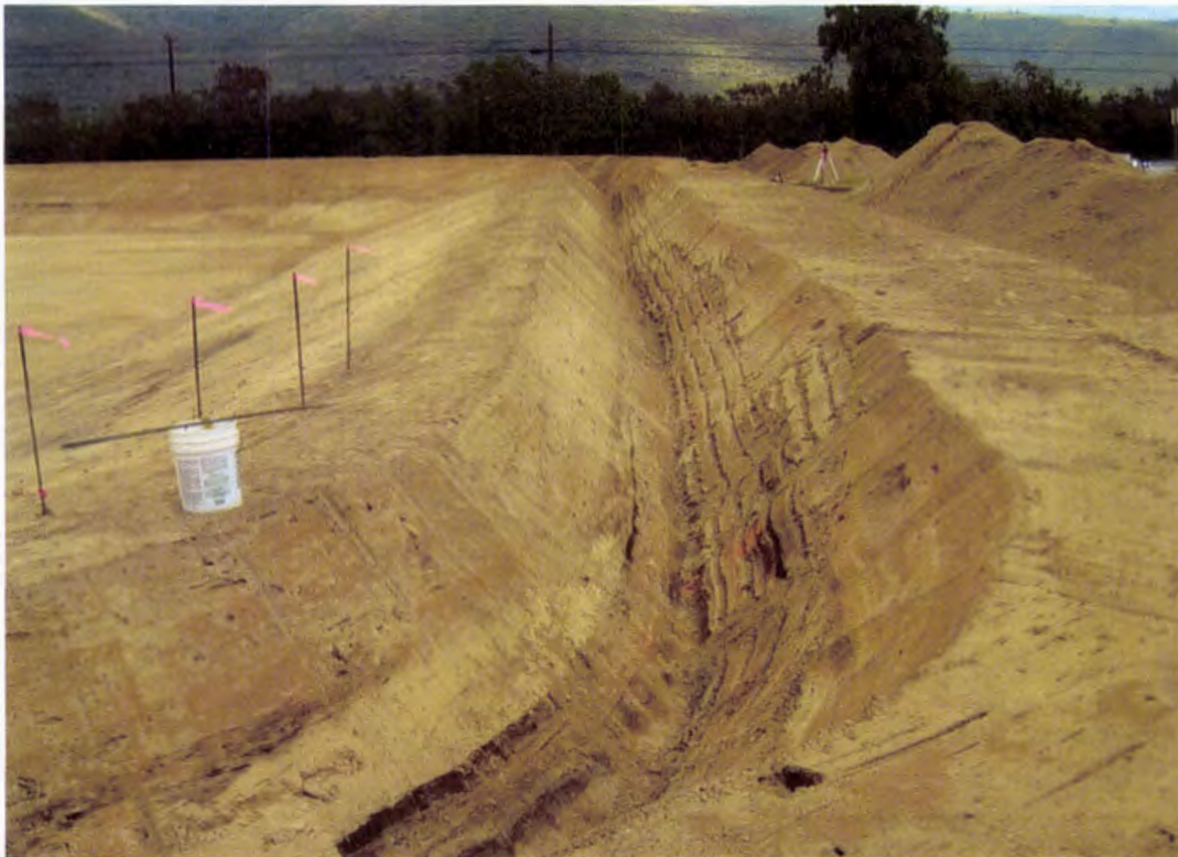
Photo 16. Perimeter anchor trench along the east berm (looking north)
