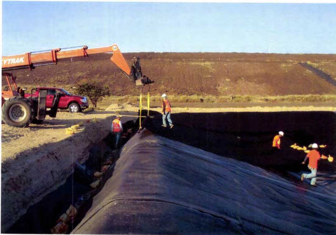
Photo 58. Deploying 16 oz/sy nonwoven cushion geotextile above the completed primary 60 mil HDPE geomembrane (looking south)
