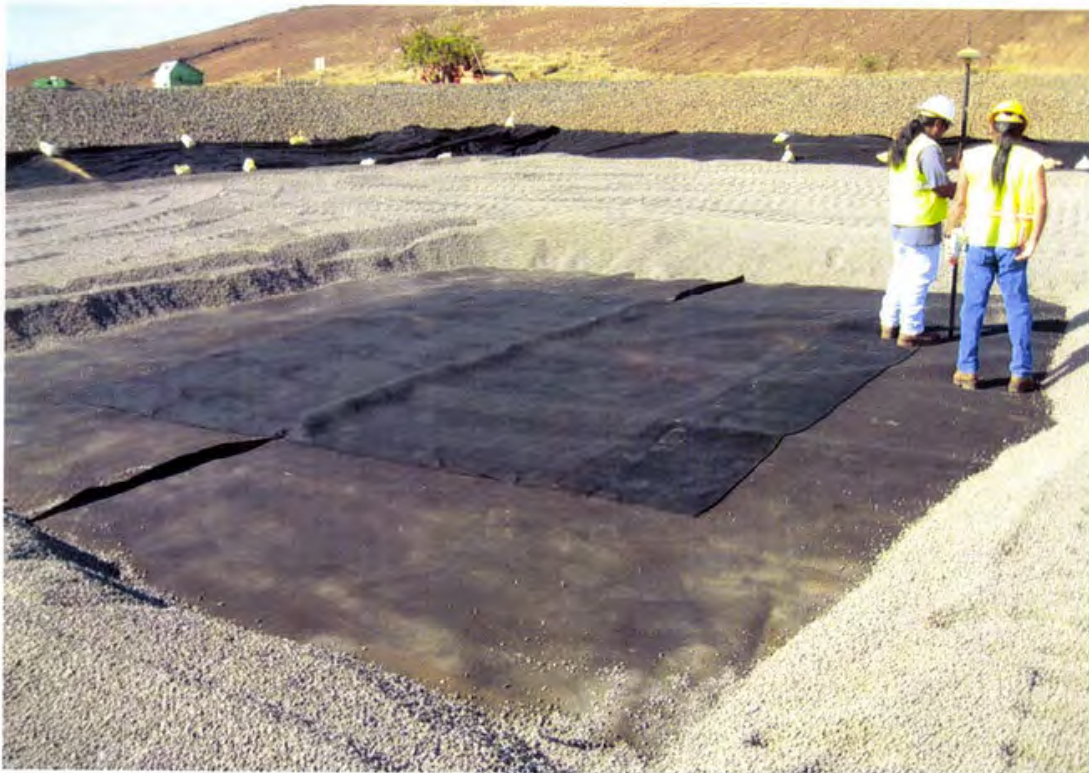
Photo 82. Two layers of 16 oz/sy nonwoven cushion geotextile is placed on the NLEP floor as part of the aerator pad construction
