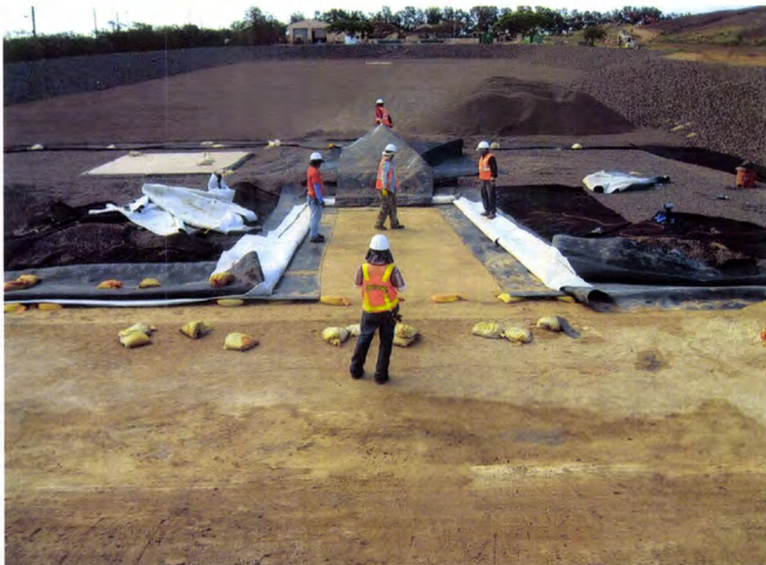
Photo 100. The area of previously damaged geosynthetics within the NLEP floor is removed (looking east)
