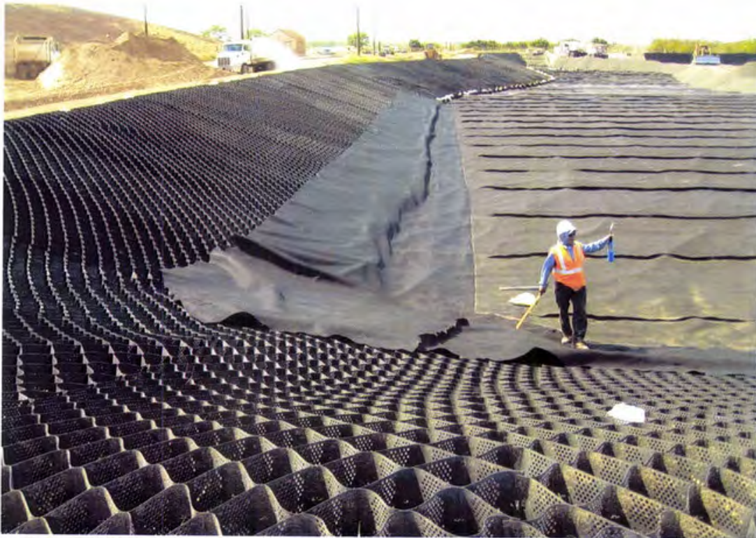
Photo 75. Bottom of perimeter 6 oz/sy nonwoven filter geotextile is heat bonded to the floor cushion geotextile prior to granular operations layer placement against the toe of slope
