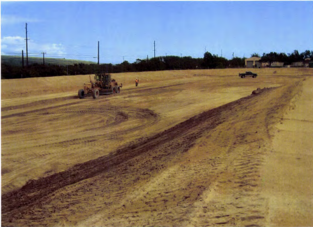
Photo 13. Fine grading the floor subbase using a Caterpillar 140H motor grader with GPS grade control (looking east)
