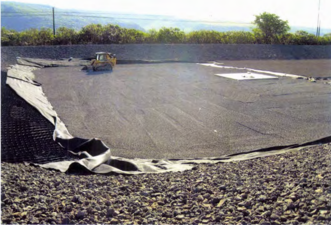
Photo 109. The 1-ft thick granular operations layer is completed over the NLEP floor (looking north)
