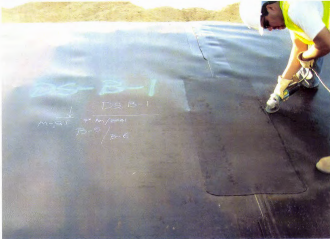
Photo 35. A repair patch is constructed over the destructive seam sample location once the sample is removed; the repair patch is ground along the edges in preparation for an extrusion weld
