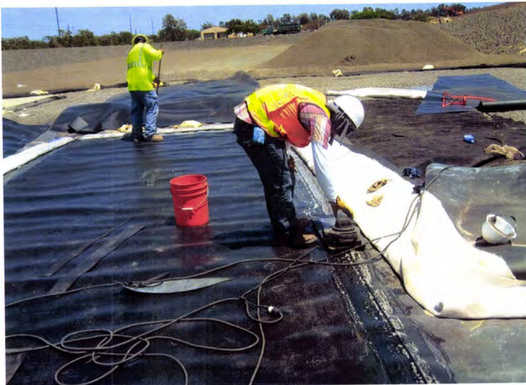
Photo 106. Performing nondestructive vacuum box testing of a primary extrusion weld (looking east)
