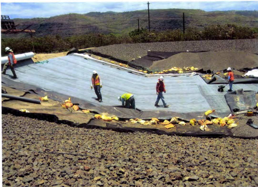
Photo 102. Deploying secondary GCL above the subbase 60 mil HDPE geomembrane (looking north)
