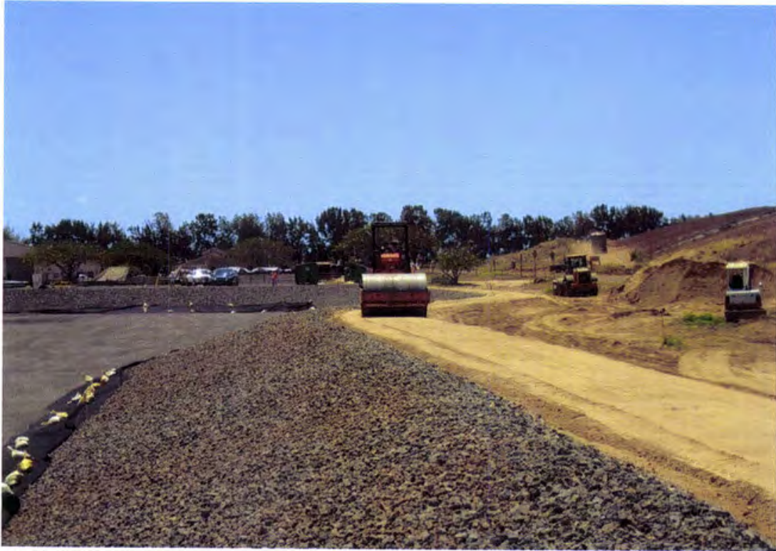
Photo 81. Compacting perimeter anchor trench sand backfill using an Ingersoll-Rand SD122DX rubber tire smooth drum vibratory compactor
