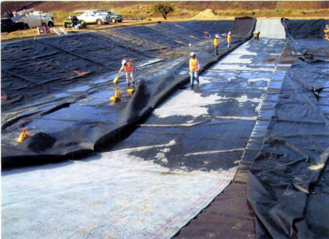
Photo 43. Sudden rains caused several panels of secondary GCL to be prematurely hydrated; per RFI #12, GCL panels shown above had an unacceptable degree of hydration and were removed and replaced with new GCL.
