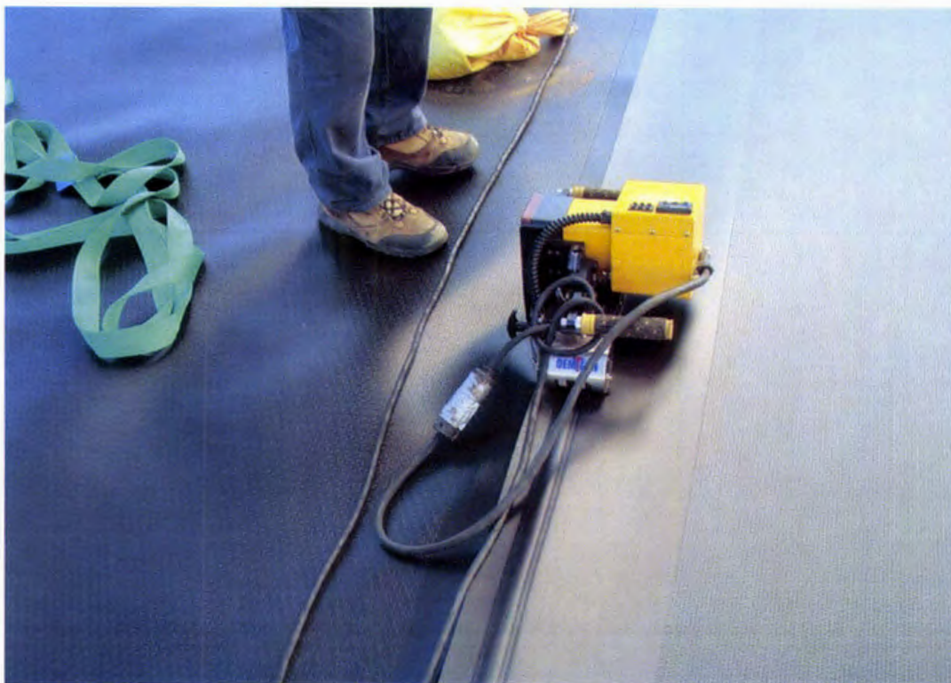
Photo 51. Production seaming primary 60 mil HDPE geomembrane using a double-fusion wedge welder
