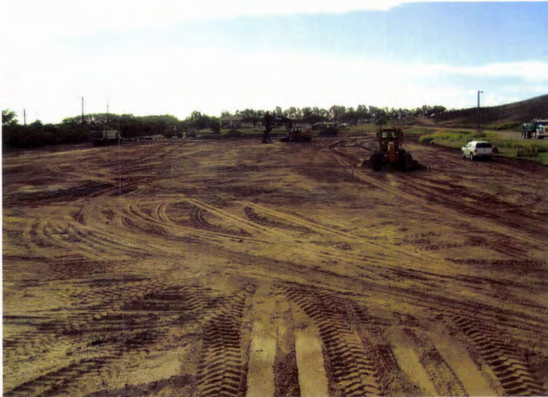
Photo 1. Clearing and grubbing the new leachate evaporation pond (NLEP) area (looking east)
