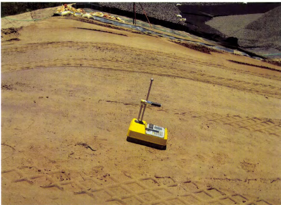
Photo 98. Verifying compaction using a portable nuclear moisture density gauge
