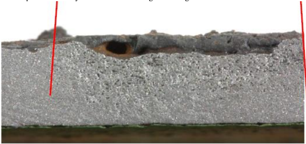
Figure 3: Detail of sandblasted surface. The sandblasting revealed that the feature was not a corrosion pit, as shiny metal was revealed when the red-colored staining was removed.
