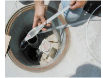
Interstitial monitoring sensor
