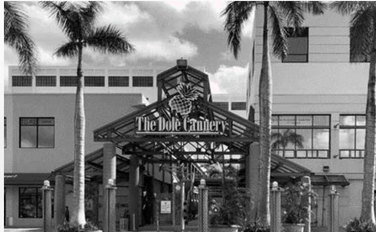
DOLE CANNERY OFFICE BUILDING
