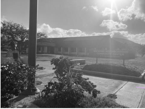
WAI'ANAe SATELLITE CITY HALL TEMPORARY WAHIAWA UNIT 85-670 FARRINGTON HIGHWAY
