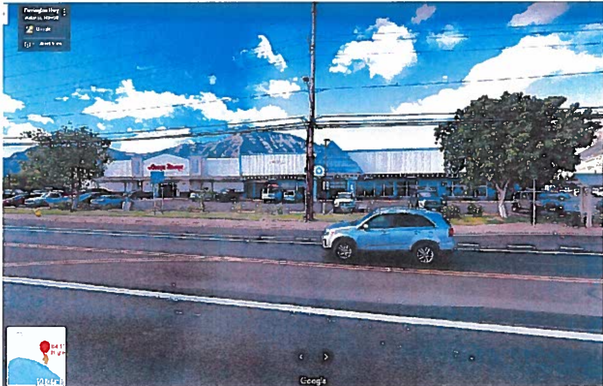
Figure 1 - Google Street View of Property
