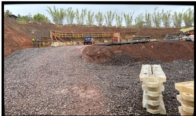
**Project Description:** Demolition of existing reservoir and installation of a 0.5 MG reservoir. Demolition of an existing reservoir and installation of a 0.1 MG reservoir. Additional piping, site clearing and grubbing, retaining walls, paving and site improvements. Installation of a new water line, demolition of an existing water line and relocating existing service laterals. Pipe installation consists of 12-, 8-, 6-, and 3-inch DIP totaling approximately 11,600 linear feet (lf).
