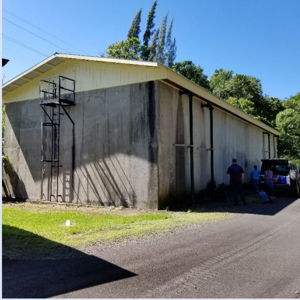
Site #19: Ookala Well Chlorinator
