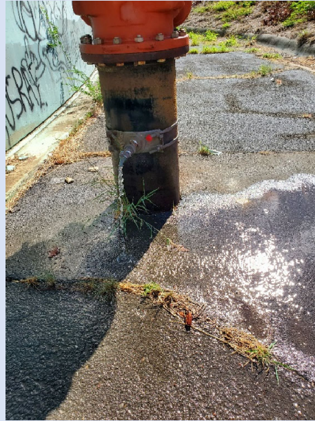
Site #7: Maui Lani Wells Chlorinator
