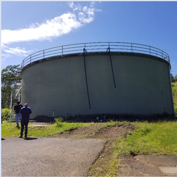
Site #20: Laupahoehoe Wells P1 and P2 Chlorinator
