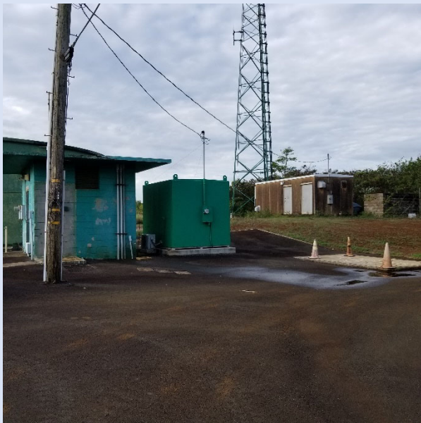
Site #10: Anahola Wells A, B and C Chlorinator
