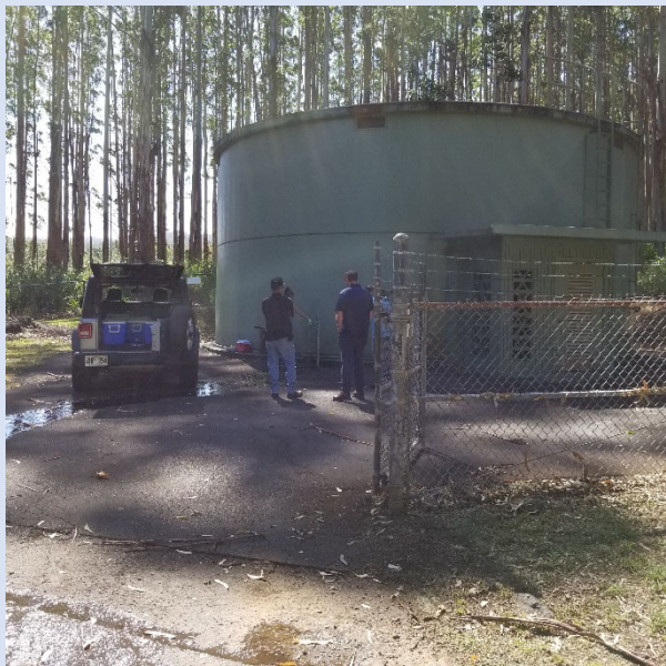
Site #18: Paauilo Wells Chlorinator EPD
