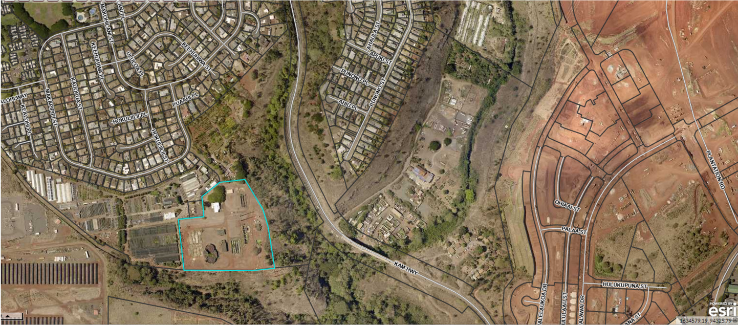
Figure 1.5 - Mililani Preliminary Treatment Facility (PTF) formerly Mililani Sewage Treatment Plant (STP).
