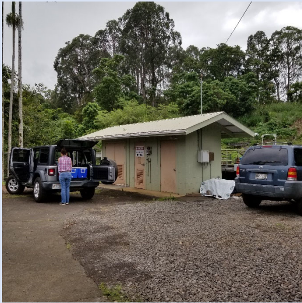
Site #21: Chaves Spring Chlorinator
