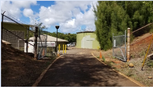
Site #2: Kahuku Wells Chlorinator
