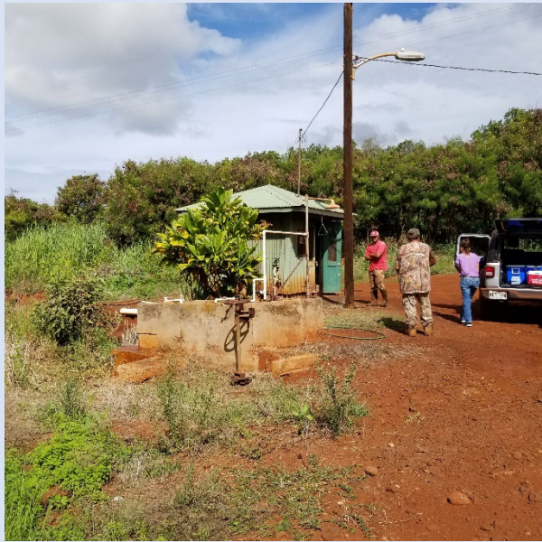
Site #11: Olokele Shaft Chlorinator
