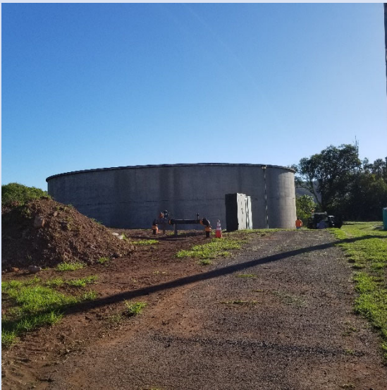
Site 12: Blend of Kauluwai Wells Chlorinator
