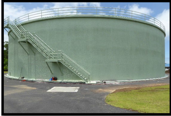
▲ New 2.0 MG tank
