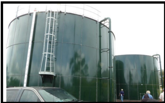
↗ New 228k-gallon steel tanks
