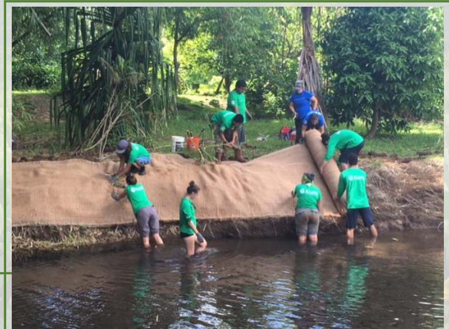
Waipa Stream stabilization and restoration/Matt Rosener
