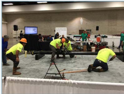
The HBWS Pipe Tapping team gets to work to try and repeat.
