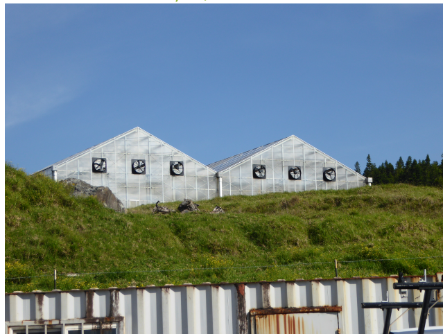
WAIMEA WTP SLUDGE DRYING BEDS (HDWS SOUTH KOHALA). $3.5M LOAN
