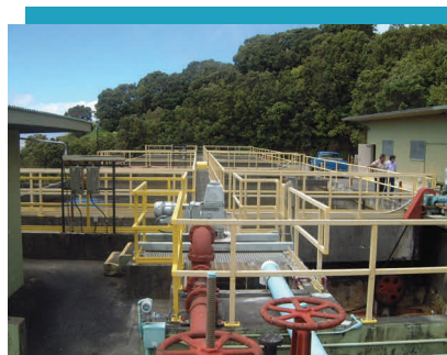
Waimea Water Treatment Plant headworks
