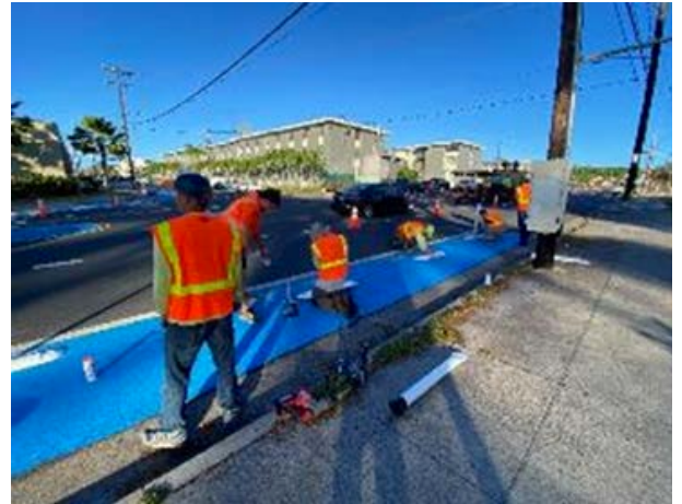
Figure 1: volunteers installing delineators
