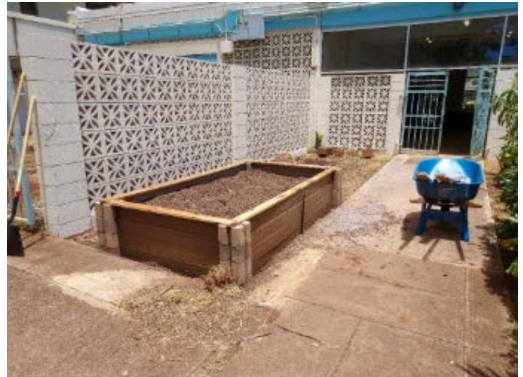
Accessible garden boxes built at HPHA site Kalanihulia in September 2023.
