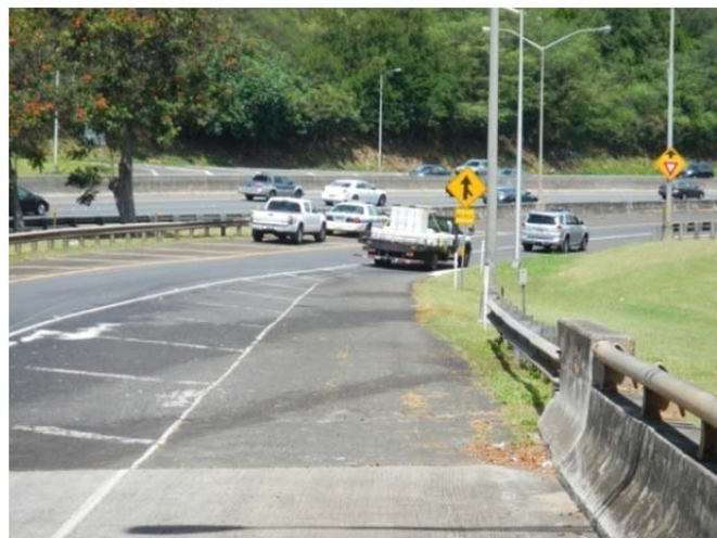
Chemical Spill on Moanalua Freeway On-Ramp
