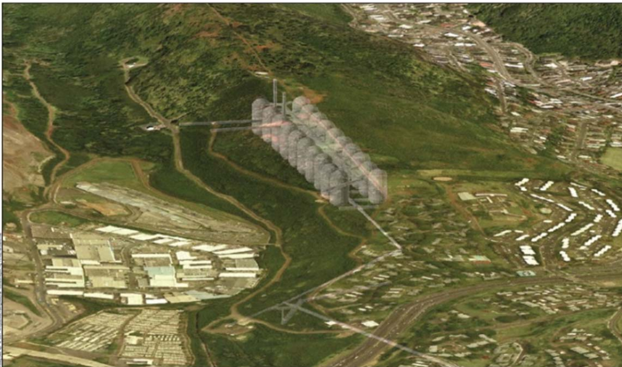
Figure 1-3 Red Hill Tanks and Surrounding Infrastructure Red Hill Fuel Storage Facility Oahu, Hawaii
