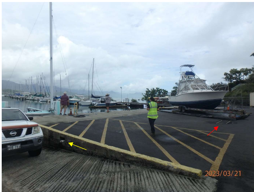
Photograph 5: View of the Facility's Maintenance Area and discharge pipe (yellow arrow). Note: sediment trap (red arrow) connects to the discharge pipe. Photograph March 22, 2023 by Jacquelyn Corpus.
