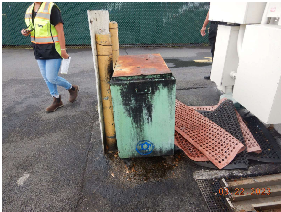
Photograph 13: View of used cooking oil from kitchen fryers, spilled on the ground near the southeast corner of the main building. Photograph taken March 22, 2023 by Bobbie Teixeira.
