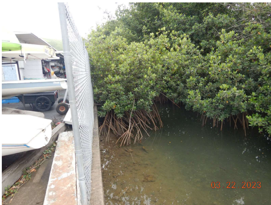
Photograph 2: View of City and County of Honolulu canal located on the southern perimeter of the Facility. The canal connects to Kaneohe Bay. Photograph taken March 22, 2023 by Bobbie Teixeira.
