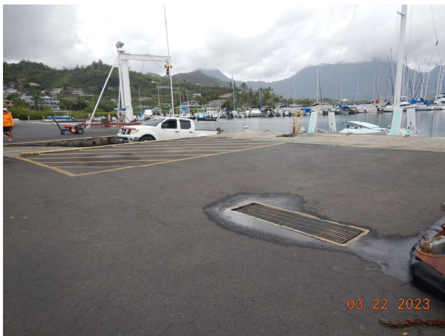
Photograph 6: Closeup view of sediment trap in Photograph 5. Photograph taken March 22, 2023 by Bobbie Teixeira.
