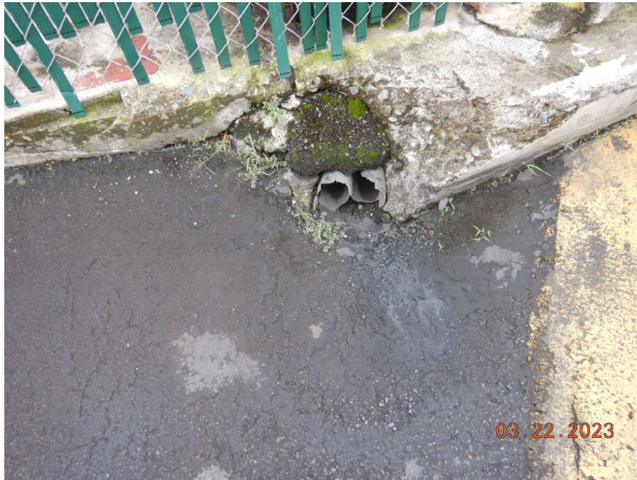
Photograph 15: Close up view of discharge pipes in Photograph 14, leading to City and County of Honolulu's canal on the southern perimeter of the Facility. Photograph taken on March 22, 2023 by Bobbie Teixeira.
