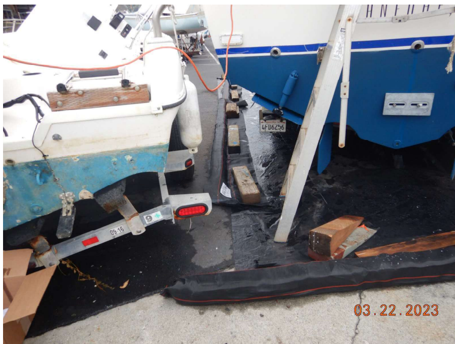
Photograph 10: View of gap in containment. Photograph taken March 22, 2023 by Bobbie Teixeira.
