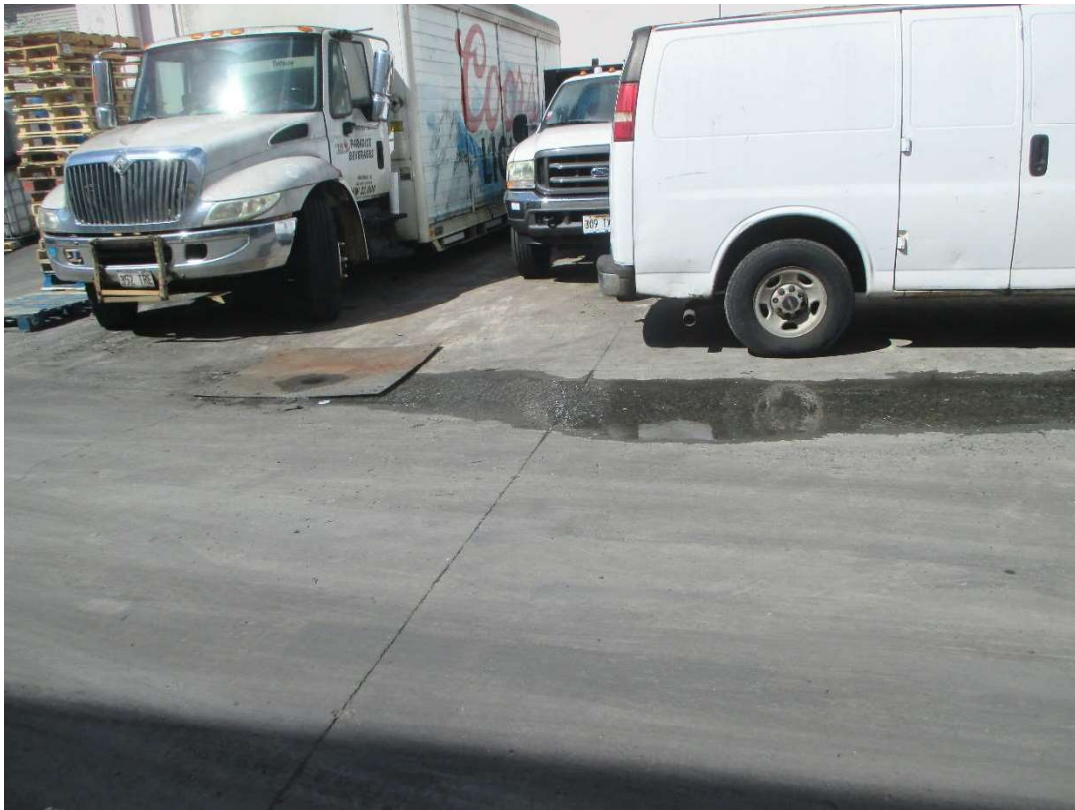
Dry weather flow with alcohol odor entering private inlet which initially discharges to a City and County of Honolulu (CCH) 84-inch reinforced concrete pipe (RCP).
