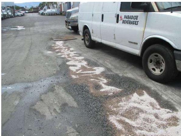
TMK: 9-4-128:002: At approximately 1:50 PM, the property was informed of the illicit discharge and washing operations were immediately halted. Absorbent material was laid down along the dry weather flow to contain the discharge. (IMG_011)
