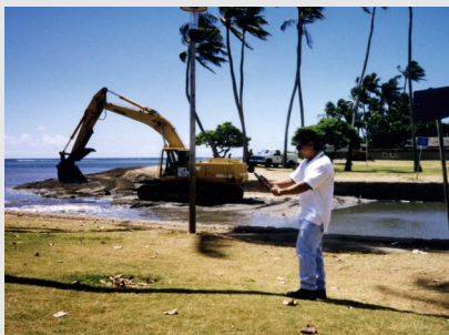
Monitoring construction noise
