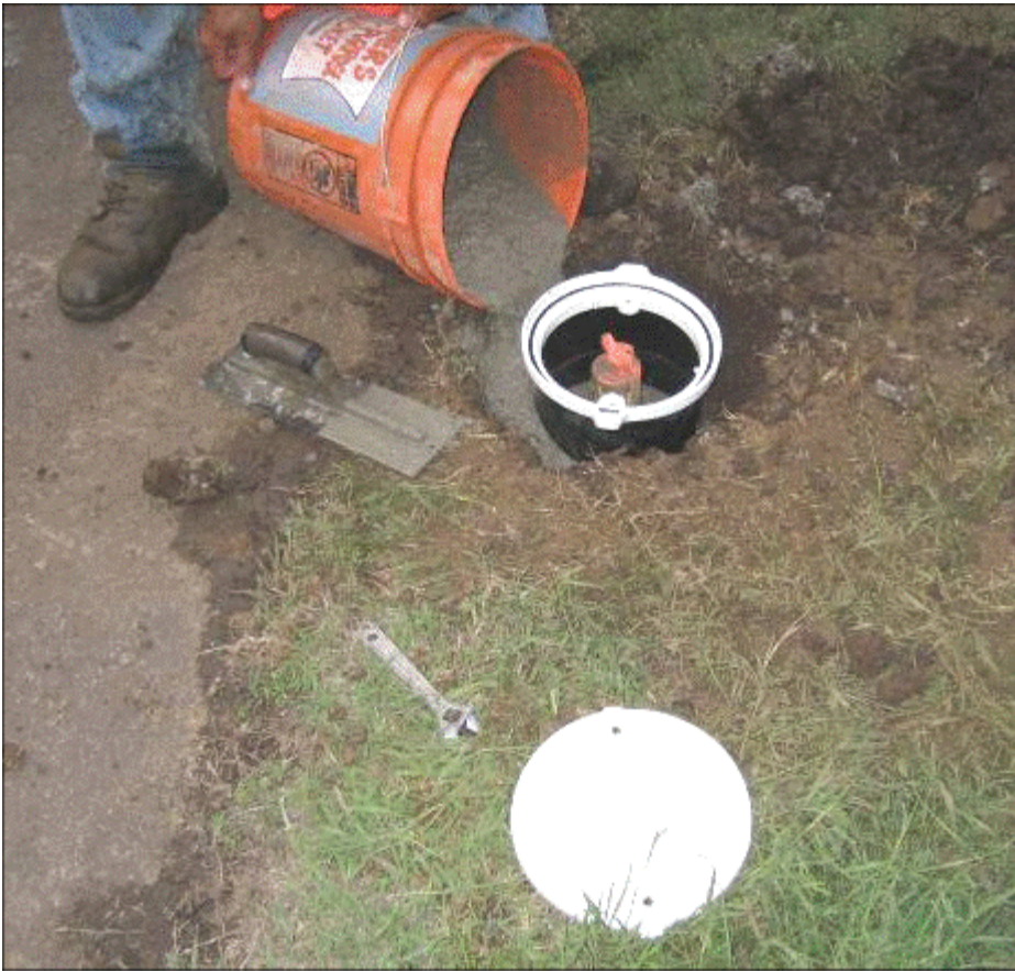
Figure 6-16. Installation of Well Head Protection
