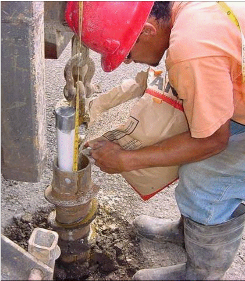
Figure 6-15. Hollow Stem Auger with PVC Well Casing.
