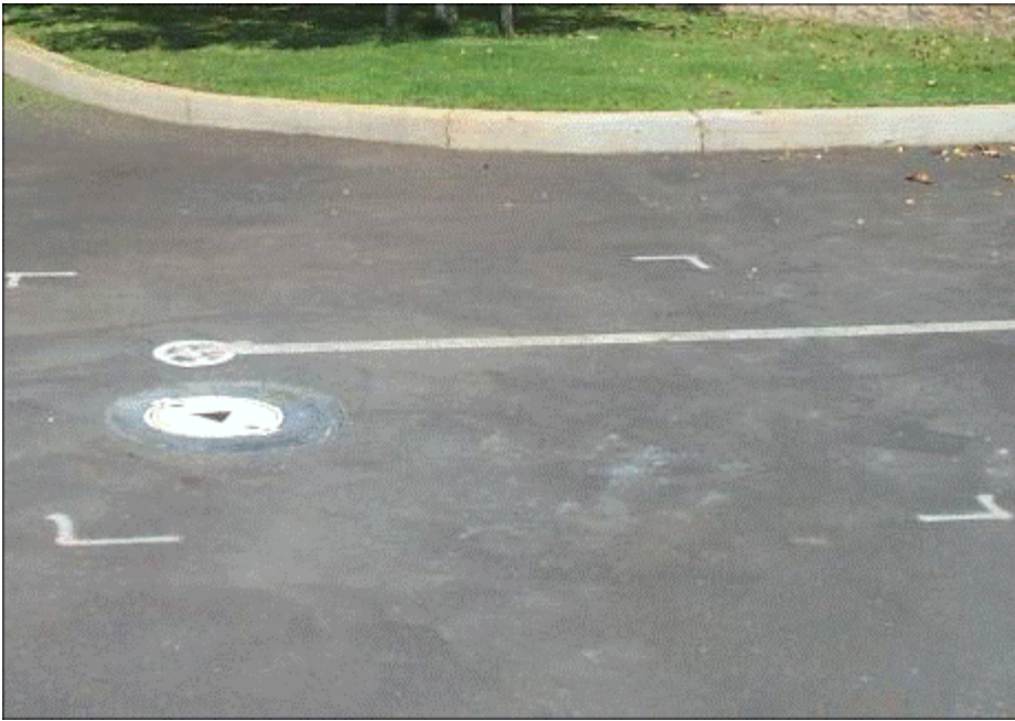
Figure 6-17. Flush-mounted well head box installed in a parking lot
