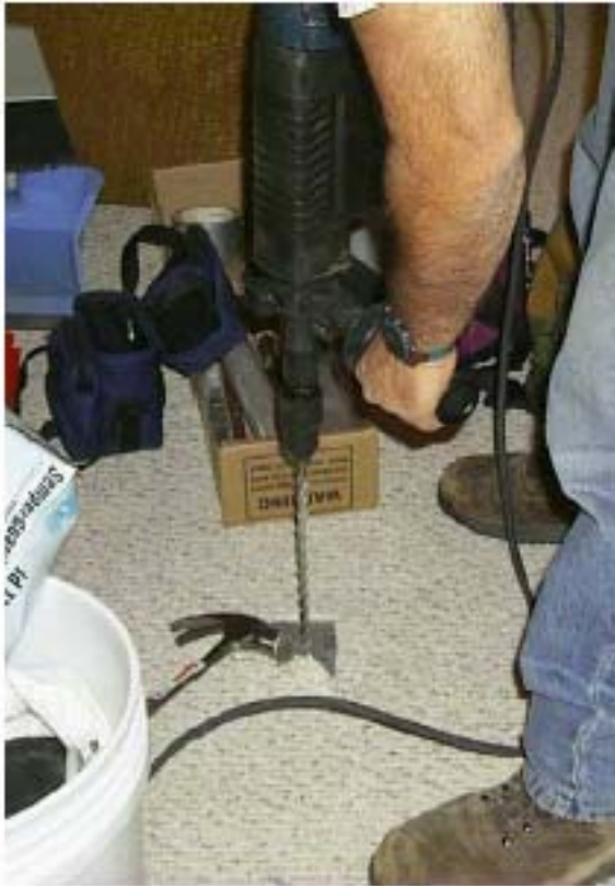
Figure 1. Drilling through a slab
