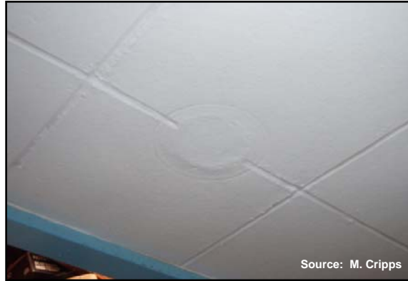
Canec ceiling panels with characteristic V-shaped groove joints.
