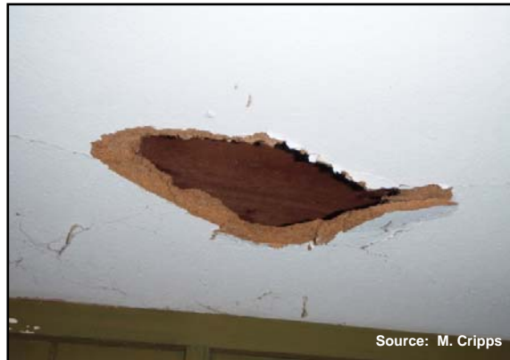
A canec panel that is broken. Note the characteristic fibrous texture and brownish color.
