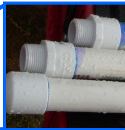
b) Screw ends attached to cut PVC, with solid cap on end of one piece (keeps water out).
