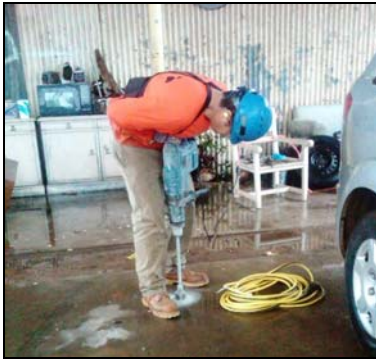
g) Coring through concrete for collection of subslab increments.
