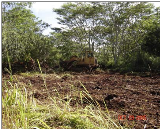
b) Clearing of 5,000ft 2 DU area for collection of MI soil sample (photo from Bureau Veritas).
