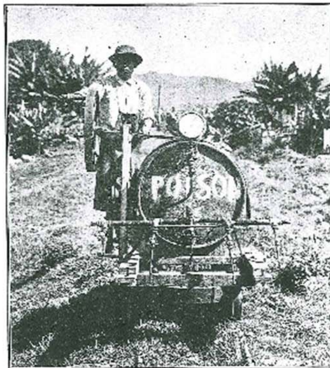
Fig. 3. Railroad Sprayer used at Kilomea.
