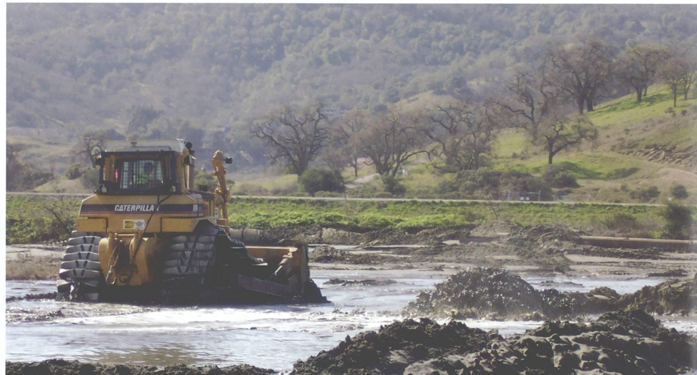
A bulldozer spreads dredged mud at the Hamilton Field wetland restoration site in Marin County, California.
