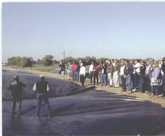
This covered lagoon is part of a new biogas energy system funded by the California Energy Commission at Joseph Gallo Farms, a dairy in Atwater, Calif. The decomposing manure creates biogas—primarily methane and carbon dioxide—which is piped to generators and burned to generate 700 kW of electricity.
