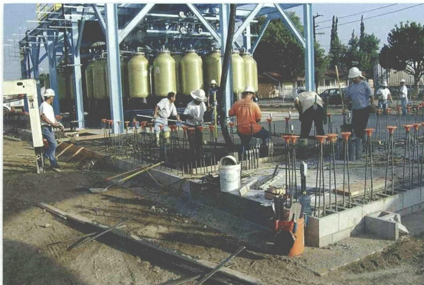
Ground water treatment plant under construction in the San Gabriel Valley.
