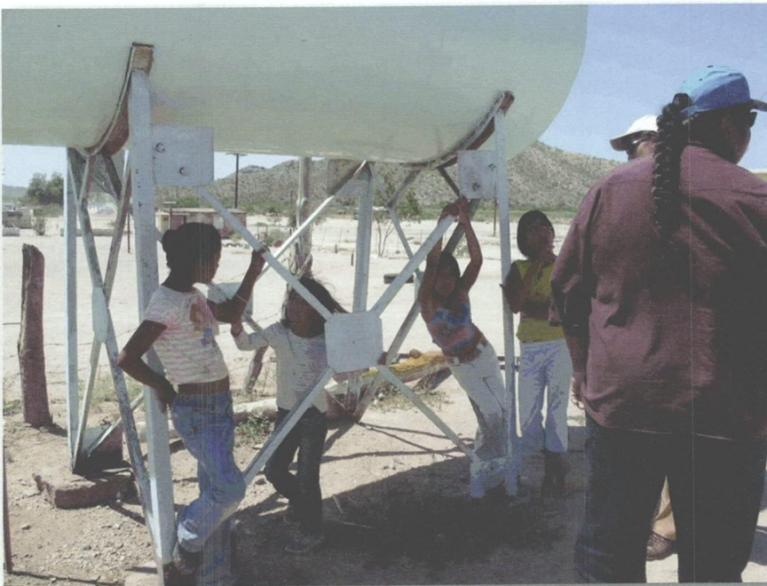
Water supply tank at the Quitovac Tohono O'odham Community in the U.S.-Mexico border region.
