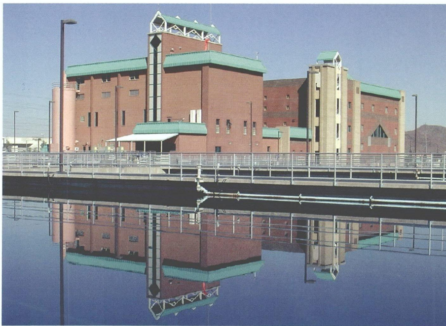
The Deer Valley Water Treatment Plant is one of Phoenix’s facilities for purifying drinking water.
