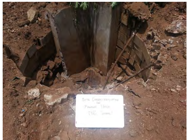
Photo 30. DU1, Test Pit 7 undocumented cesspool.
