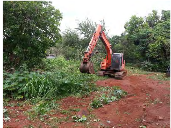
Photo 2. DU1: Clearing vegetation by trampling with excavator. No grubbing performed.
