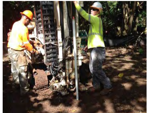
Photo 40. Drilling/installing temporary monitoring well.
