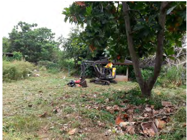
Photo 4. DU2: Clearing vegetation by trampling with mini excavator. No grubbing performed.
