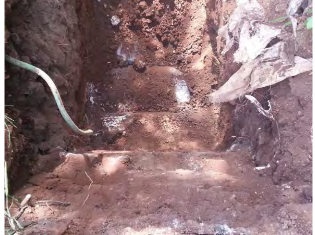
Photo 26. DU3, Test Pit 1 Debris and potential concrete pipe at bottom of test pit.
