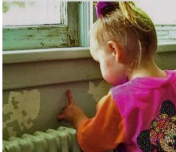
Lead-based paint is still present in many homes in Hawai'i. Children are at risk from eating paint chips and flakes. The paint chips can also fall off the house exterior and get in the soil adjacent to the foundation where children may play.
