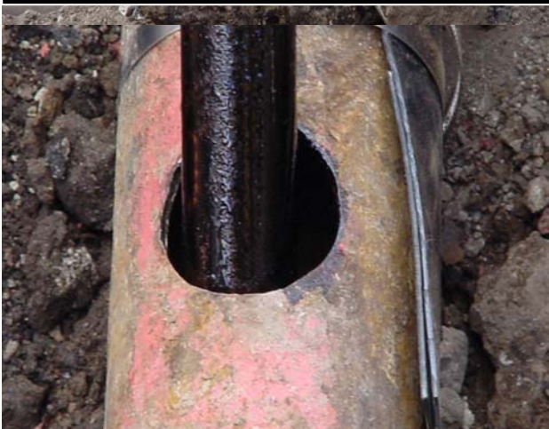
Tapped Pipeline Oil Recovery
