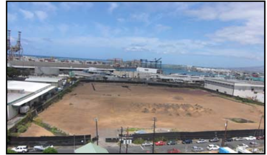
Top – Soil excavation and treatment.
