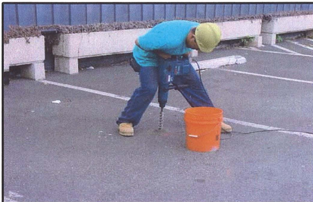
Photograph 1: View of passive soil vapor boring advancement.
