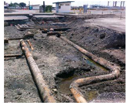
Buried Pipes in Iwilei
