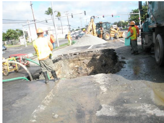
Emergency Utility Repair
