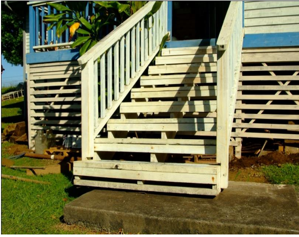
Above : Post-and-pier construction home and the storage space under a post-and-pier construction home.
