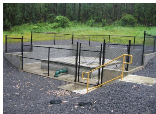
Photo 10b: Completed DWSRF Project
