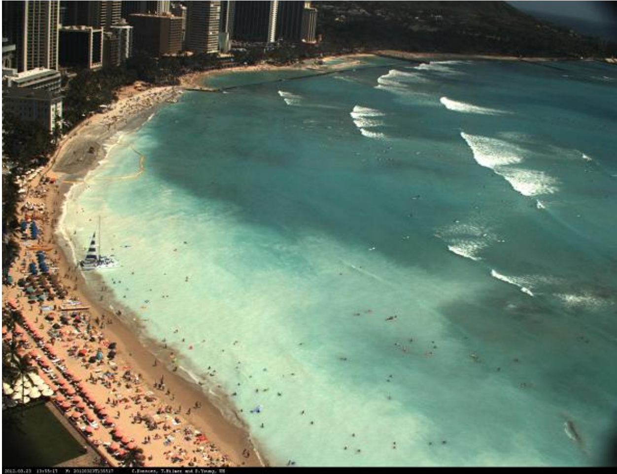
Photo 6: View of Waikiki during the beach replenishment project
