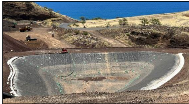
Figure 5 — Leachate Basin Adjacent to Ash and Debris Storage Area
