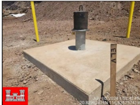
Figure 7 —Groundwater Monitoring Well at TDS Site
