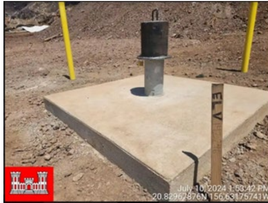
Figure 7 —Groundwater Monitoring Well at TDS Site
